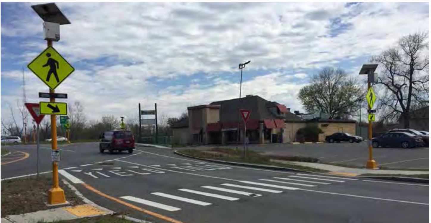
Rectangular Rapid Flash Beacons installed at the rotary are within 100' of the traffic signal and may pose a danger to pedestrians.
