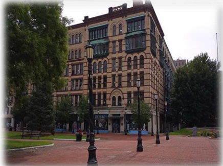
31 Elm – Work Has Begun!
