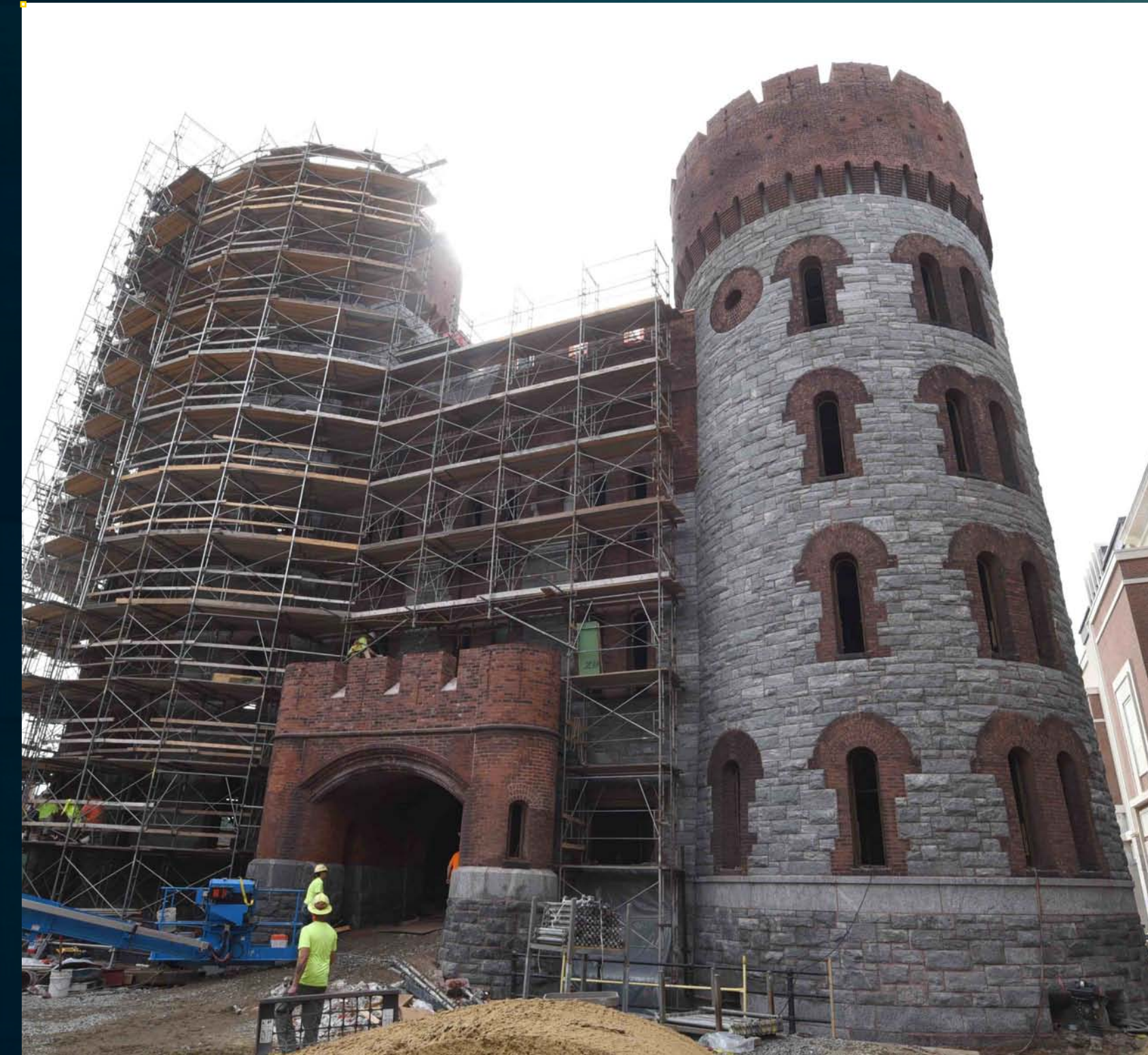
Armory Progress - June 20, 2018
