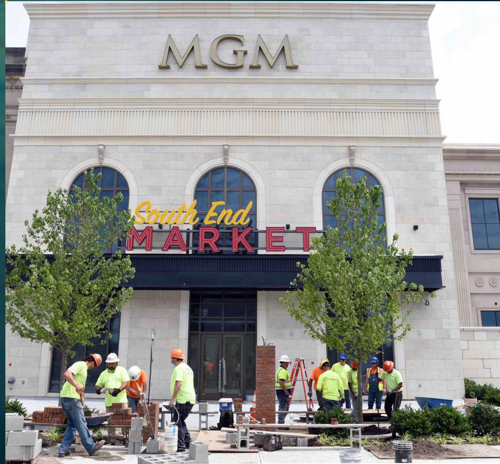
Podium Exterior - June 20, 2018
