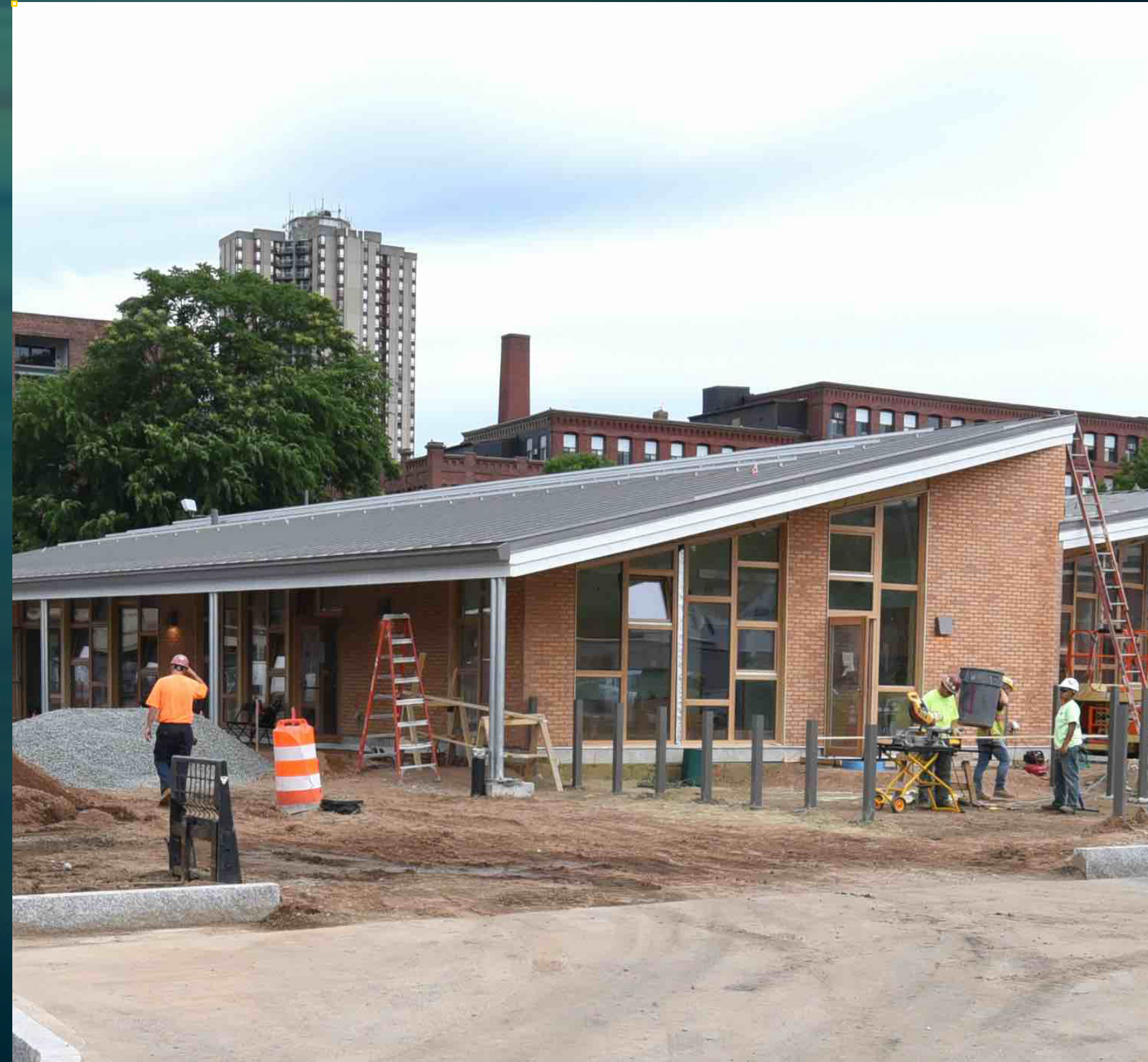
Daycare Progress - June 27, 2018
