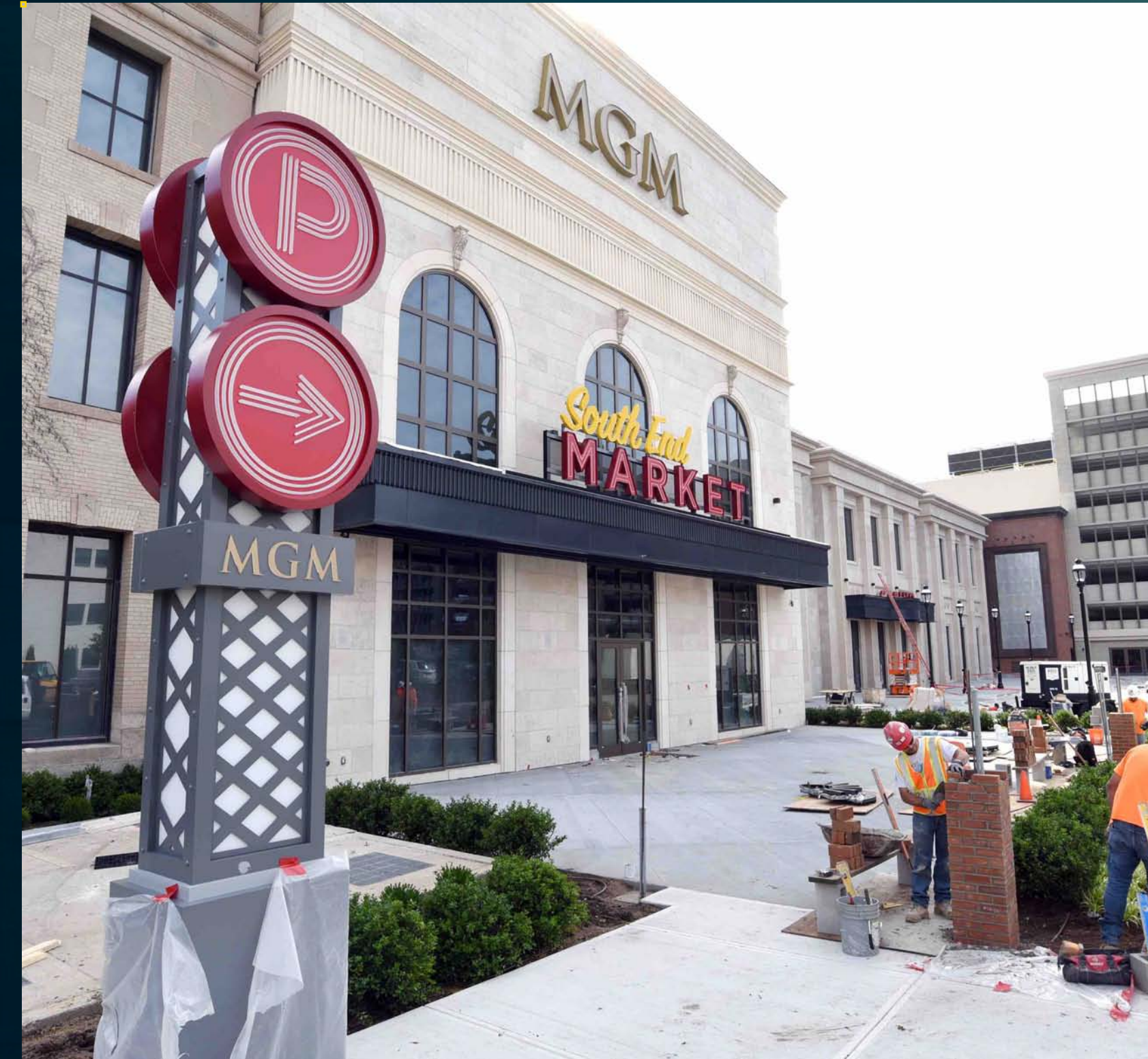
Podium Exterior - June 20, 2018
