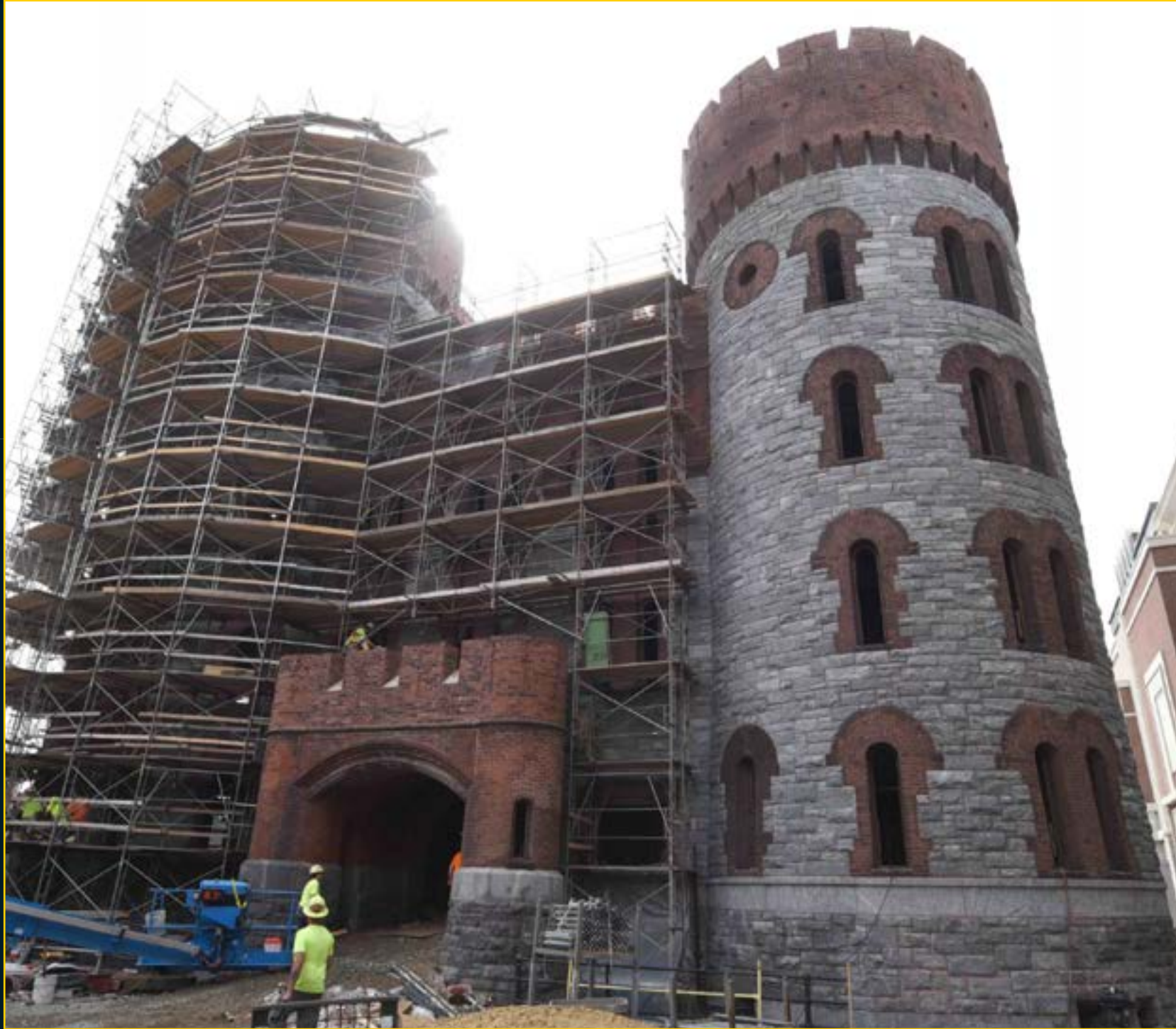
Armory Progress - June 20, 2018
