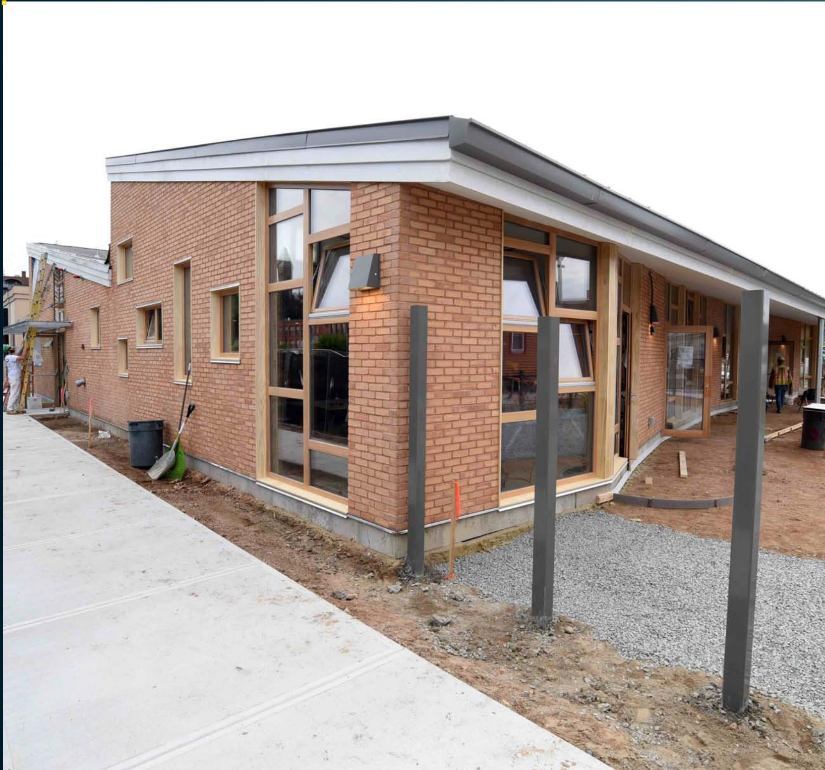
Daycare Progress - June 27, 2018
