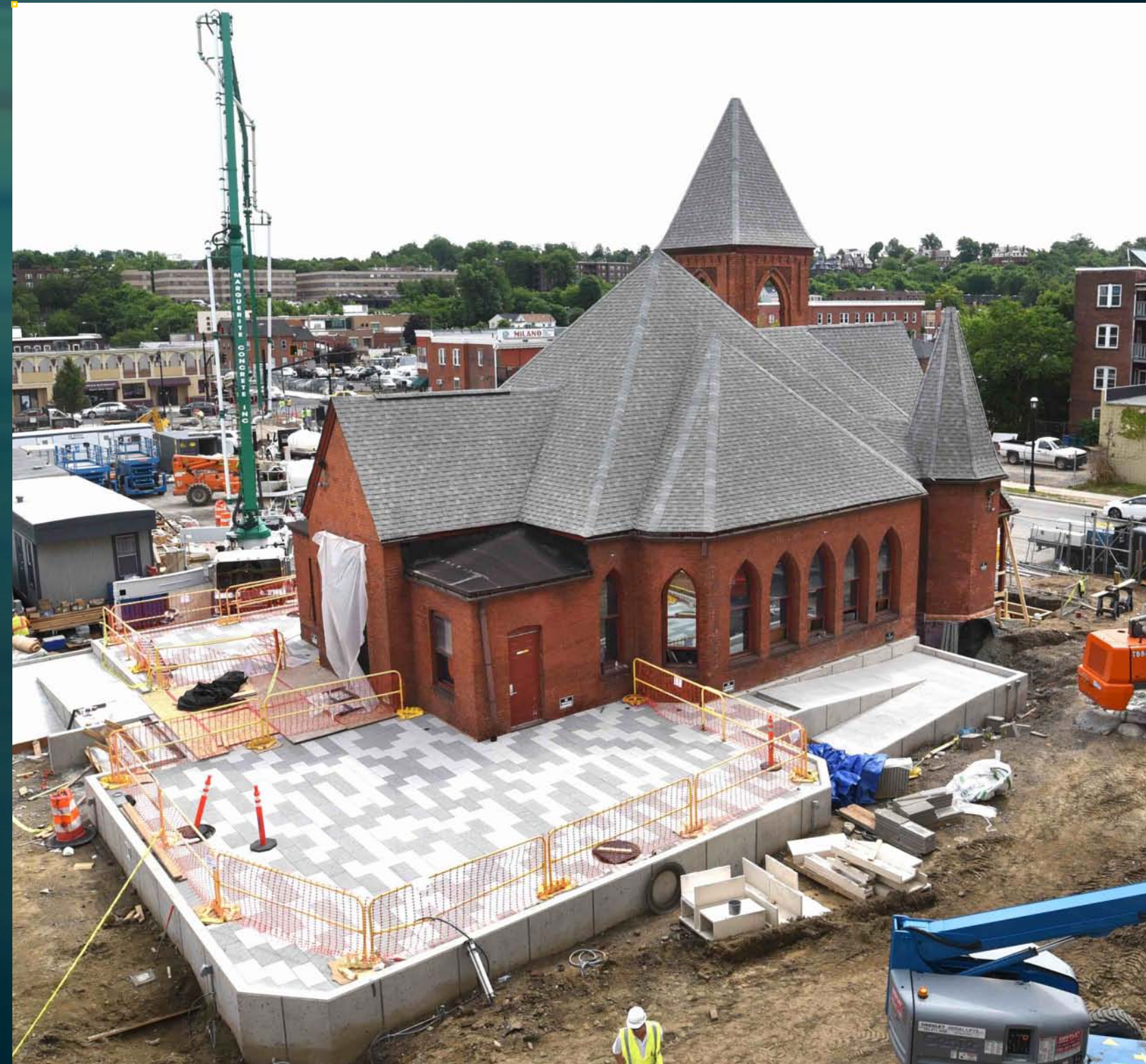
Church Exterior Progress - June 20, 2018
