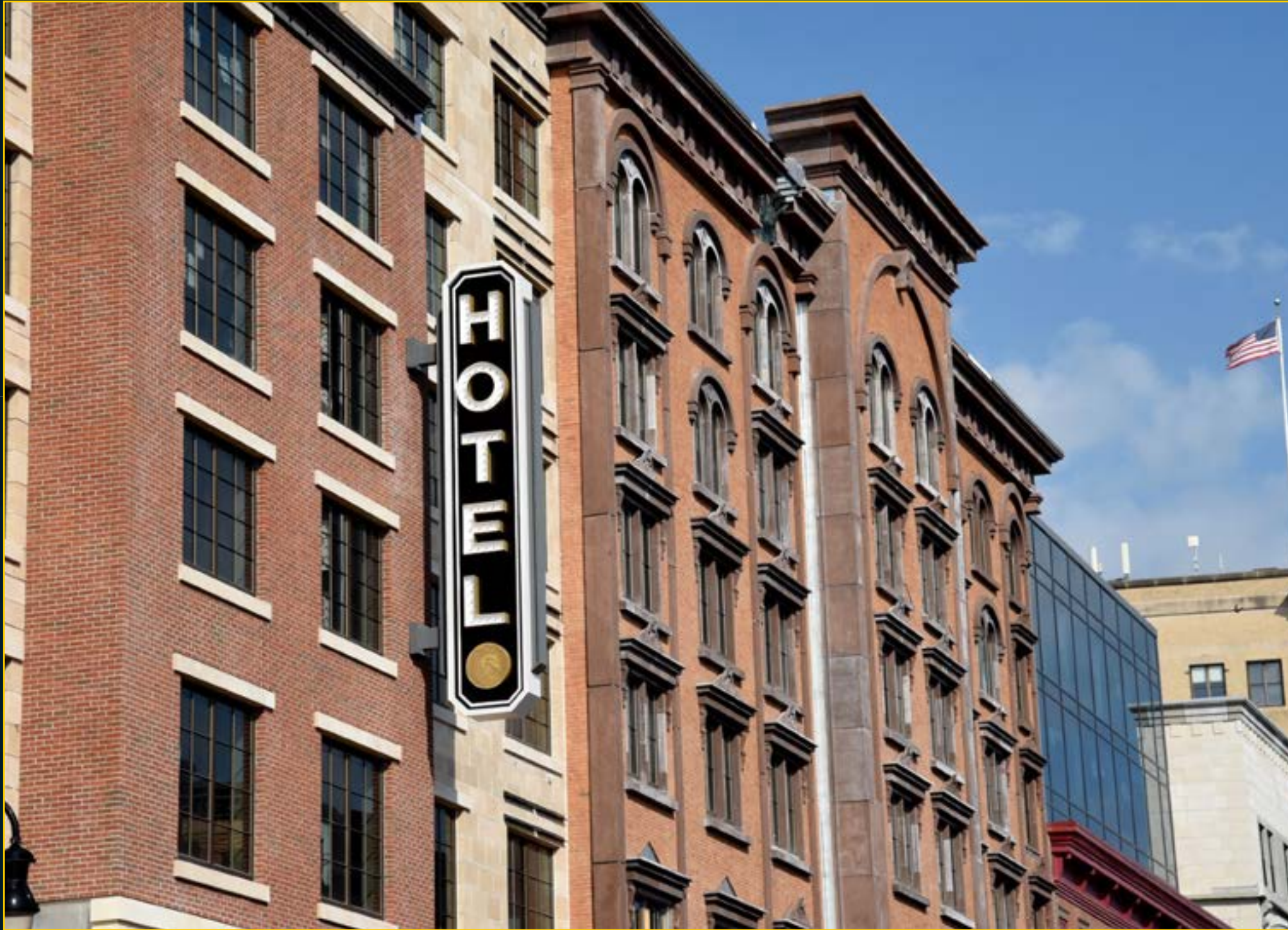
Hotel Exterior - May 30, 2018
