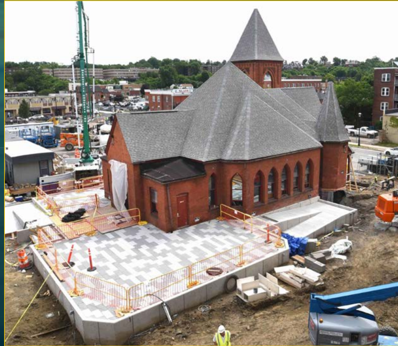
Church Exterior Progress - June 20, 2018
