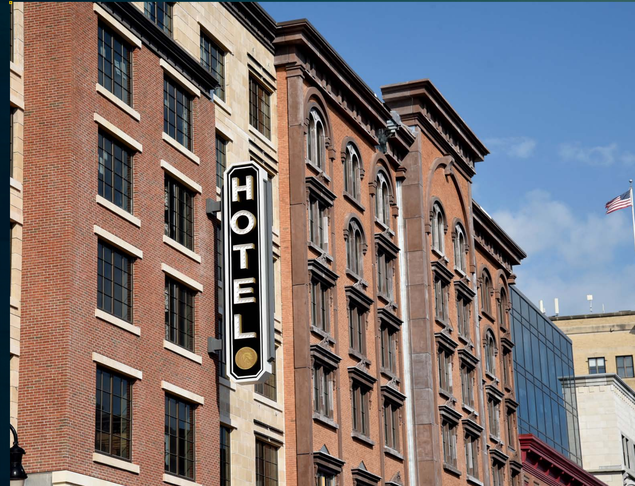
Hotel Exterior - May 30, 2018
