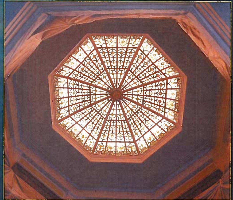
73 State Street Dome Construction
