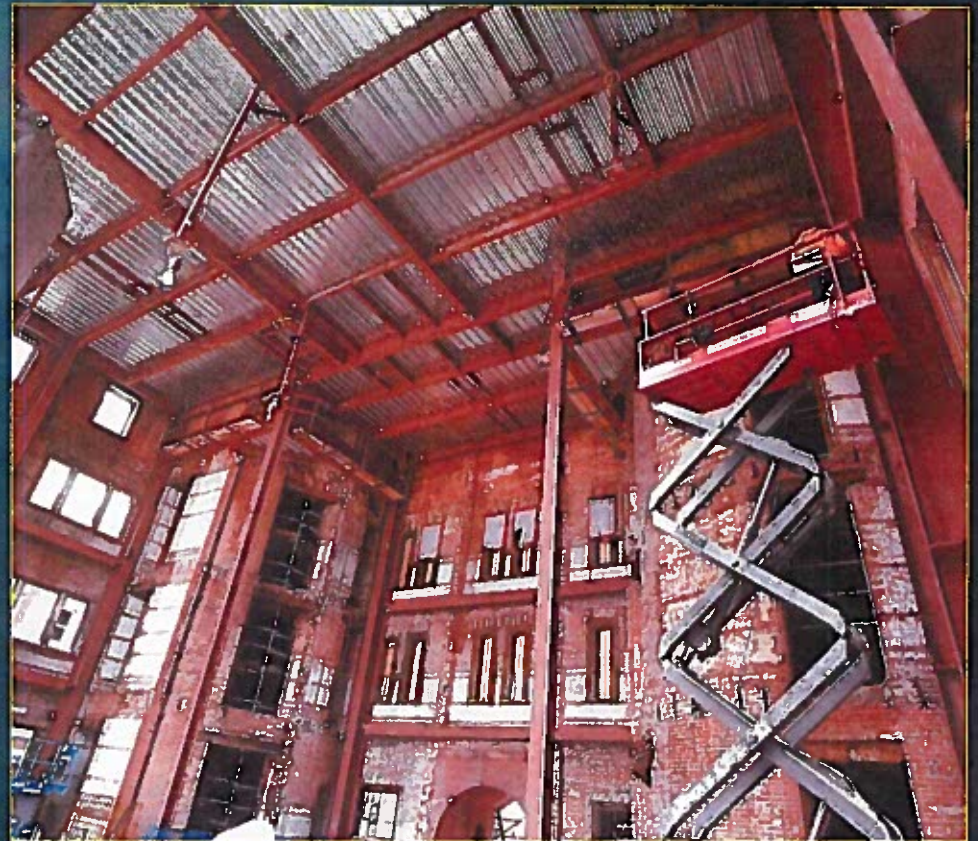
Armory Interior Construction
