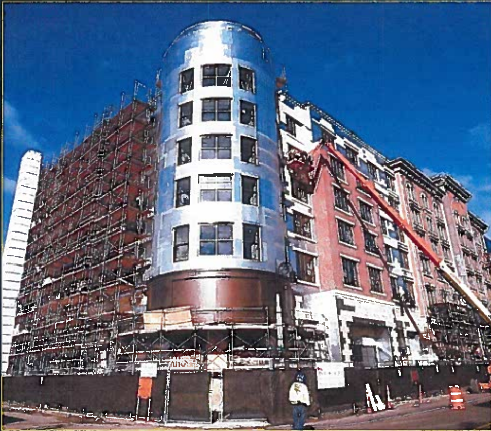
Main Entrance Construction
