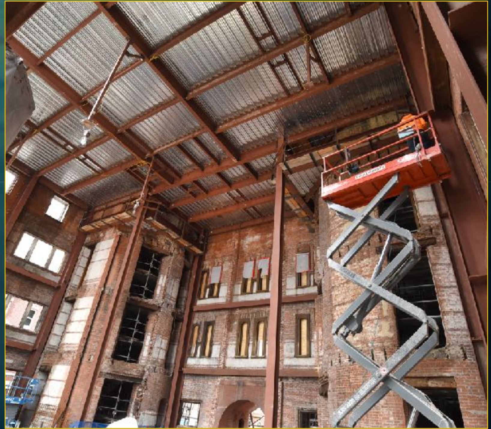
Armory Interior Construction
