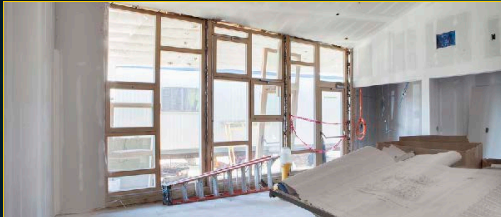
Early Childhood Center Construction
