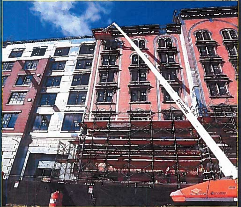
Main Street Facade Construction
