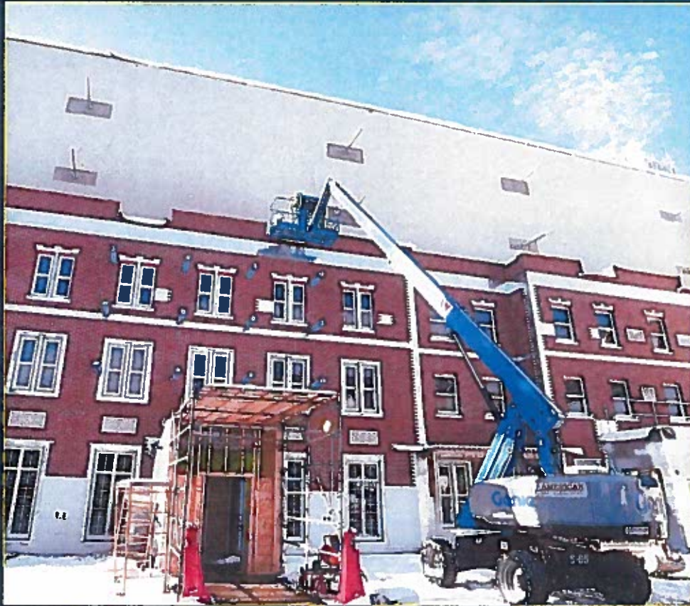
Entertainment Block Facade Construction
