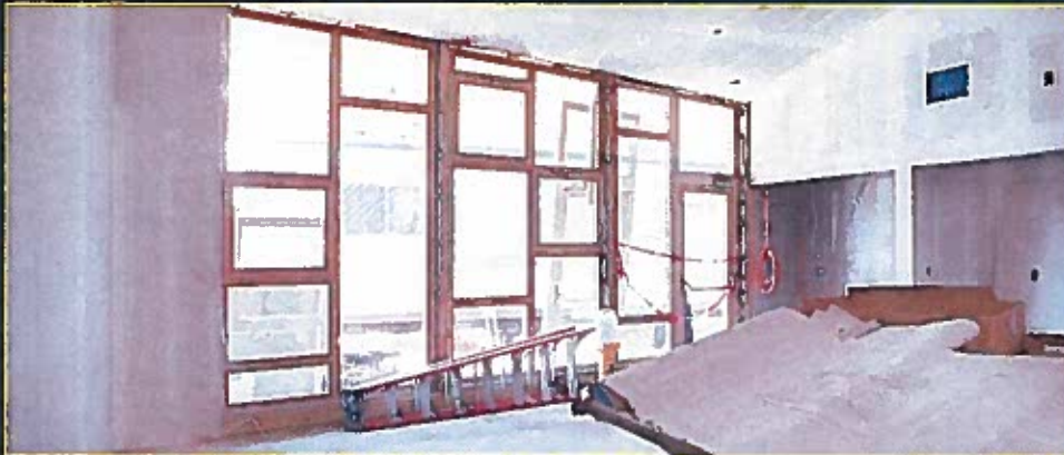
Early Childhood Center Construction
