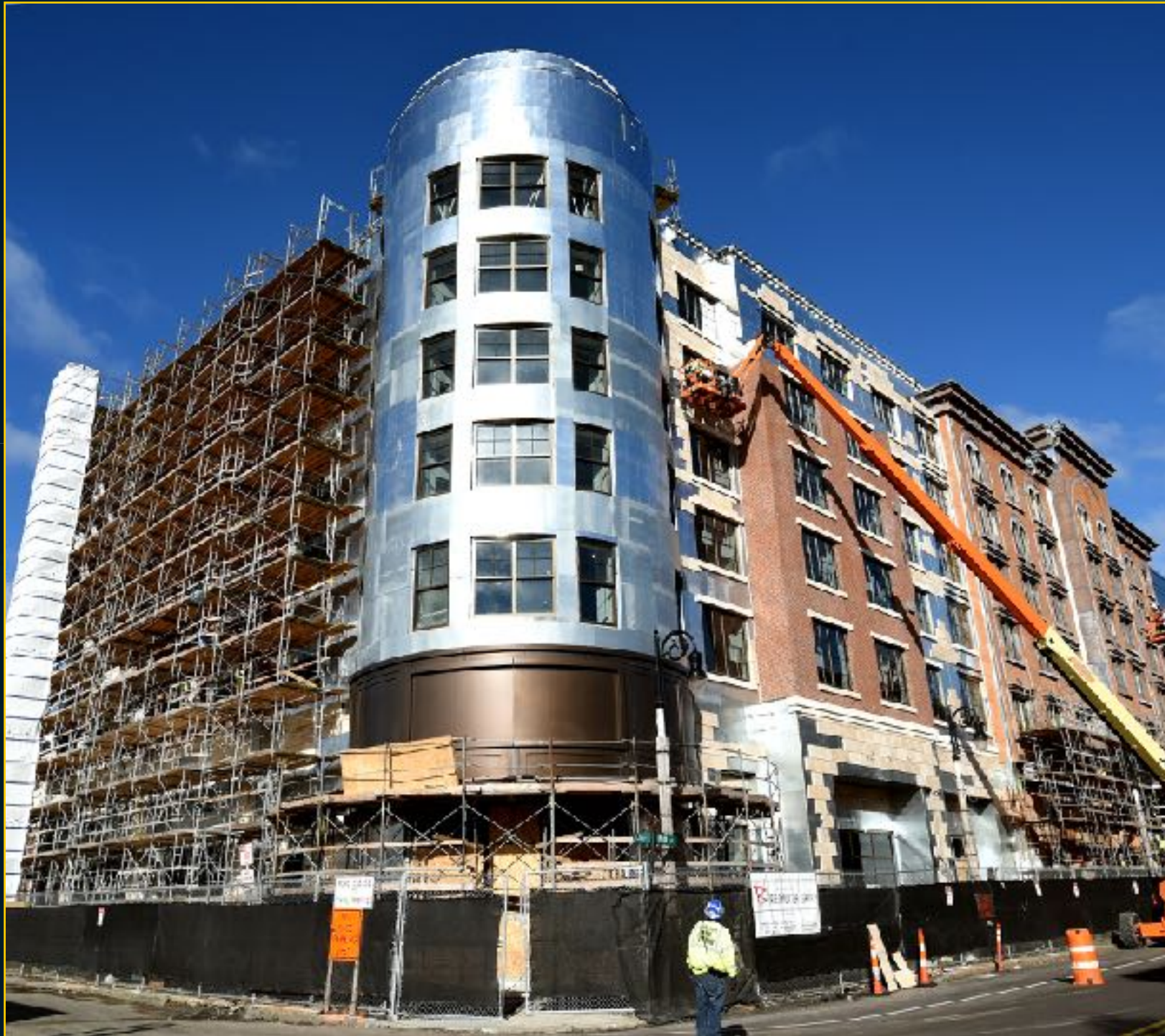
Main Entrance Construction
