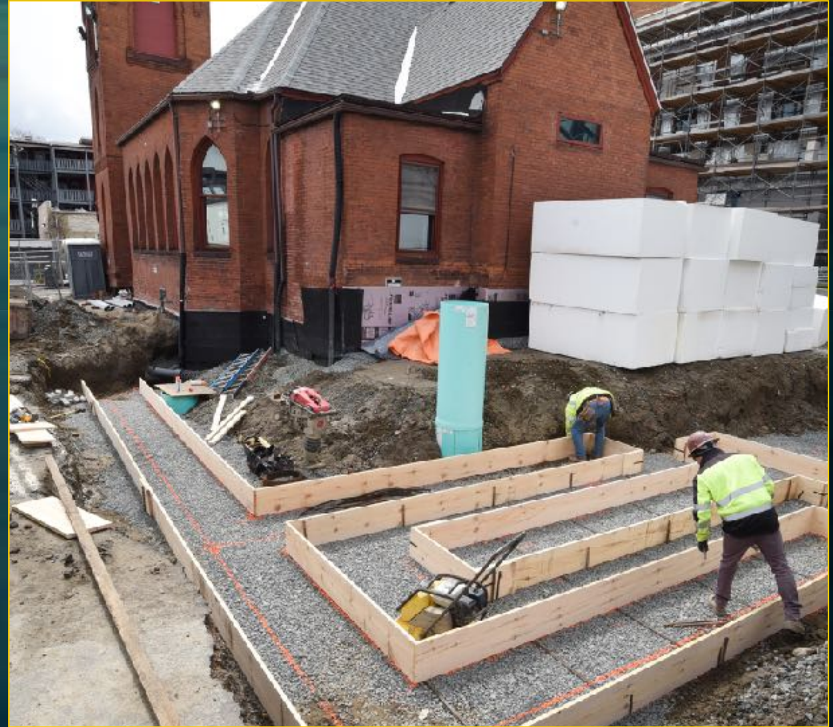
Church Exterior Construction
