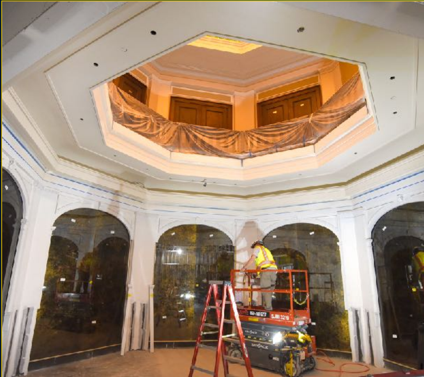
73 State Street Dome Construction
