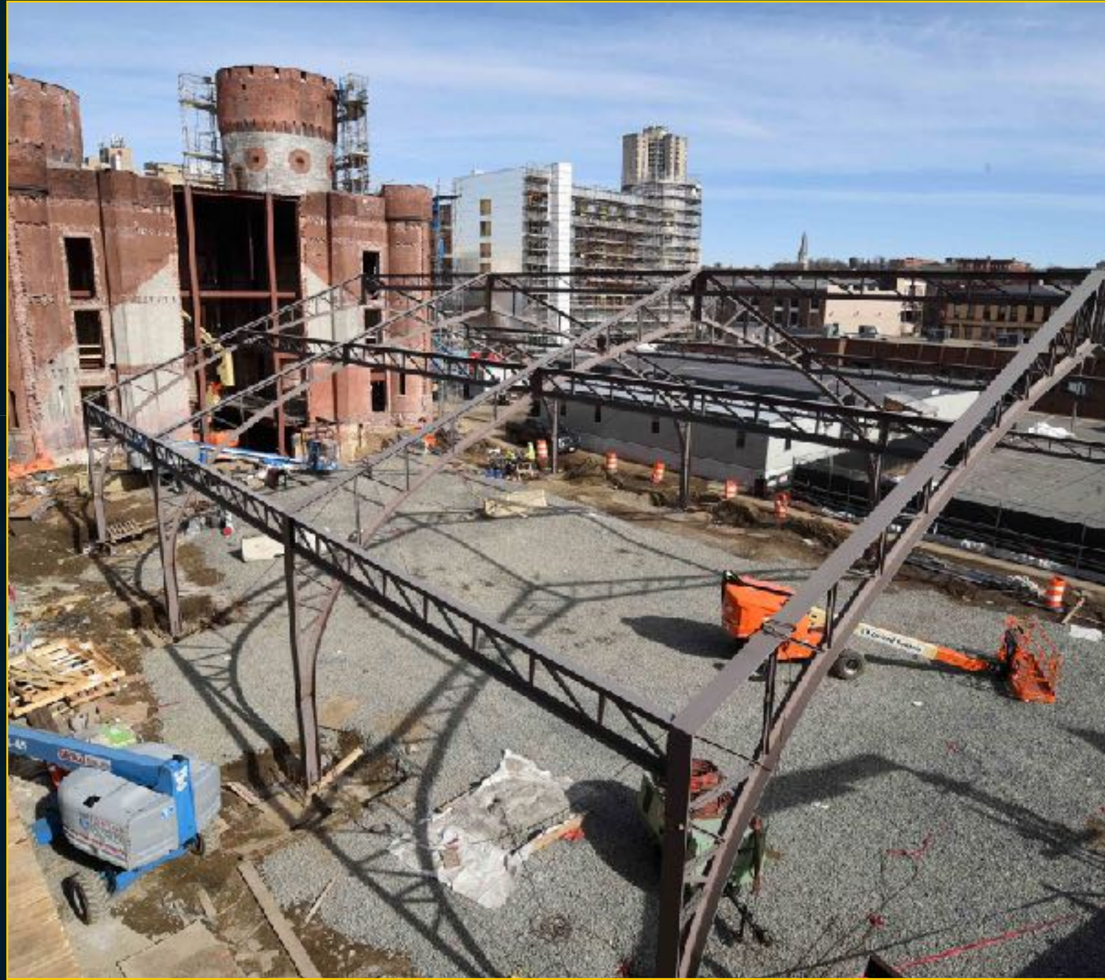
Armory Exterior Construction
