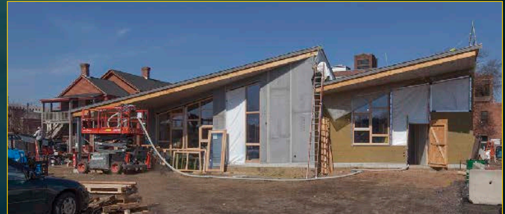
Early Childhood Center Construction
