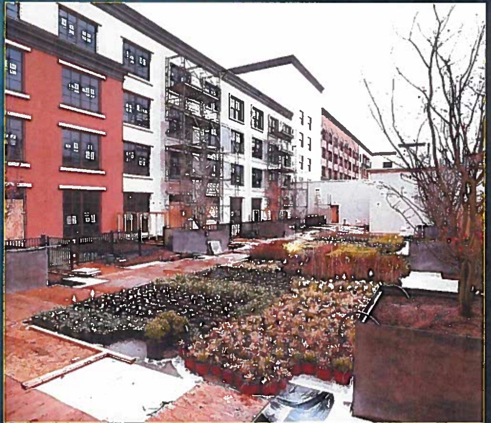
Main Street Facade Construction
