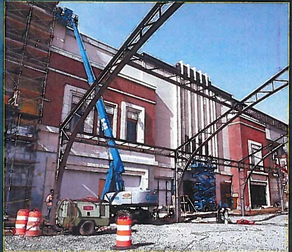
Entertainment Block Facade Construction
