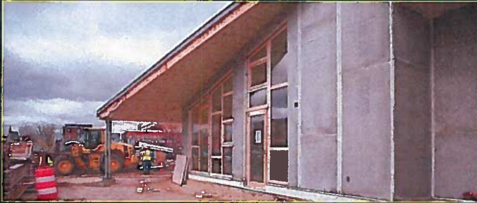
Early Childhood Center Construction
