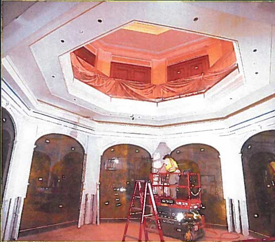
73 State Street Dome Construction
