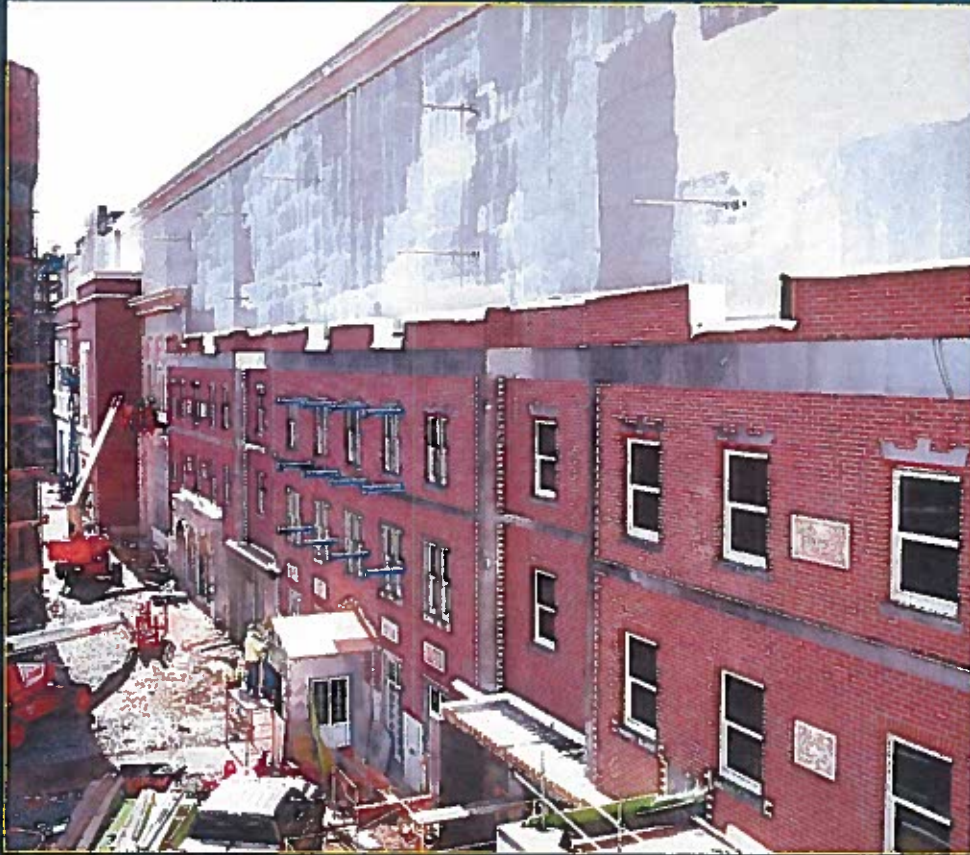
Entertainment Block Facade Construction
