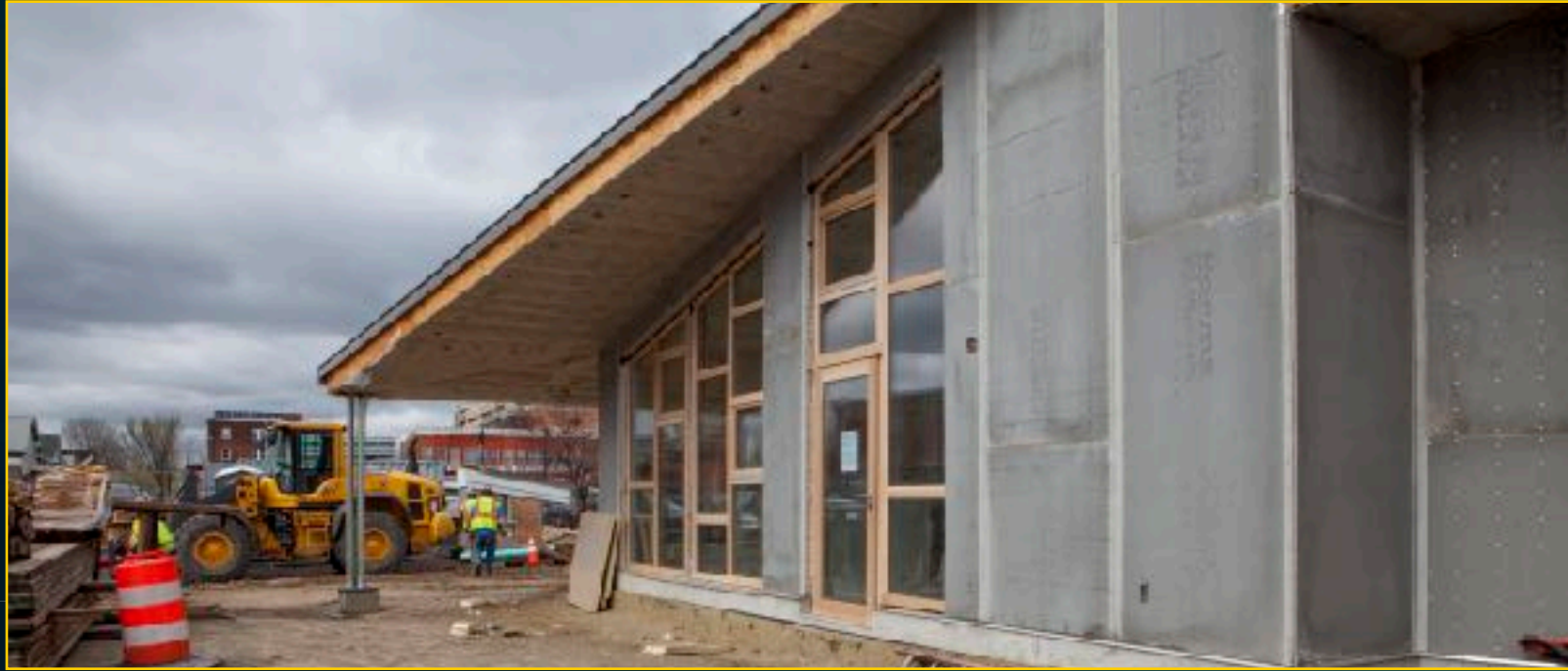
Early Childhood Center Construction
