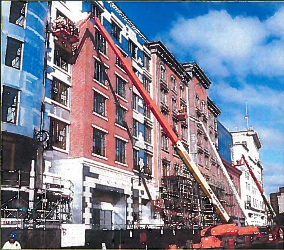
Main Street Facade Construction
