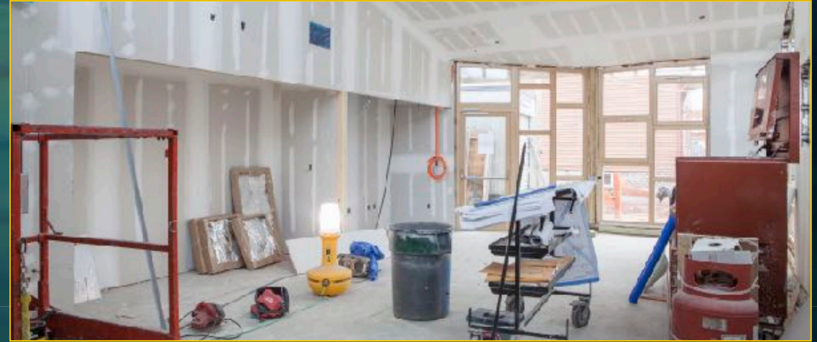
Early Childhood Center Construction
