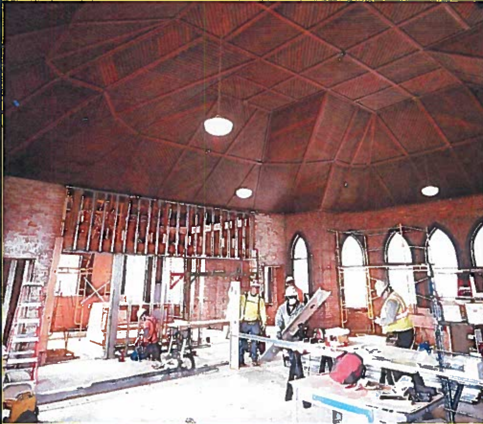
Church Interior Construction
