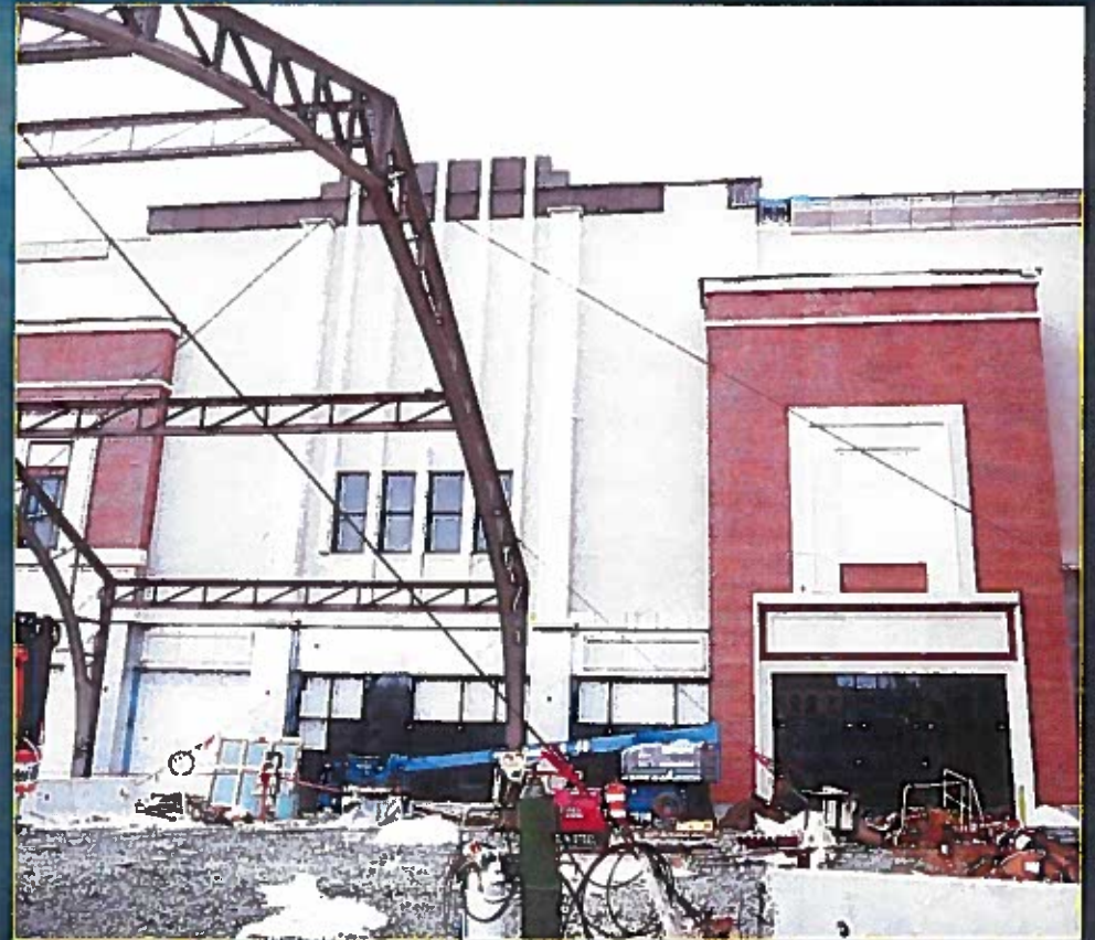
Entertainment Block Facade Construction
