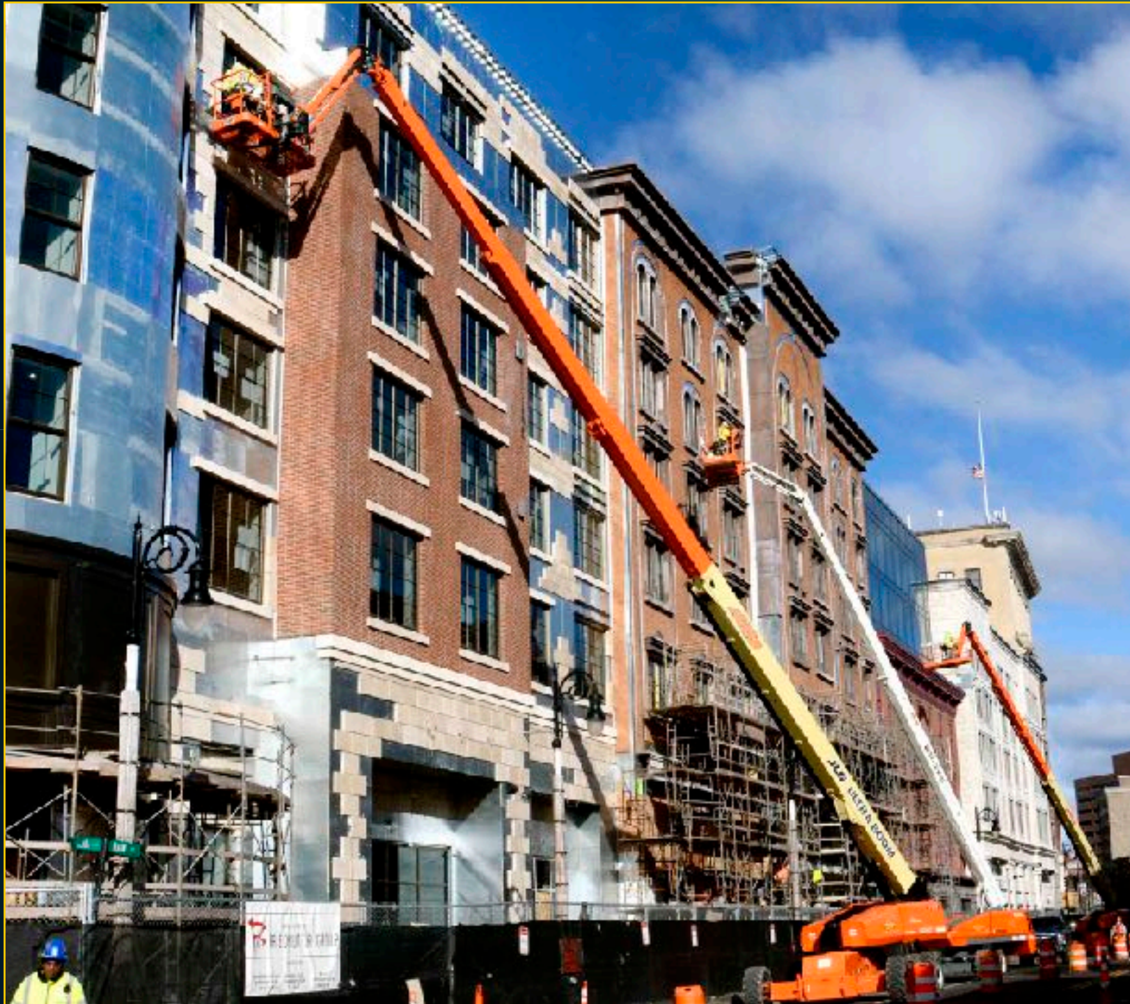
Main Street Facade Construction
