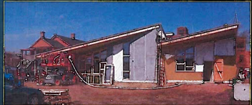
Early Childhood Center Construction
