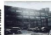
View from Worthington Street
