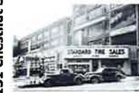
Looking at West Facade from Chestnut Street
