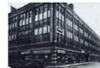
View from Worthington Street
