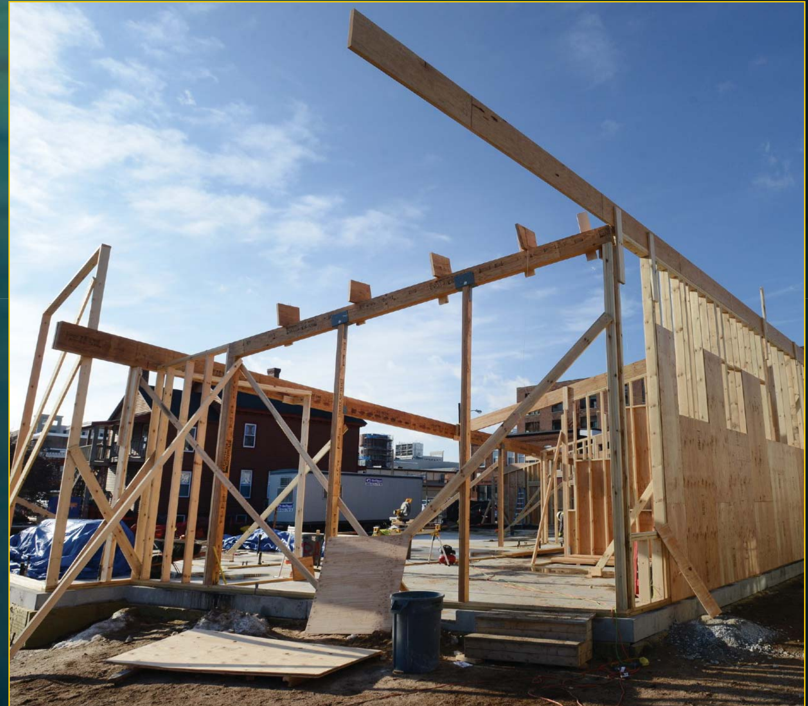
Daycare Construction - December 19, 2017
