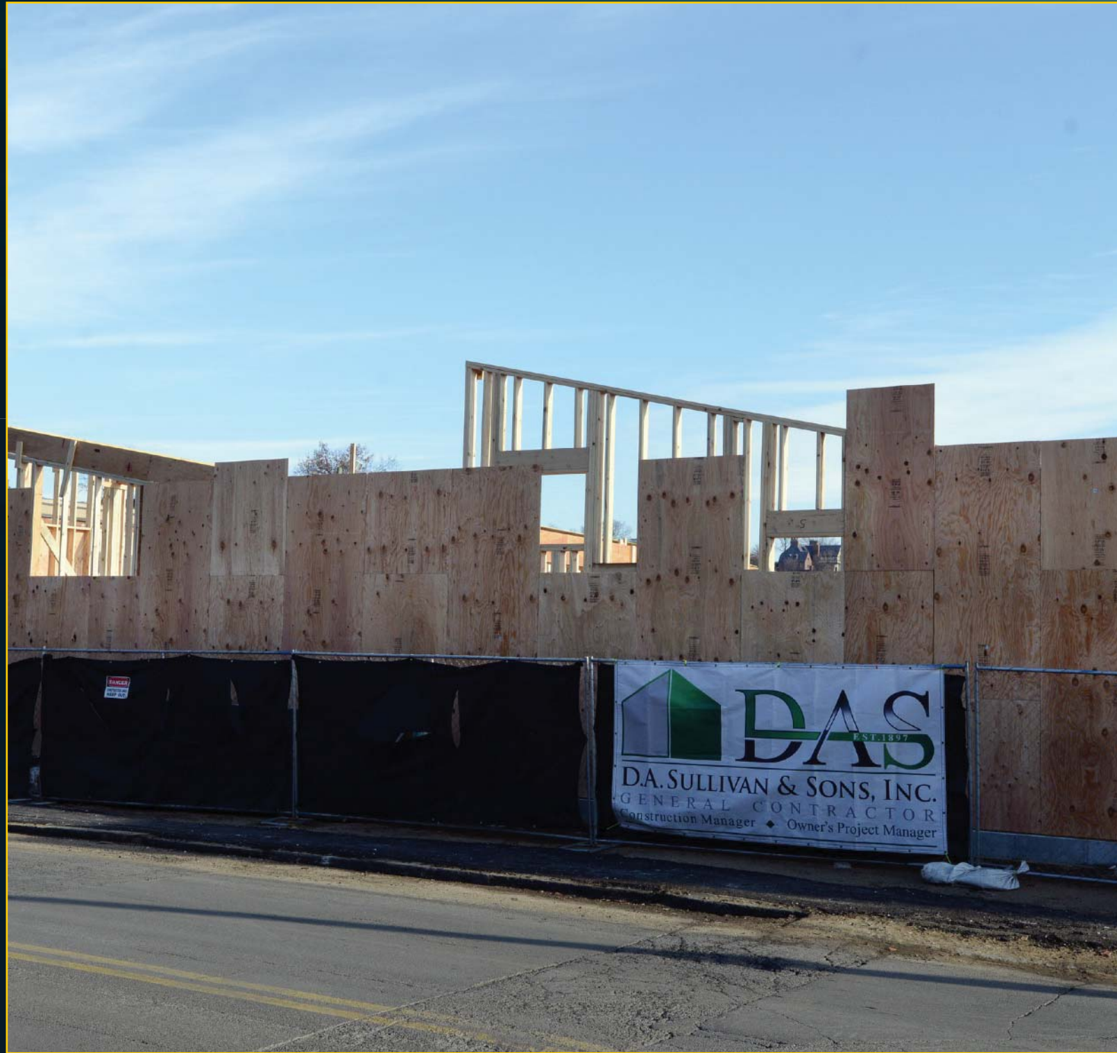
Daycare Construction - December 19, 2017
