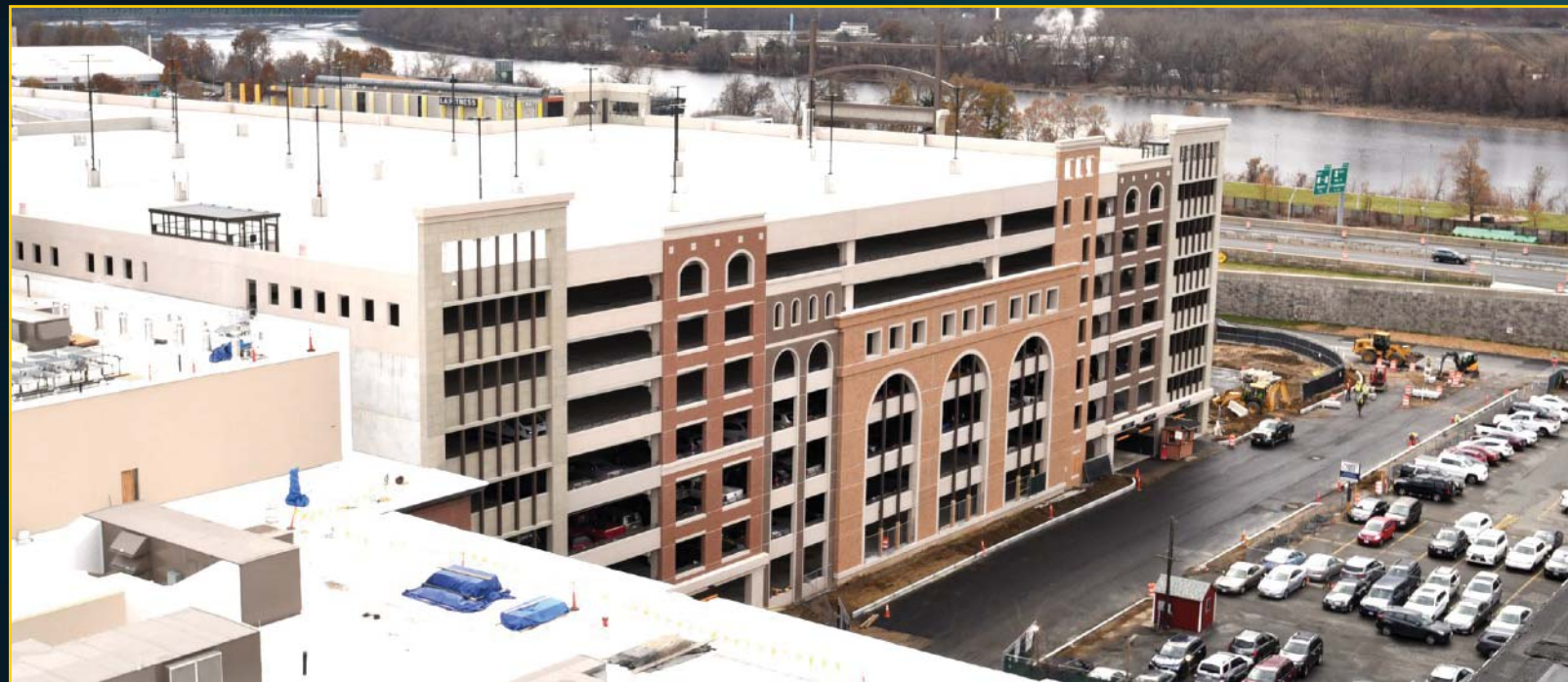
Garage Construction - December 1, 2017
