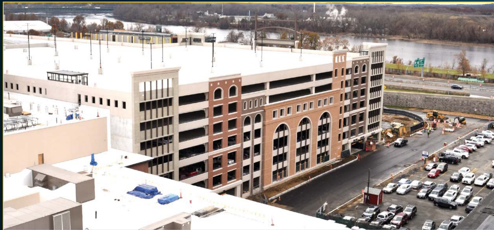
Garage Construction - December 1, 2017
