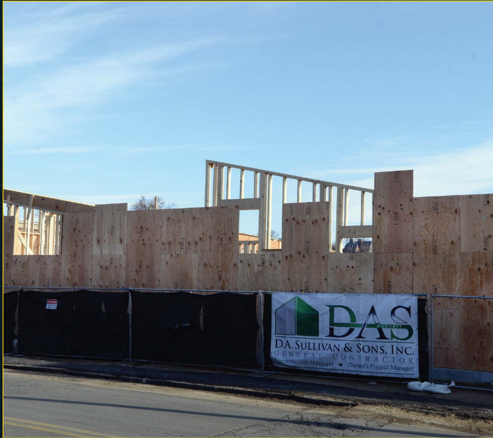
Daycare Construction - December 19, 2017
