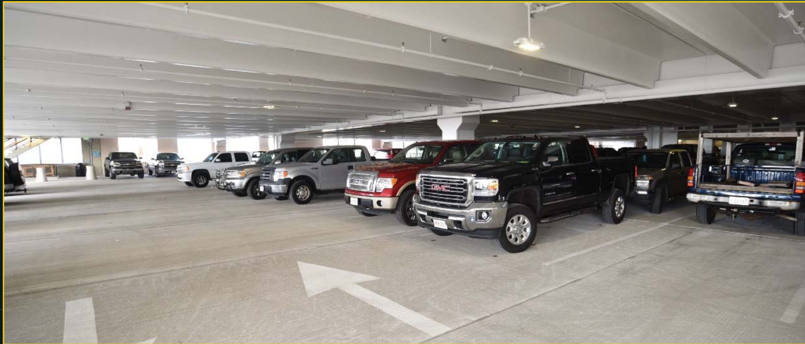
Workers Parking in Garage - October 10, 2017
