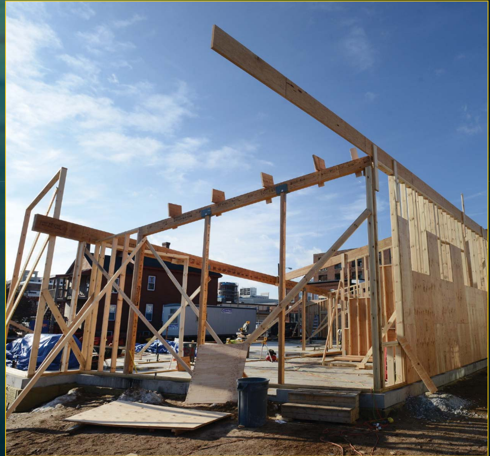
Daycare Construction - December 19, 2017
