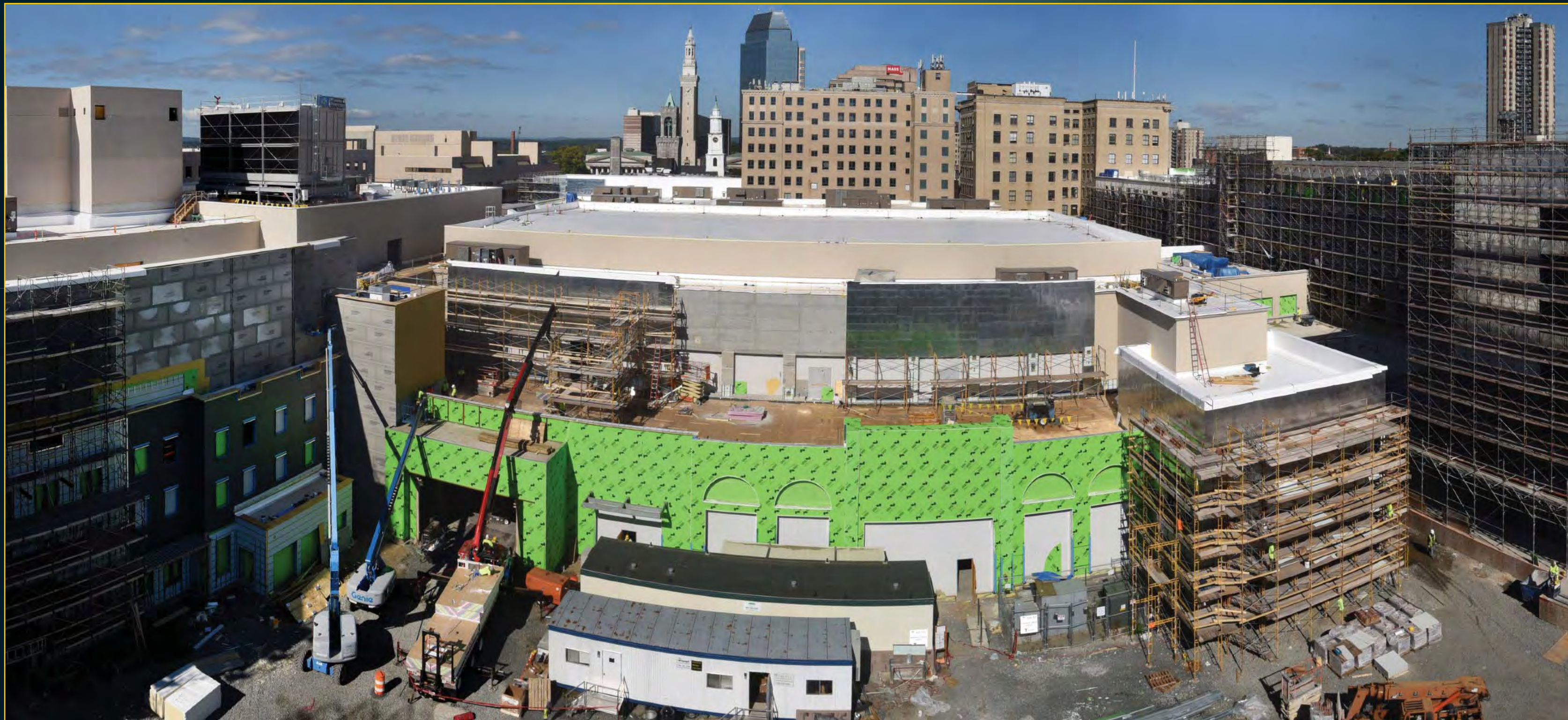
Overall Site Activity from Armory - October 3, 2017
