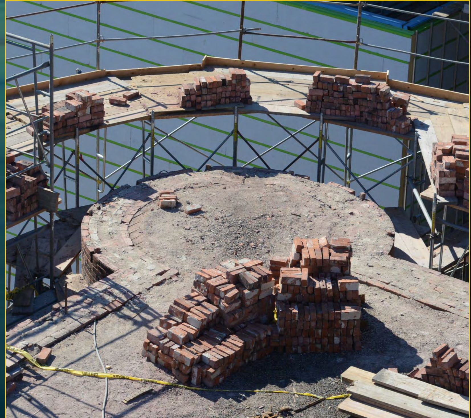
Armory Construction - October 3, 2017
