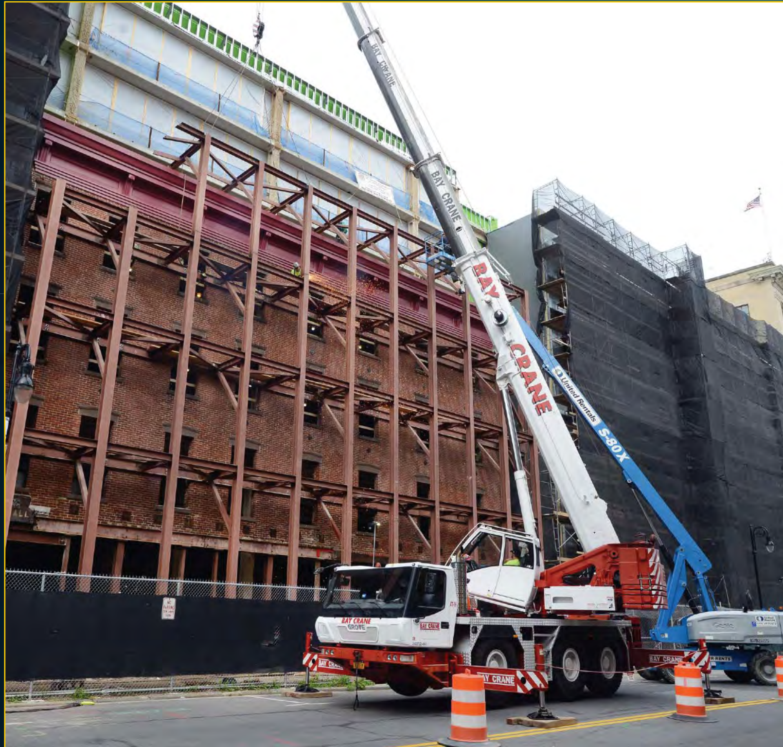
Union Chandler Construction - July 29, 2017
