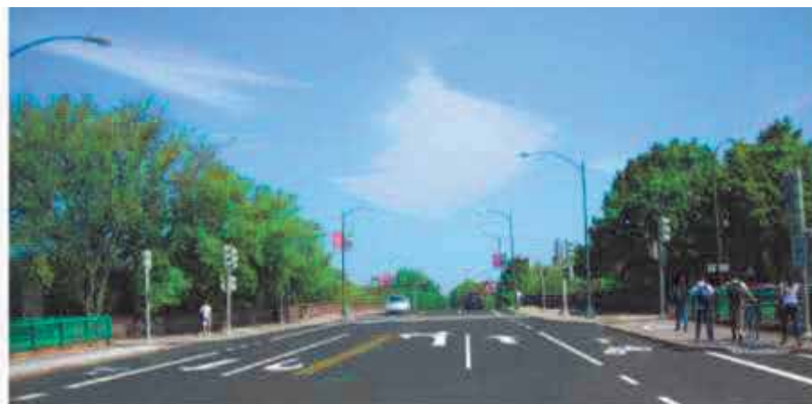
Lane Markings Make a Significant Difference - Before (top) and After (bottom) Location: Anderson Bridge, Cambridge, MA Source: MassDOT
