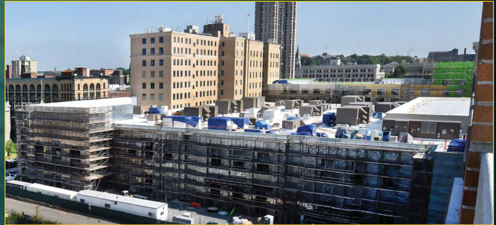
Podium Construction - August 31, 2017
