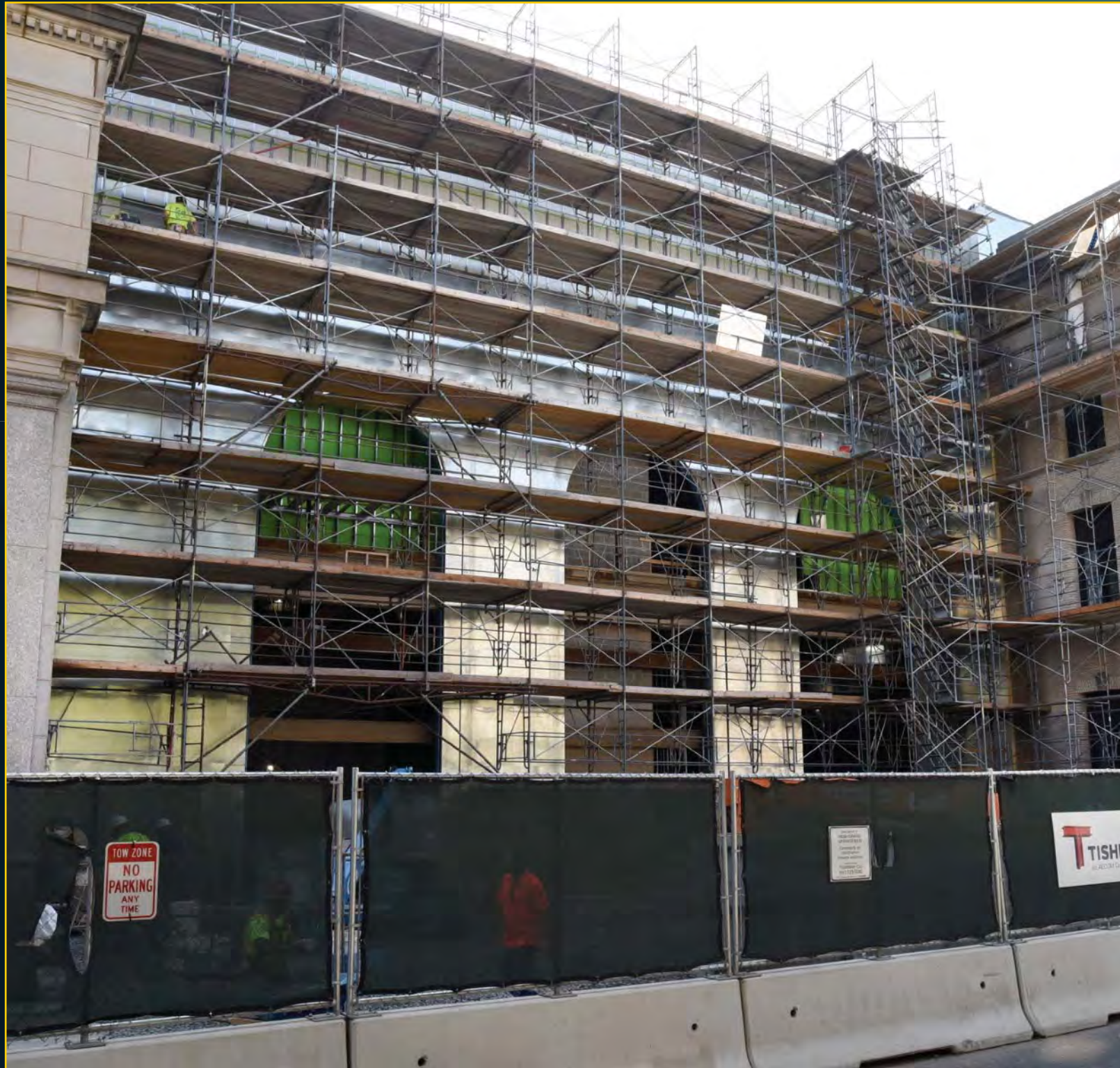
Podium Framing - August 31, 2017
