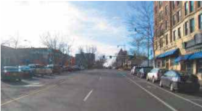
Angled Parking along a Median (left side) with a Bicycle Lane (right side) Location: Brookline, MA Source: MAPC
