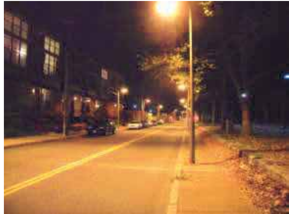
Street and Sidewalk Lighting Location: Jamaica Plain, MA Source: MAPC
