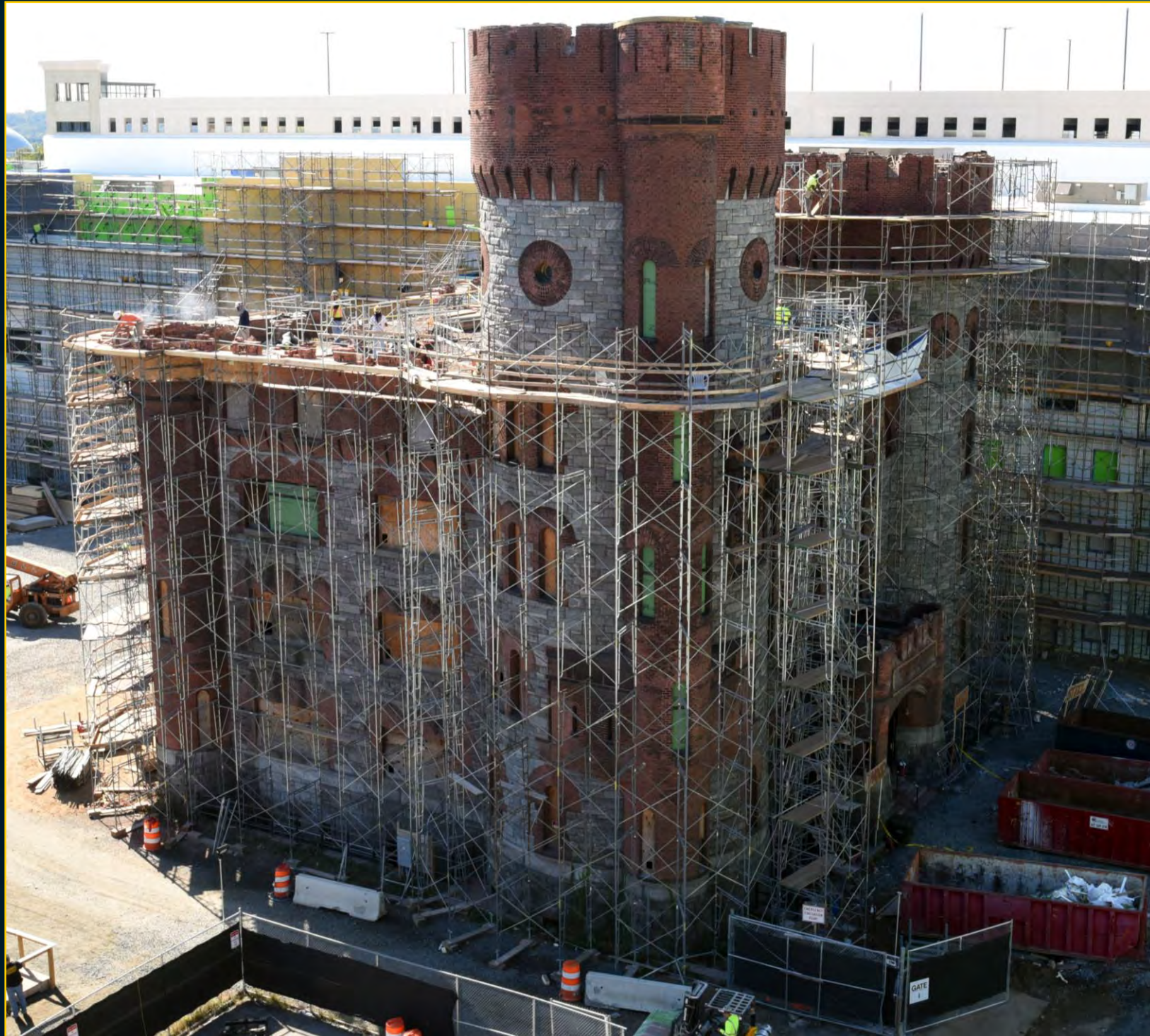
Armory Construction - October 3, 2017
