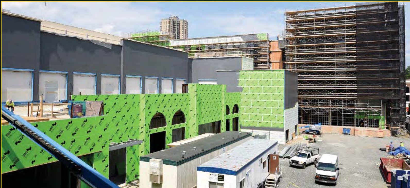
Podium Construction - August 21, 2017
