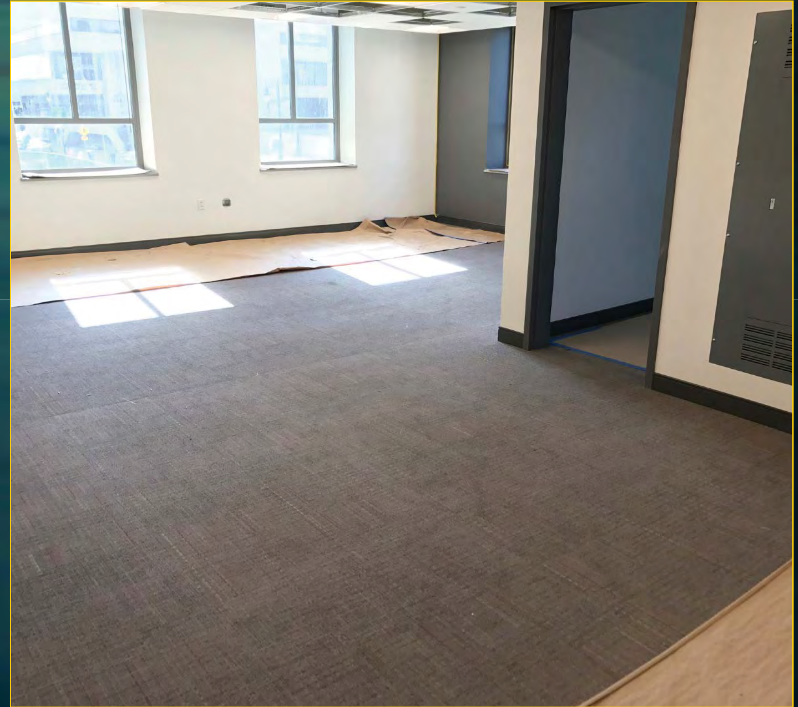
95 State Office Near Completion - September 15, 2017
