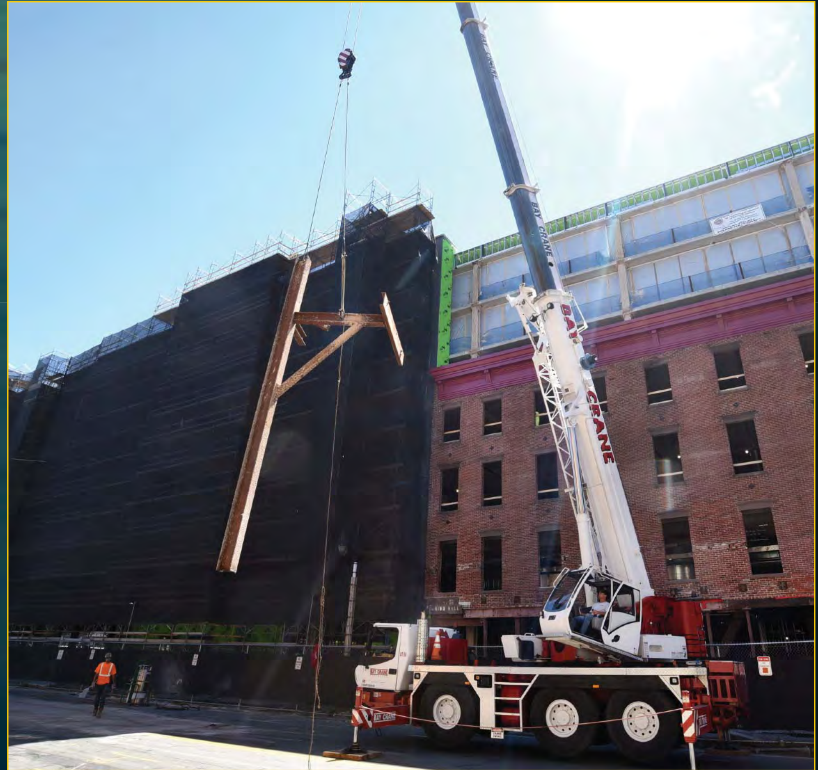
Union Chandler Construction - July 30, 2017
