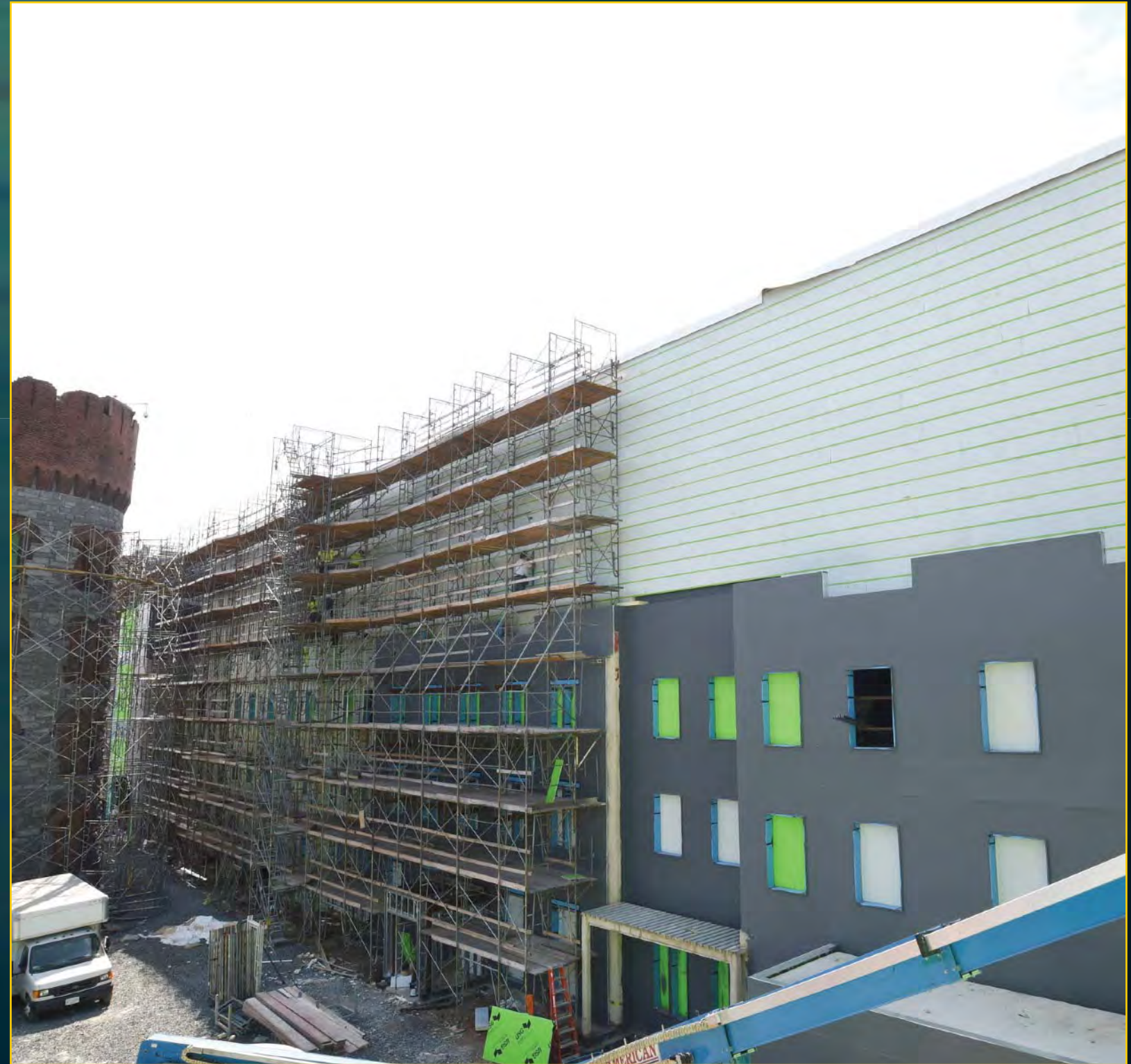
Entertainment Block Construction - September 13, 2017
