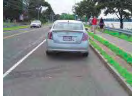
Excess Parking Lane Width Can be Reallocated for Pedestrian Space Location: Lake Quannapowitt, Wakefield Source: MAPC
