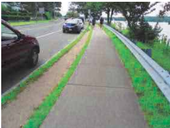
Well-Worn Desire Line Adjacent to Sidewalk Location: Lake Quannapowitt, Wakefield Source: MAPC
