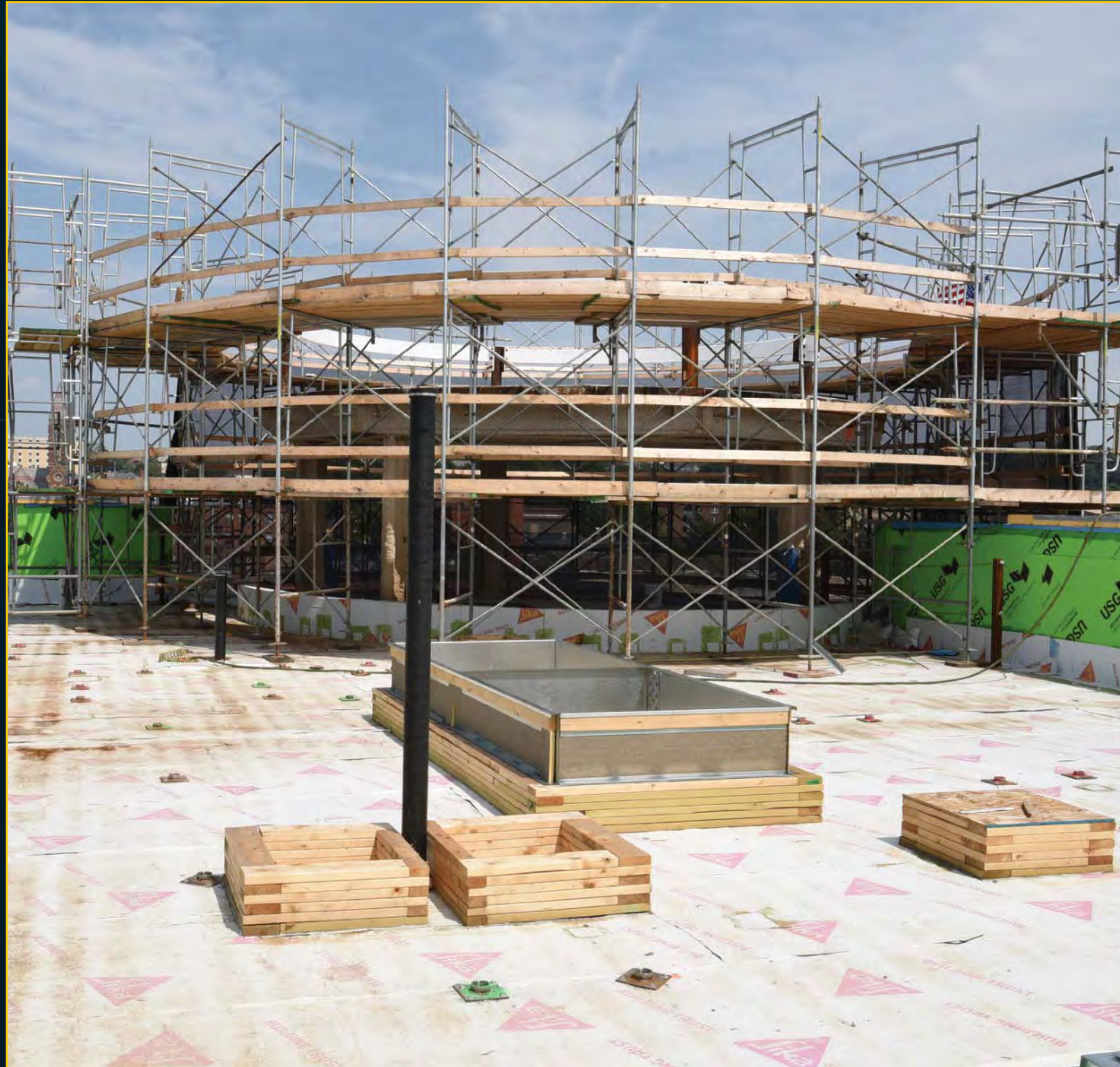
Hotel Construction - August 21, 2017
