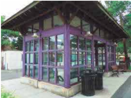
Commuter Rail Enclosed Shelter Location: Wyoming Hill Station, Melrose Source: MAPC
