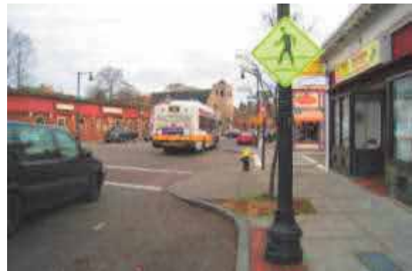
Curb Extension Location: West Roxbury, MA Source: MAPC
