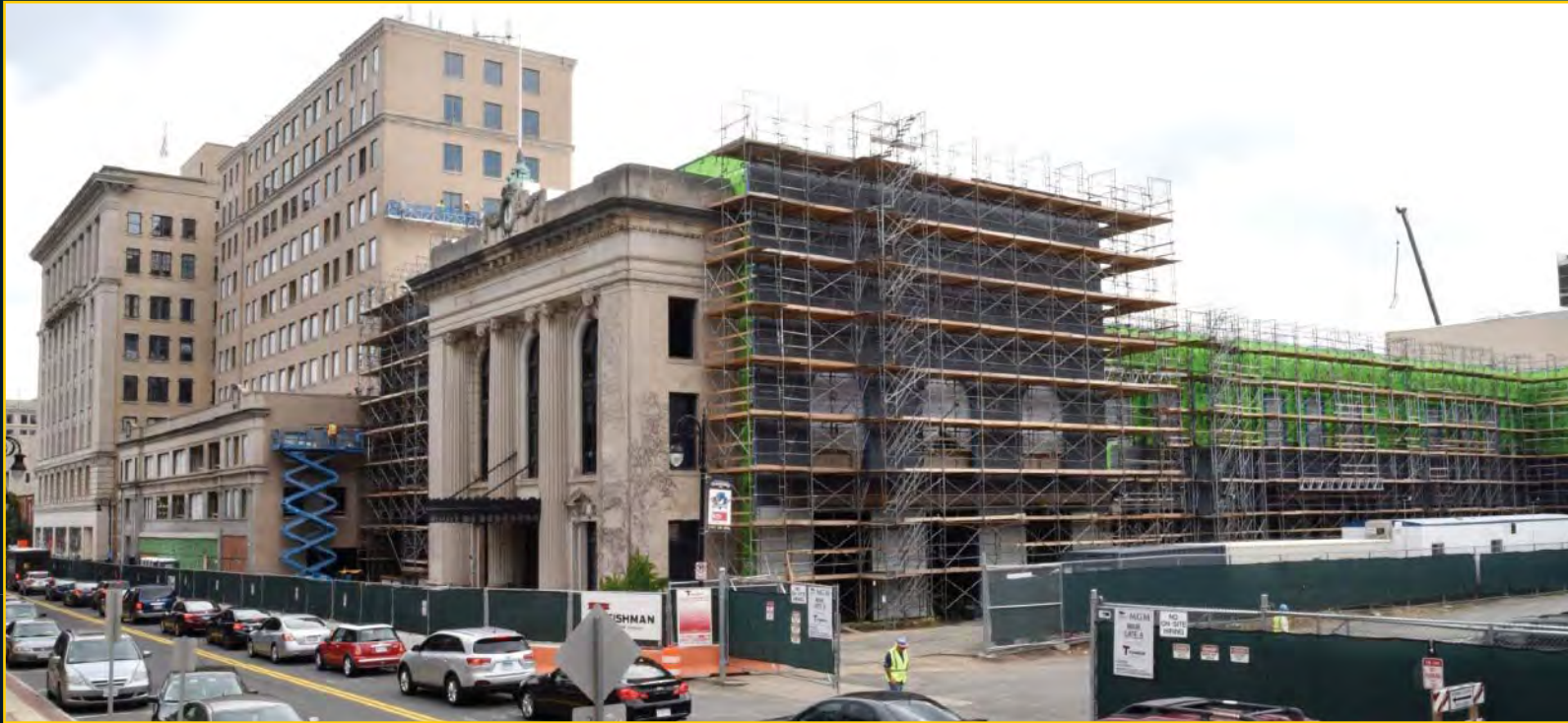
Podium Framing - July 18, 2017
