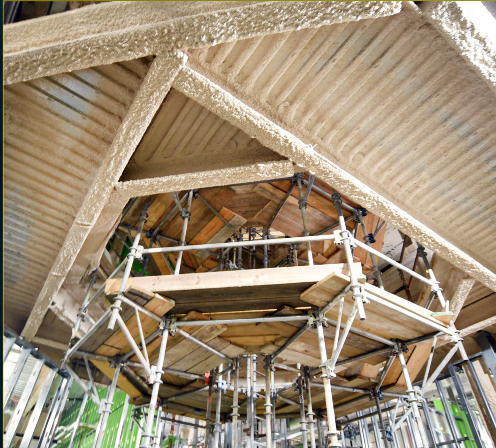
Scaffolding Prepared for Dome Relocation - September 13, 2017
