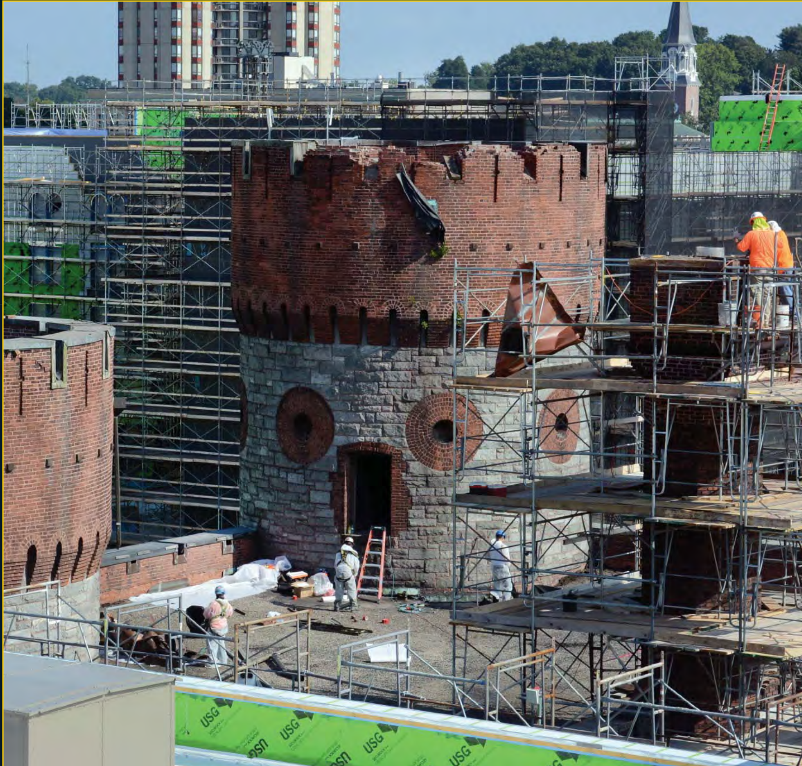
Armory Construction - August 31, 2017
