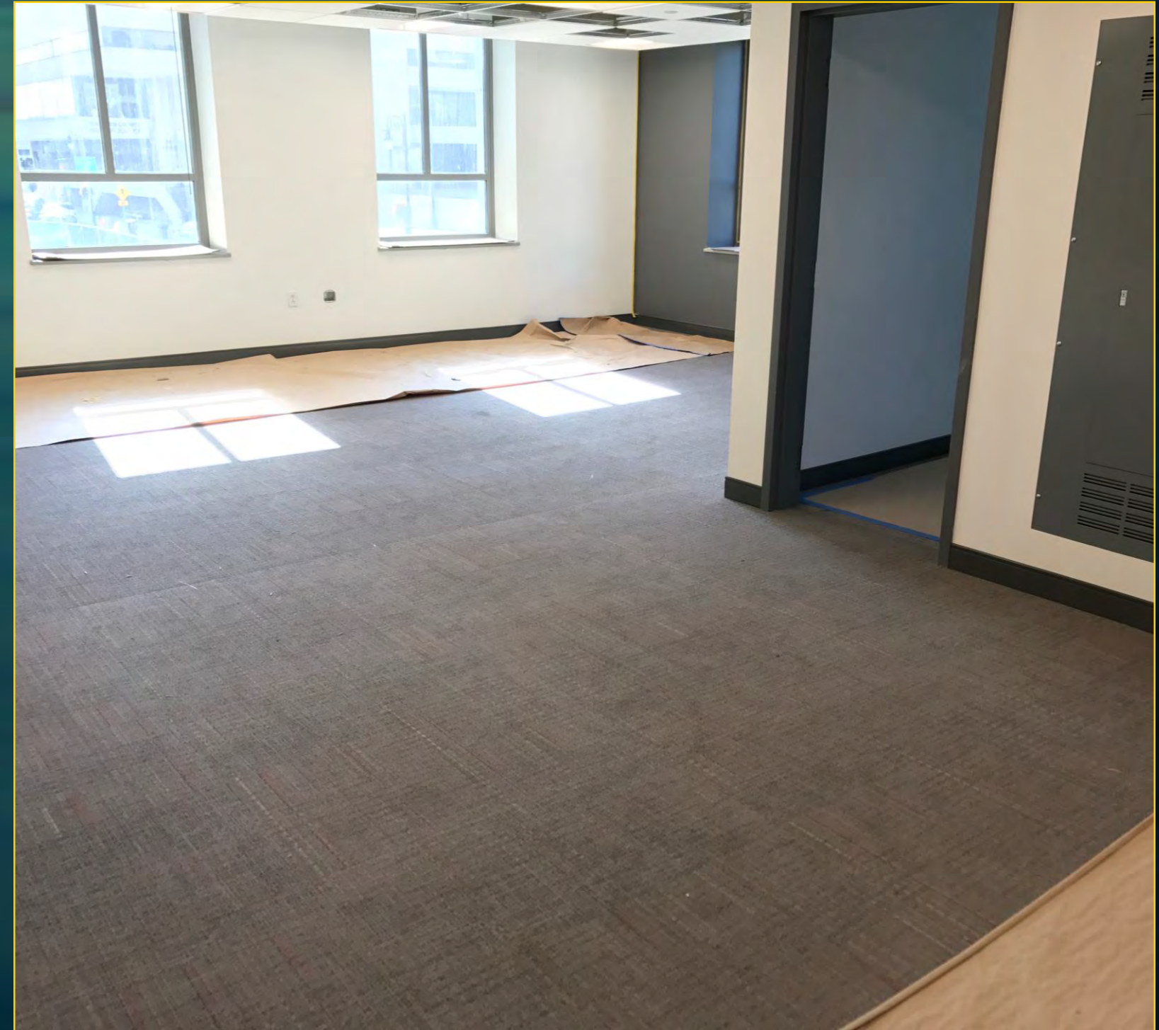
95 State Office Near Completion - September 15, 2017
