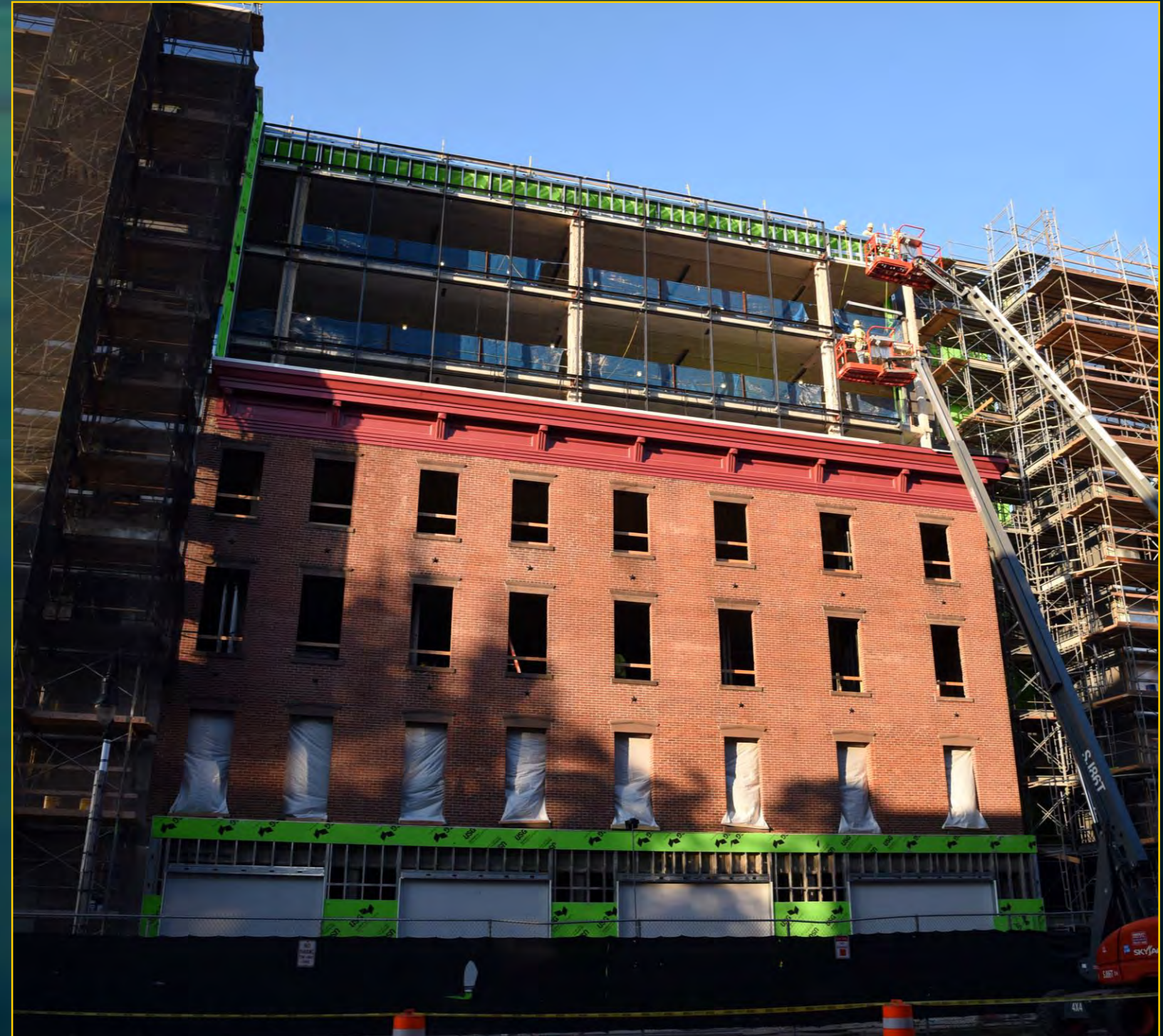
Union Chandler Construction - September 28, 2017
