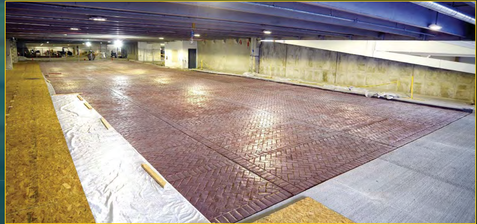
Valet Area Concrete
