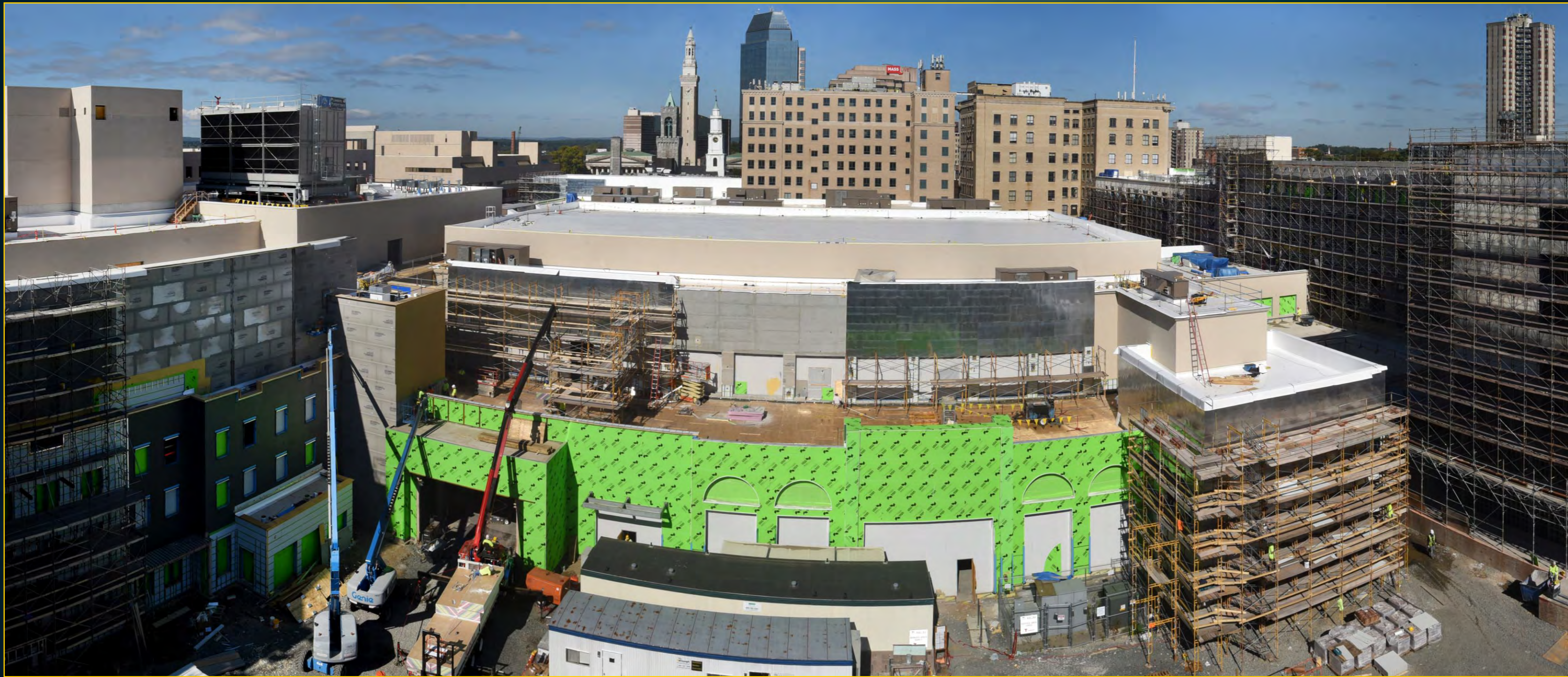
Overall Site Activity from Armory - October 3, 2017
