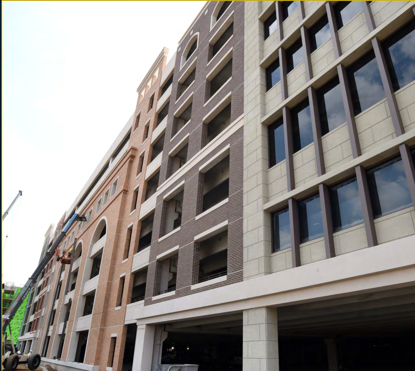
Garage Construction - July 18, 2017
