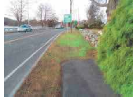
Example of Abruptly Ending Sidewalk Across from Lake Quannapowitt Location: Wakefield Source: MAPC
