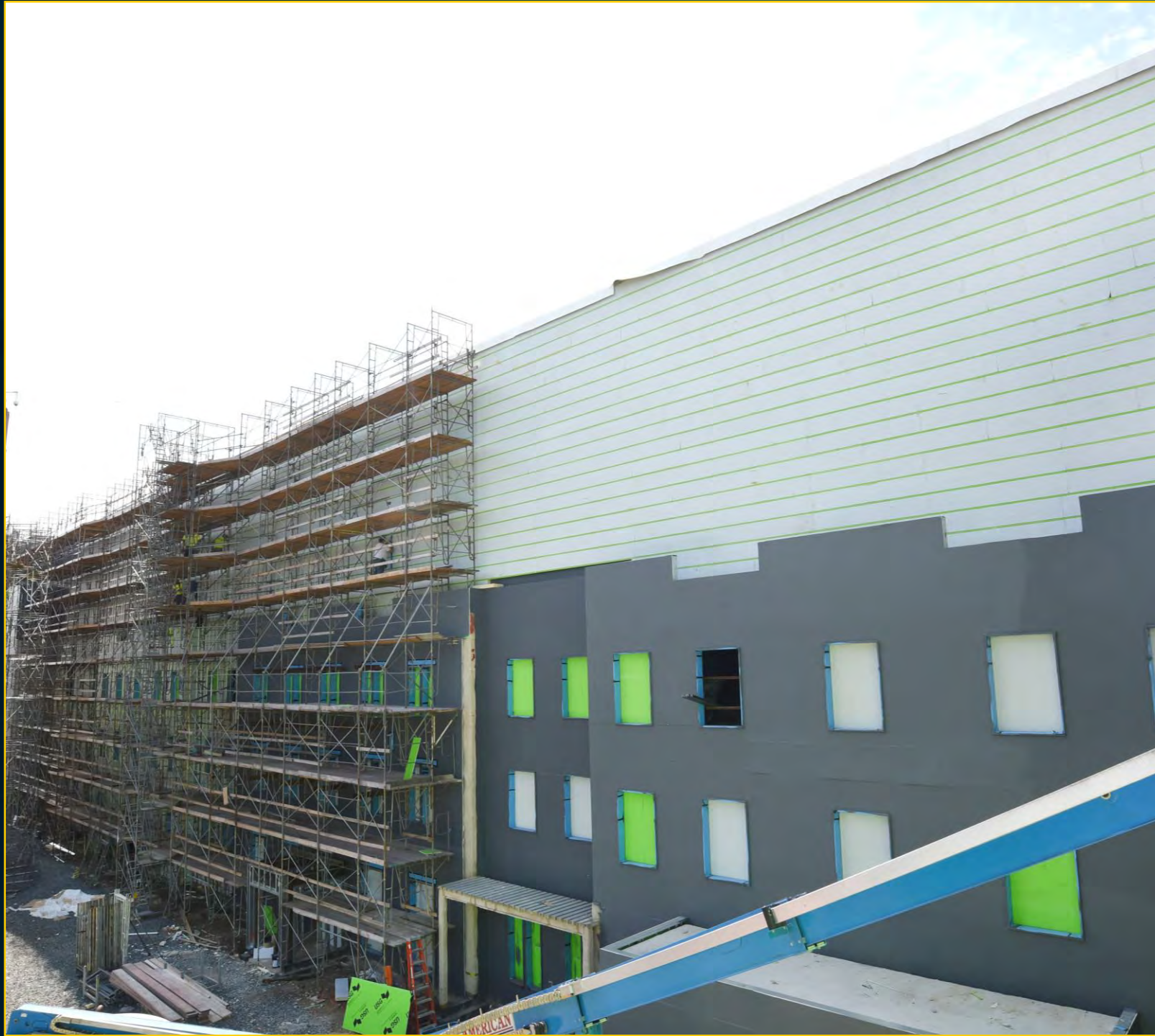
Entertainment Block Construction - September 13, 2017
