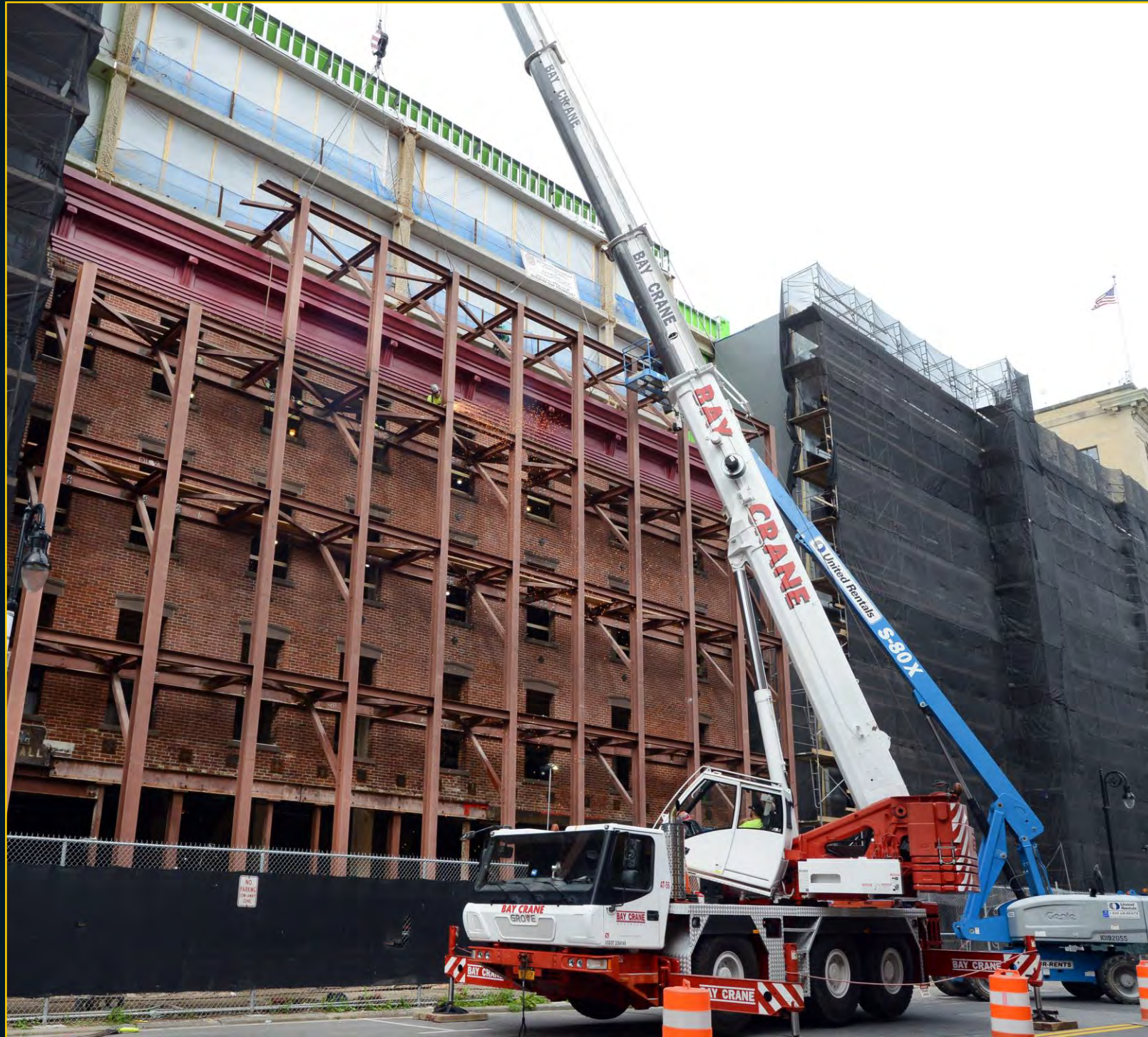
Union Chandler Construction - July 29, 2017
