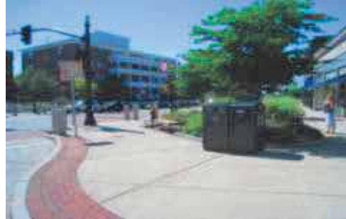
Newly Installed Sidewalk in Downtown Reading Source: MAPC
