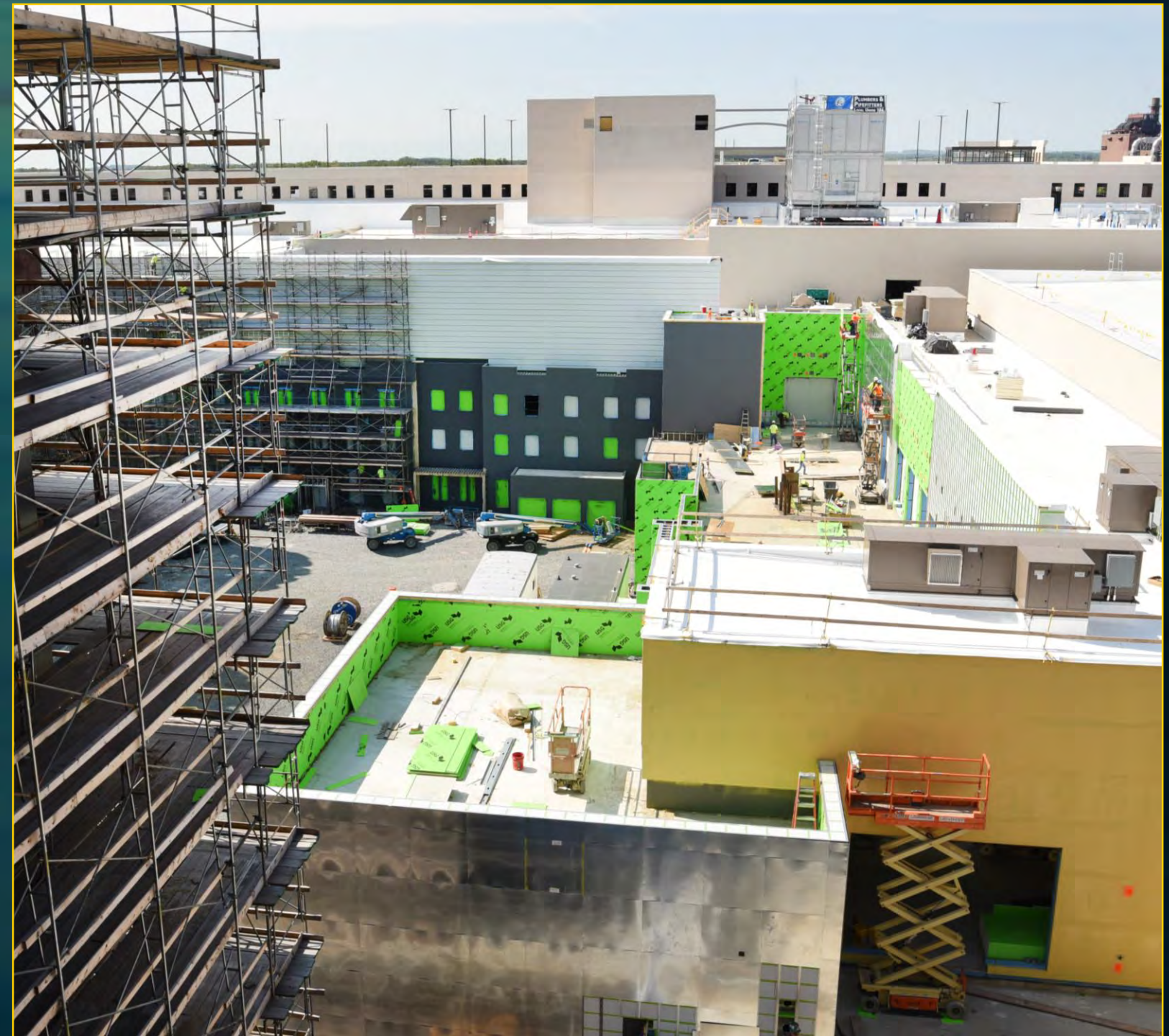
Podium Construction - September 13, 2017
