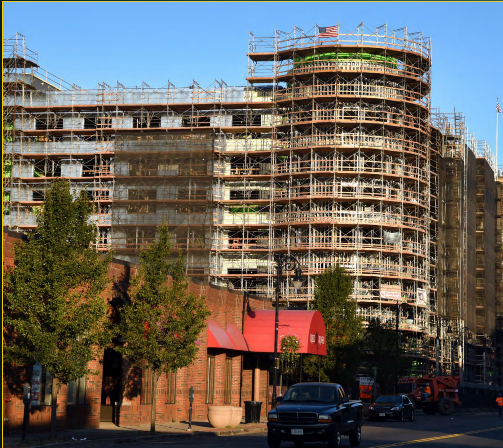
Hotel Construction - September 28, 2017
