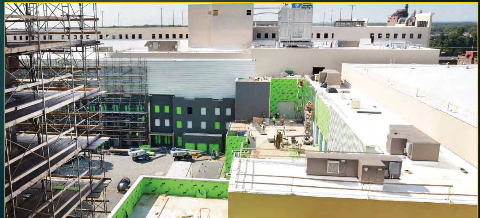
Podium Construction - September 13, 2017
