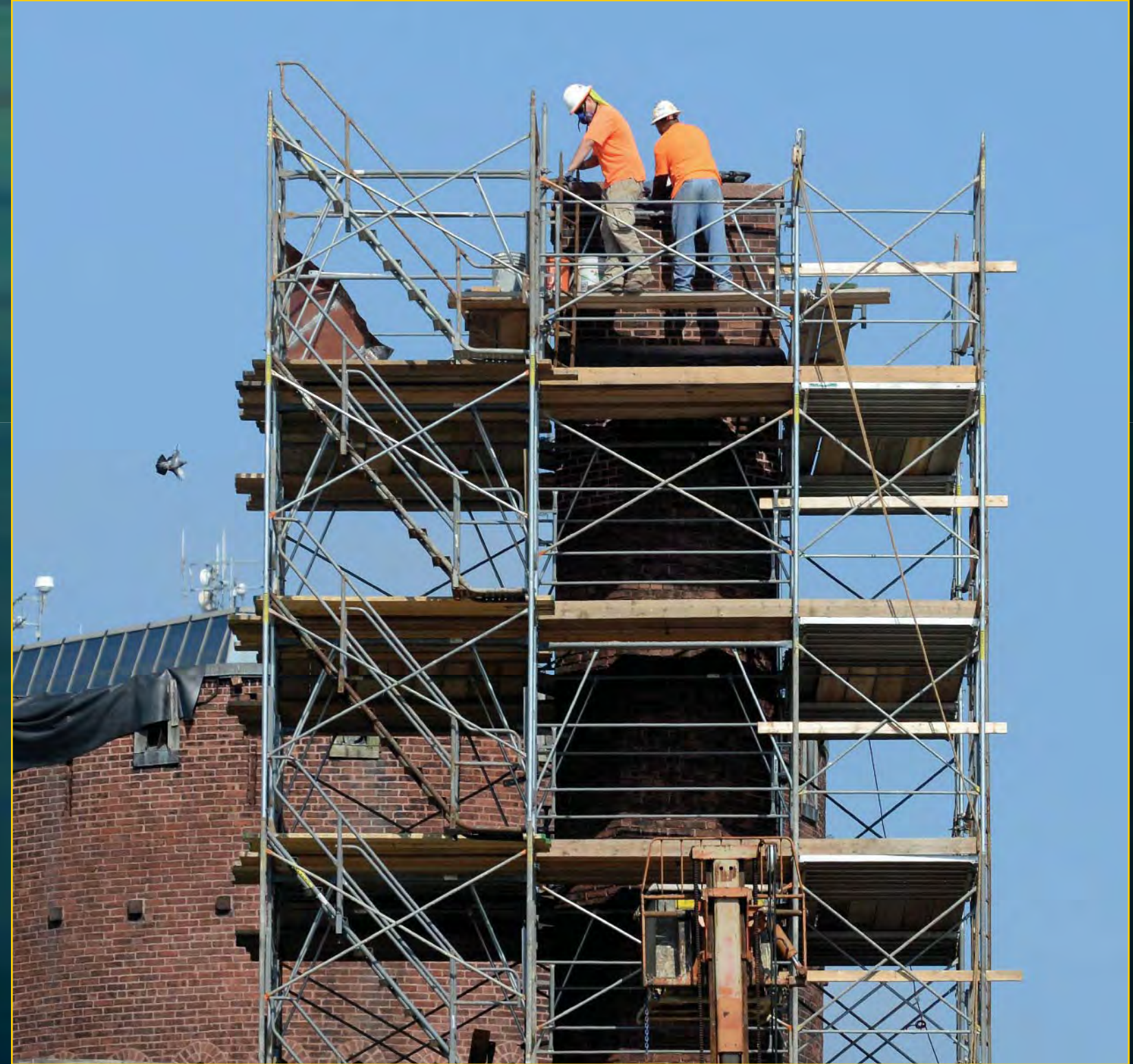
Armory Construction - August 31, 2017
