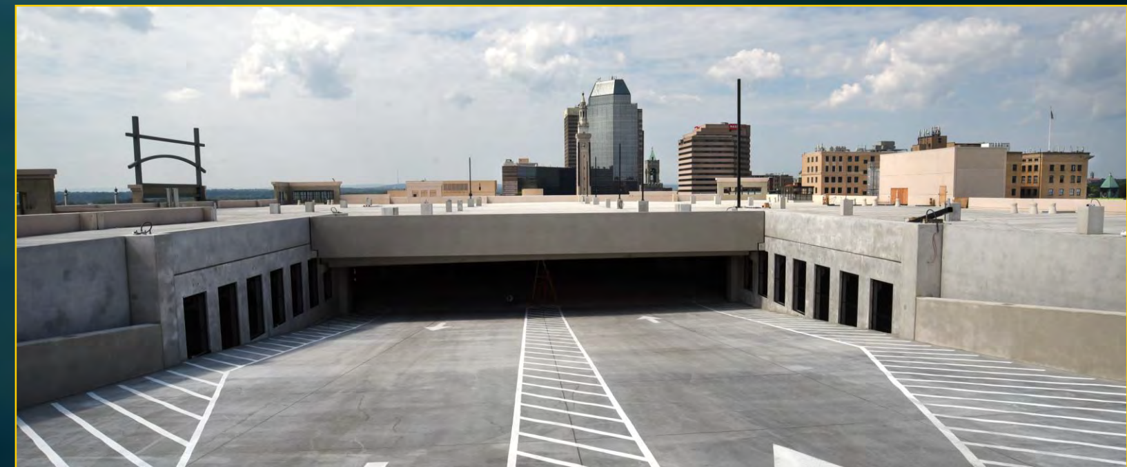
Garage Construction - August 21, 2017
