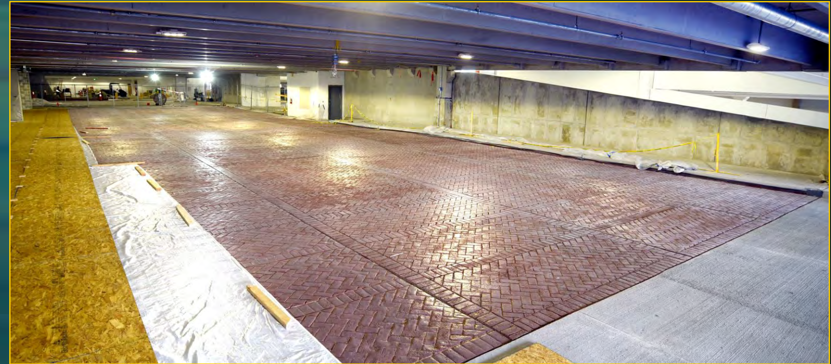
Valet Area Concrete
