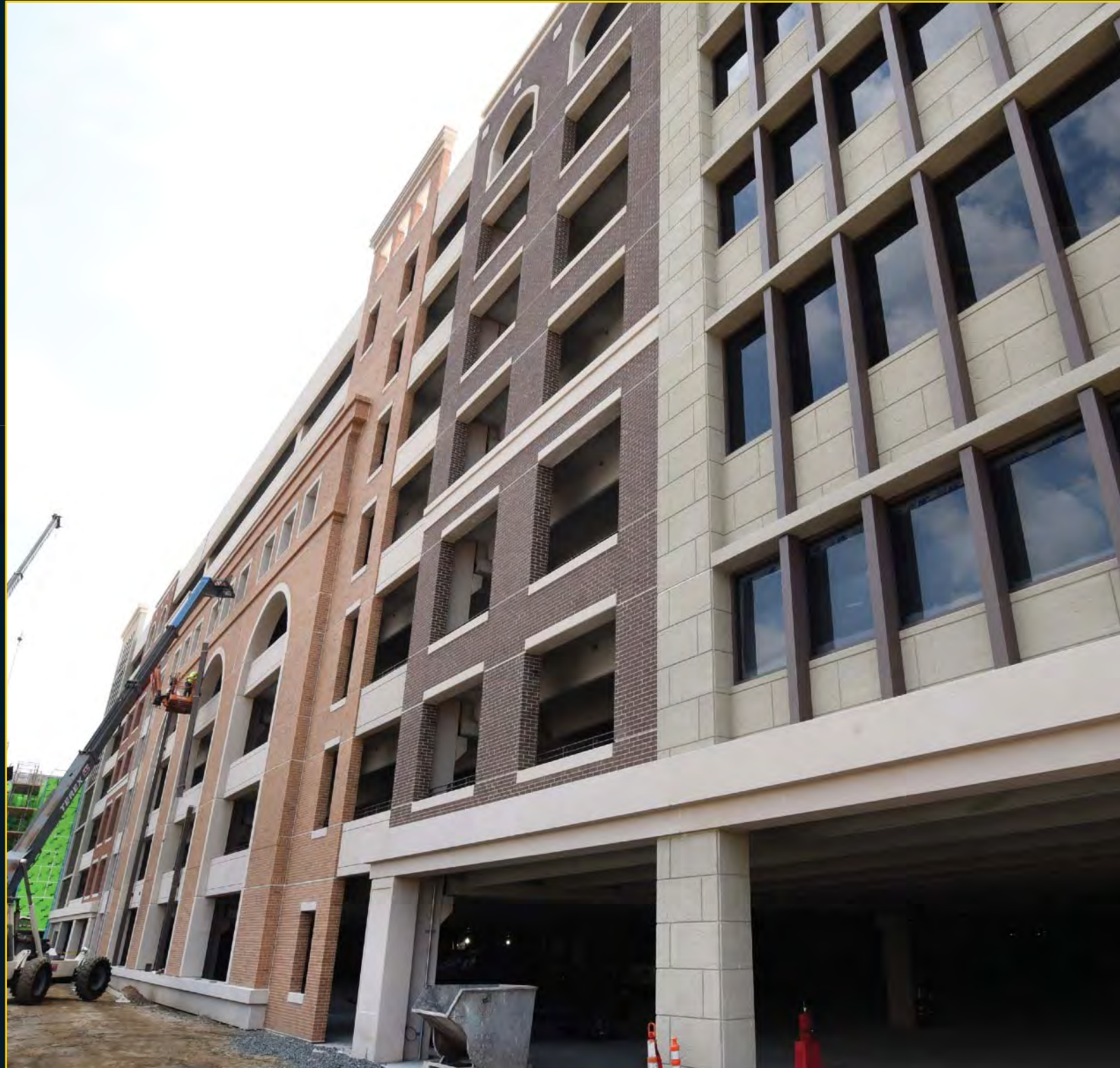
Garage Construction - July 18, 2017
