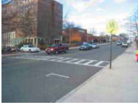
A Crosswalk with a Continental or Ladder Design Location: Melrose Source: MAPC
