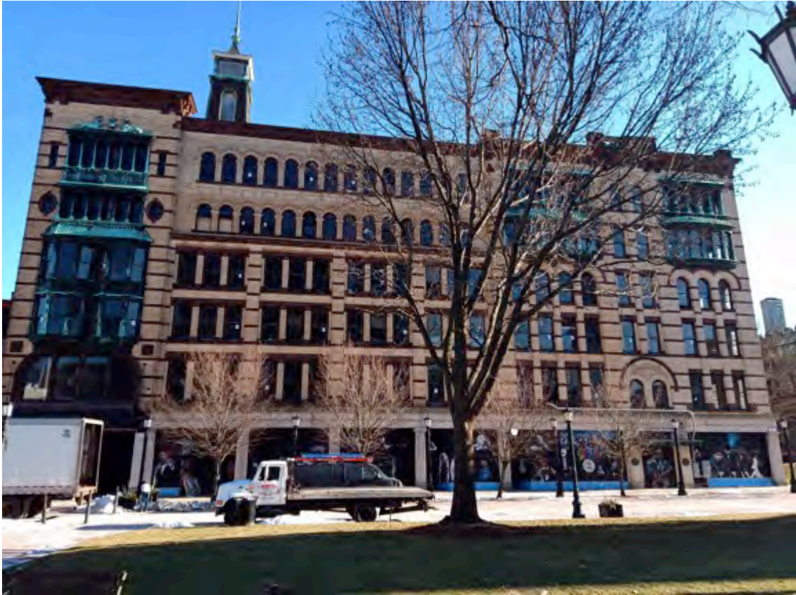
13-31 Elm St.: Lack of connection with street/park; future Ground Floor Restaurant / Retail
