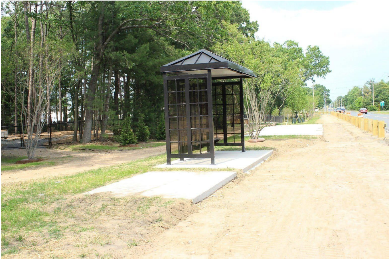
Attachment 6 Transit Stop with Slabs poured for Bicycle Infrastructure in Foreground and Background
