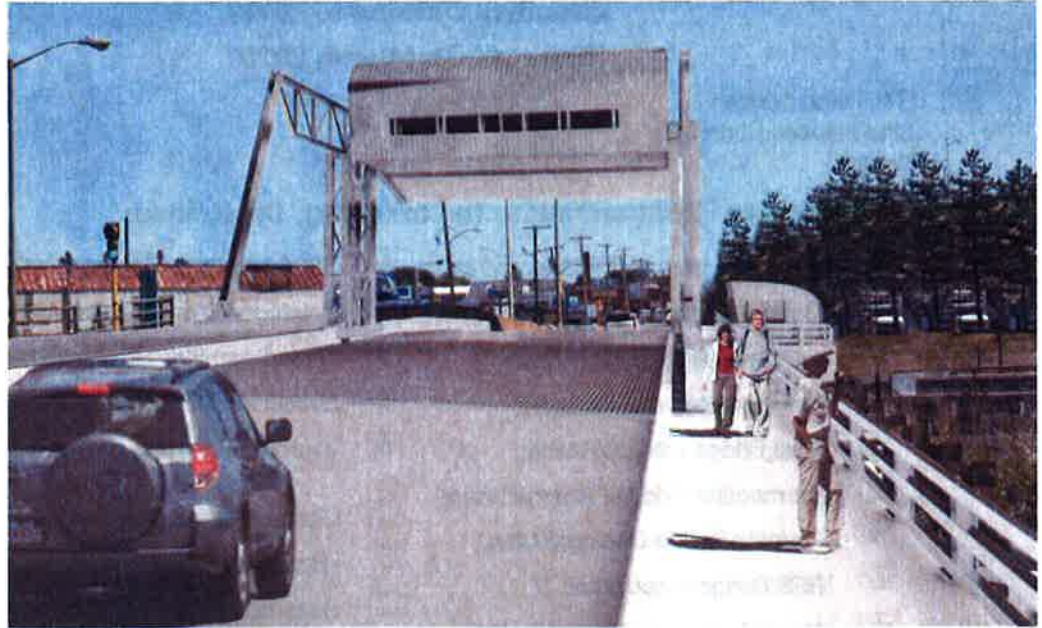
THE BELDEN BLY BRIDGE WILL FEATURE A SINGLE-LEAF, HEEL-TRUNNION BASCULE CENTER SPAN THAT WILL ROTATE ALONG FOUR SEPARATE POINTS AS IT OPENS.
