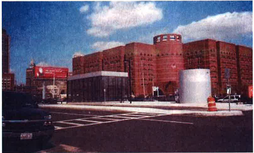
NORTHERN AVENUE WAS REDESIGNED AS PART OF THE TRANSITWAY PROJECT, WHICH LINKED DOWNTOWN BOSTON TO THE SEAPORT DISTRICT.
