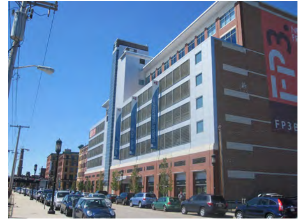
Parking garage facades should have fenestration or grillwork to obscure views to cars. From left: the “green screen” on the garage above helps to soften the appearance of the structure and provide additional vegetation at this busy corner; the brick base and metal grille help the garage to blend in with adjacent commercial buildings.
