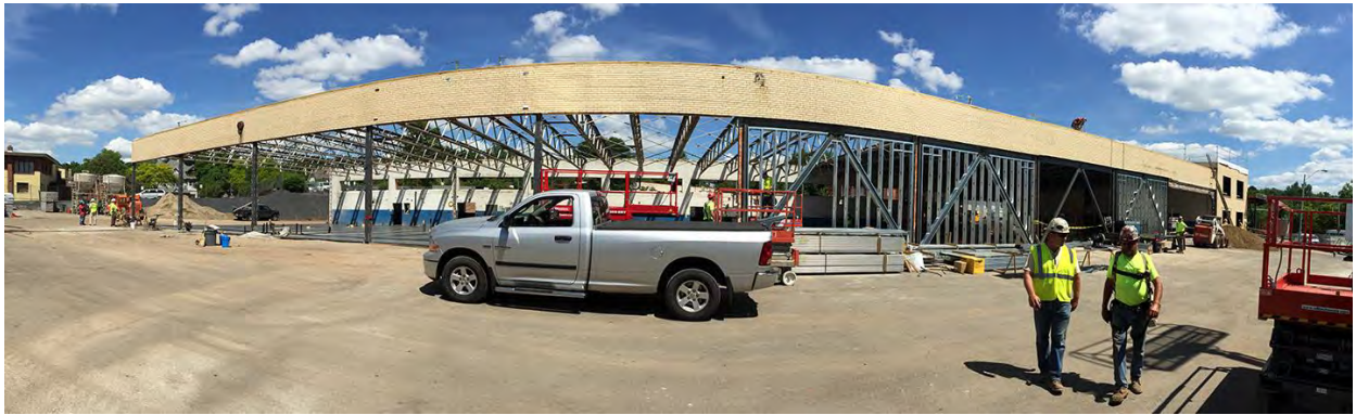
05-29-15 Mission Core and Shell Progress
