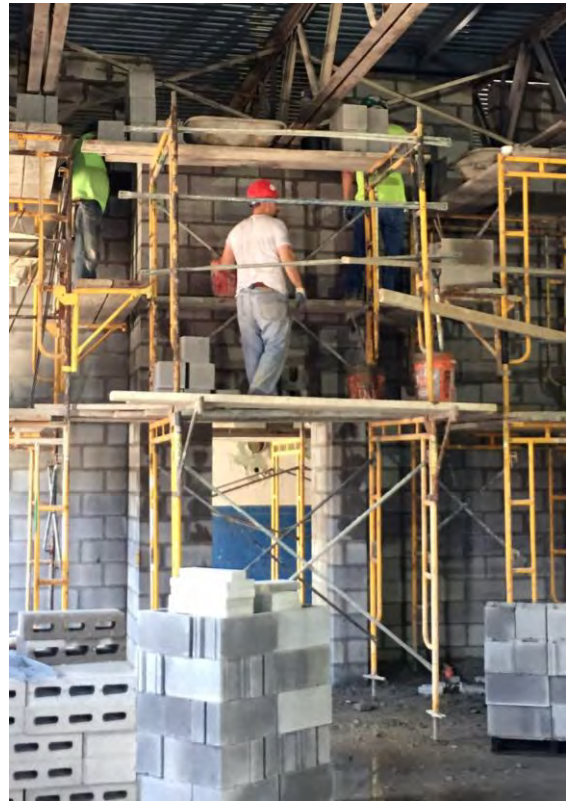
06-10-15 Mission Construction Progress
