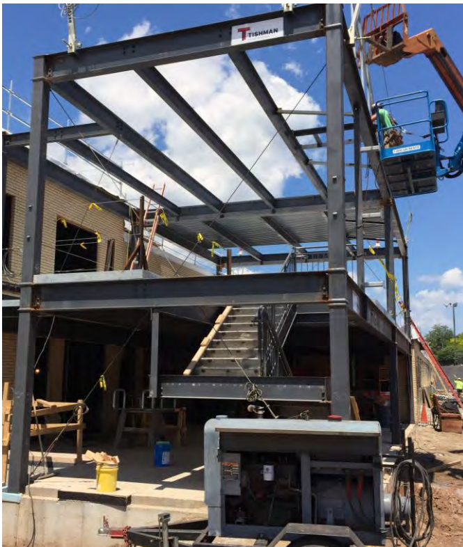
06-22-15 Mission Construction Progress
