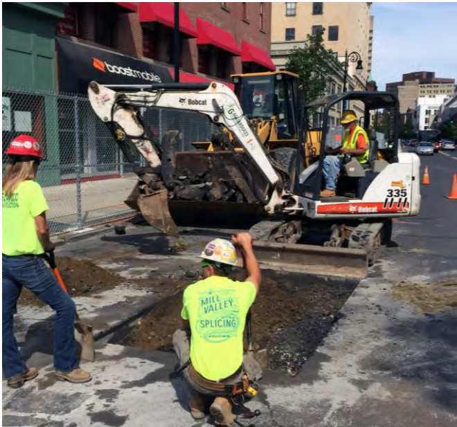
06-17-15 Cut and Cap Utility Progress
