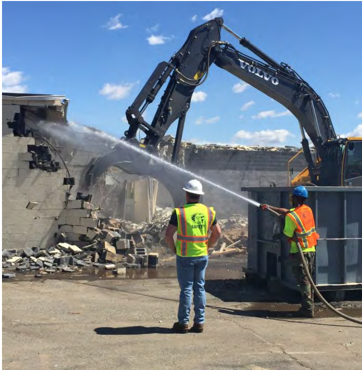
04-29-15 Car Wash Demolition
