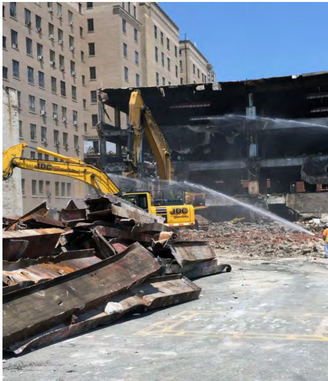
06-30-15 Demolition of Garage at State and Bliss
