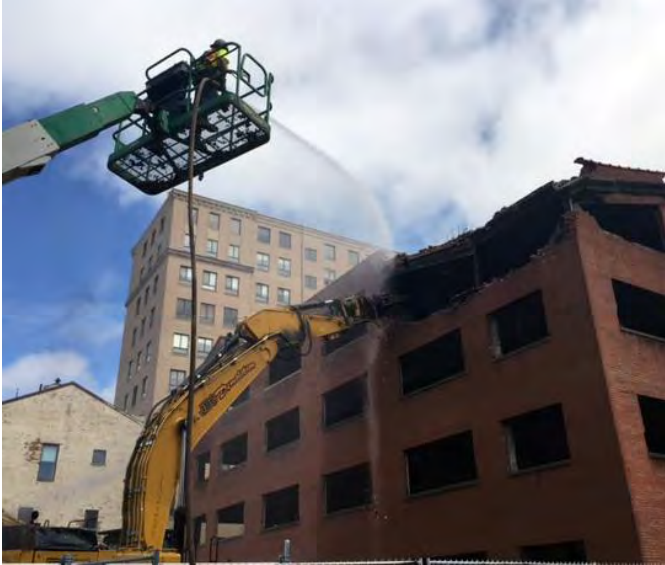
06-29-15 Demolition of Garage at State and Bliss
