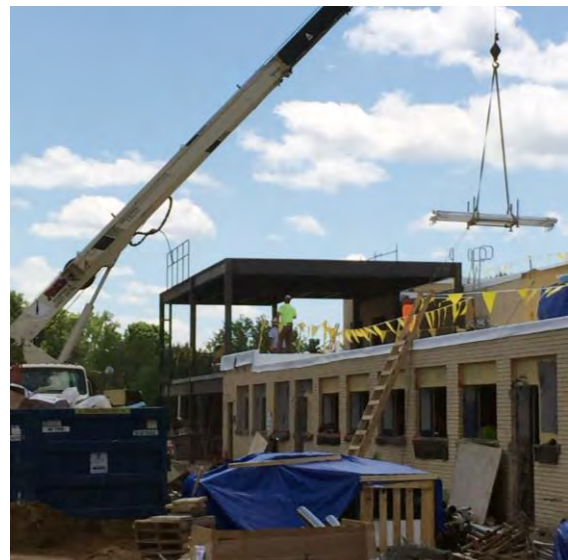
06-26-15 Mission Construction Progress
