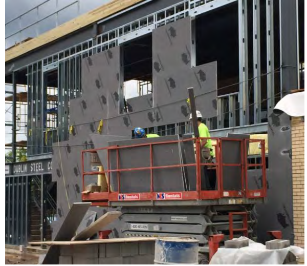
06-29-15 Mission Construction Progress
