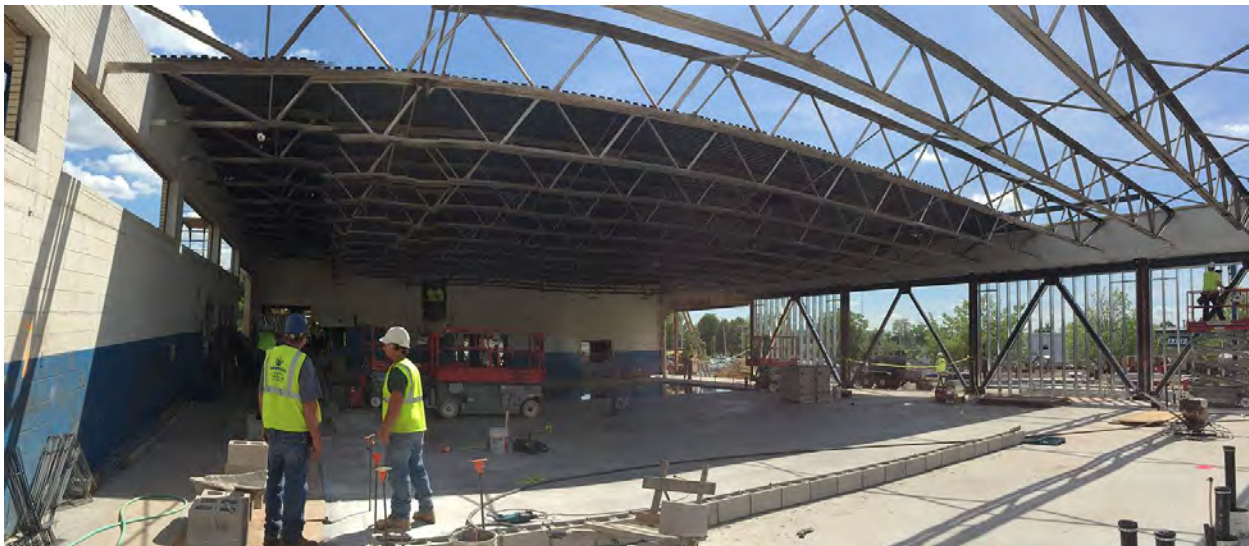
05-29-15 Mission Core and Shell Progress
