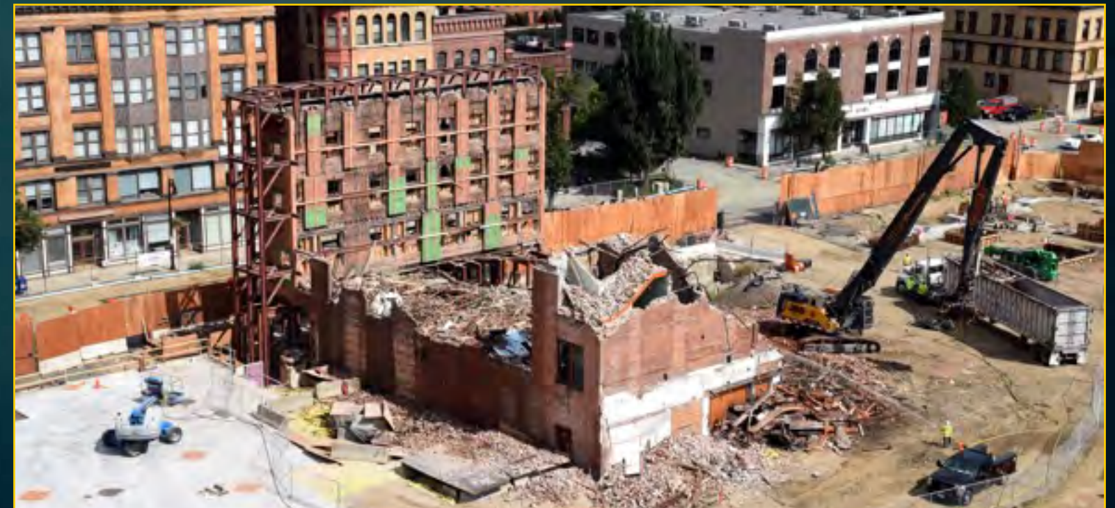
Union Chandler Rear Portion Demolition - September 14, 2016
