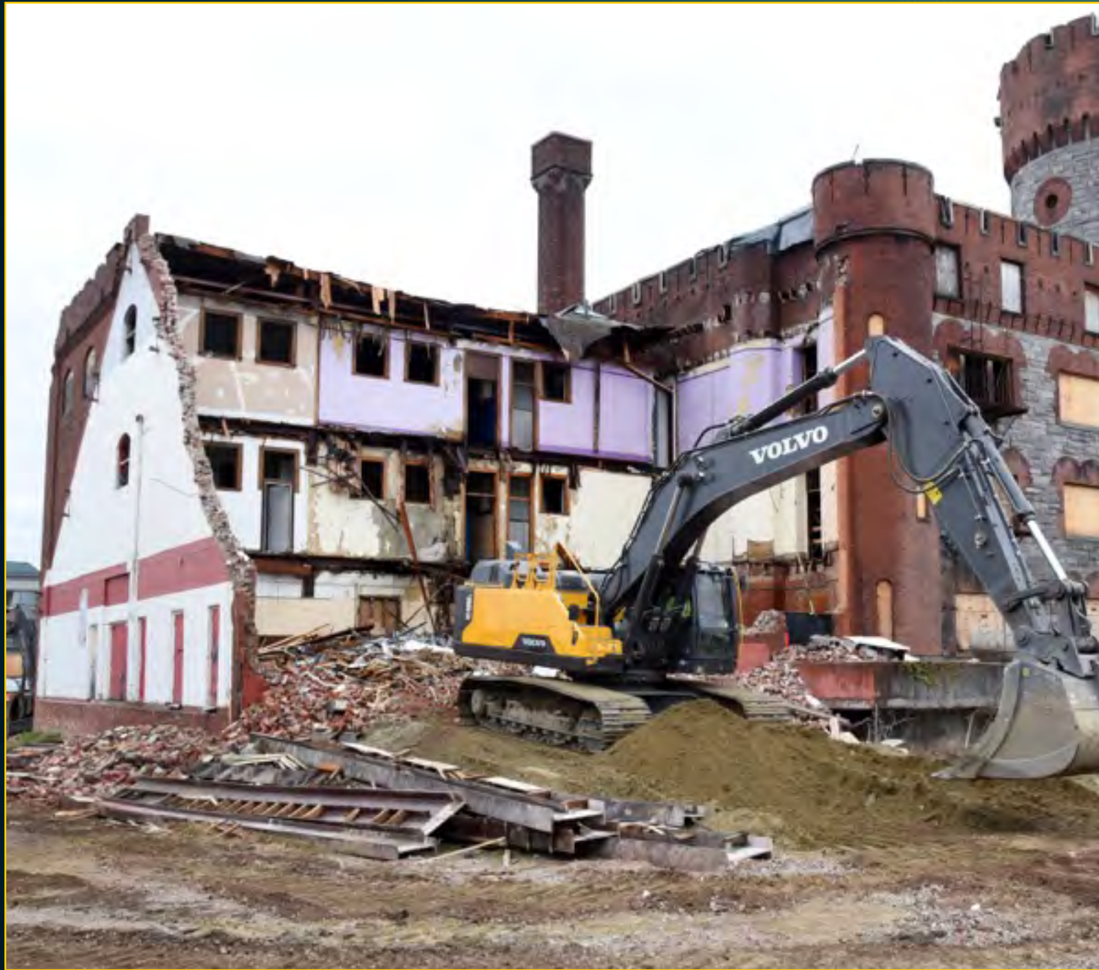
Armory Demolition - May 5, 2016
