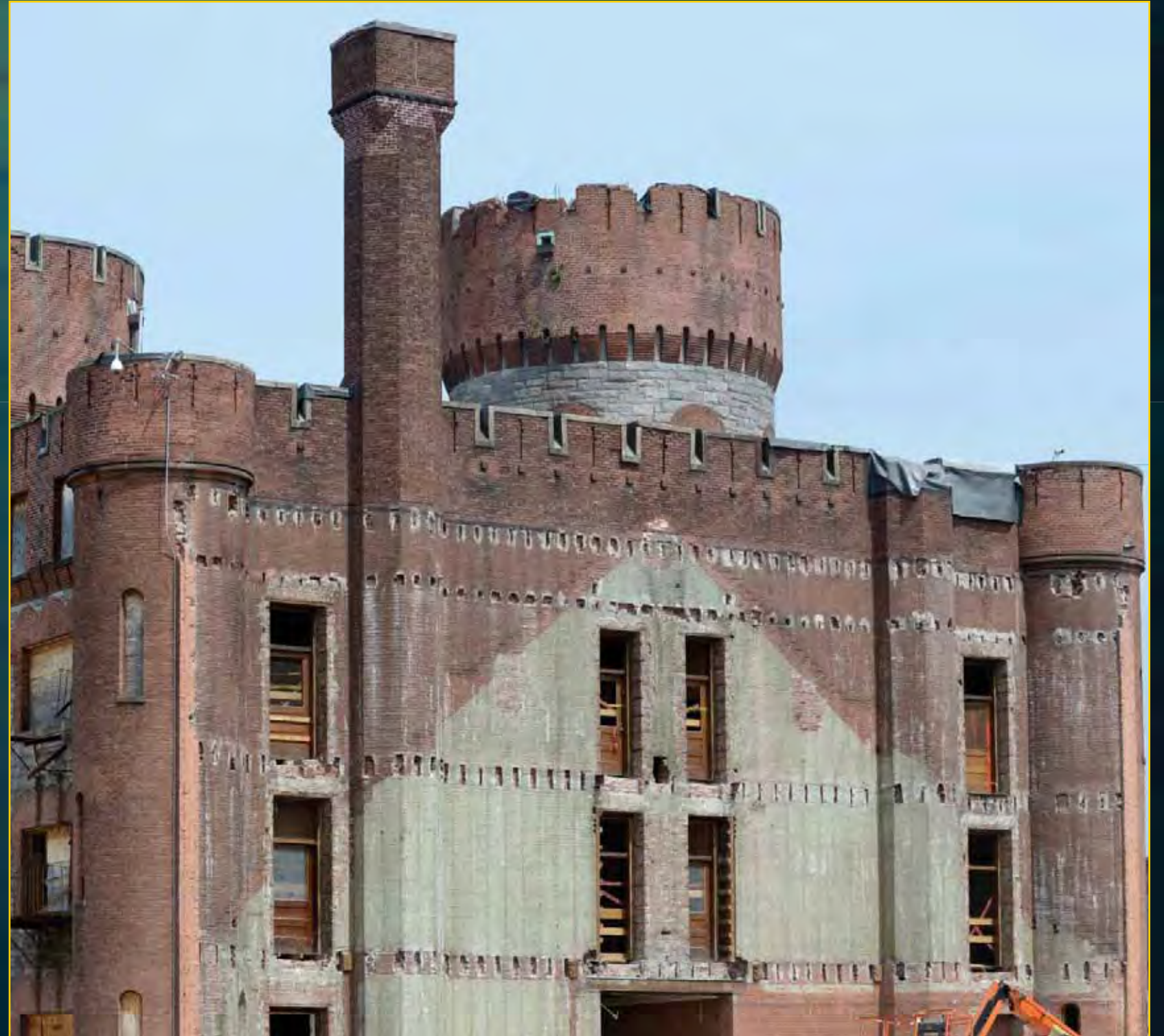
Armory Back Completion - May 26, 2016
