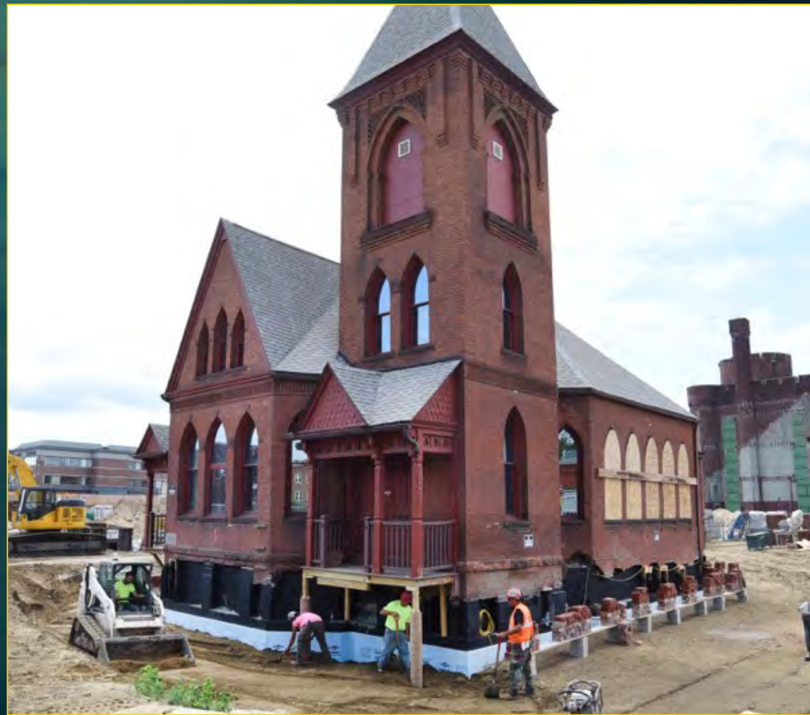
New Church Foundation - June 28, 2016
