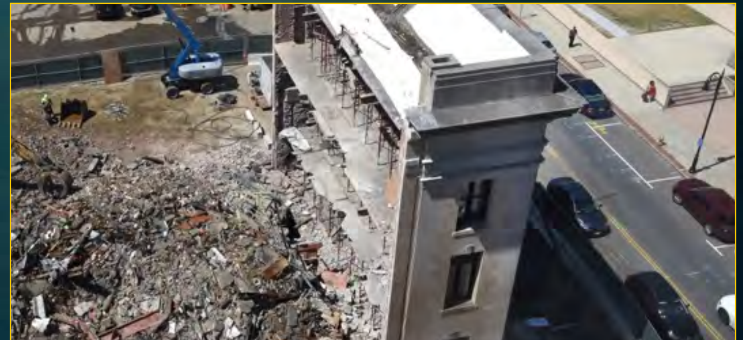
73 State Demolition - June 24, 2016
