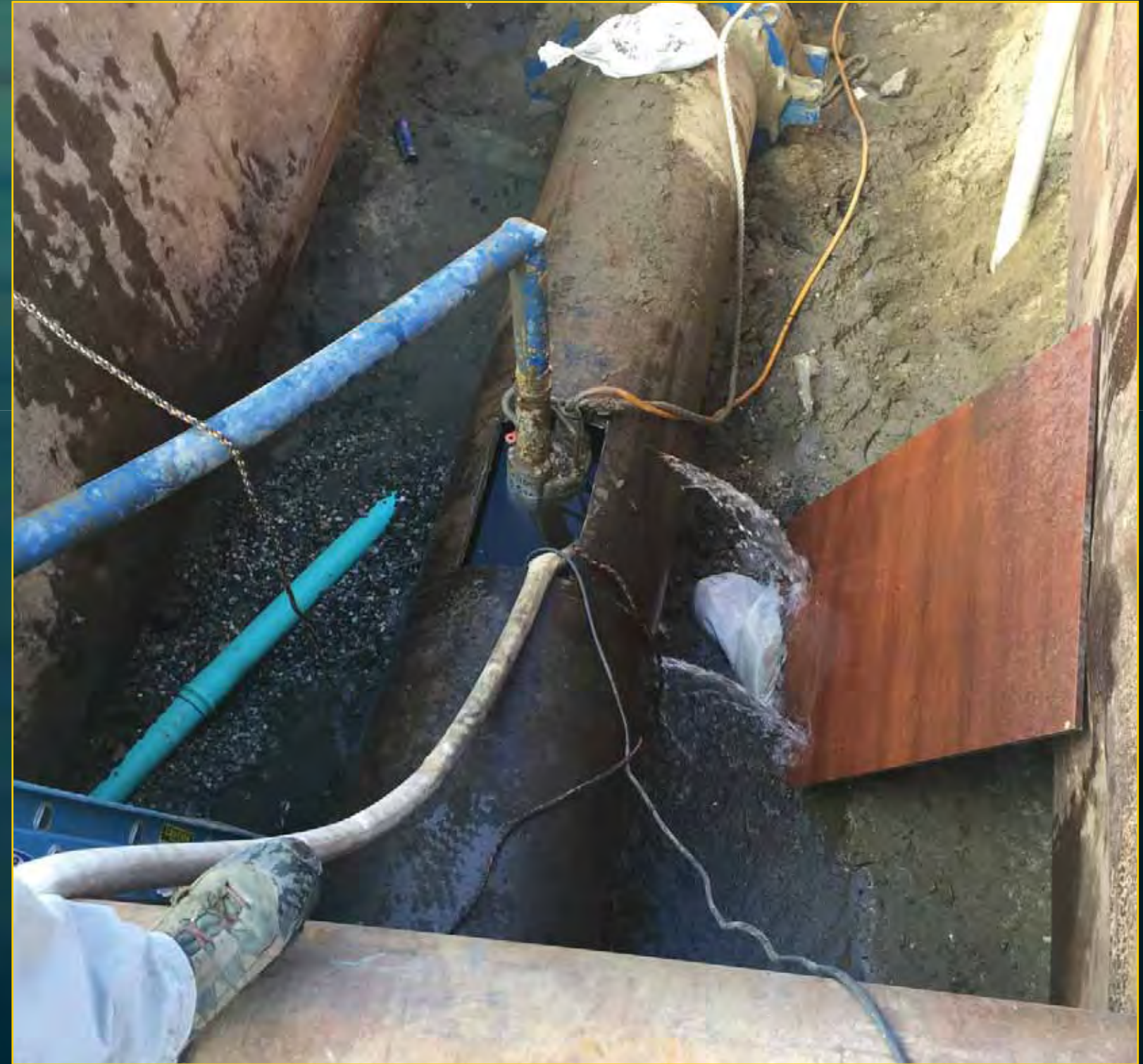
Offsite Utility Work - June 13, 2016
