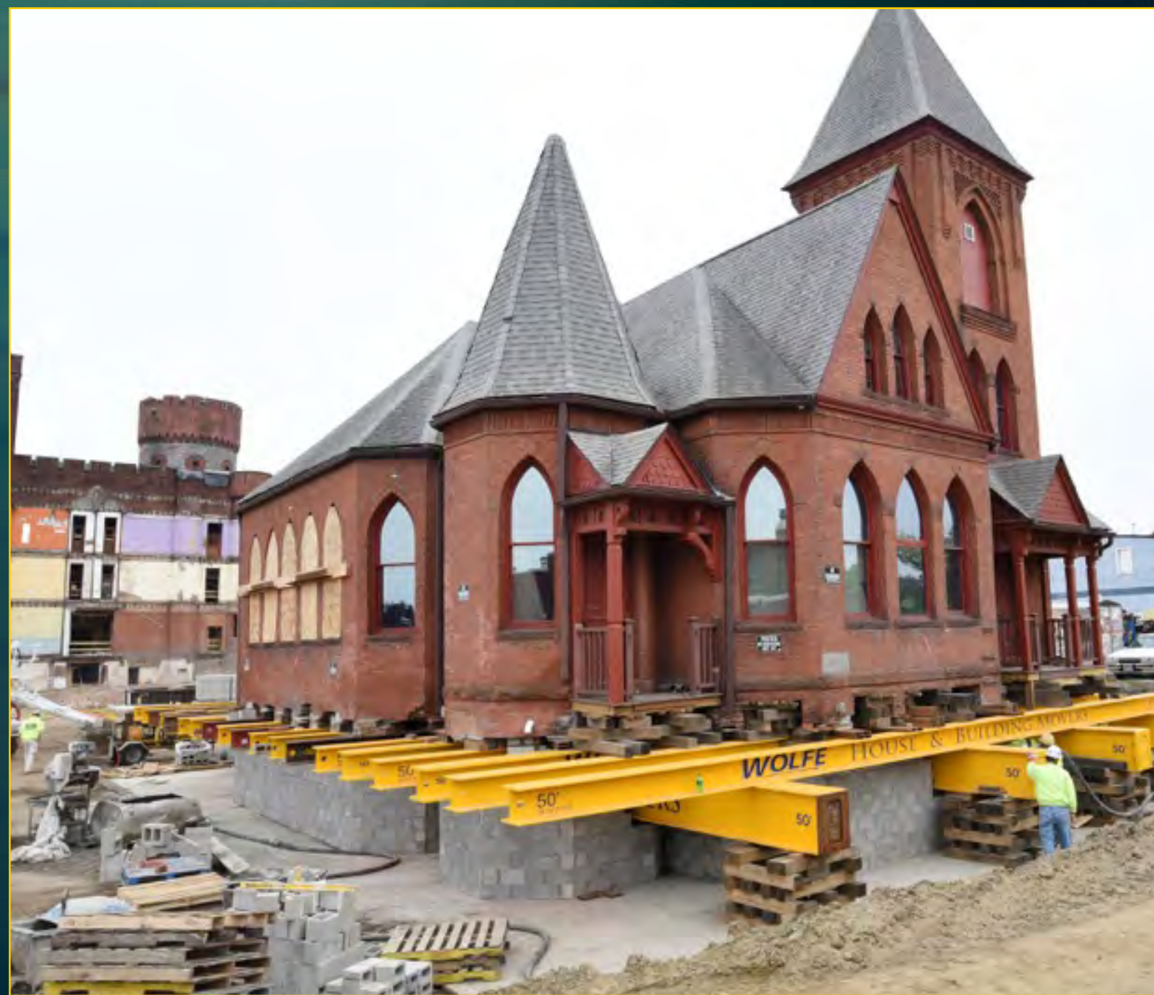
New Church Foundation - May 17, 2016
