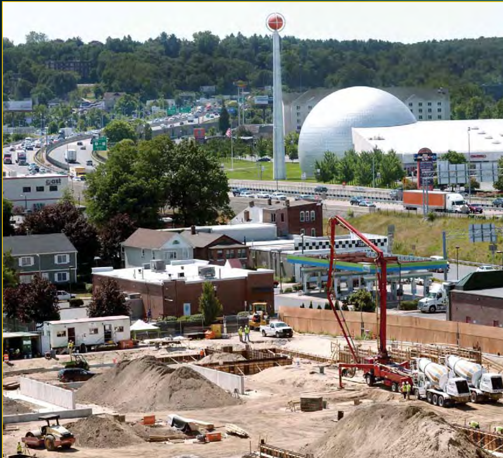
Garage Construction - June 24, 2016
