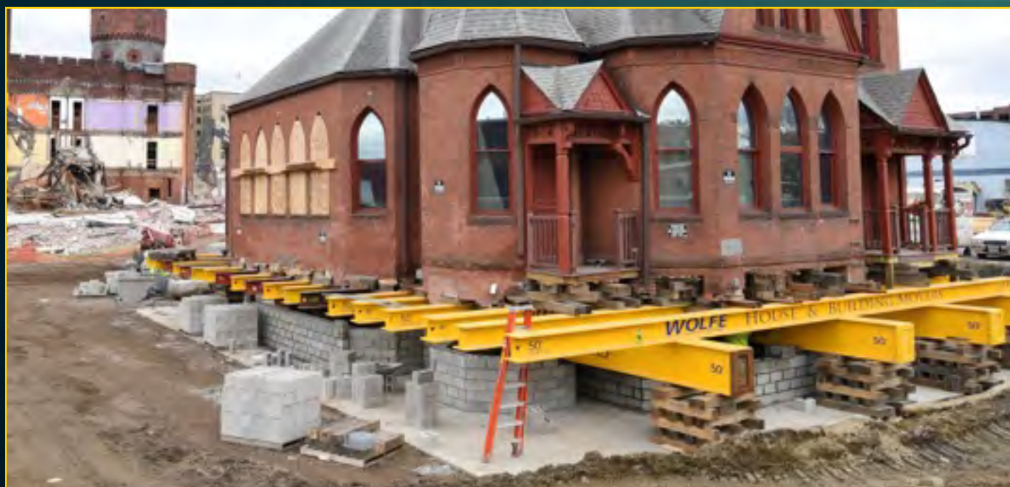
New Church Foundation - May 6, 2016
