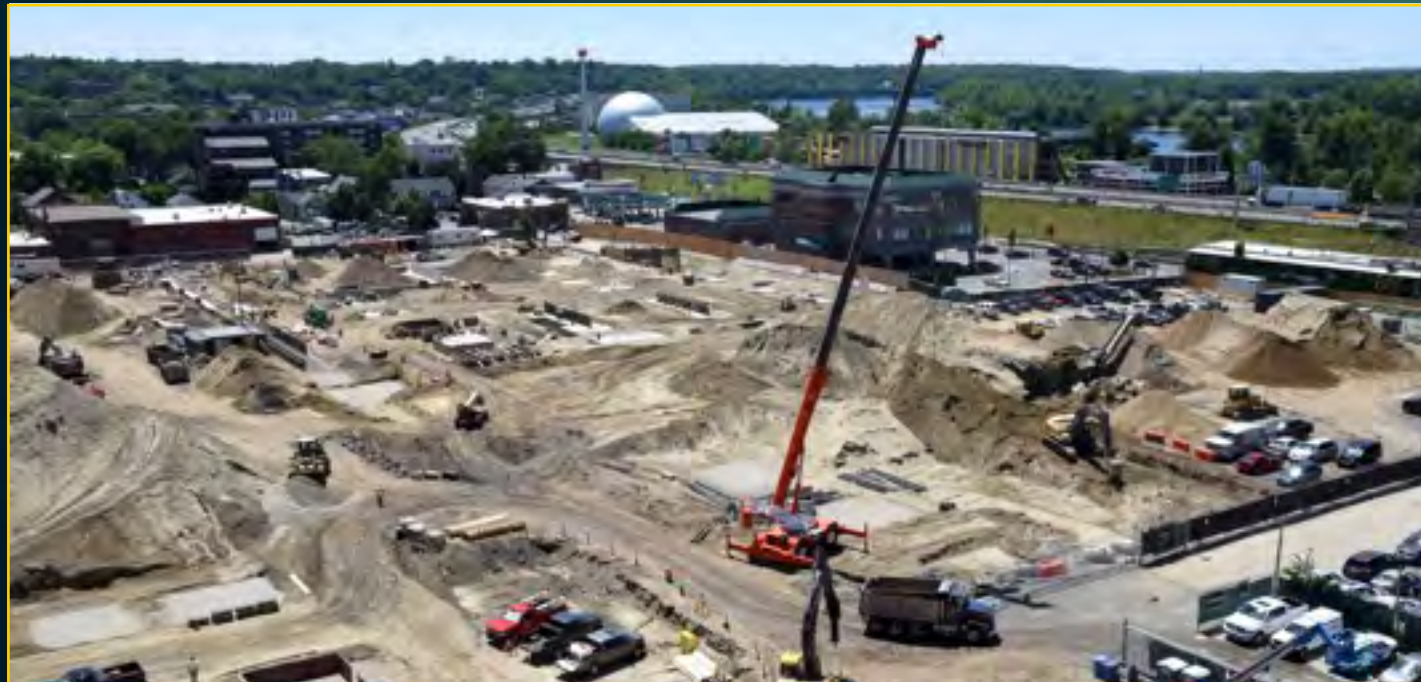
Podium Footings Prepared - June 21, 2016
