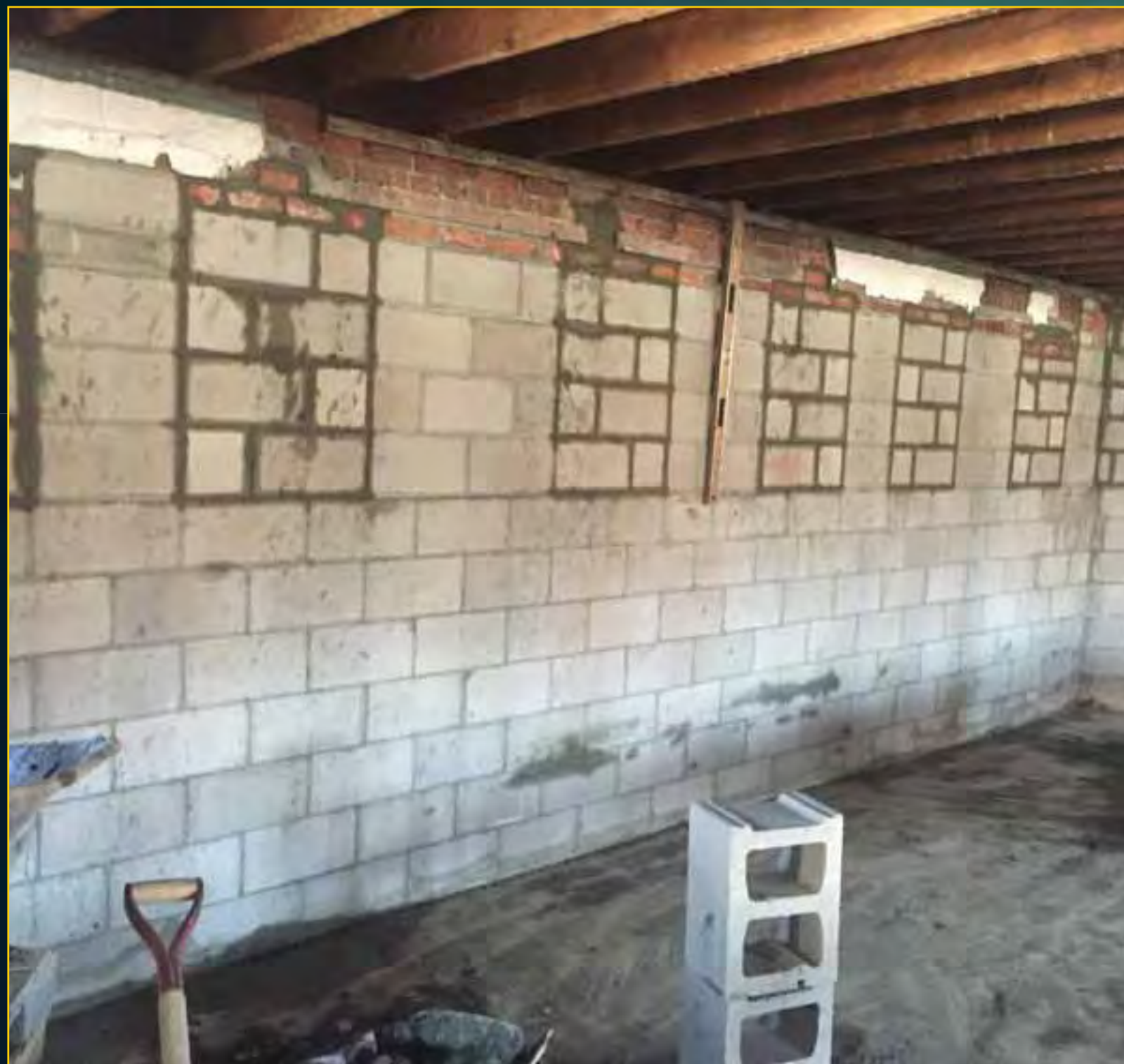
New Church Foundation - June 20, 2016
