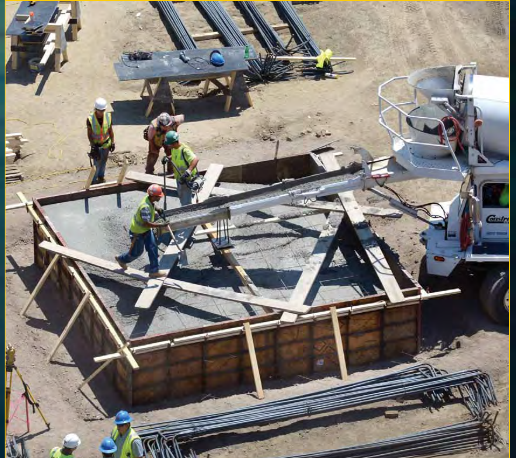
Podium Footings Prepared - June 25, 2016
