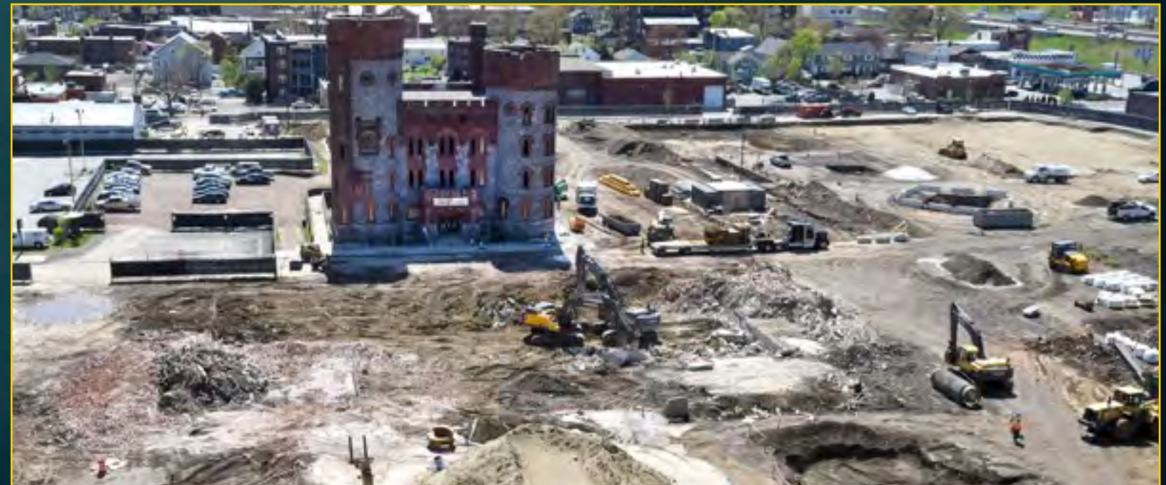
YWCA Site Cleared - April 27, 2016
