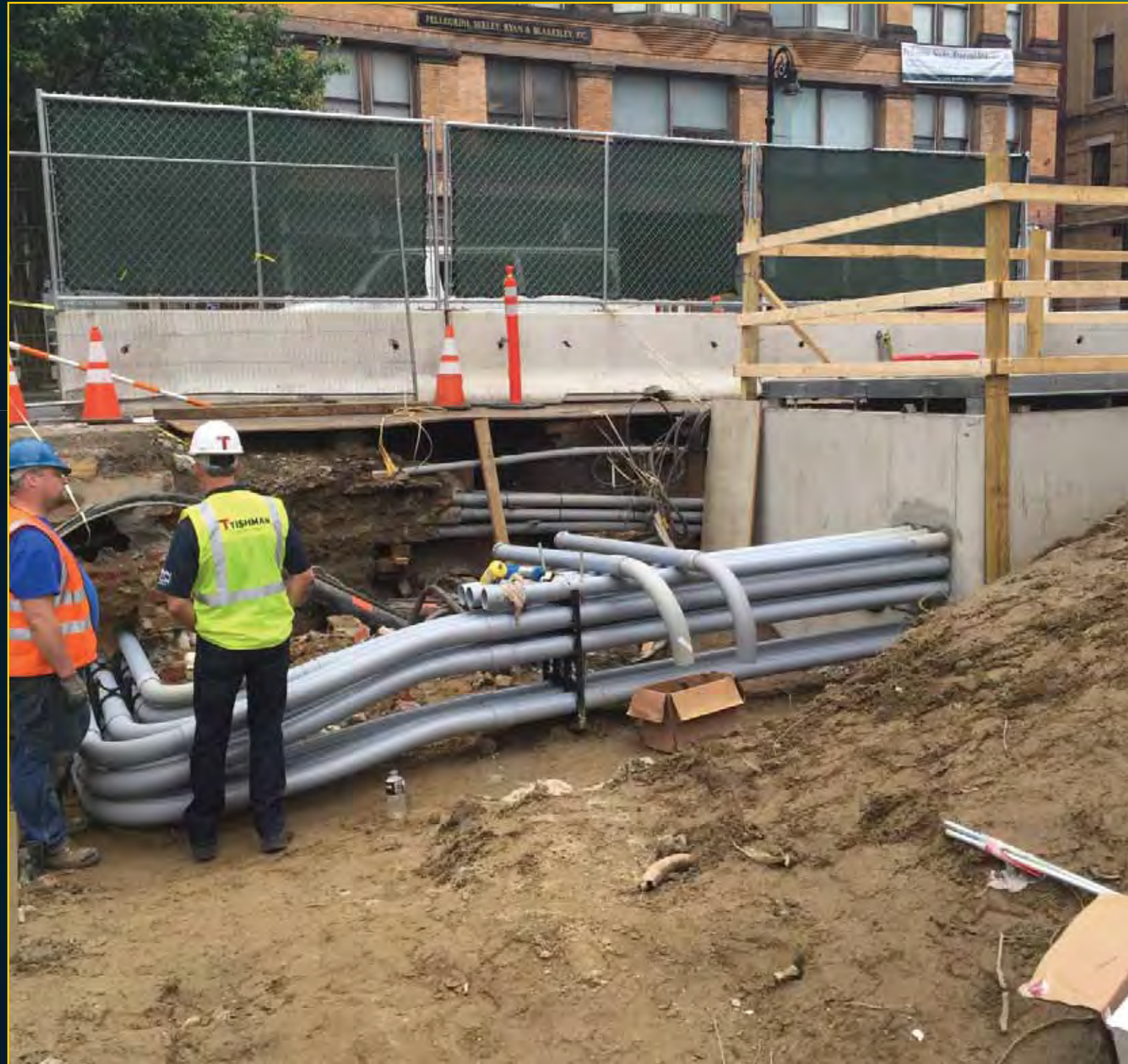
Vault Progress - May 24, 2016
