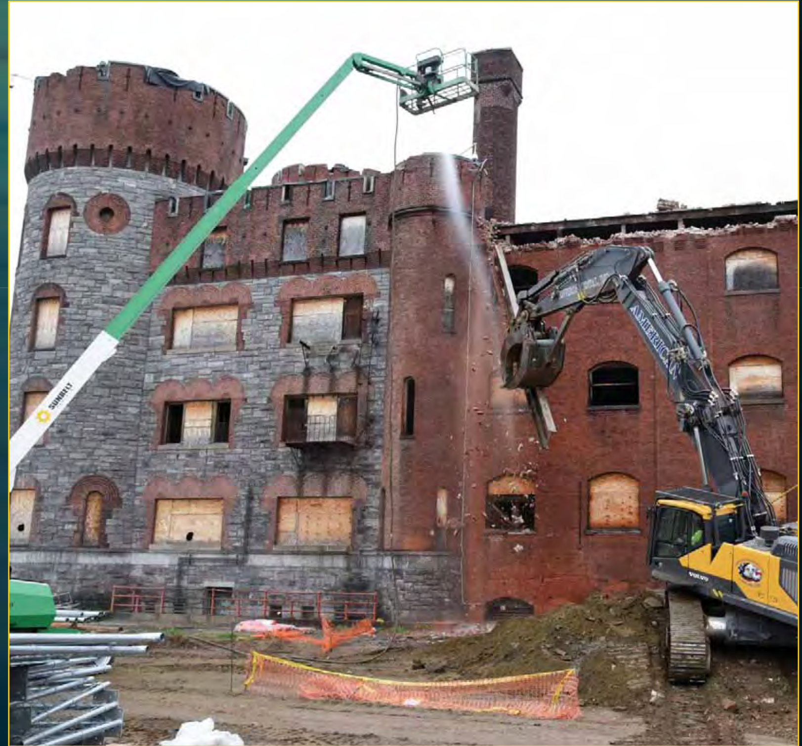
Armory Demolition - May 5, 2016
