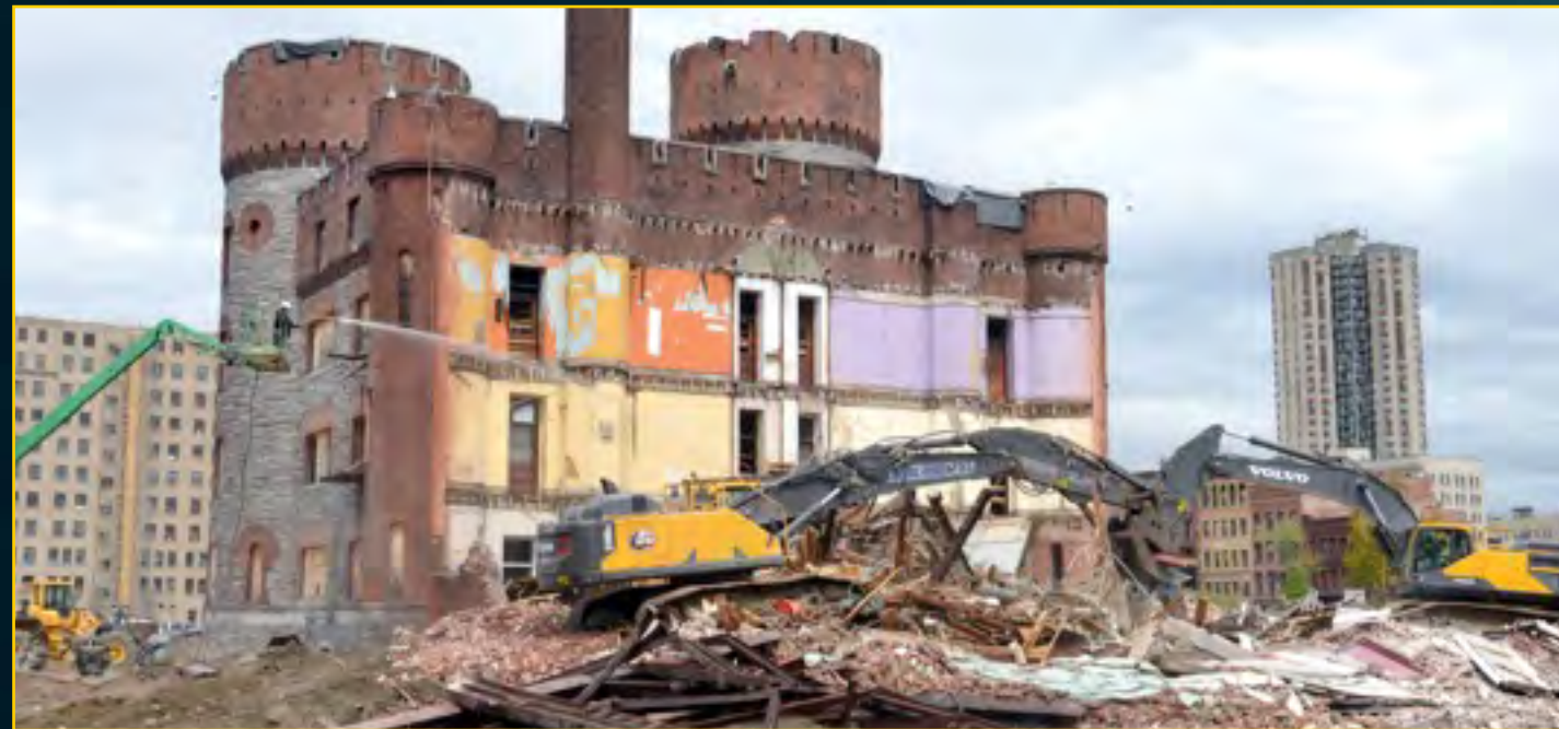
Armory Back Demolition - May 6, 2016
