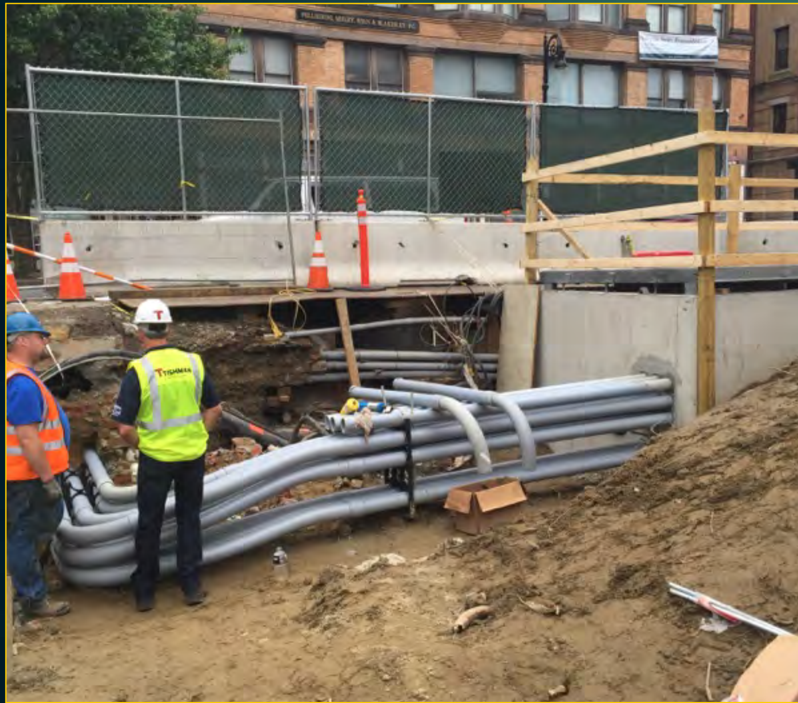
Vault Progress - May 24, 2016
