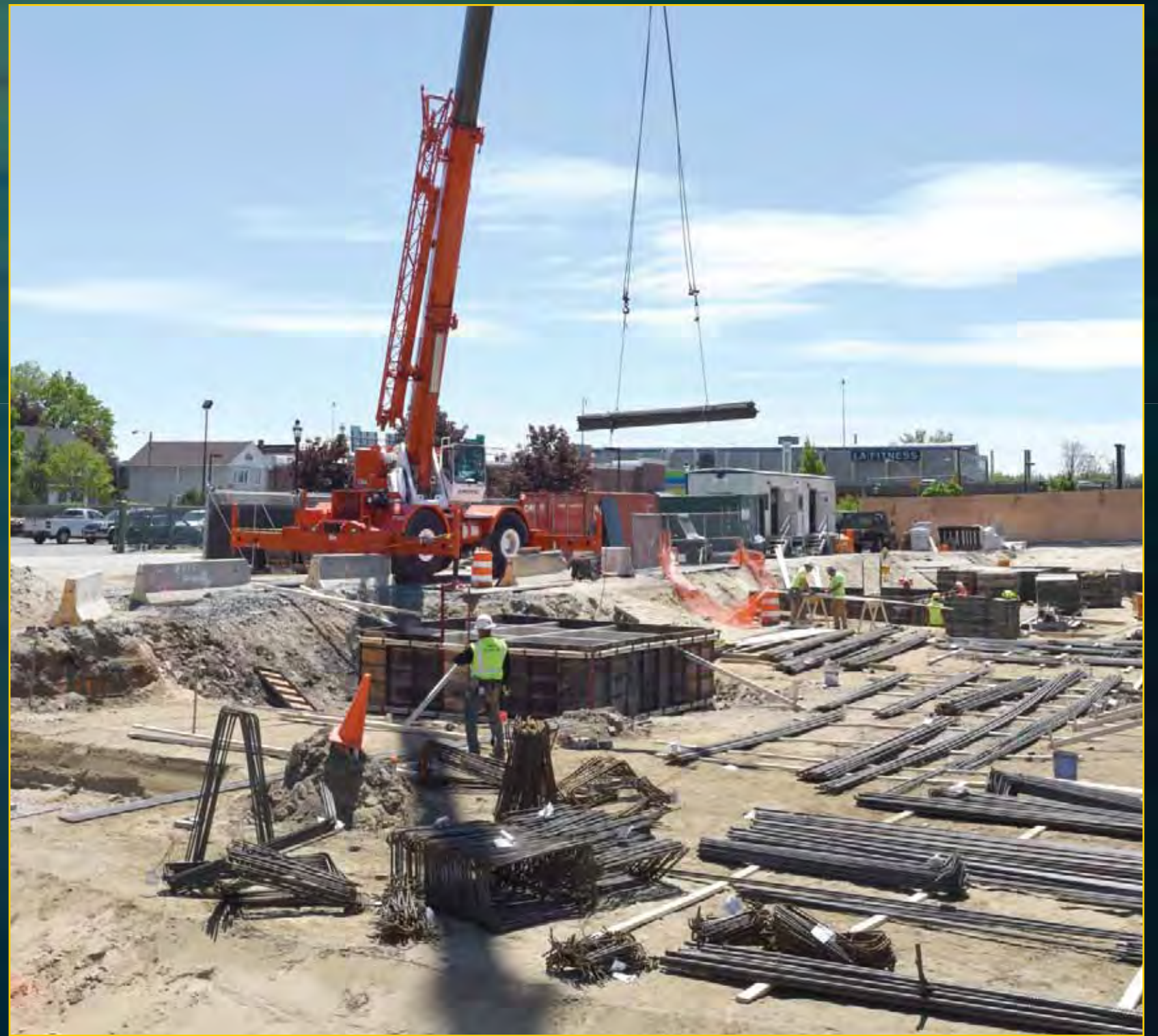
Garage Construction - May 18, 2016
