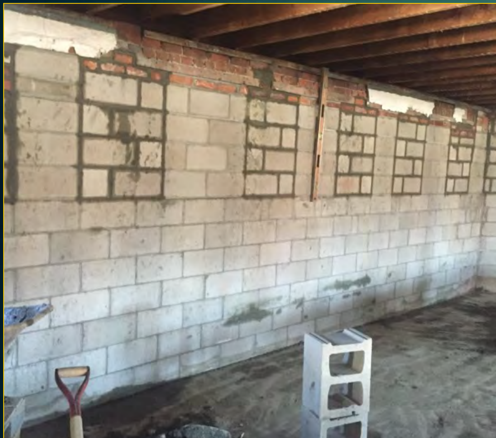
New Church Foundation - June 20, 2016
