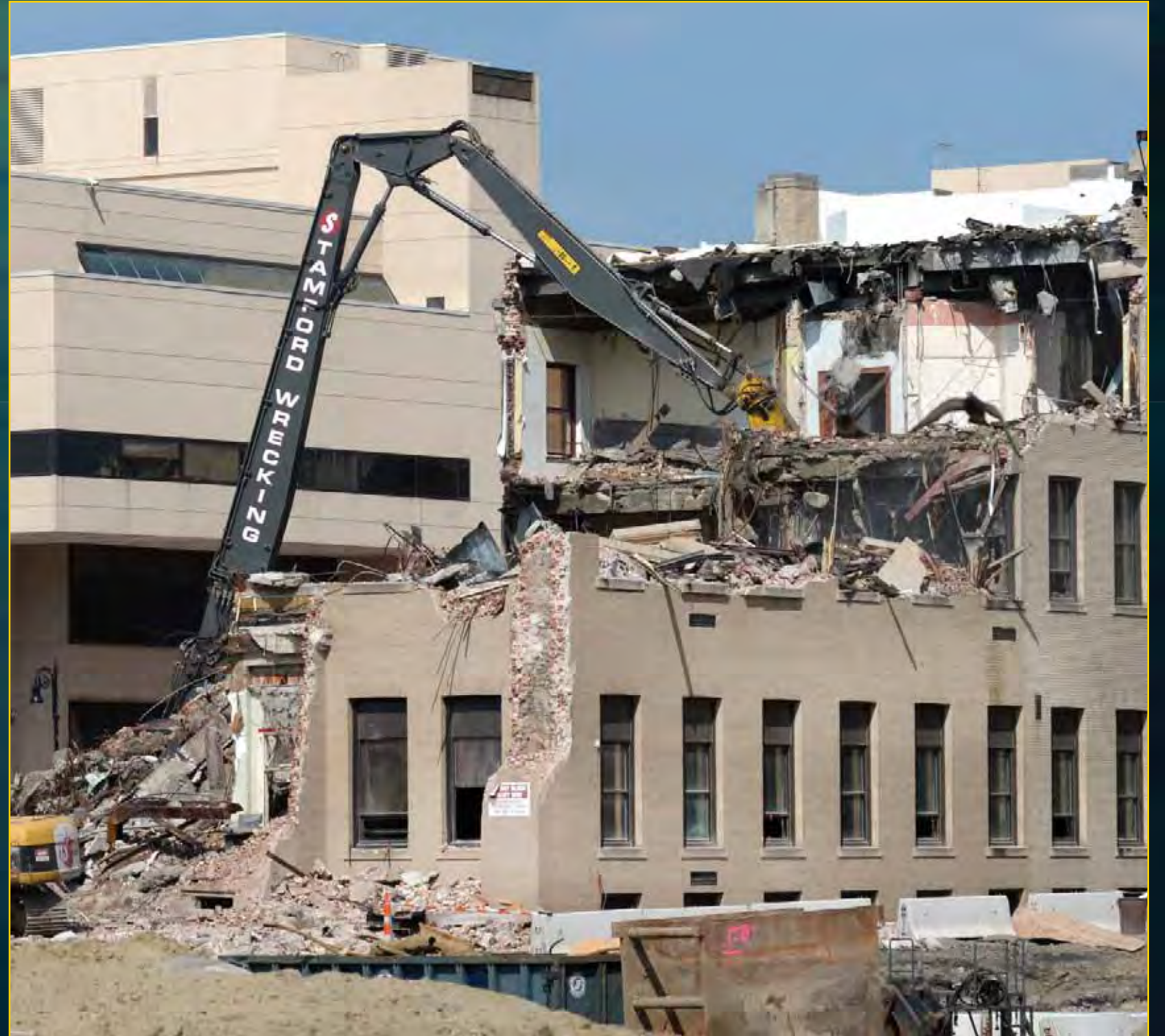
73 State Demolition - June 20, 2016
