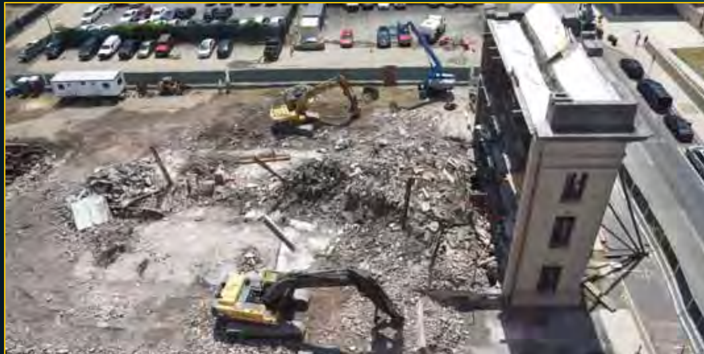
73 State Demolition - June 28, 2016
