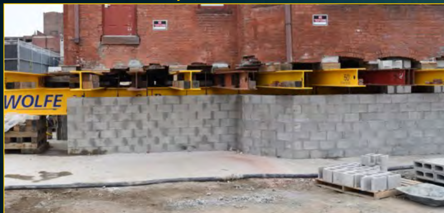
New Church Foundation - May 17, 2016
