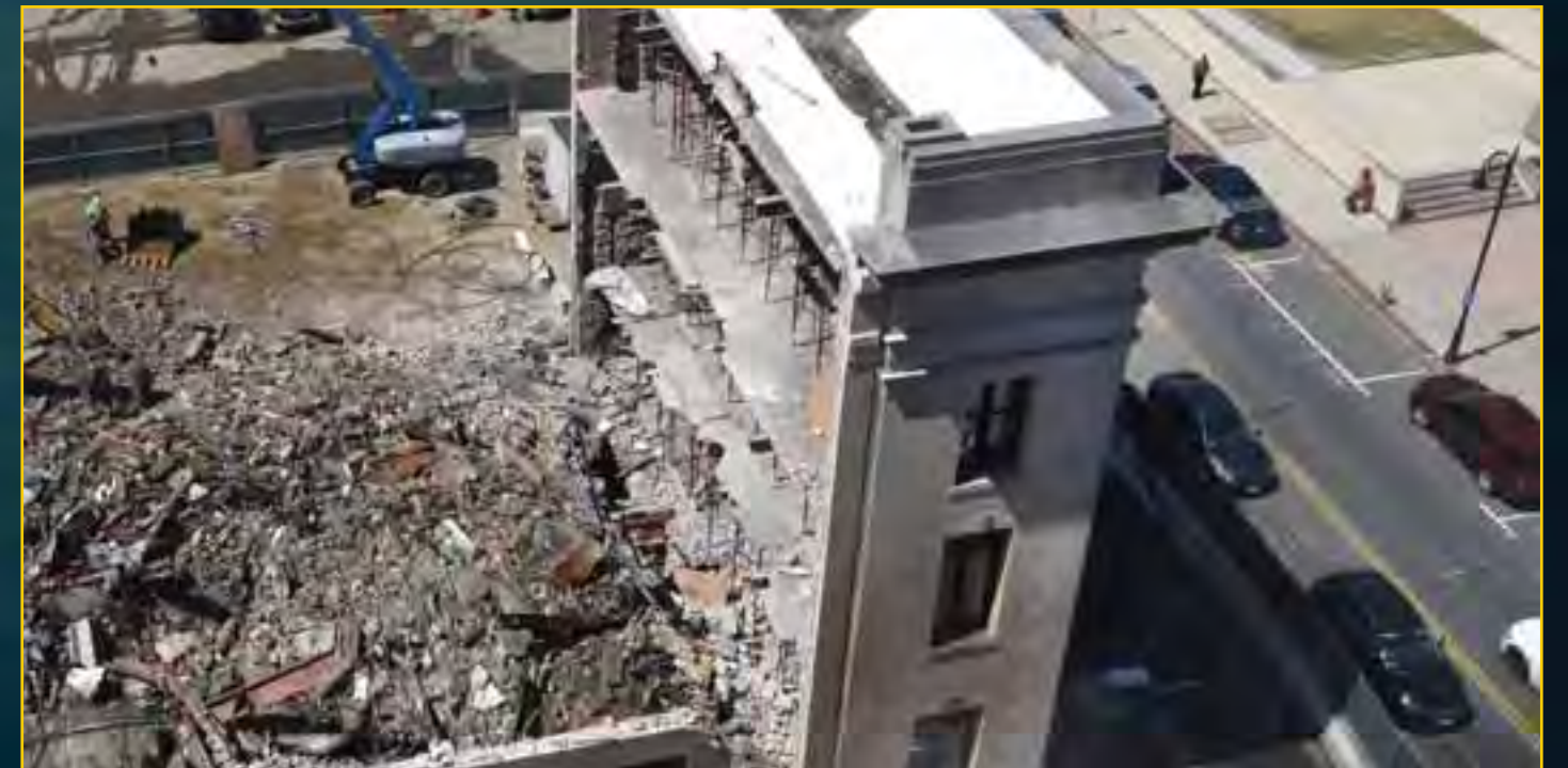
73 State Demolition - June 24, 2016
