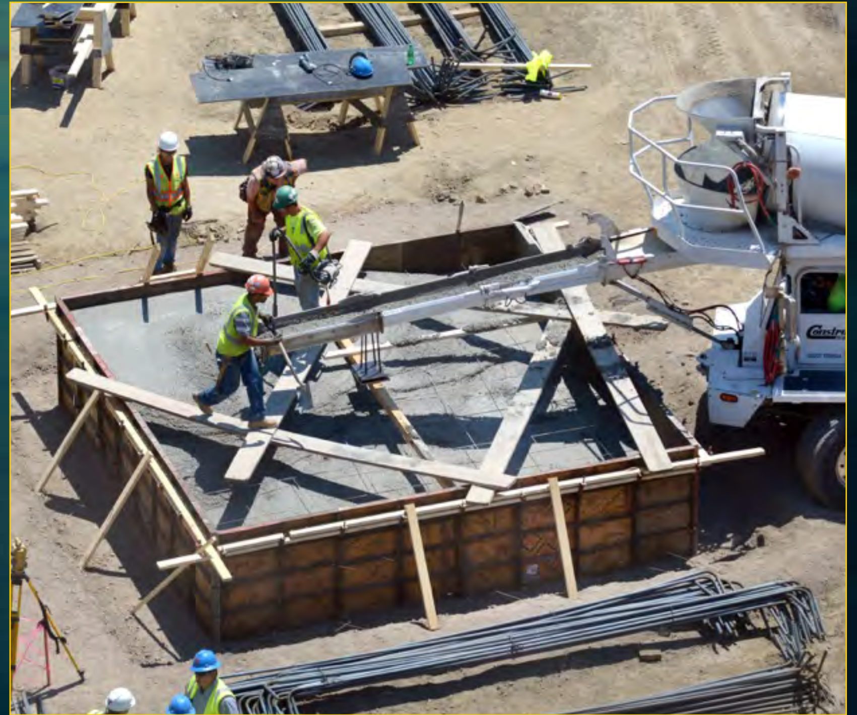
Podium Footings Prepared - June 25, 2016
