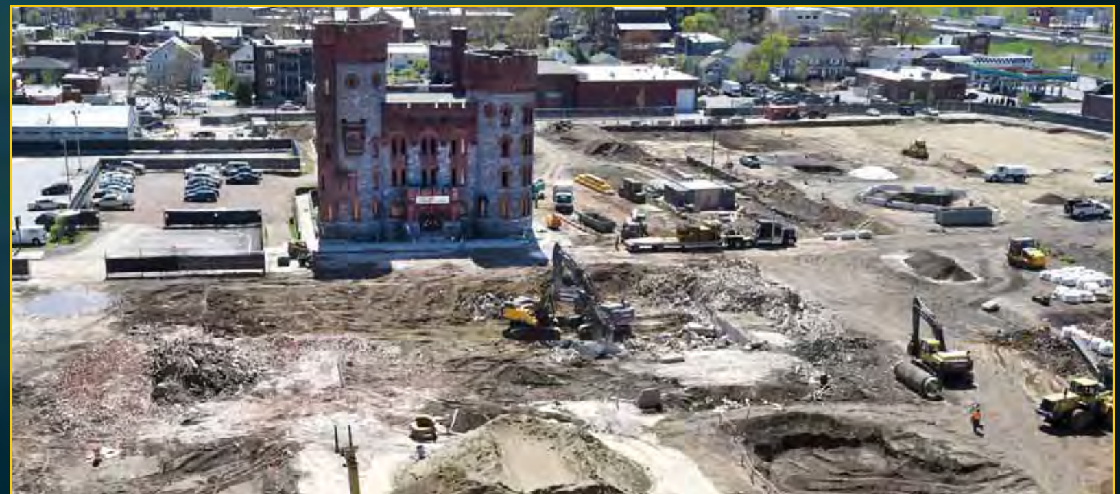
YWCA Site Cleared - April 27, 2016
