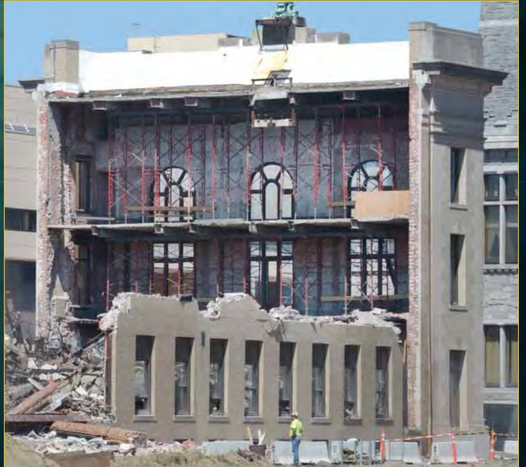
73 State Demolition - June 24, 2016
