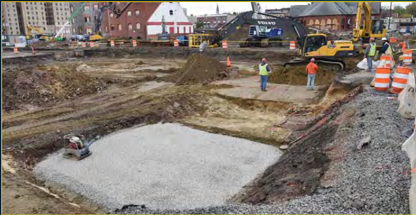
Garage Footings - May 5, 2016
