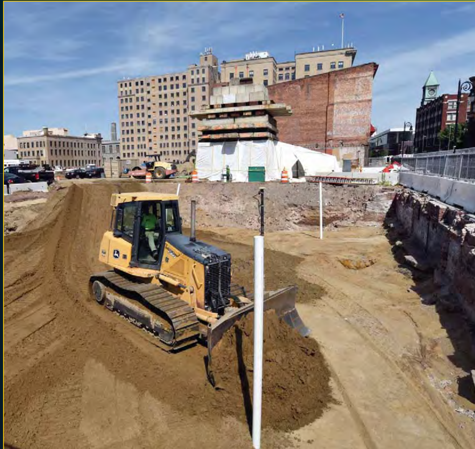
Backfill Along Main Street - June 1, 2016
