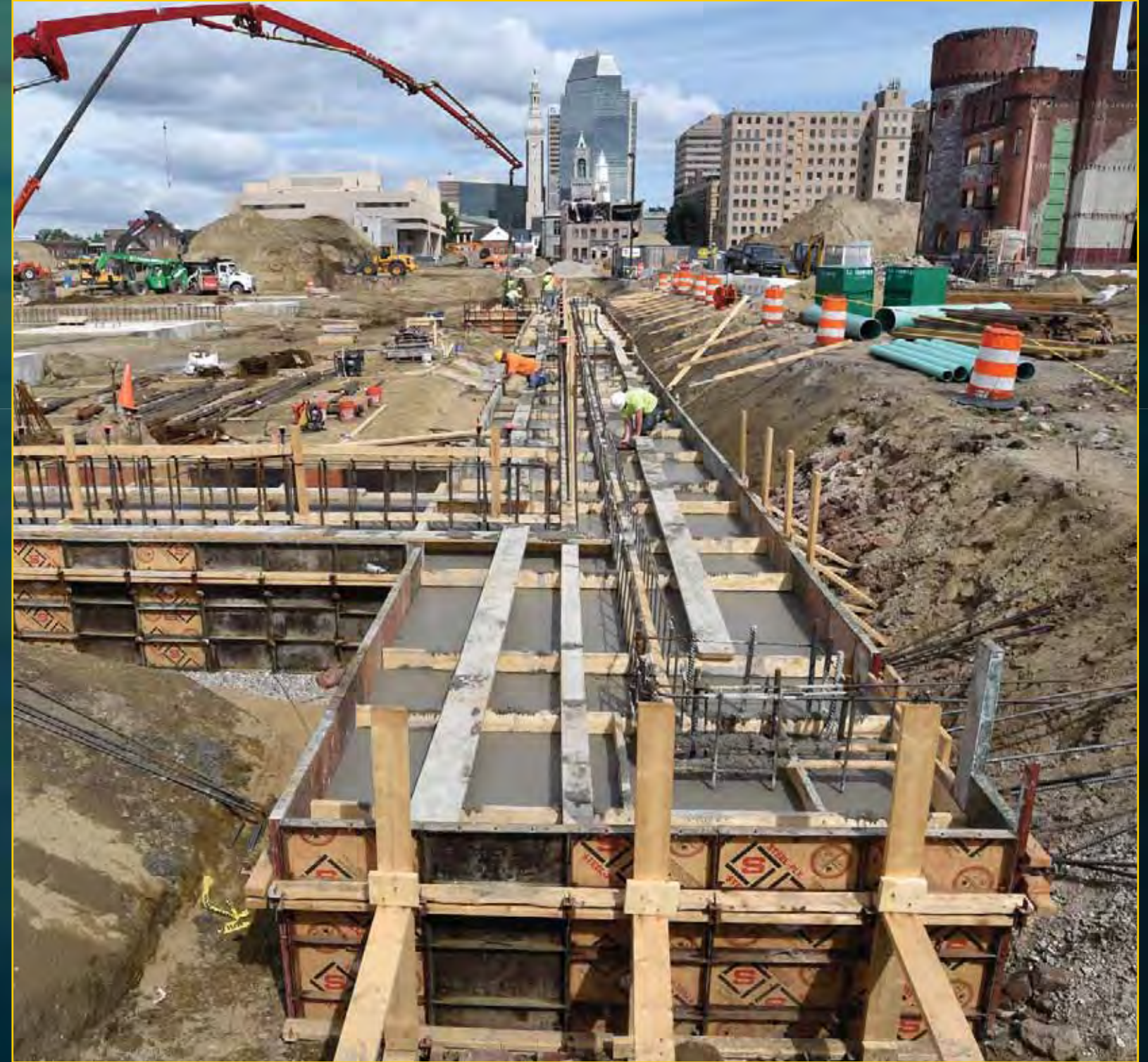
Garage Construction - June 8, 2016
