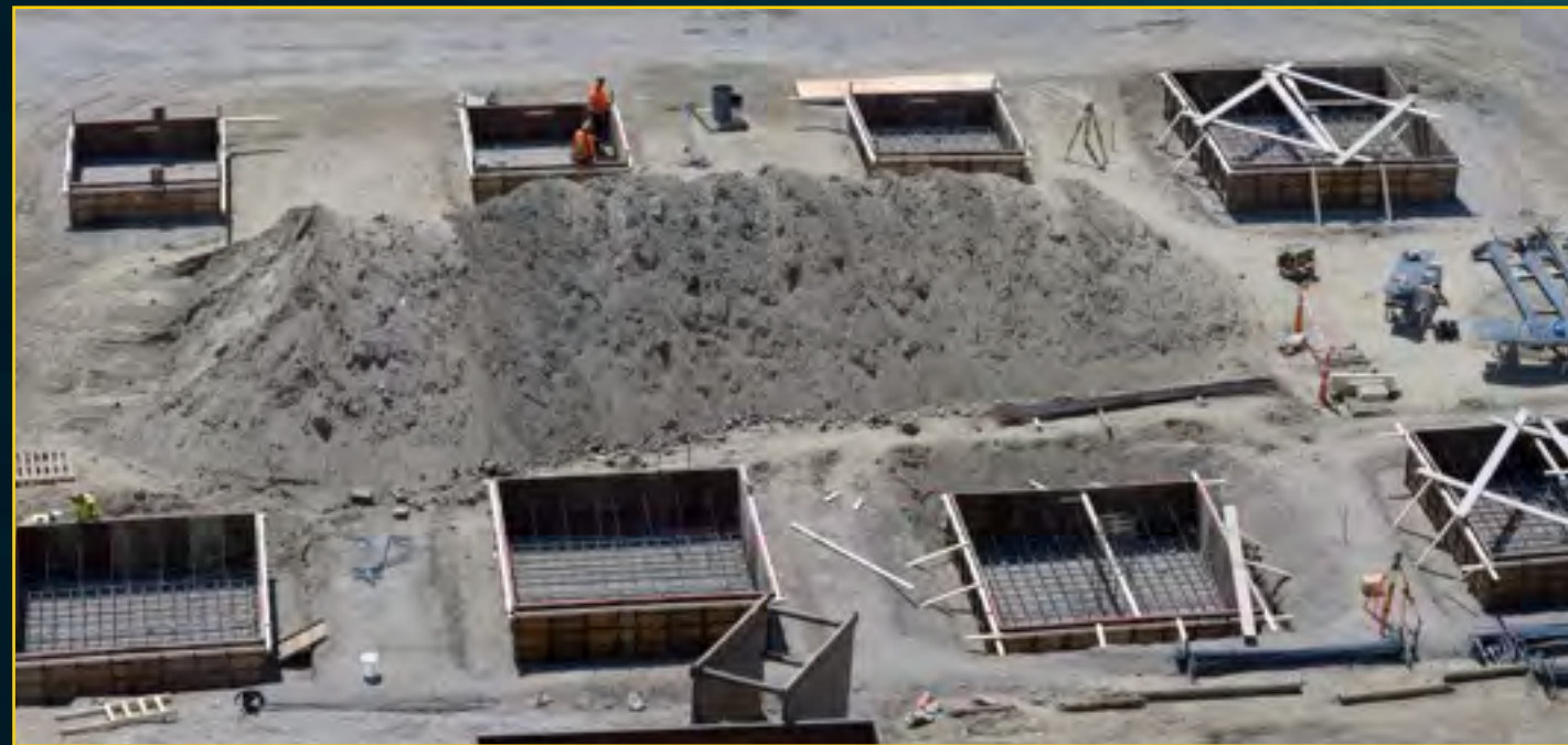
Podium Footings Prepared - June 21, 2016
