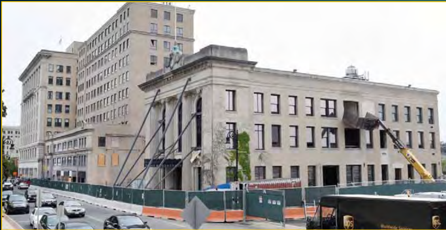
73 State Demolition - May 7, 2016
