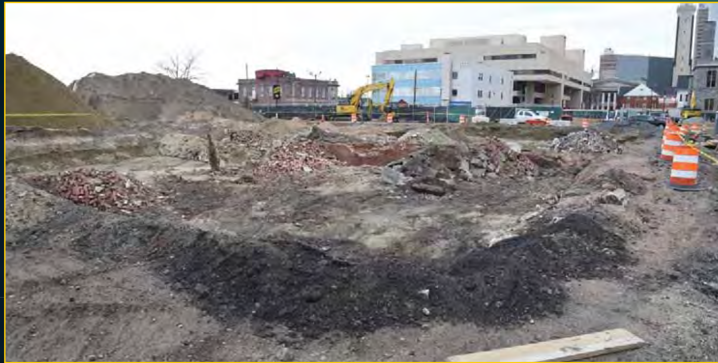
Garage Site Preparation - April 11, 2016
