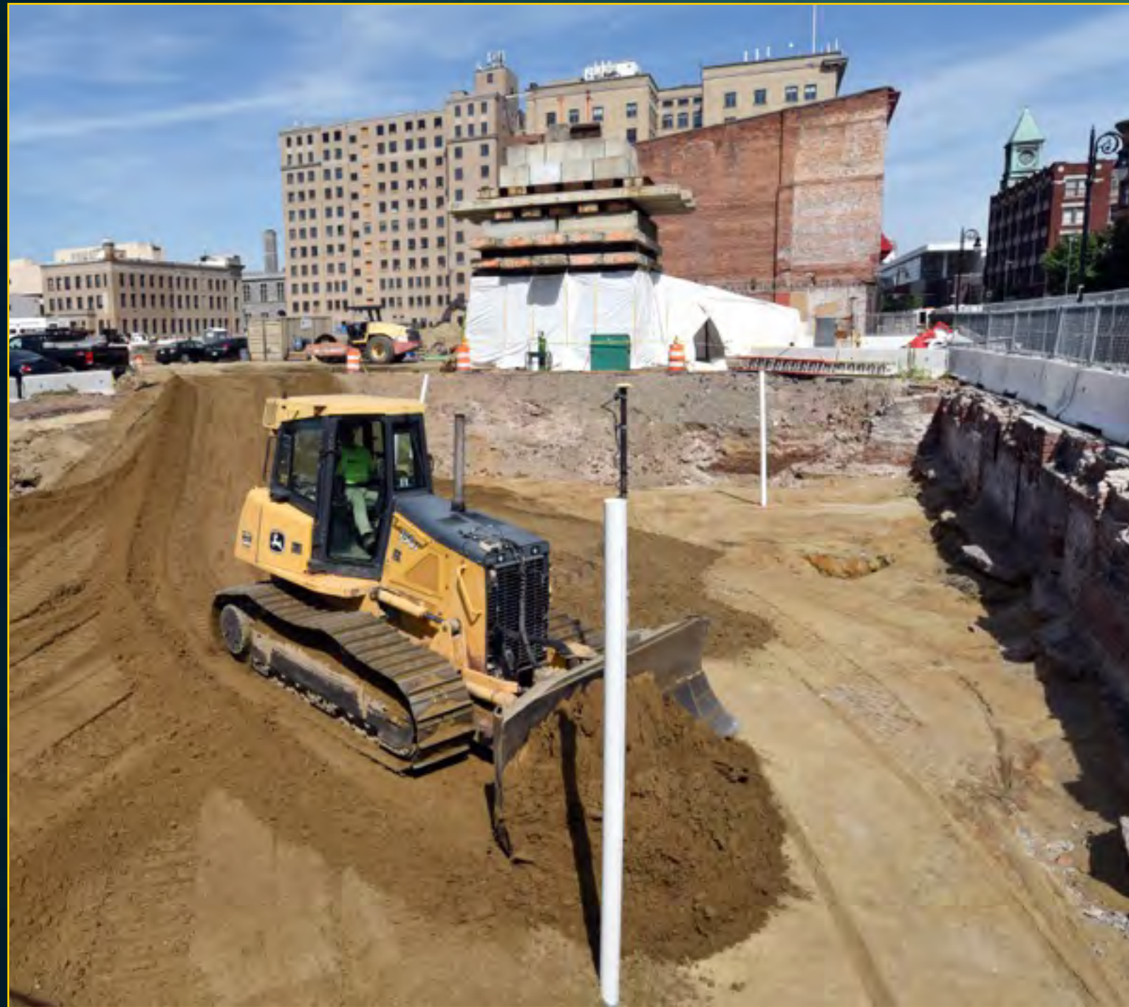
Backfill Along Main Street - June 1, 2016
