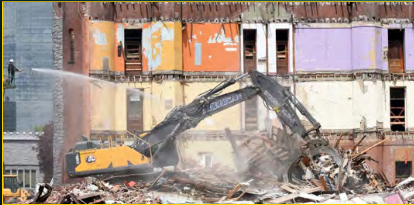
Armory Back Demolition - May 6, 2016
