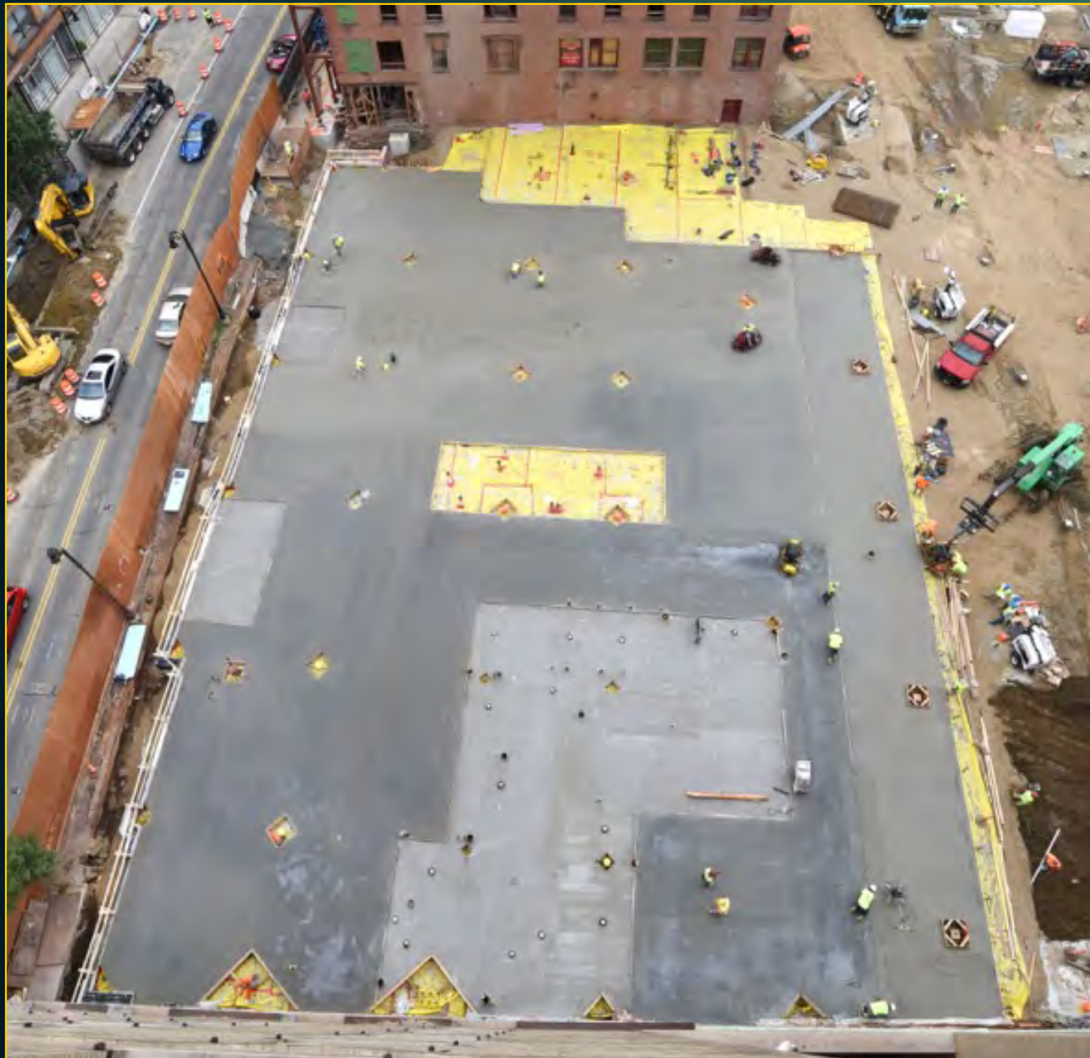
Hotel Foundation - August 17, 2016
