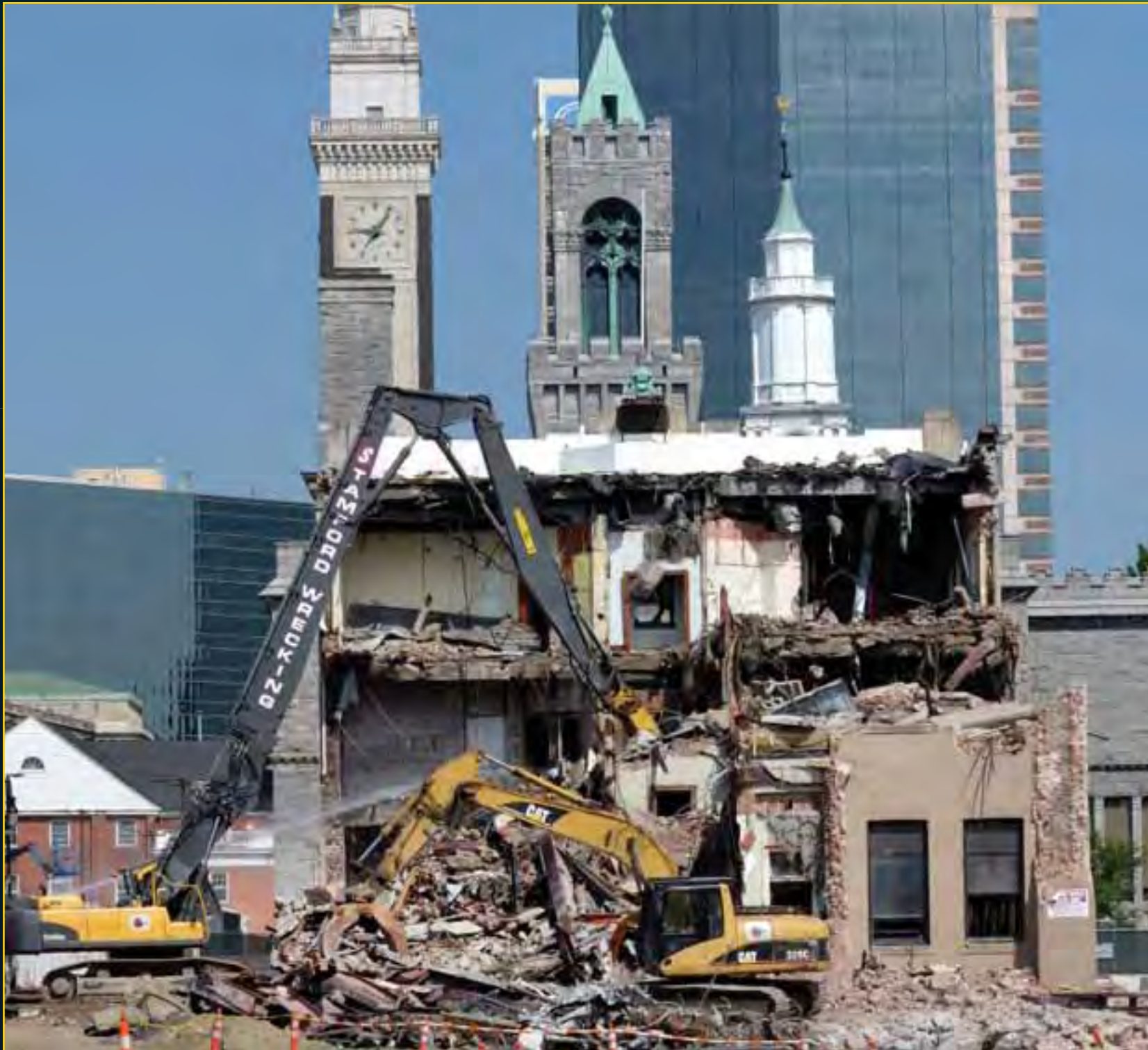
73 State Demolition - June 20, 2016
