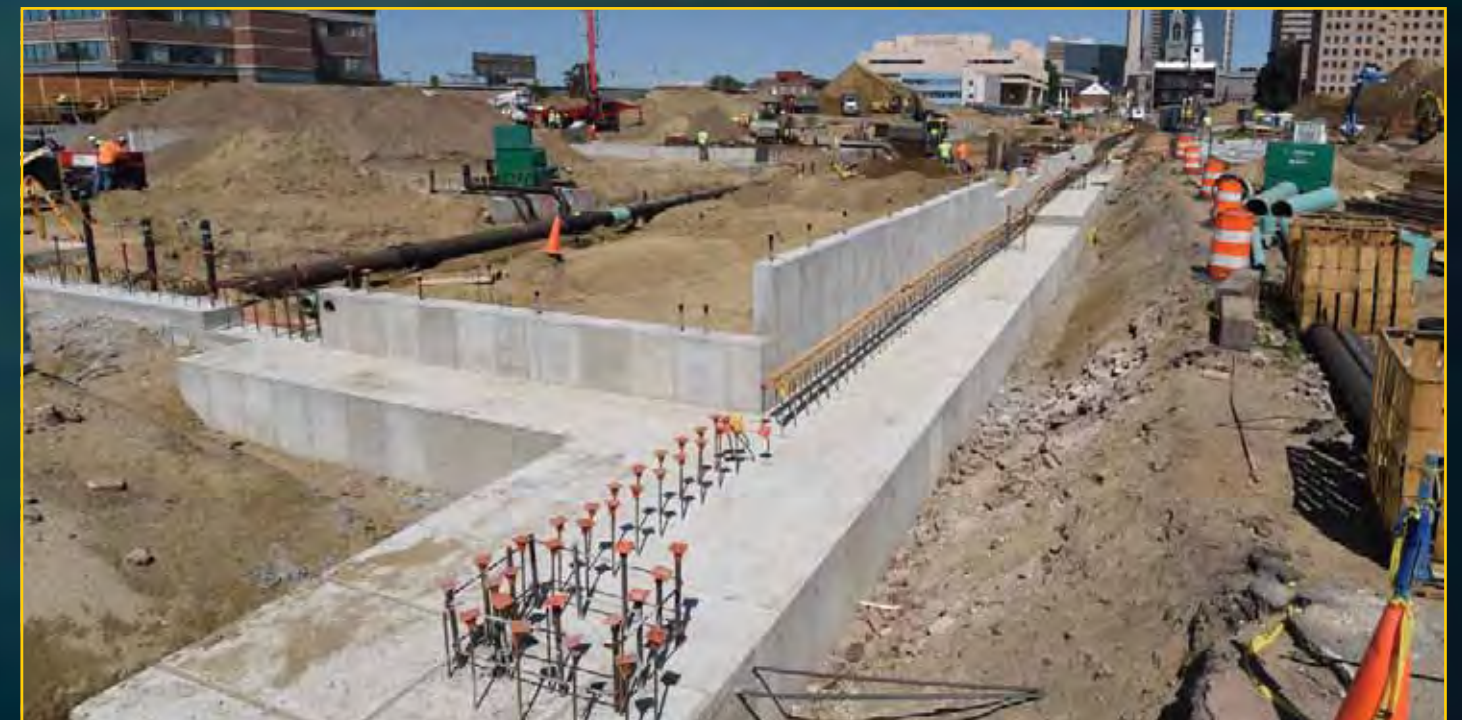
Garage Construction - June 25, 2016
