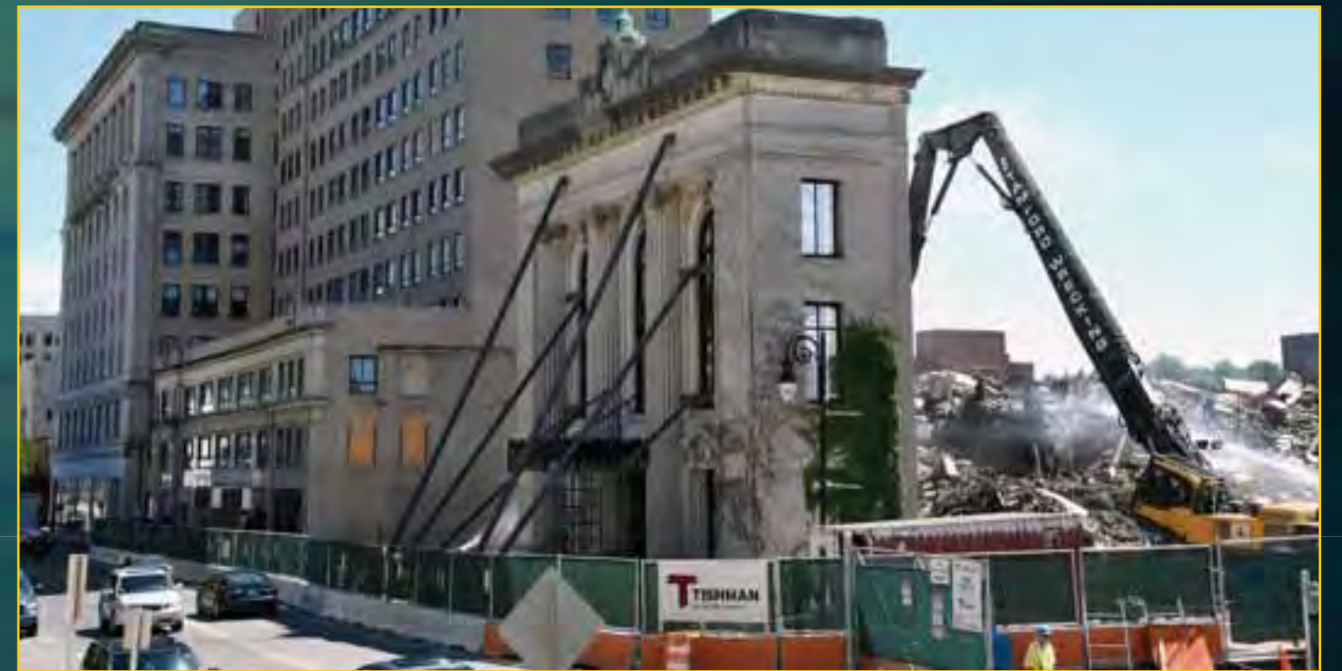
73 State Demolition - June 21, 2016
