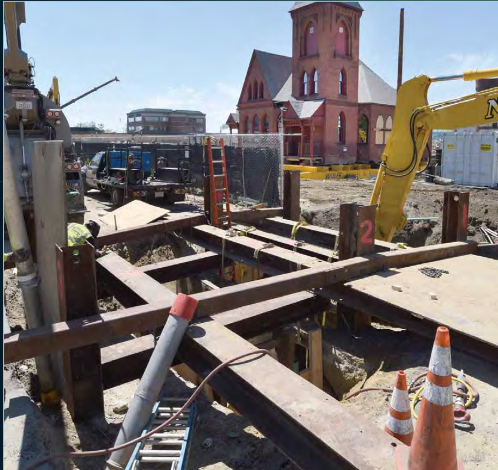
Union St. Pipes - May 18, 2016
