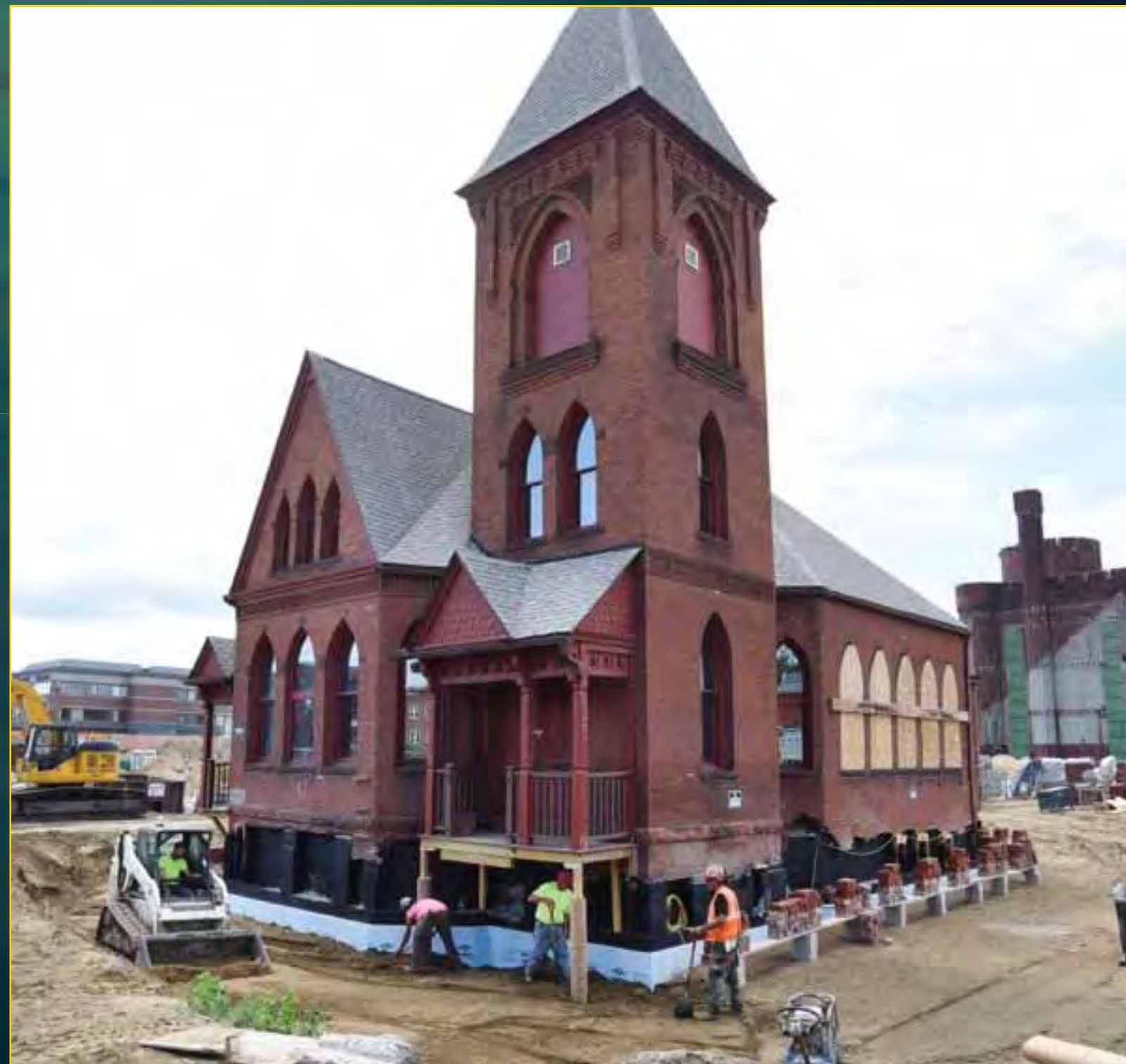
New Church Foundation - June 28, 2016
