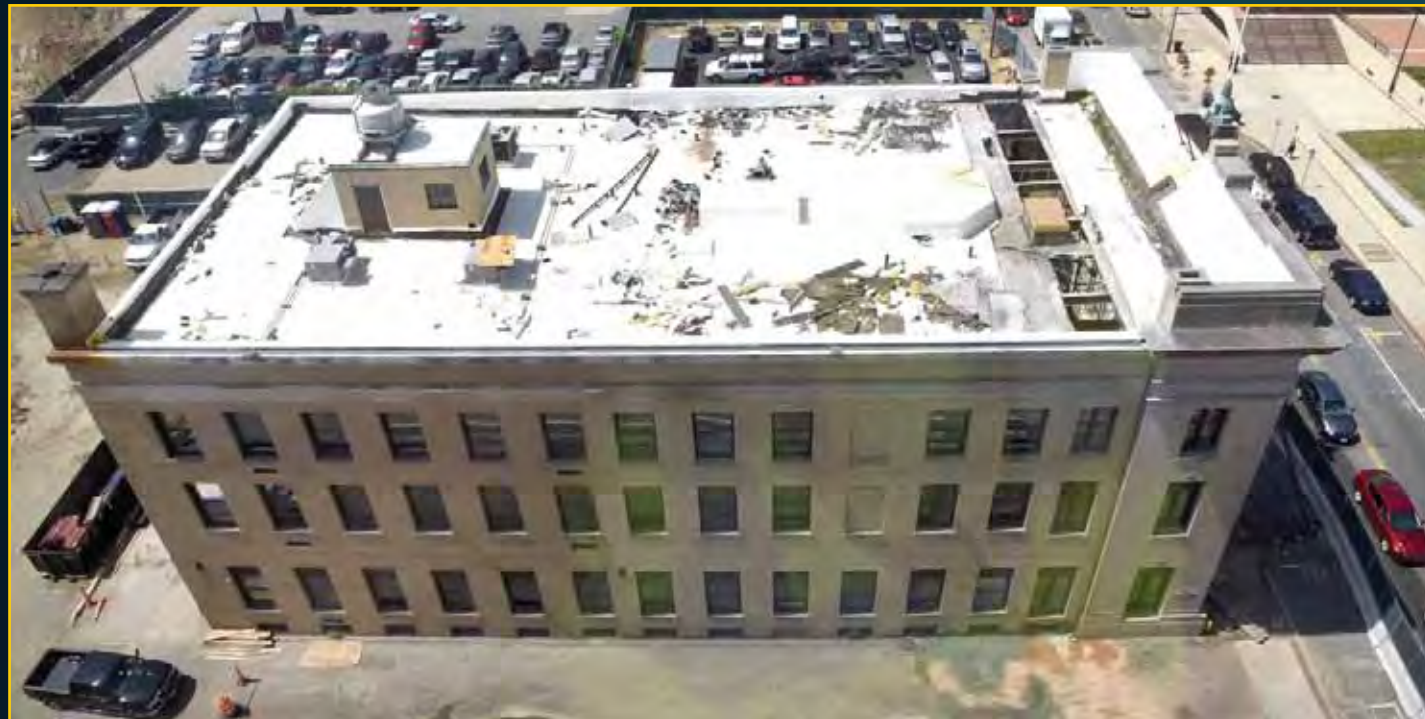
73 State Demolition - June 1, 2016
