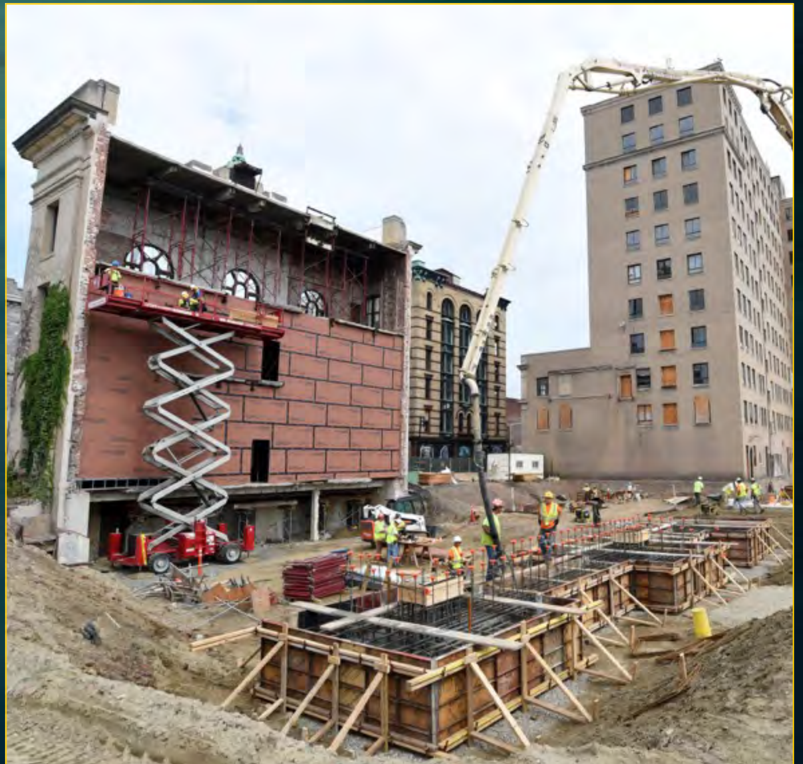
Podium Foundation & 73 State Demo - August 16, 2016
