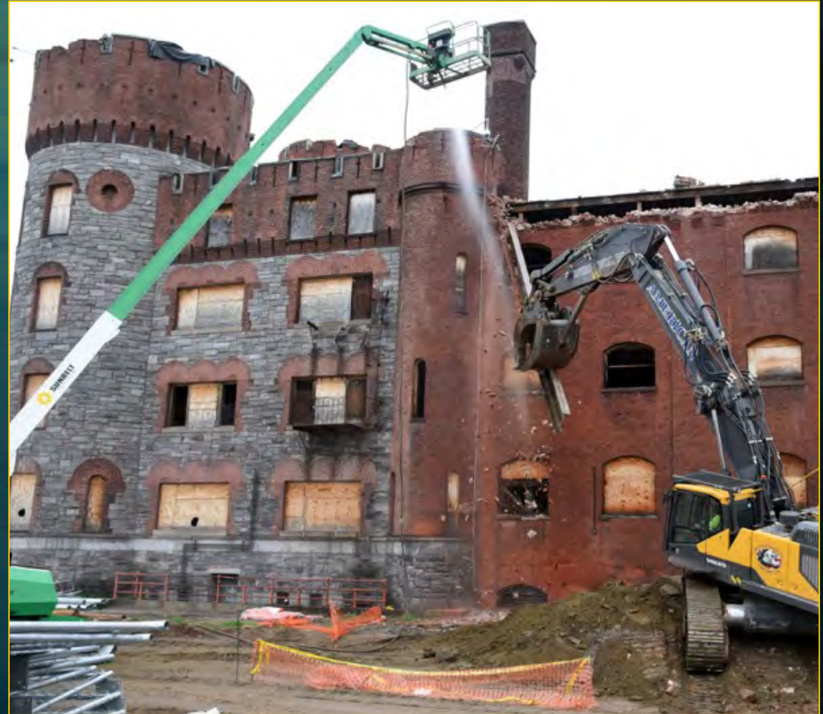
Armory Demolition - May 5, 2016
