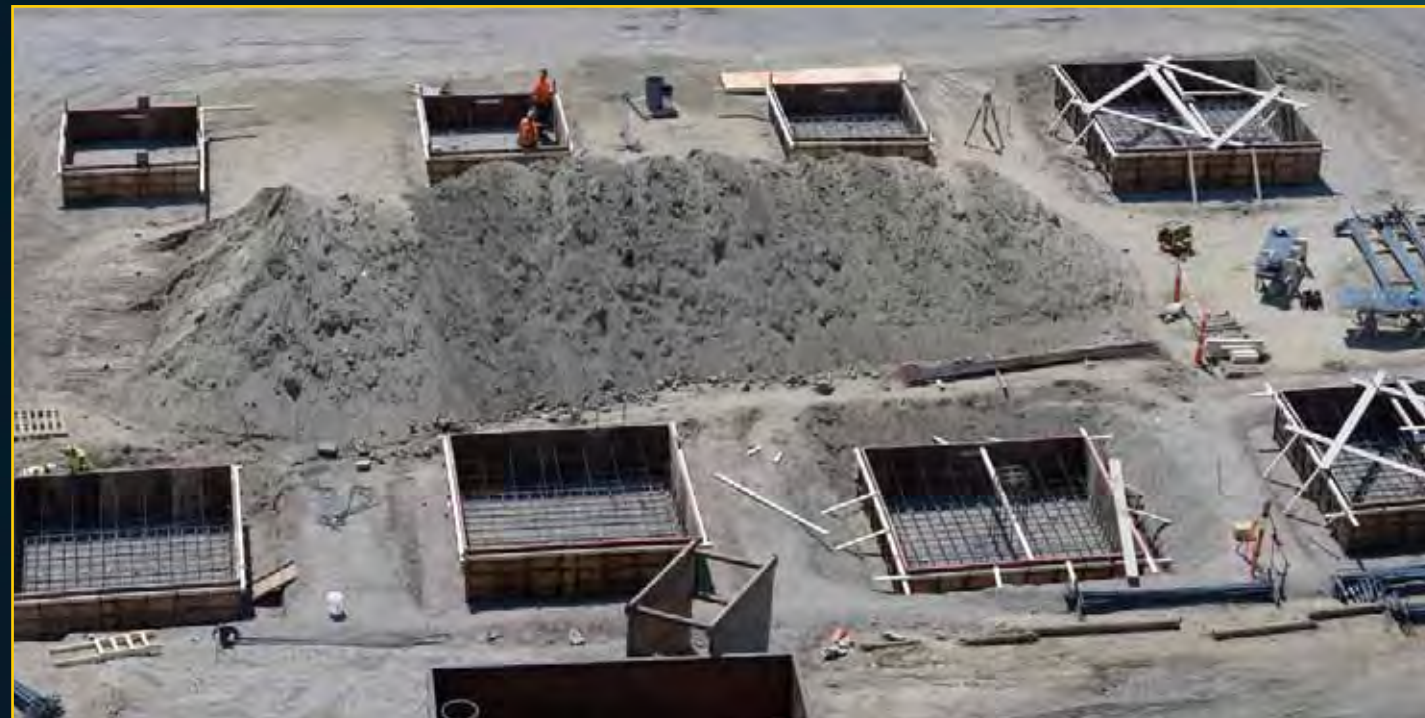
Podium Footings Prepared - June 21, 2016
