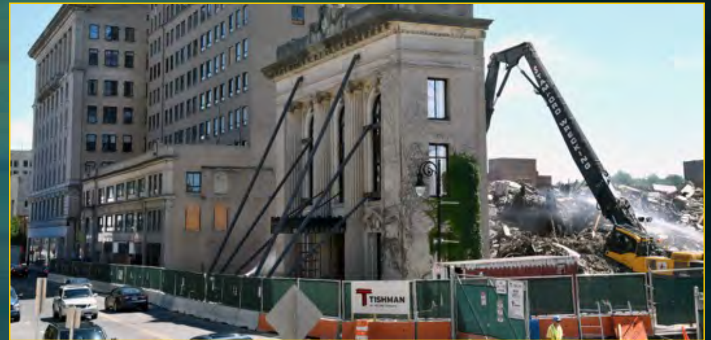
73 State Demolition - June 21, 2016
