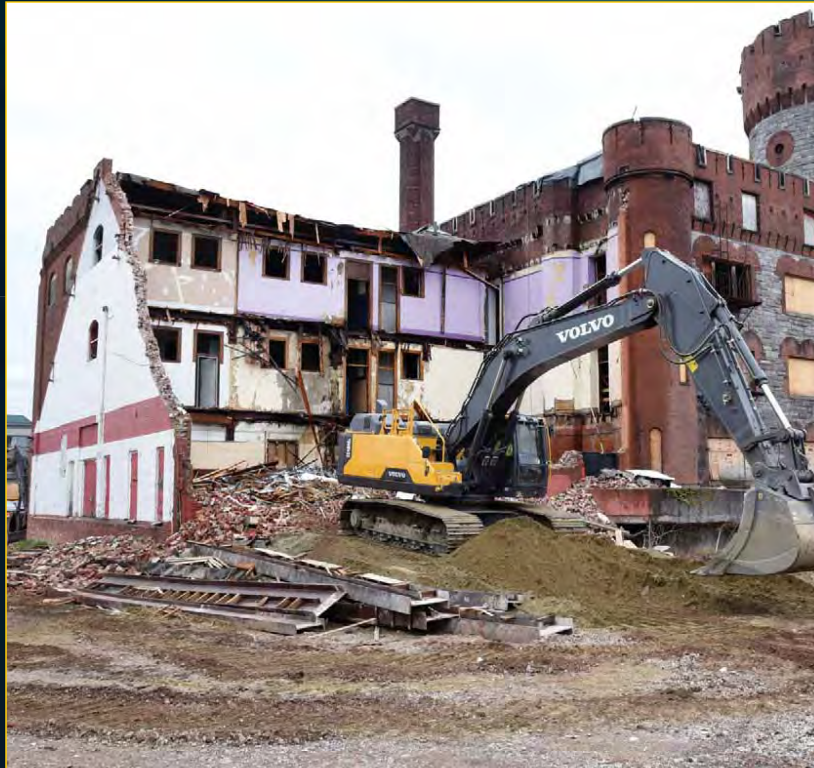
Armory Demolition - May 5, 2016
