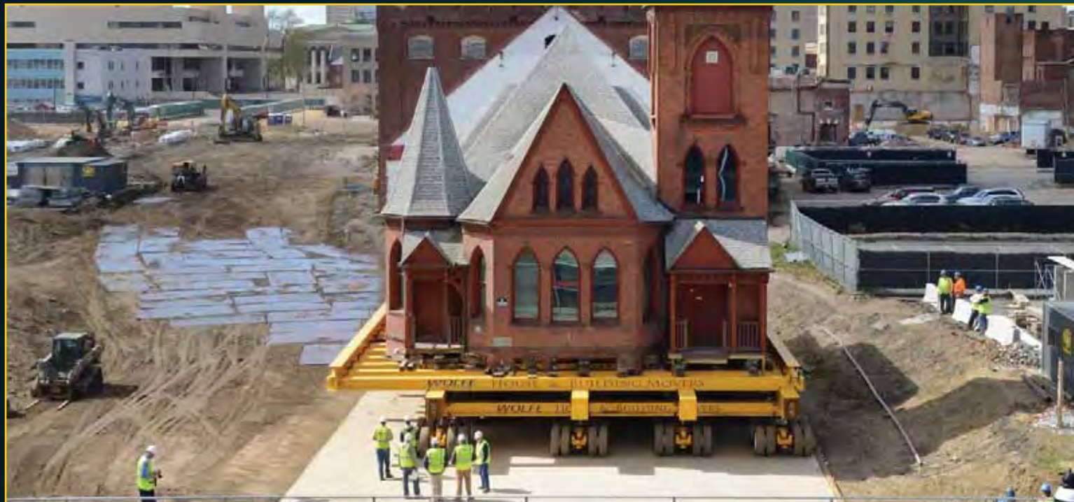
Church arrives at new location - April 19, 2016
