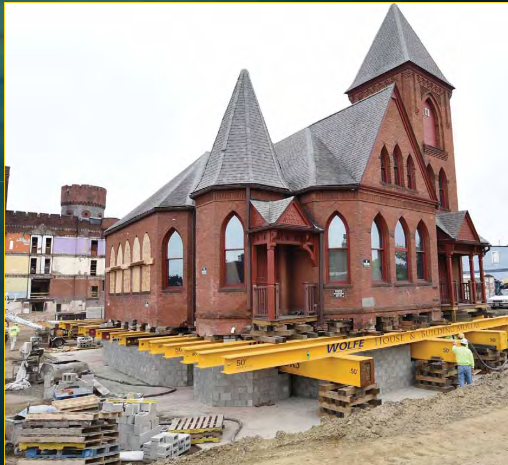
New Church Foundation - May 17, 2016
