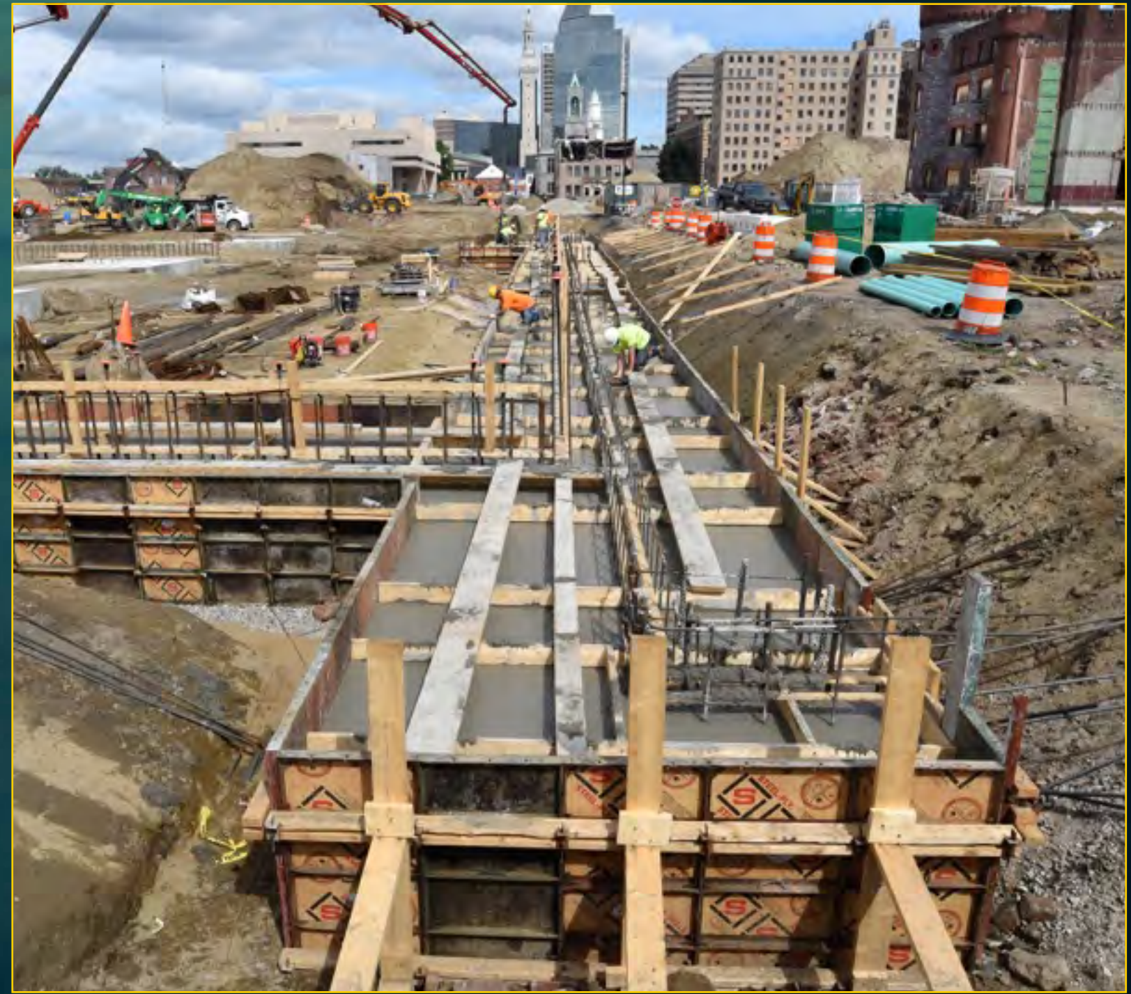
Garage Construction - June 8, 2016
