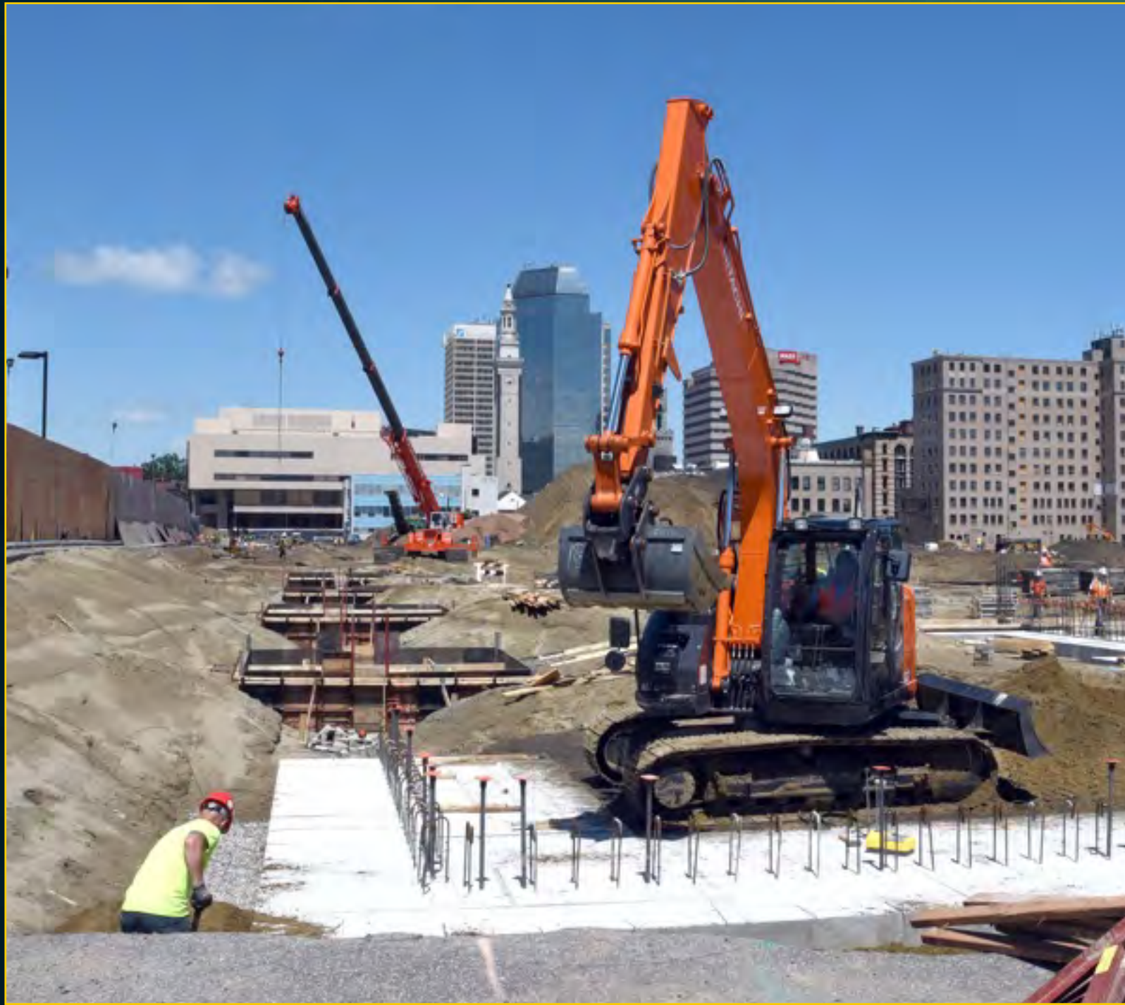
Garage Construction - June 6, 2016
