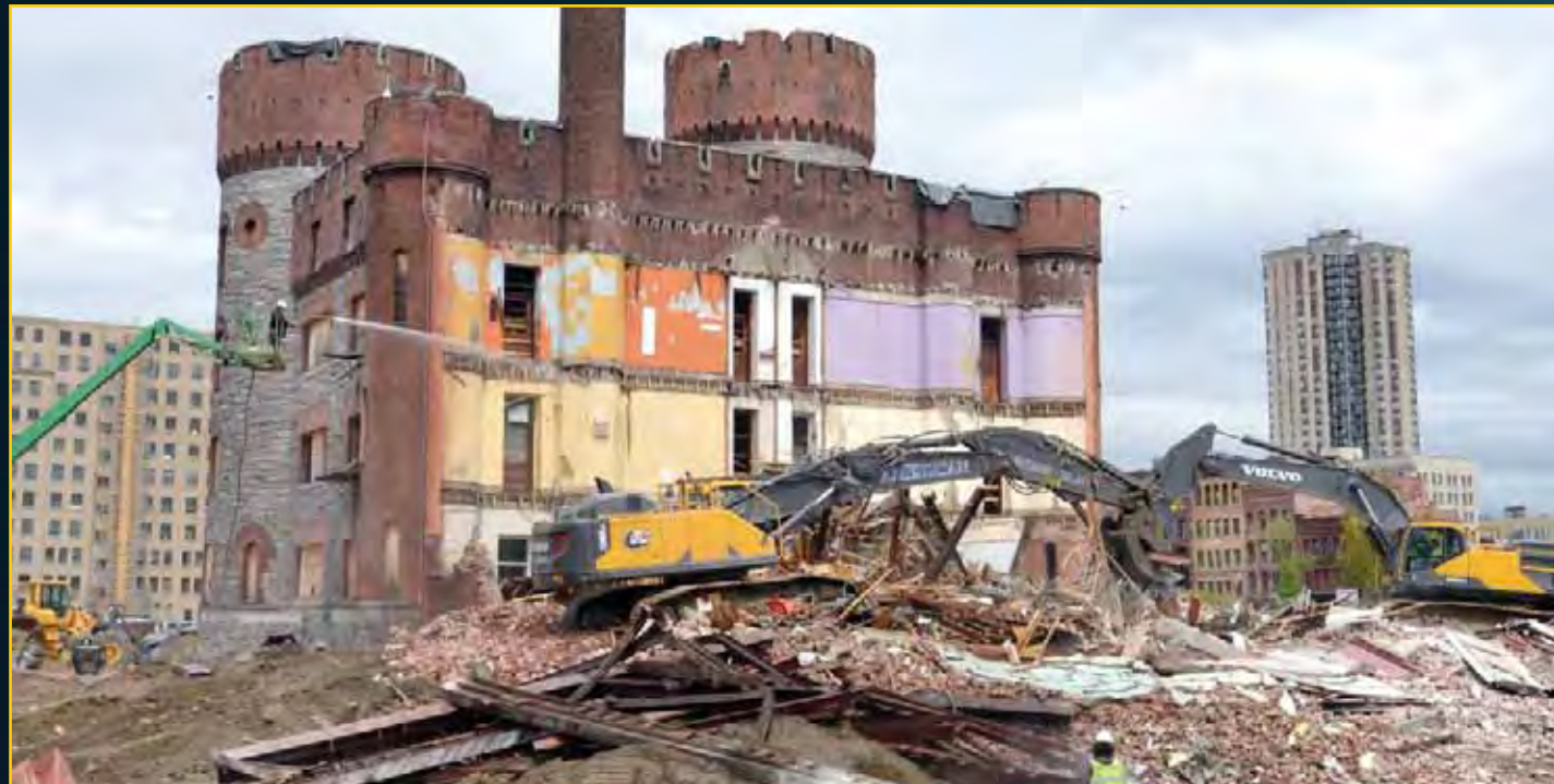
Armory Back Demolition - May 6, 2016
