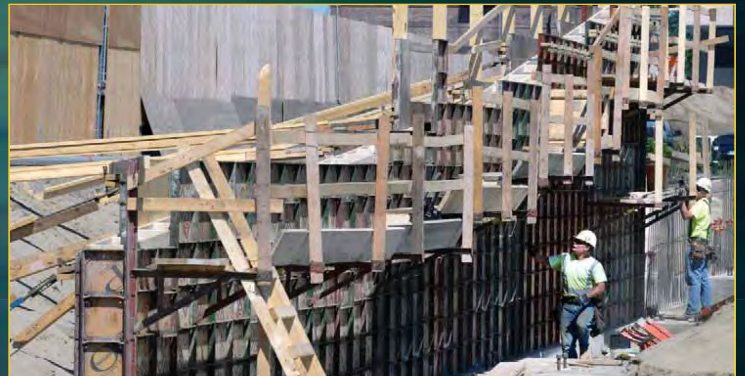
Garage Construction - June 24, 2016
