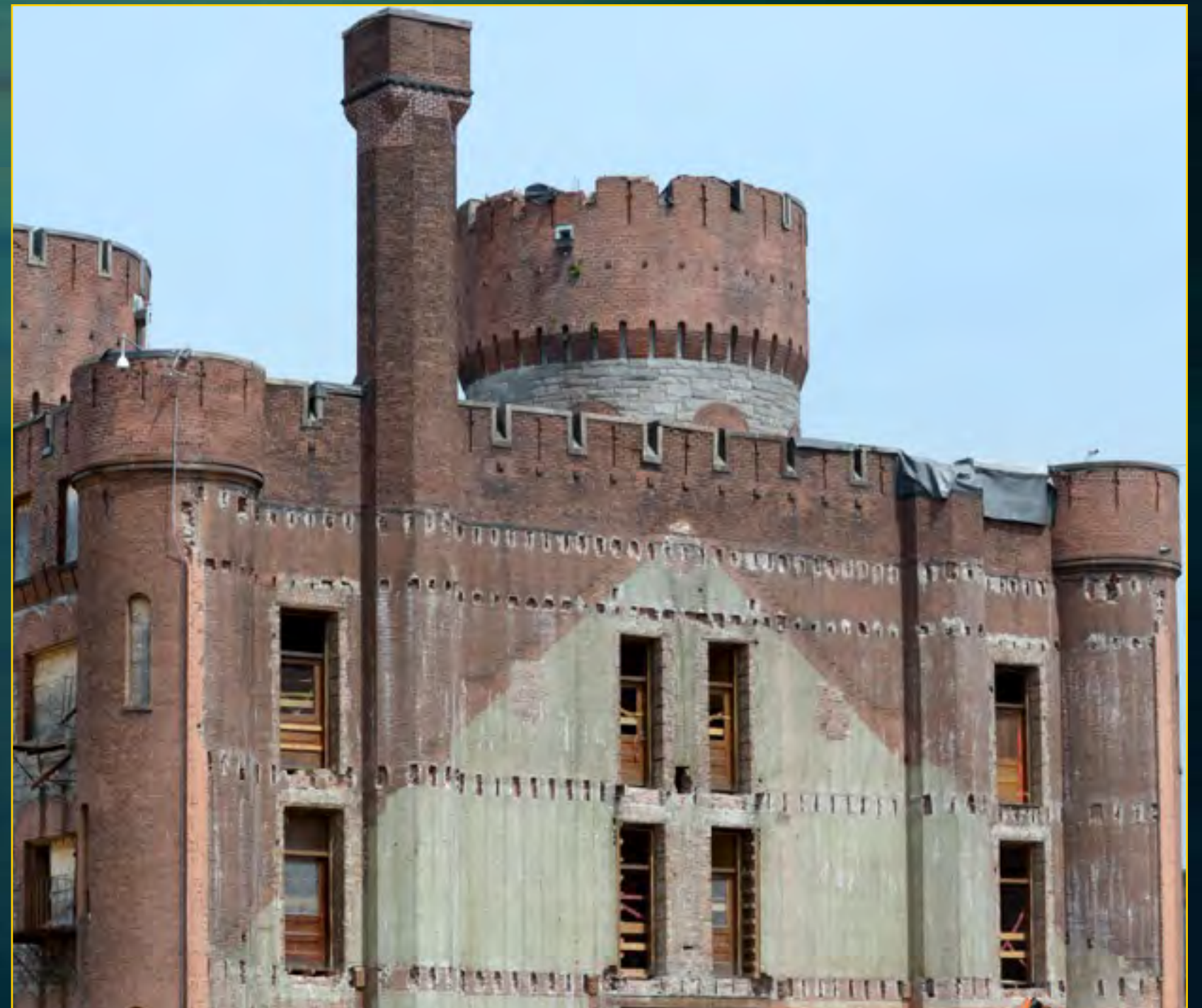
Armory Back Completion - May 26, 2016
