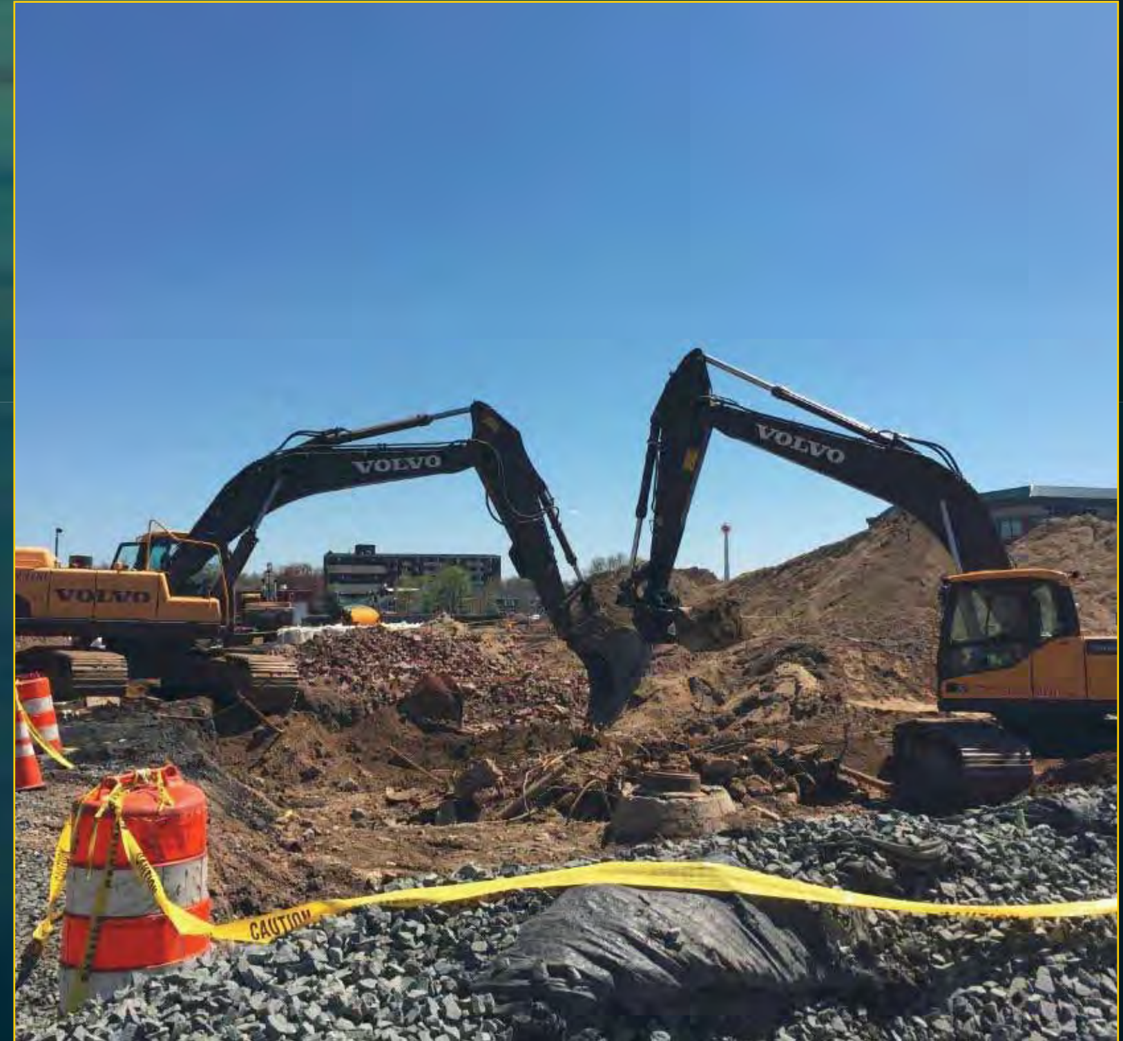
Mass Excavation - June 9, 2016
