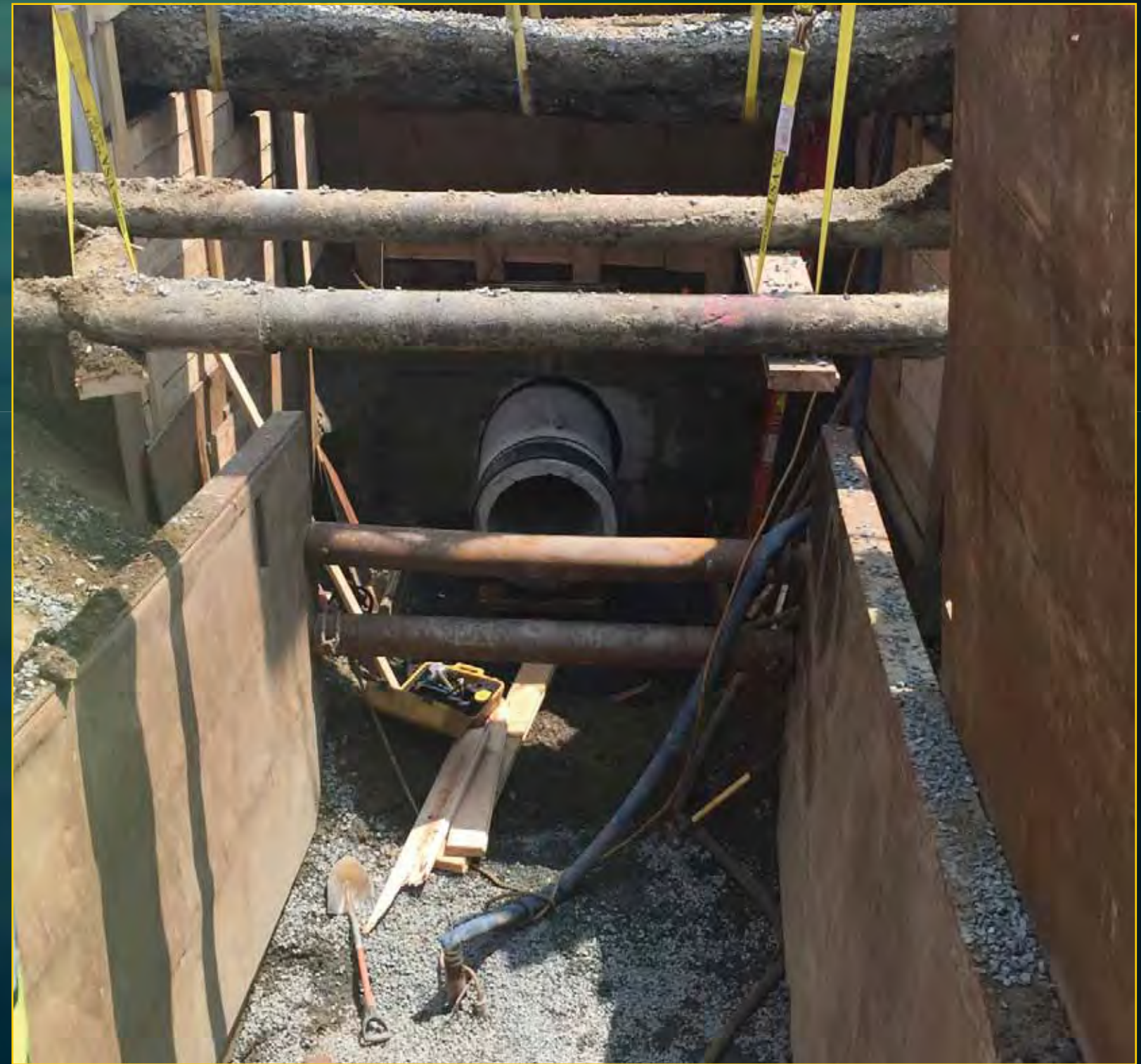
Offsite Utilities - May 20, 2016
