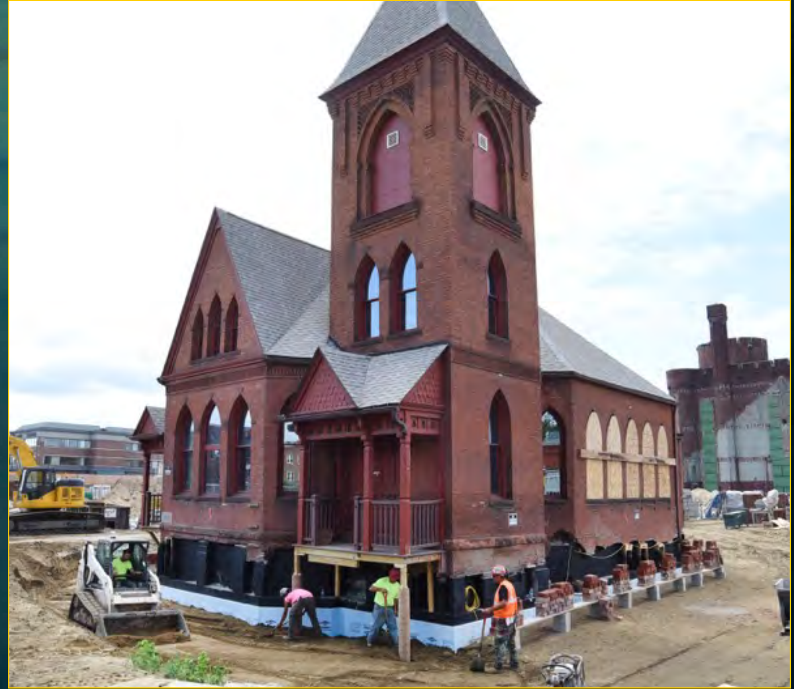
New Church Foundation - June 28, 2016
