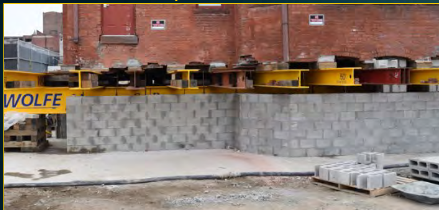
New Church Foundation - May 17, 2016
