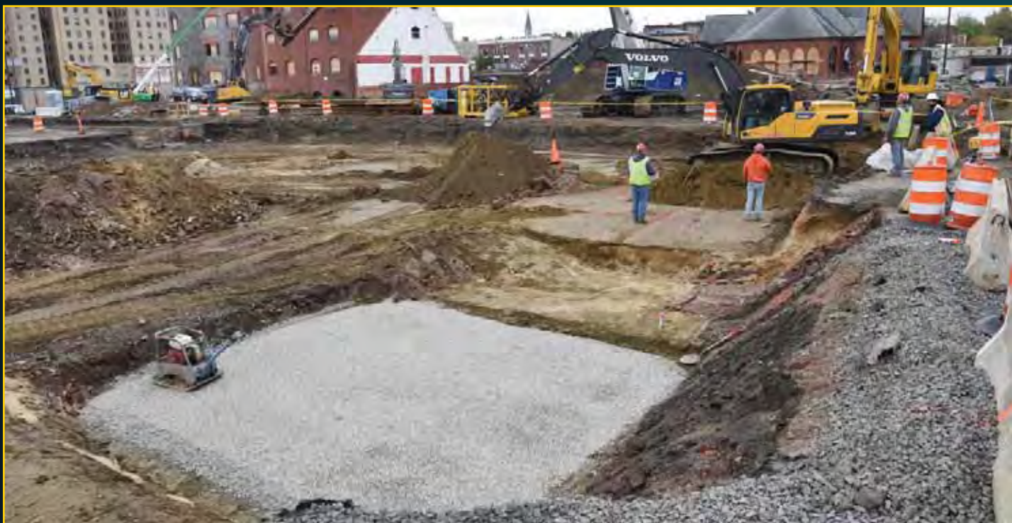
Garage Footings - May 5, 2016
