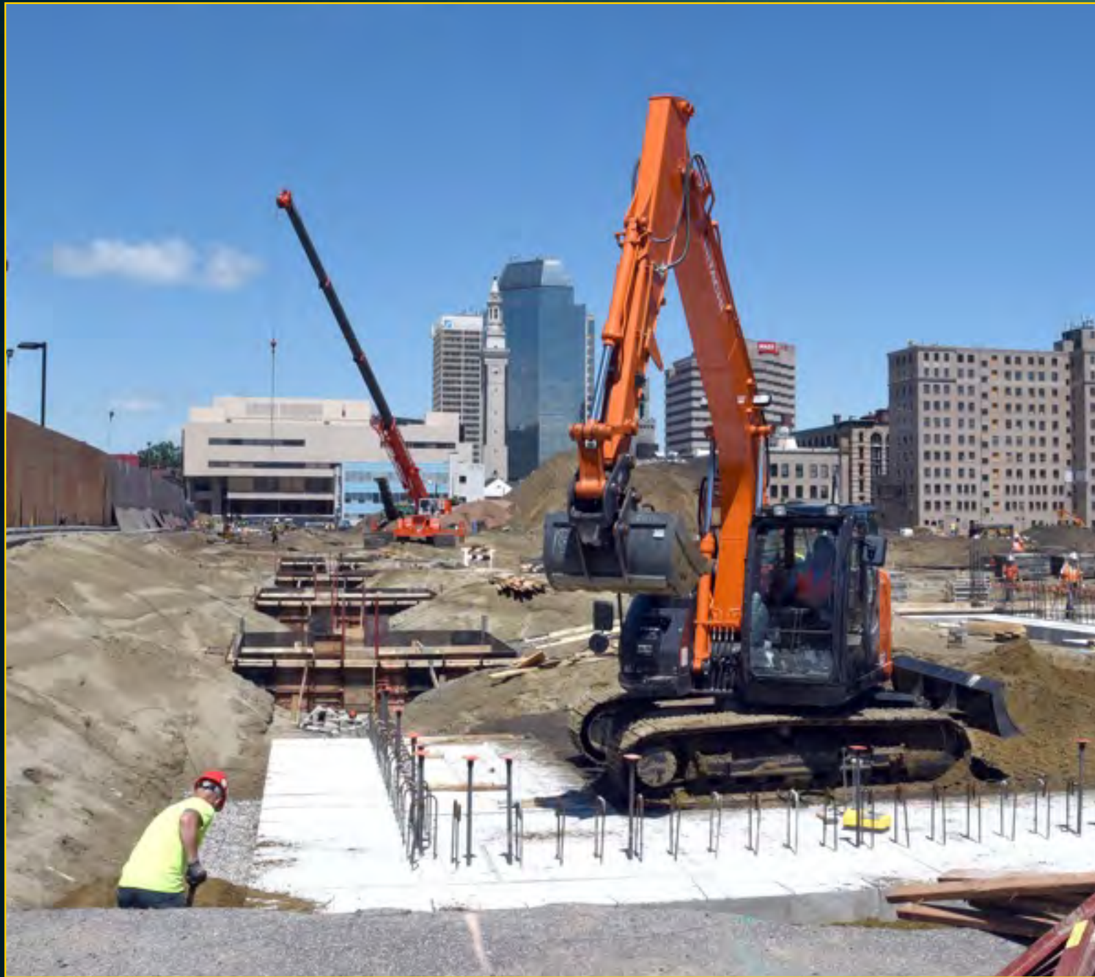
Garage Construction - June 6, 2016
