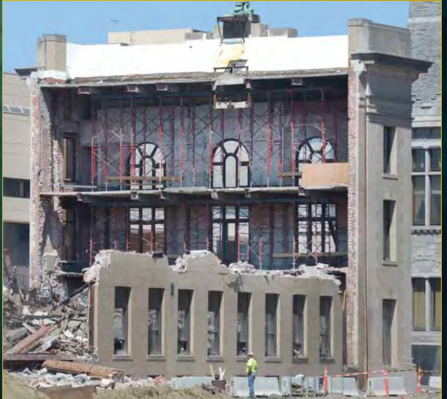
73 State Demolition - June 24, 2016
