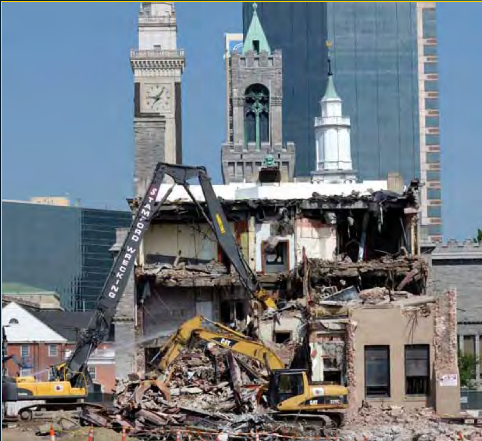
73 State Demolition - June 20, 2016
