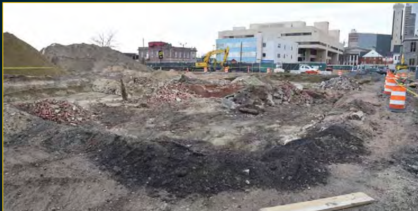
Garage Site Preparation - April 11, 2016
