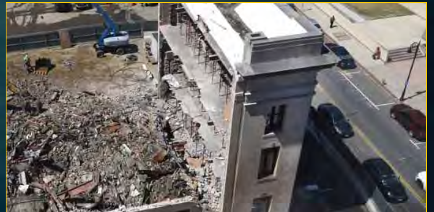
73 State Demolition - June 24, 2016
