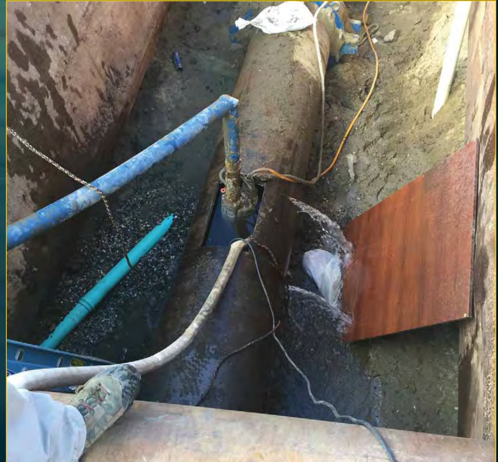
Offsite Utility Work - June 13, 2016
