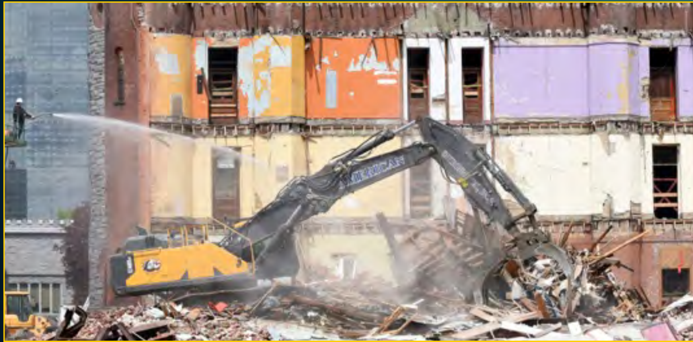
Armory Back Demolition - May 6, 2016
