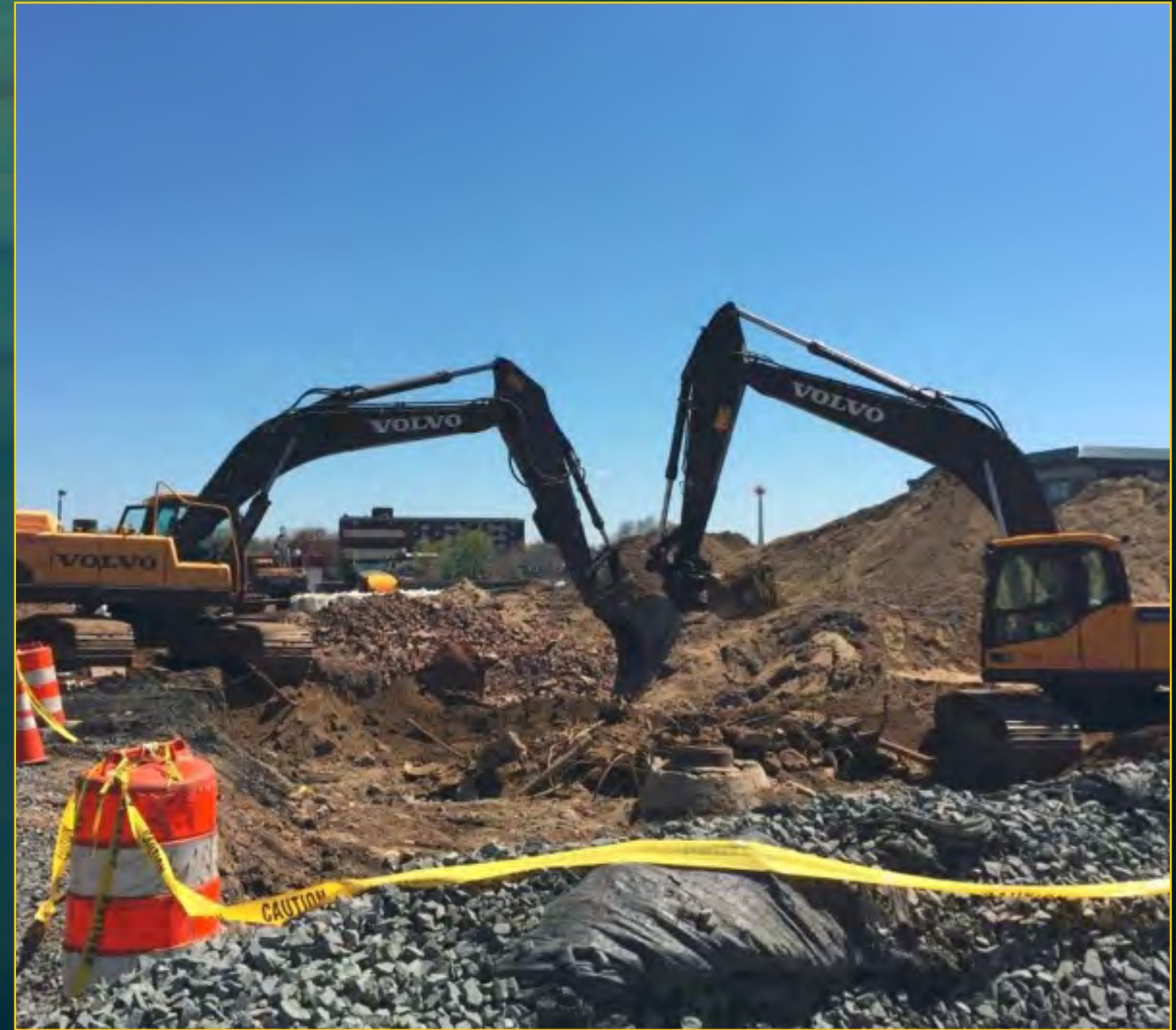
Mass Excavation - June 9, 2016
