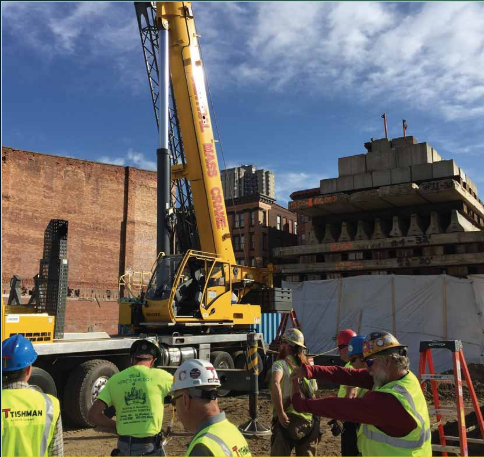
Union Chandler Test Pile- June 9, 2016
