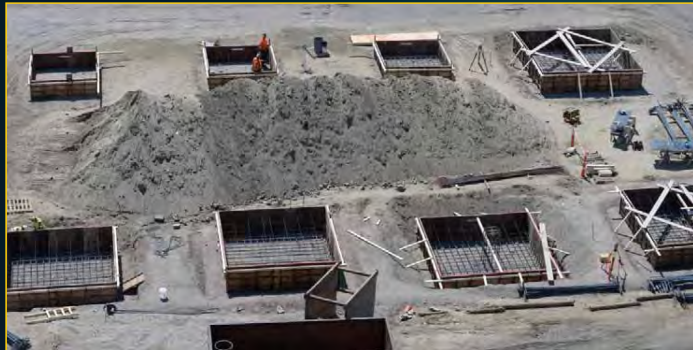
Podium Footings Prepared - June 21, 2016
