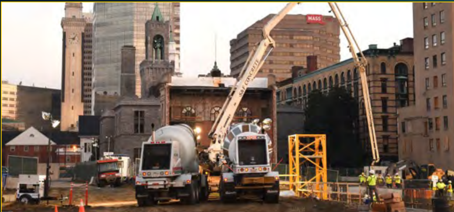
Hotel Foundation - August 13, 2016
