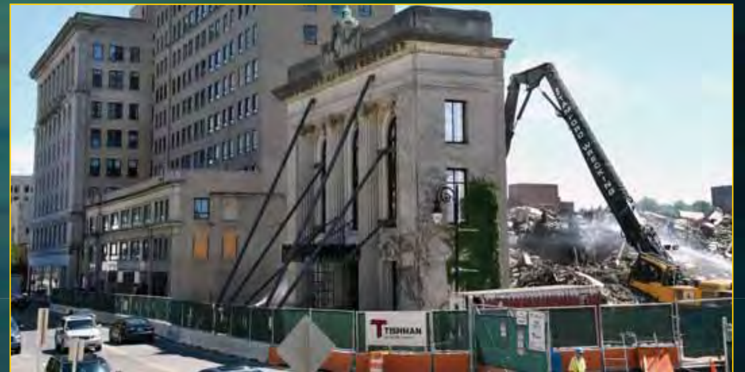
73 State Demolition - June 21, 2016
