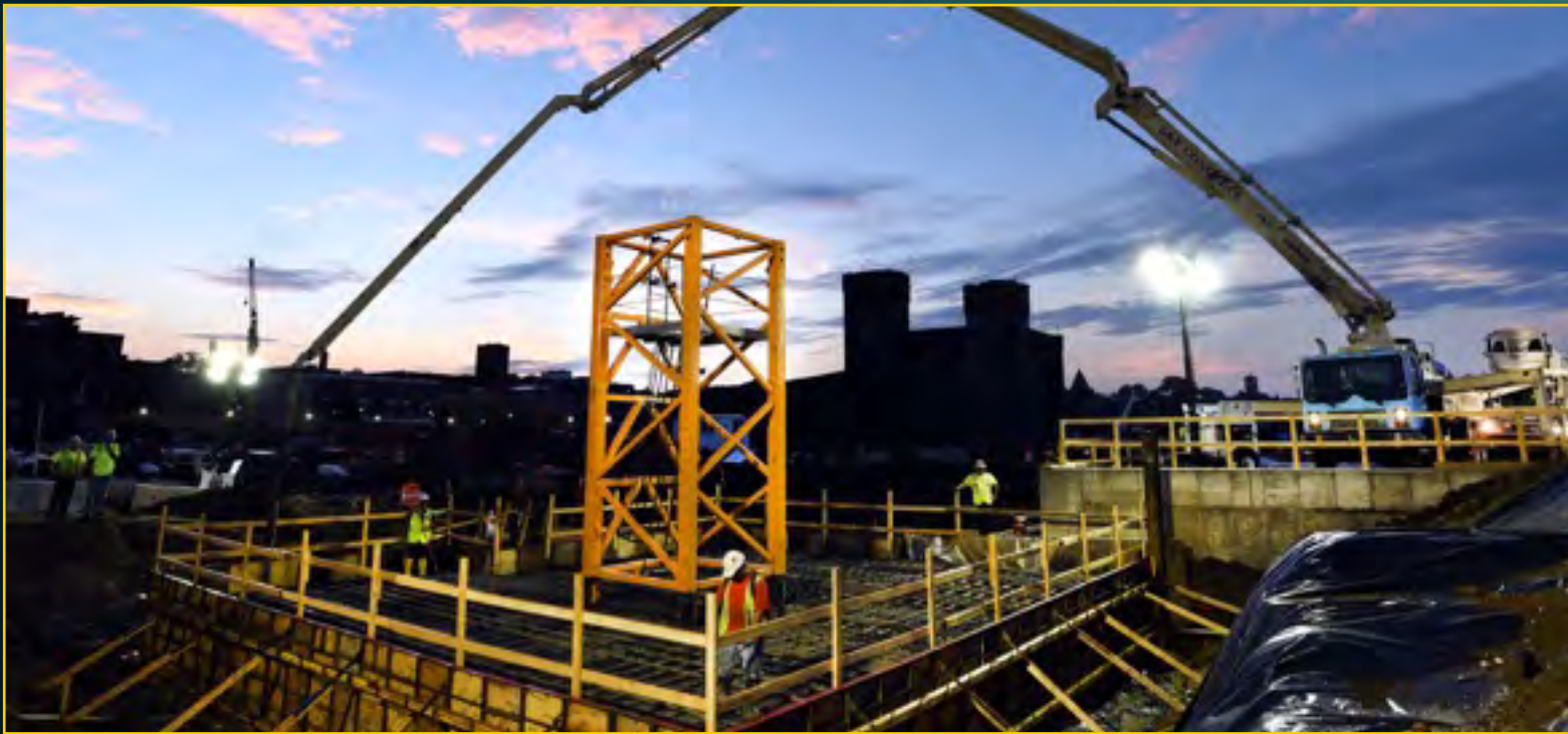
Hotel Foundation - August 13, 2016
