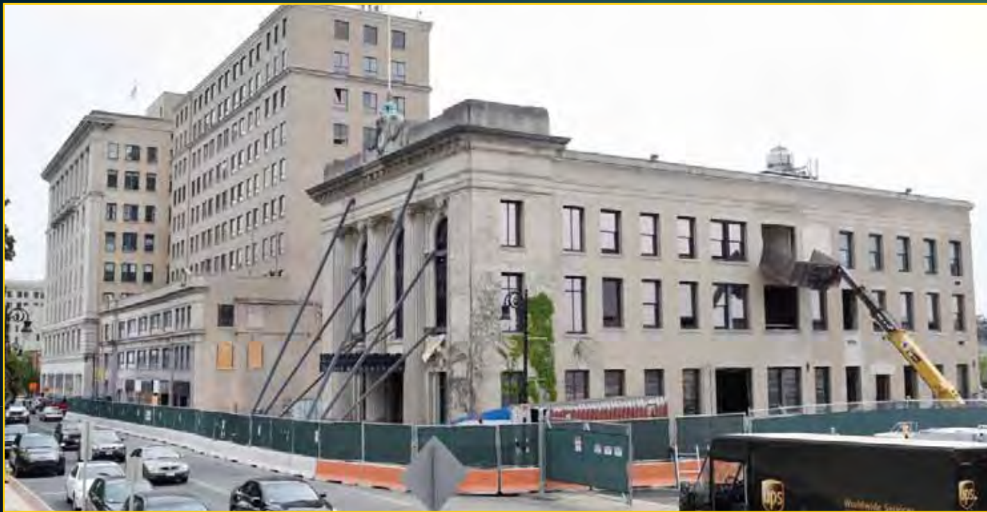
73 State Demolition - May 7, 2016
