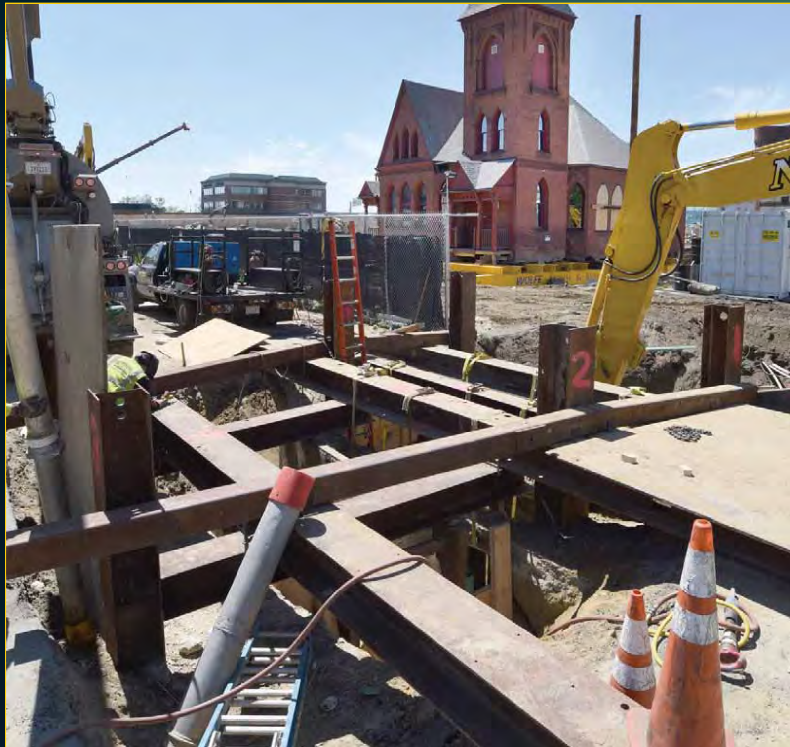
Union St. Pipes - May 18, 2016
