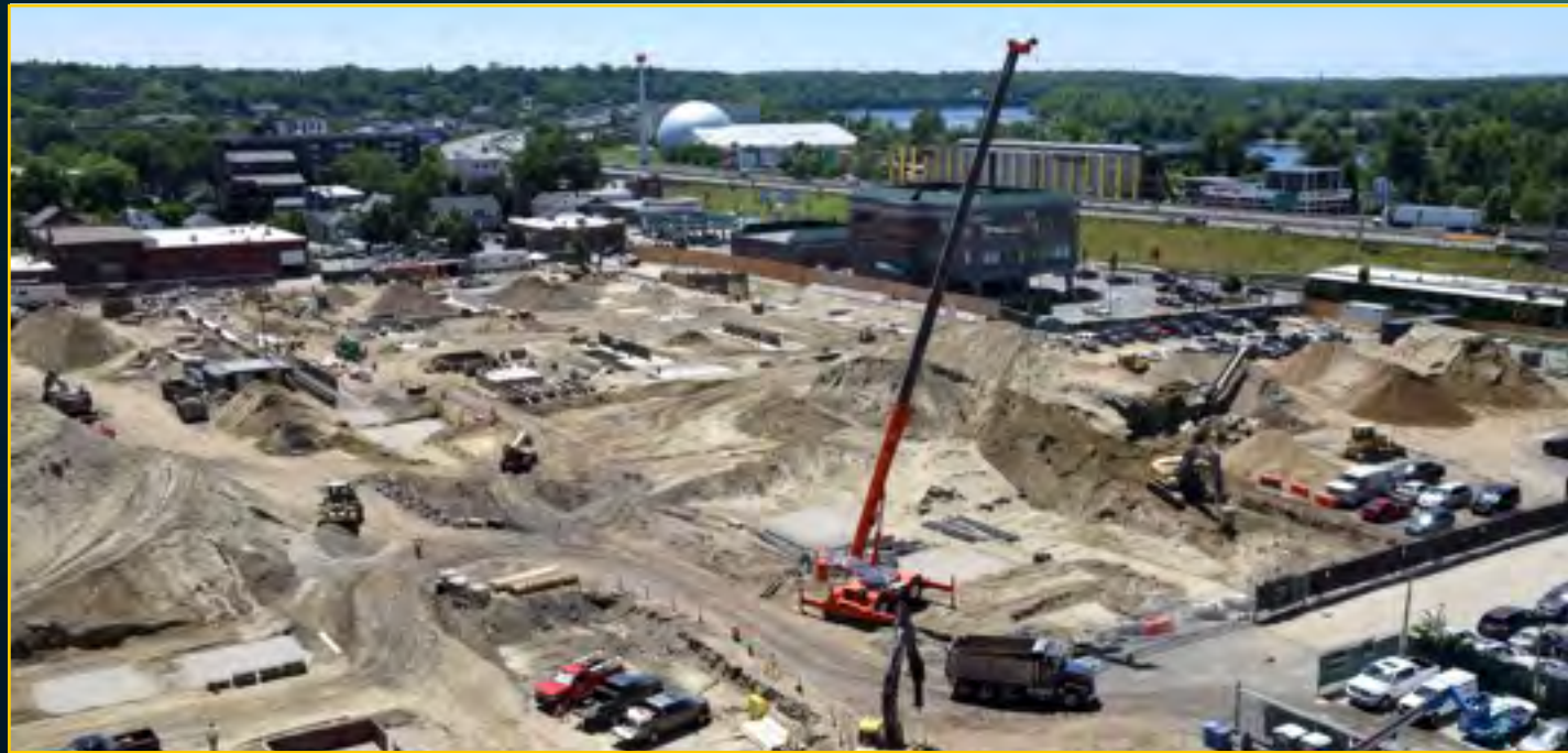
Podium Footings Prepared - June 21, 2016
