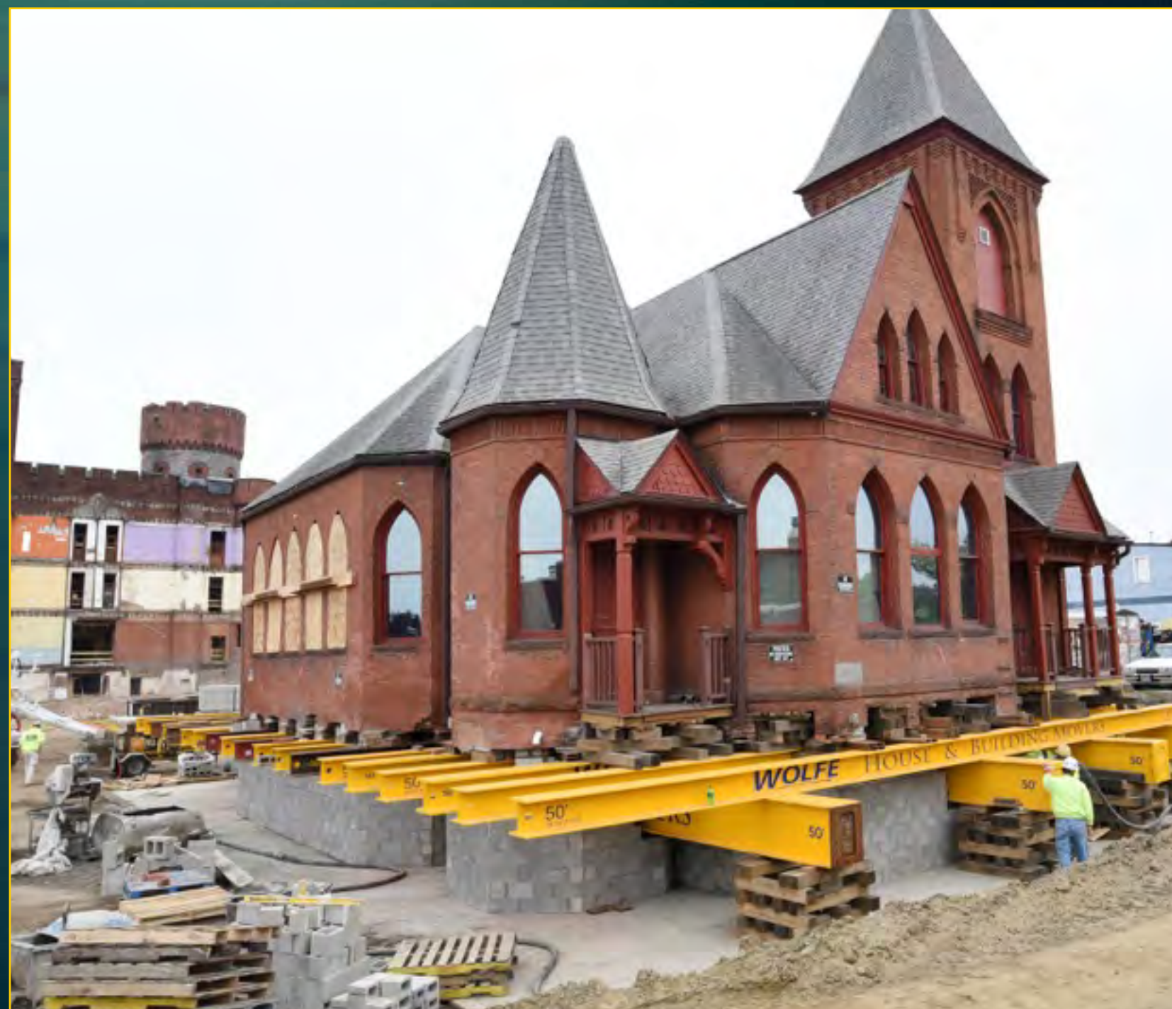
New Church Foundation - May 17, 2016
