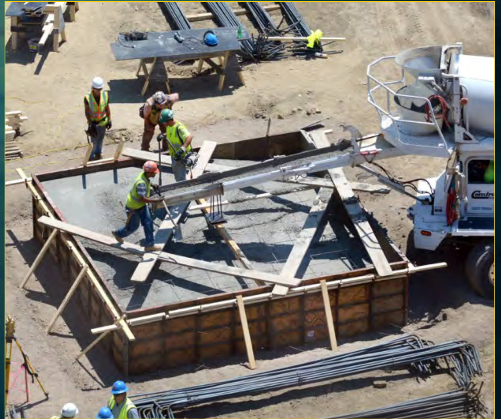
Podium Footings Prepared - June 25, 2016
