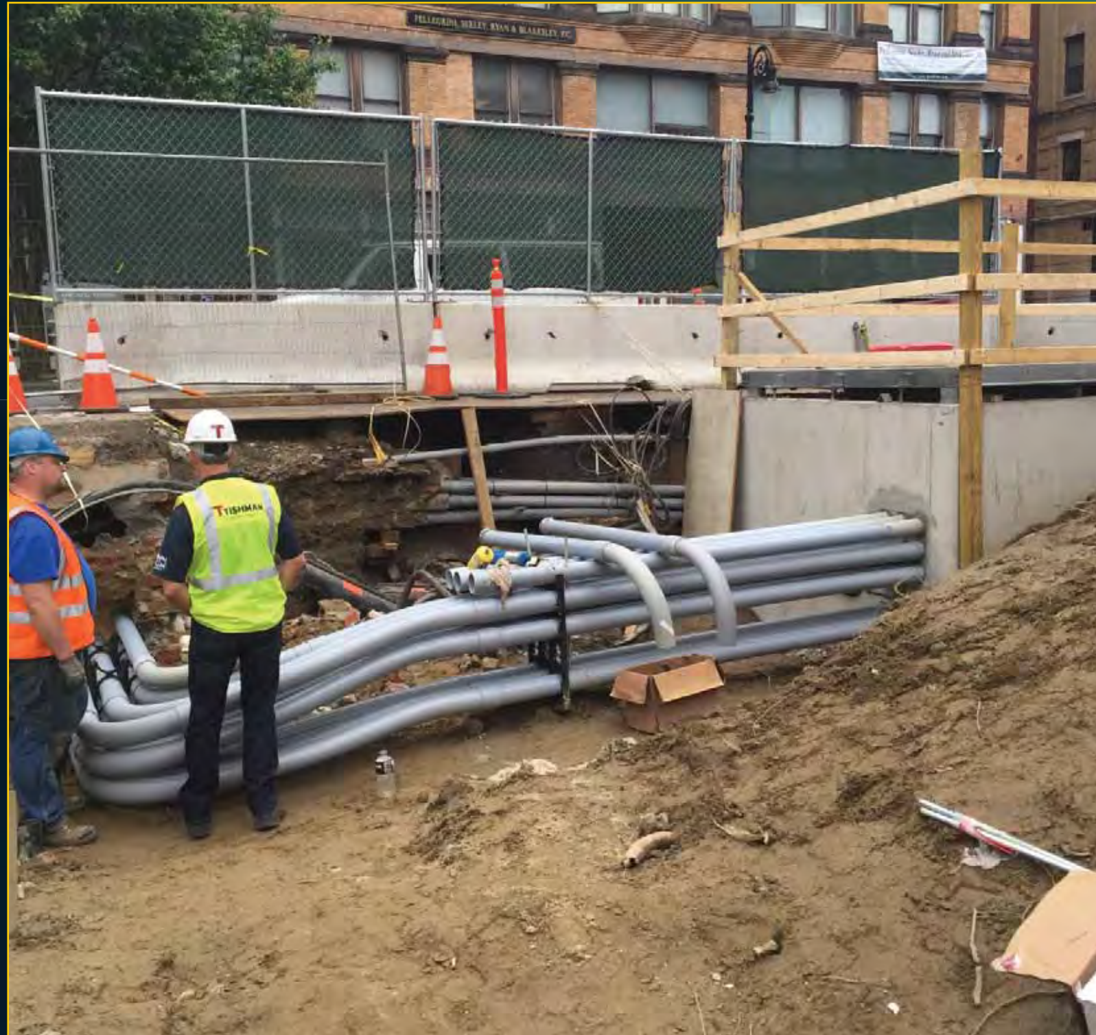
Vault Progress - May 24, 2016
