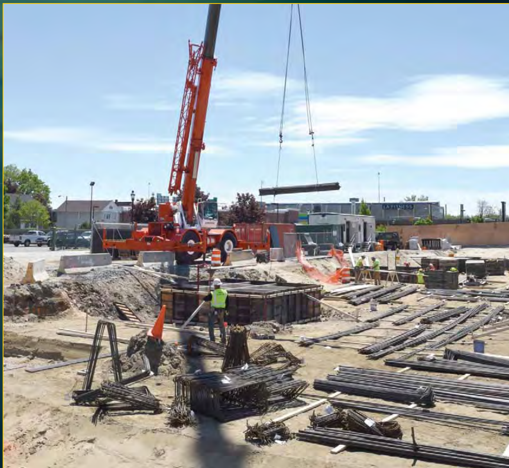
Garage Construction - May 18, 2016
