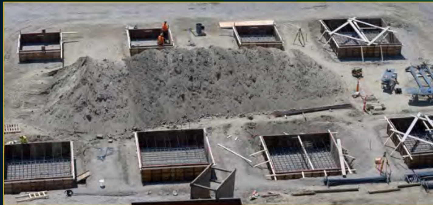
Podium Footings Prepared - June 21, 2016
