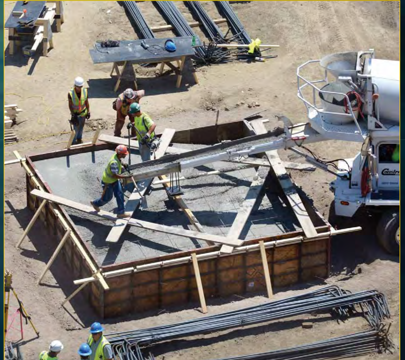
Podium Footings Prepared - June 25, 2016
