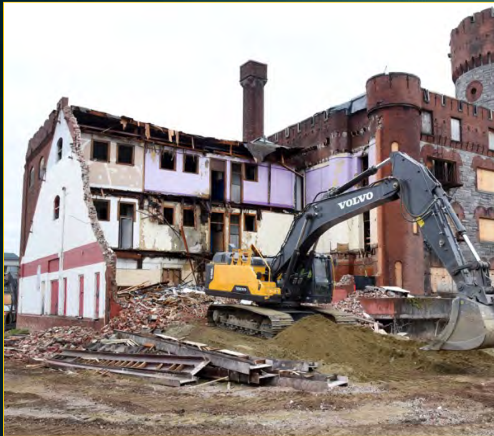
Armory Demolition - May 5, 2016
