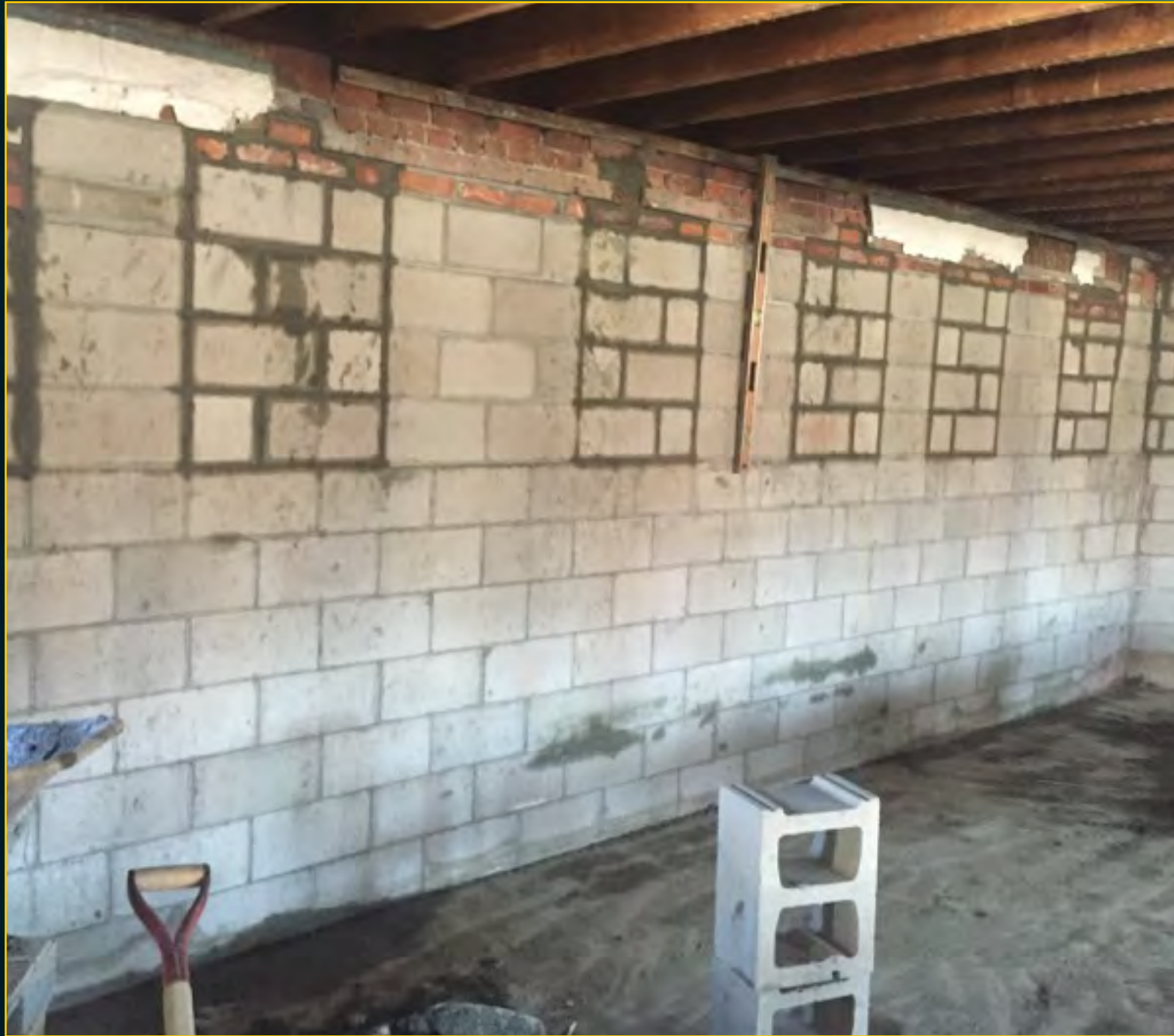
New Church Foundation - June 20, 2016
