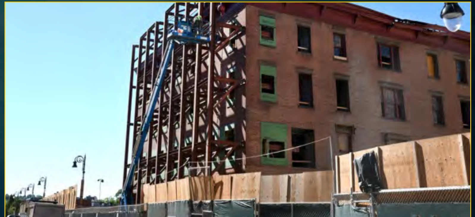
Union Chandler Facade Stabilization - August 22, 2016
