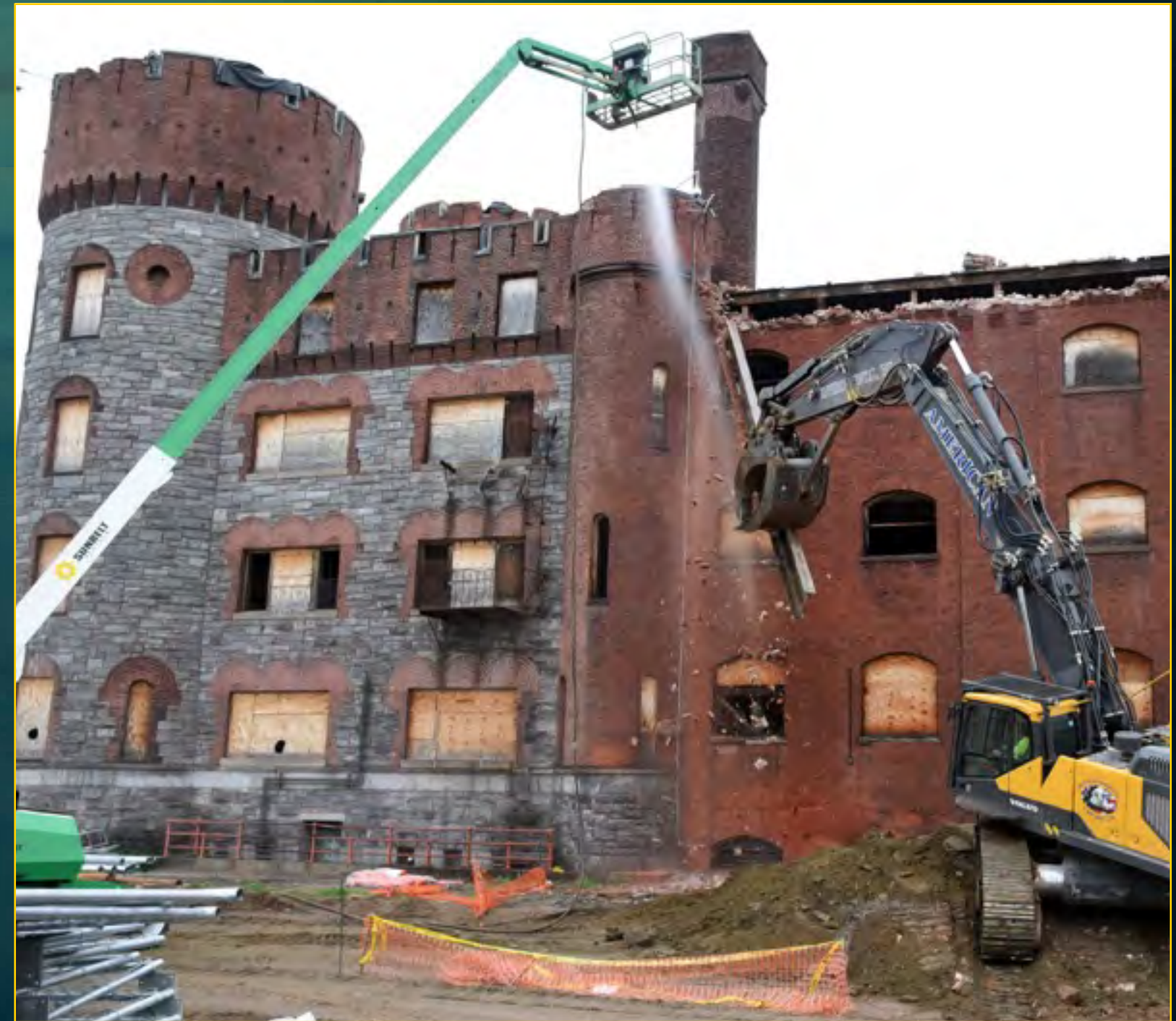
Armory Demolition - May 5, 2016
