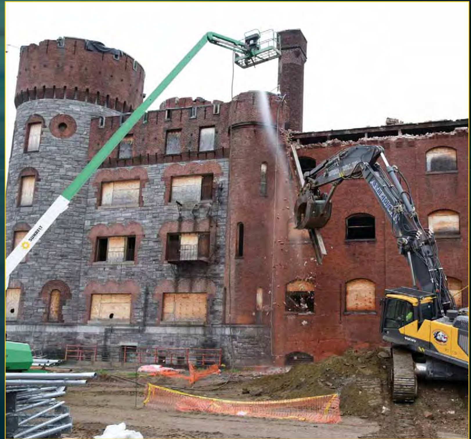
Armory Demolition - May 5, 2016
