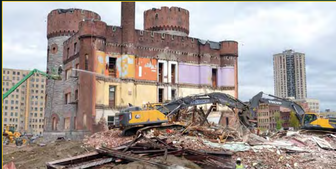
Armory Back Demolition - May 6, 2016
