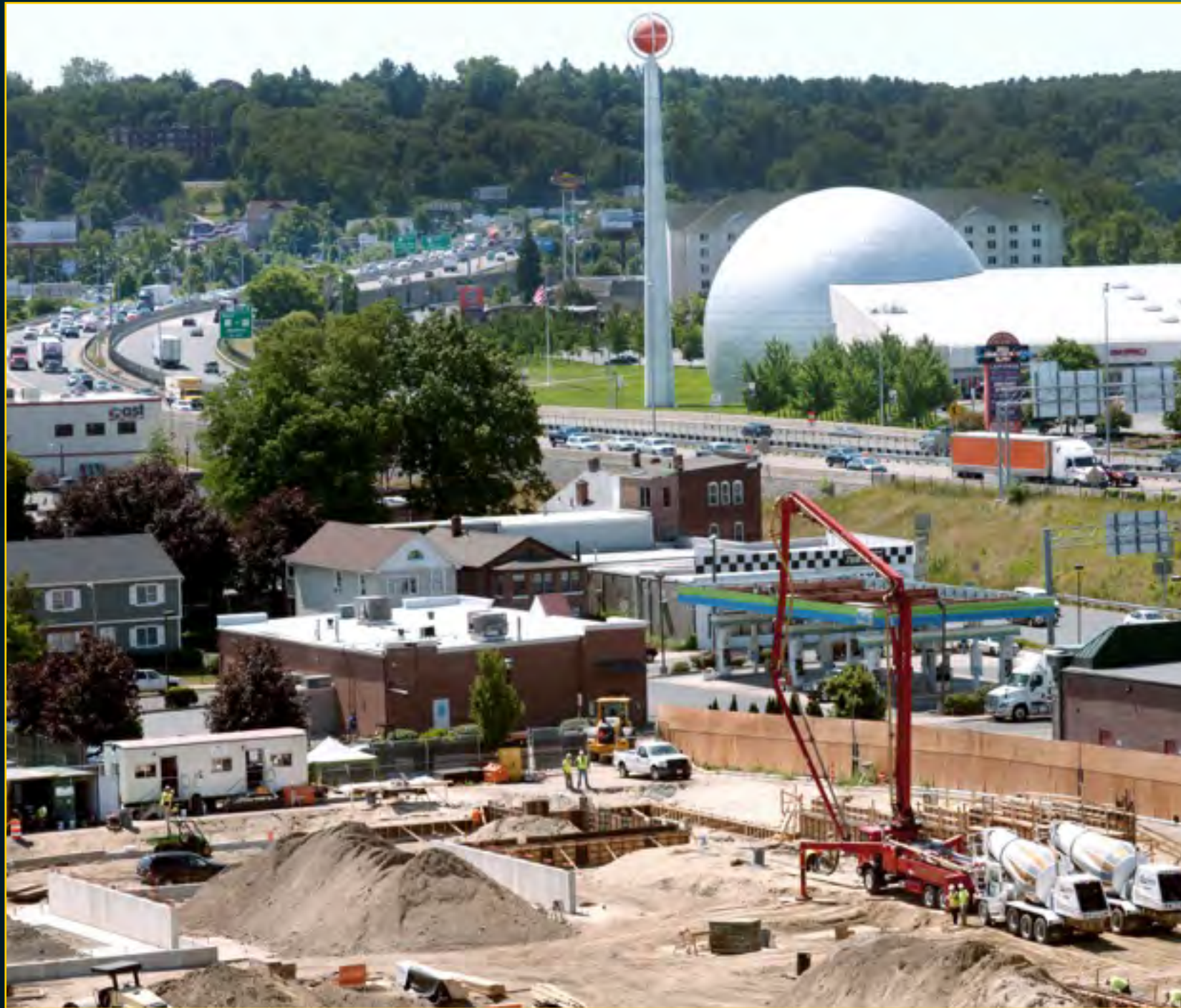
Garage Construction - June 24, 2016
