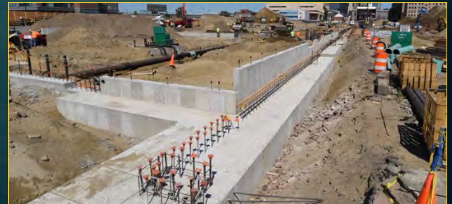
Garage Construction - June 25, 2016
