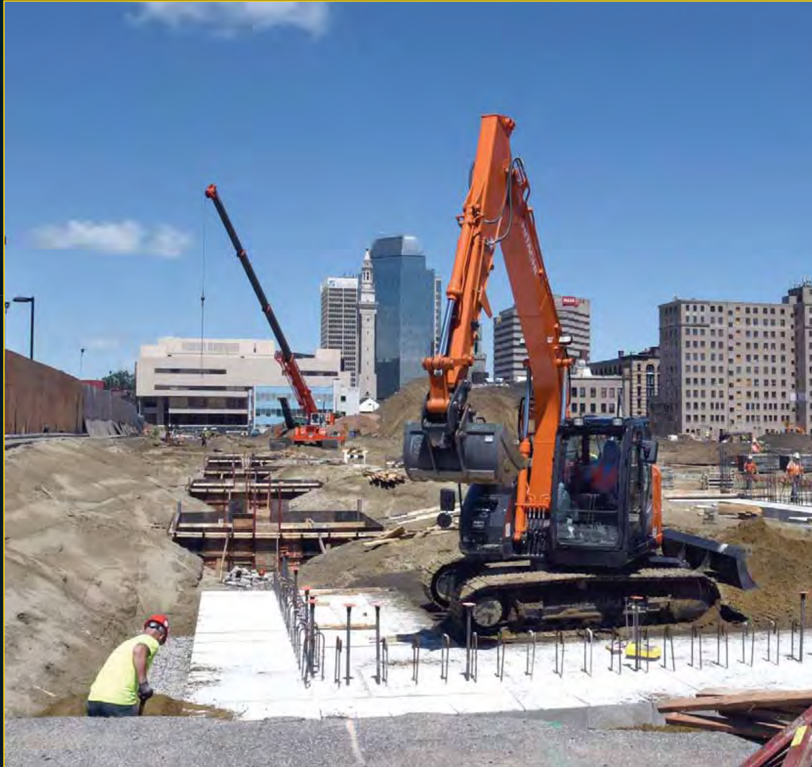
Garage Construction - June 6, 2016
