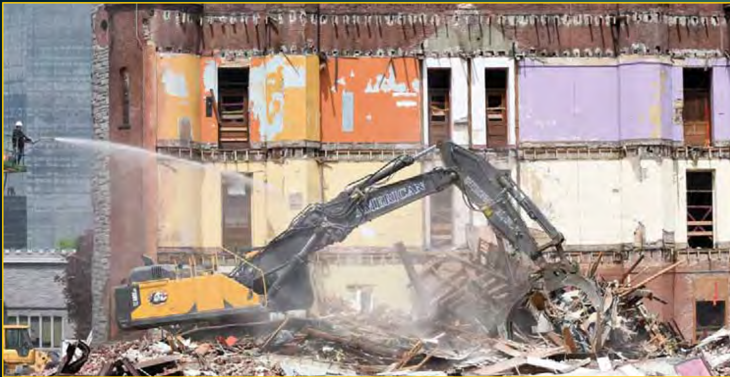
Armory Back Demolition - May 6, 2016
