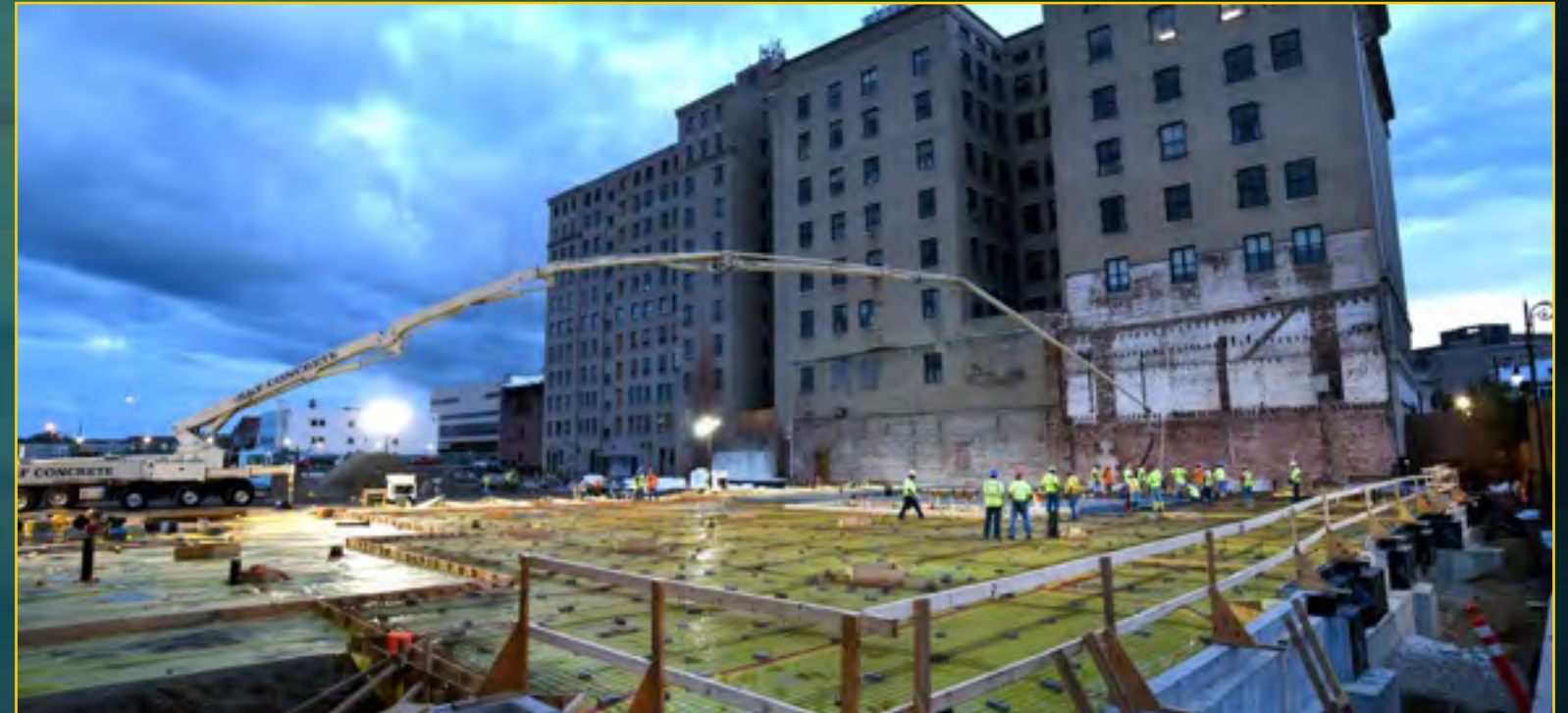
Hotel Foundation - August 17, 2016
