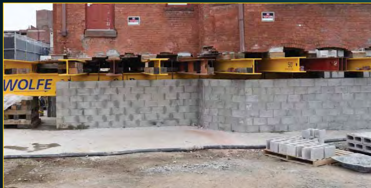
New Church Foundation - May 17, 2016
