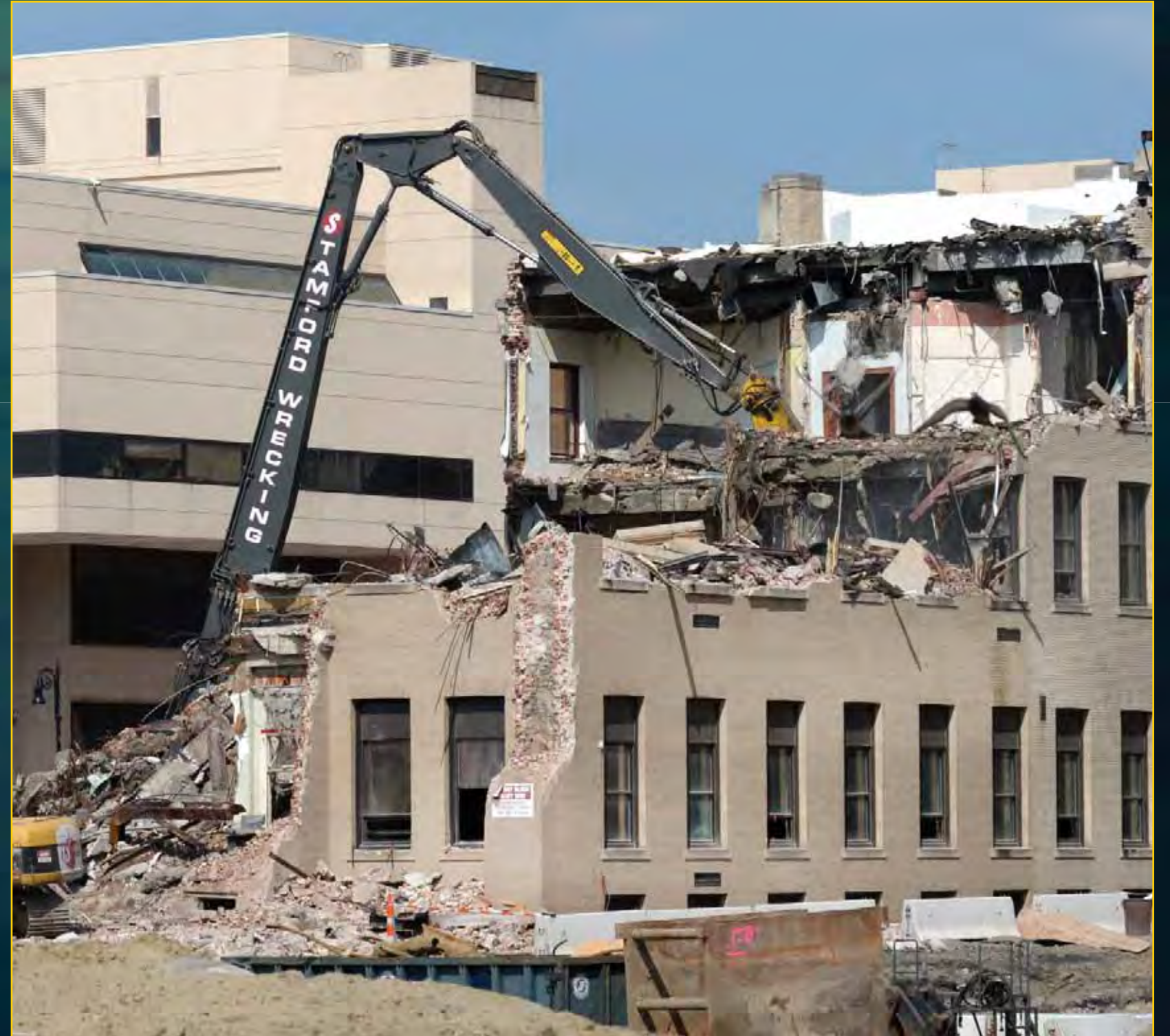
73 State Demolition - June 20, 2016
