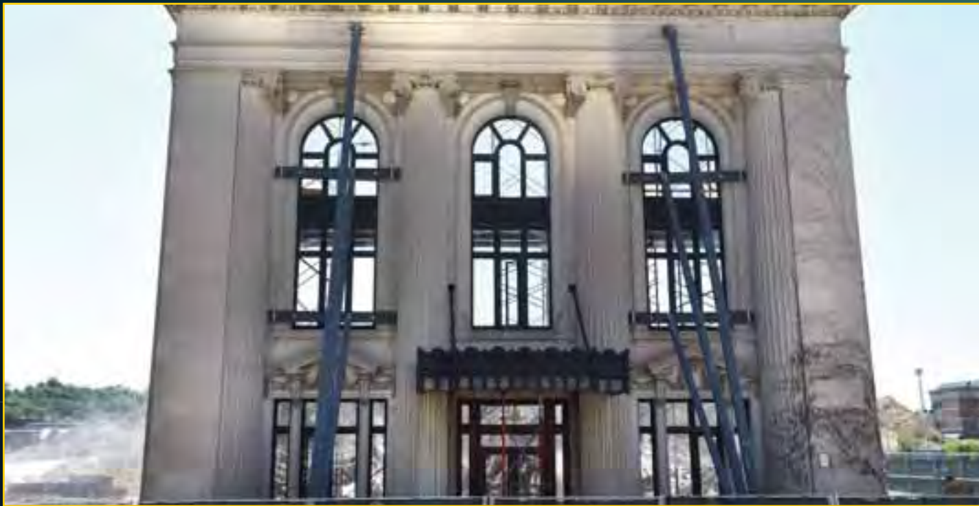
73 State Demolition - June 24, 2016
