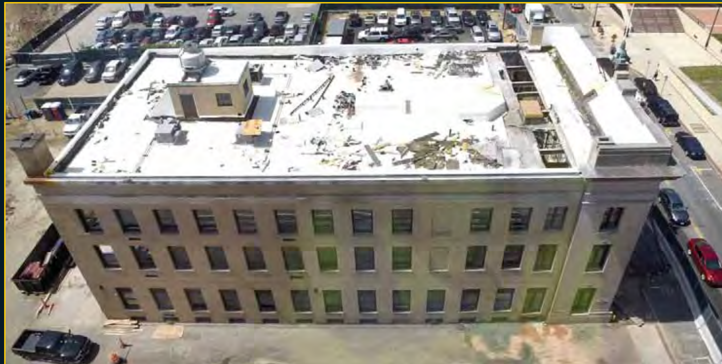
73 State Demolition - June 1, 2016
