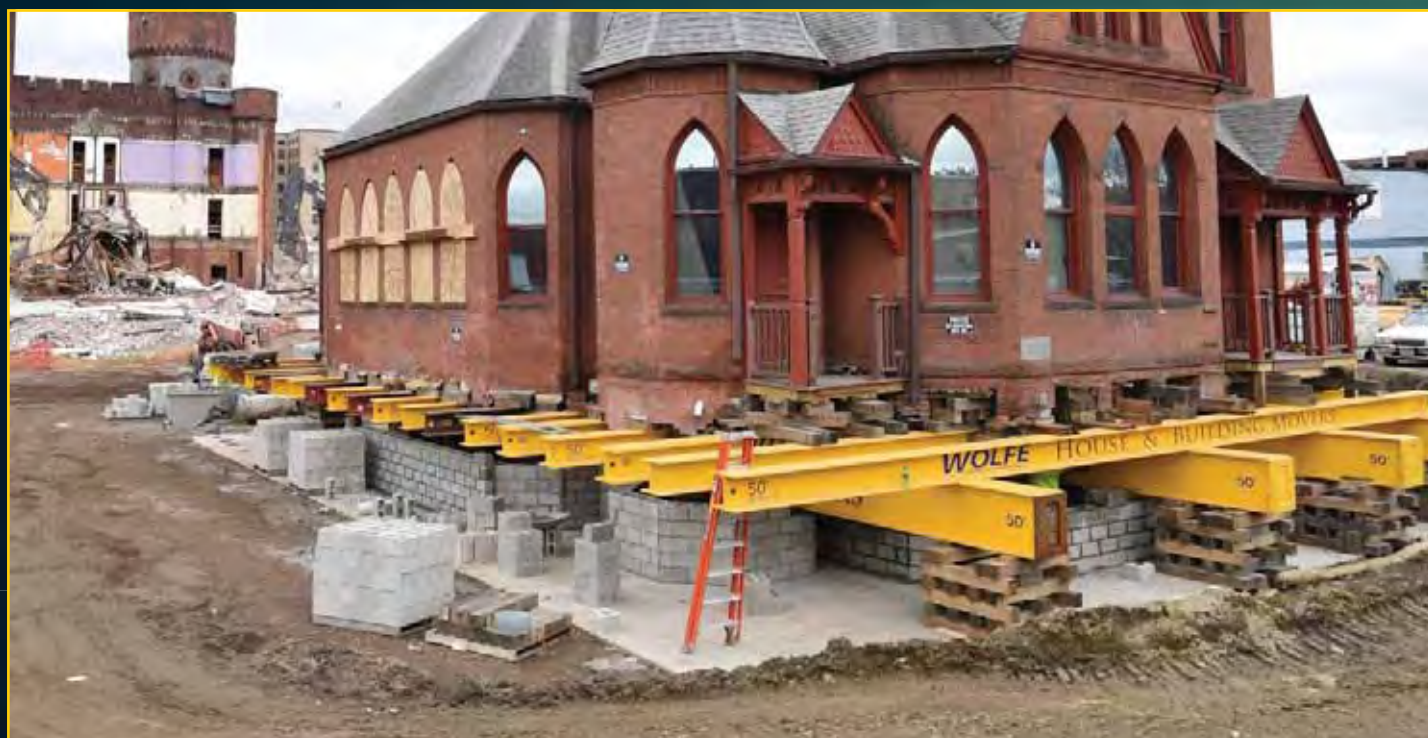
New Church Foundation - May 6, 2016
