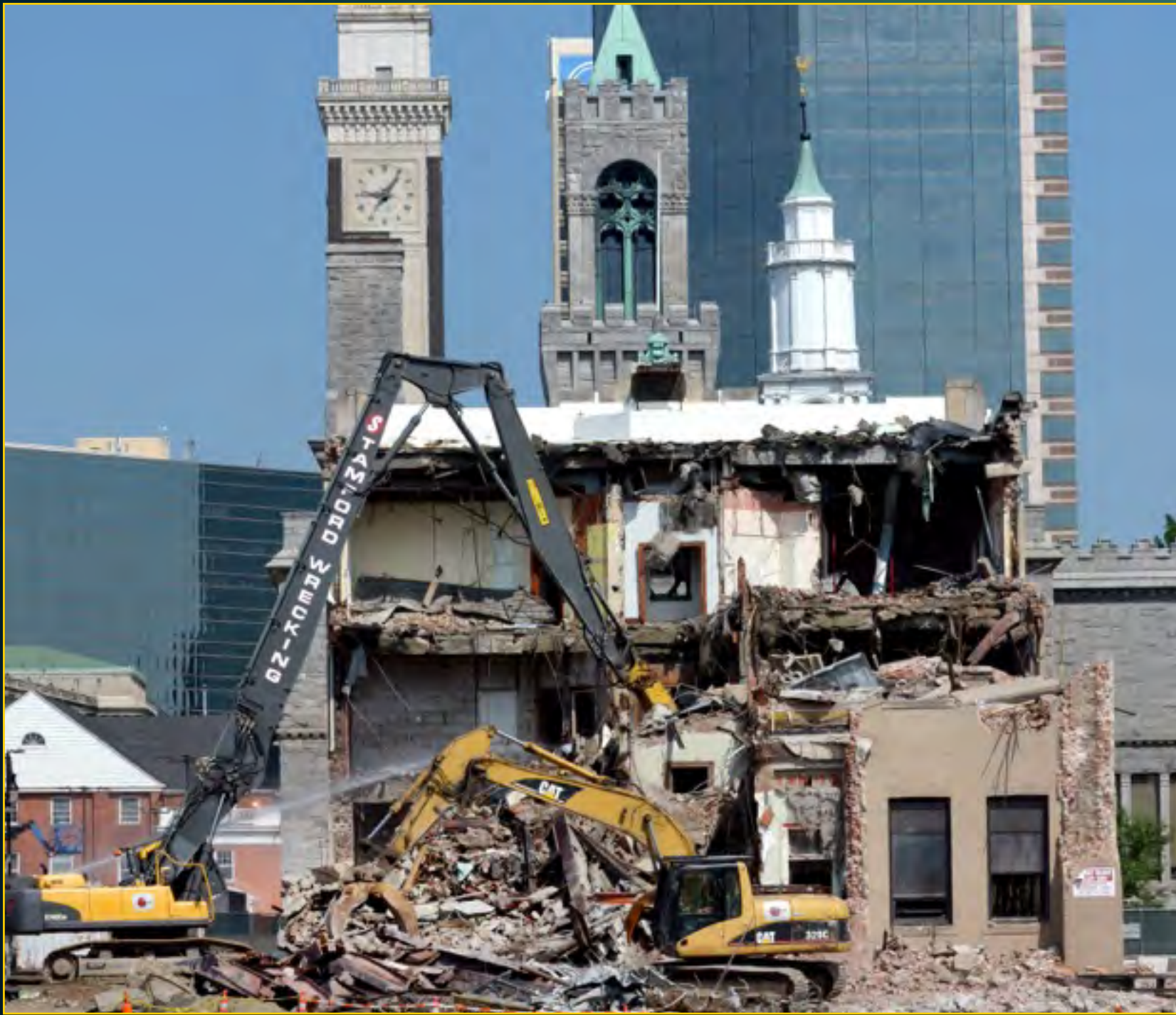
73 State Demolition - June 20, 2016
