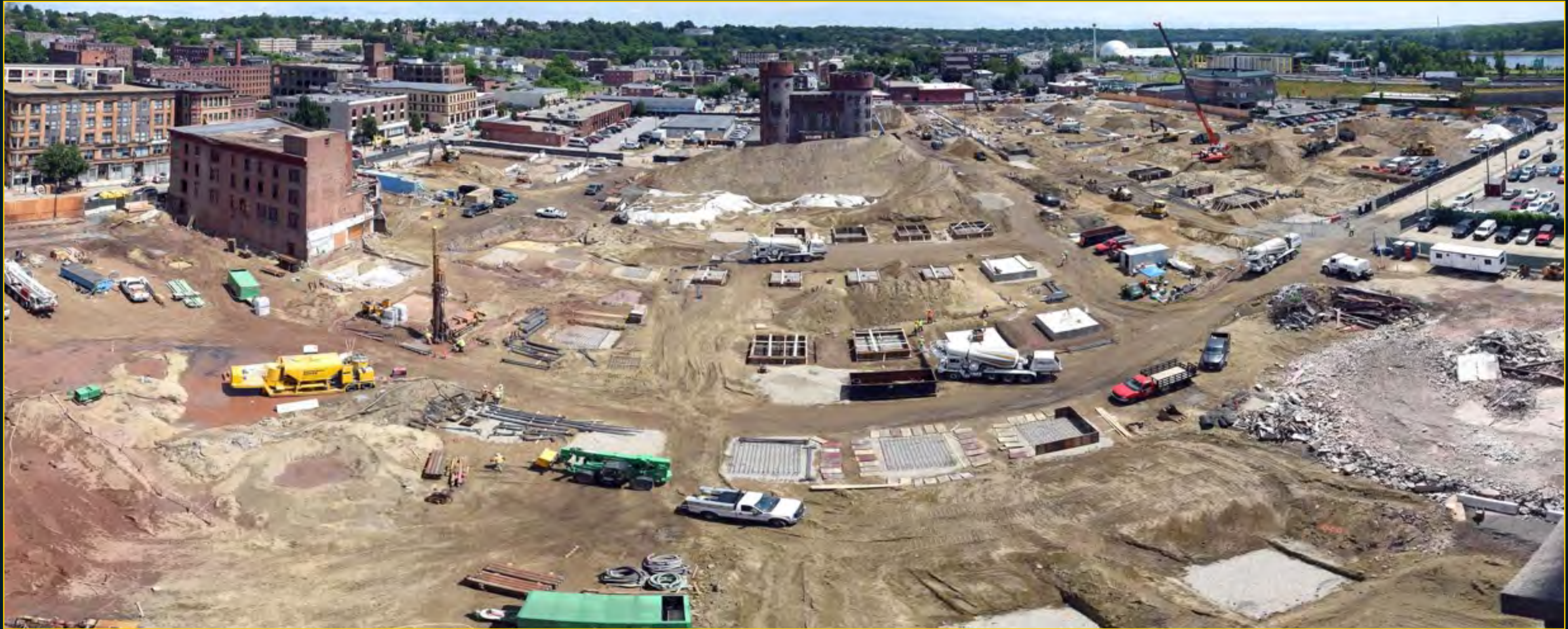
Overall Site Activity - June 28, 2016
