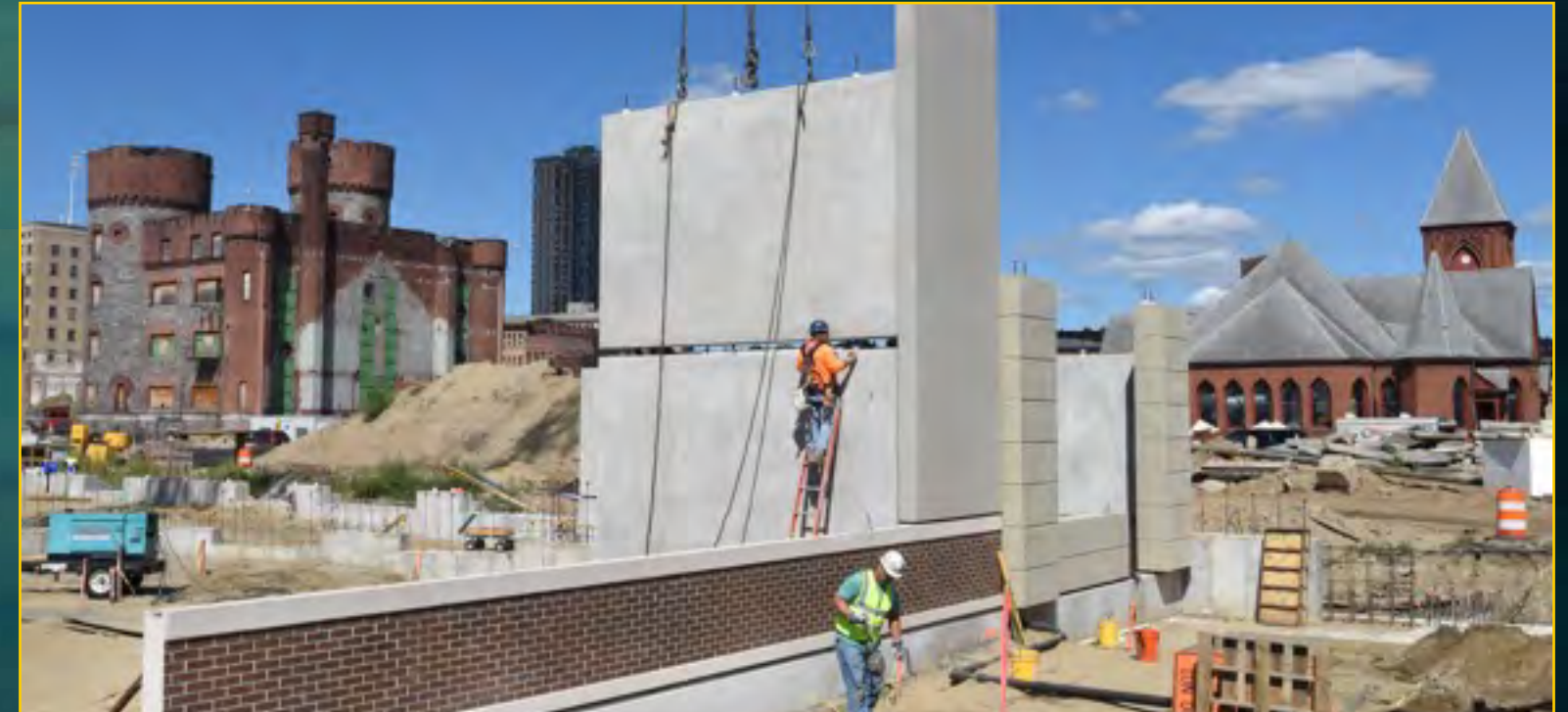
Garage Precast Panels - September 14, 2016
