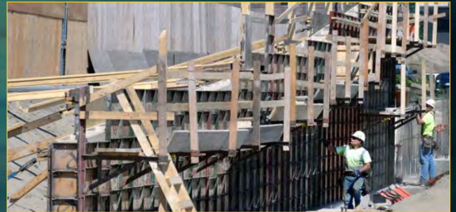
Garage Construction - June 24, 2016
