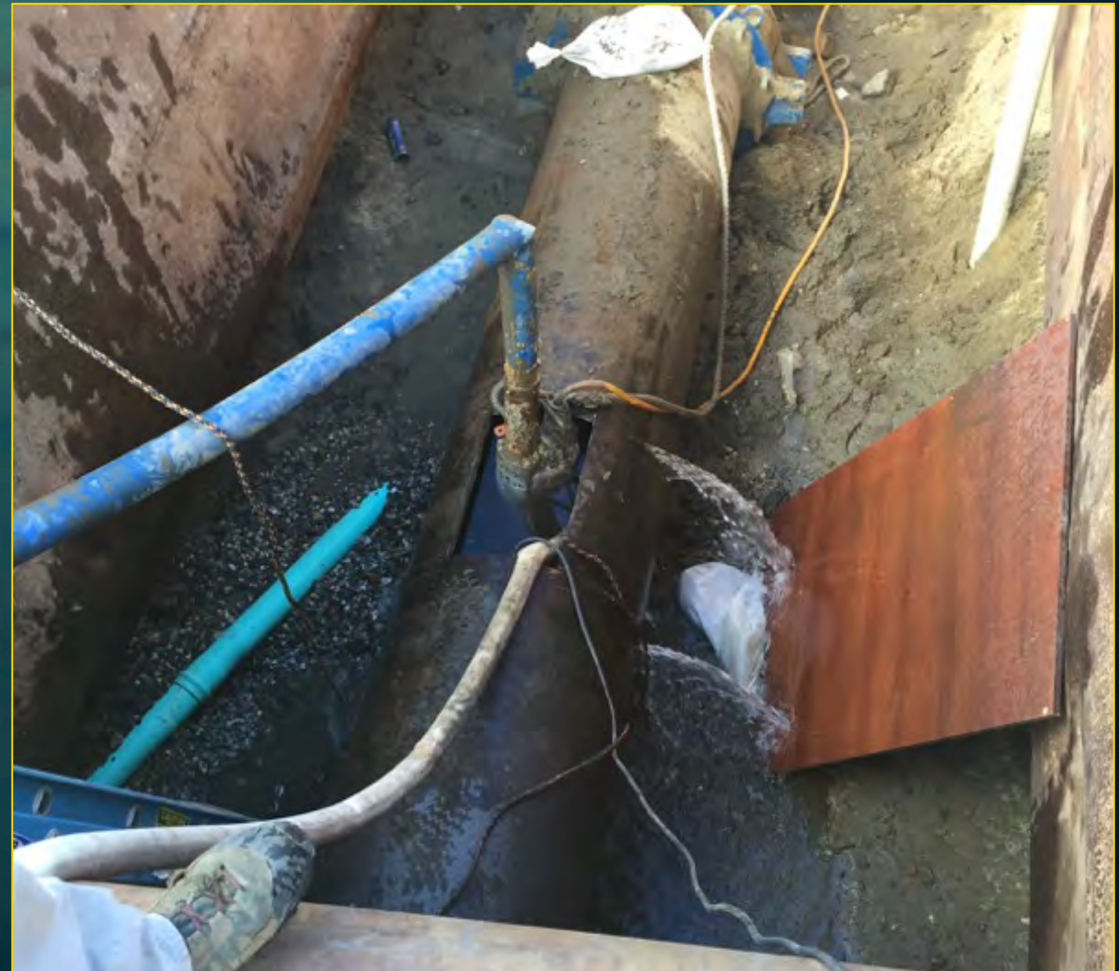
New Valve Work at Union Street Water Main - June 13, 2016
