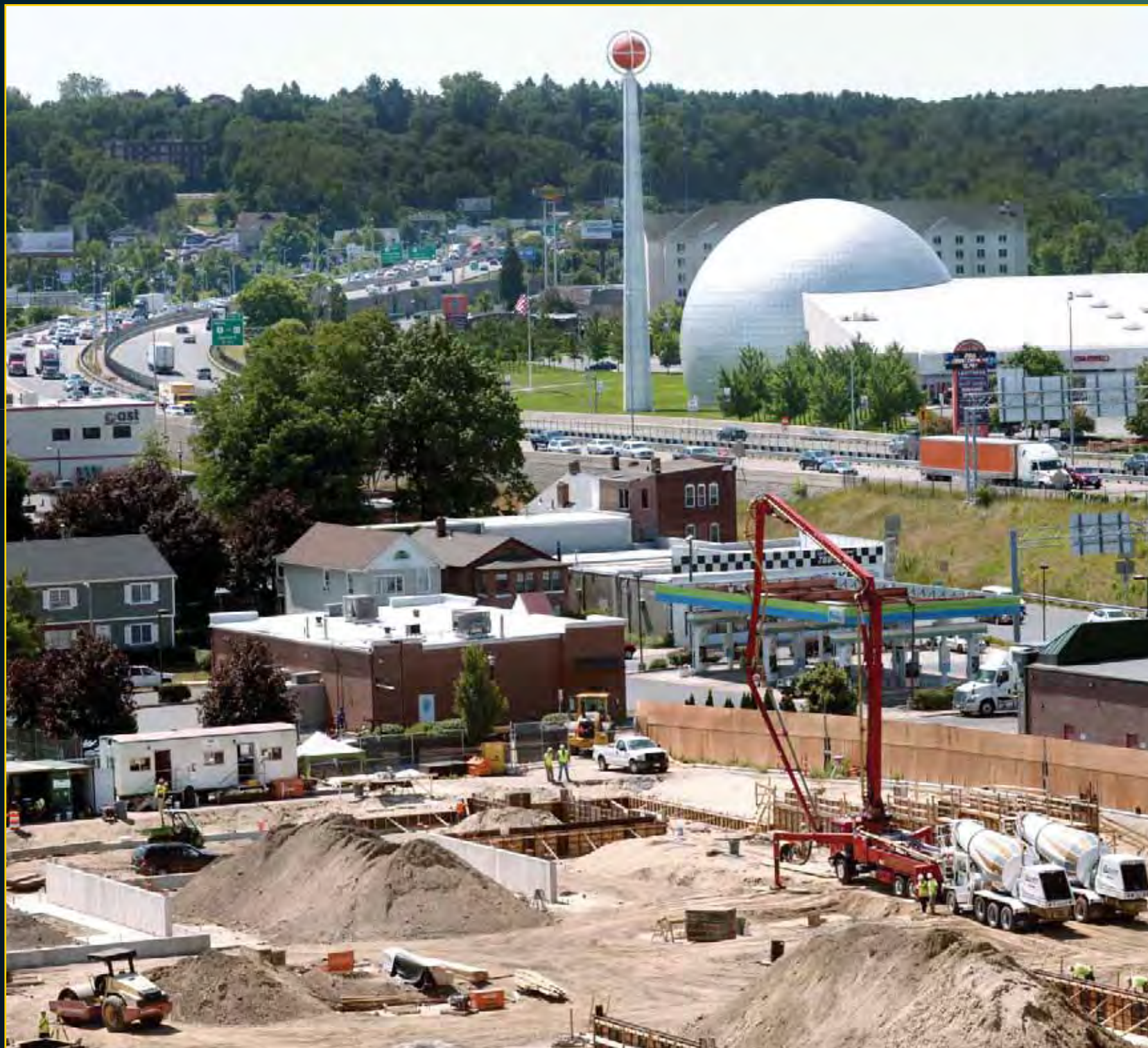
Garage Construction - June 24, 2016
