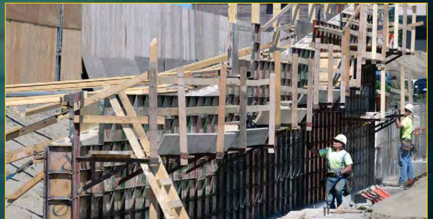
Garage Construction - June 24, 2016
