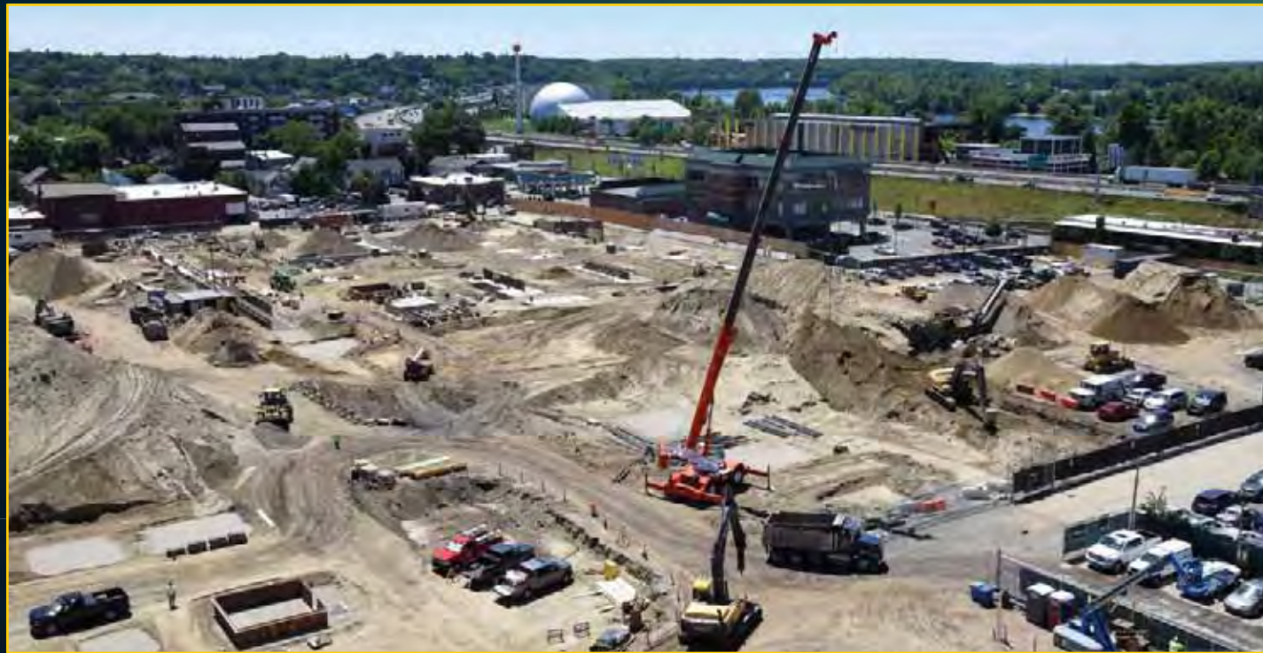
Podium Footings Prepared - June 21, 2016
