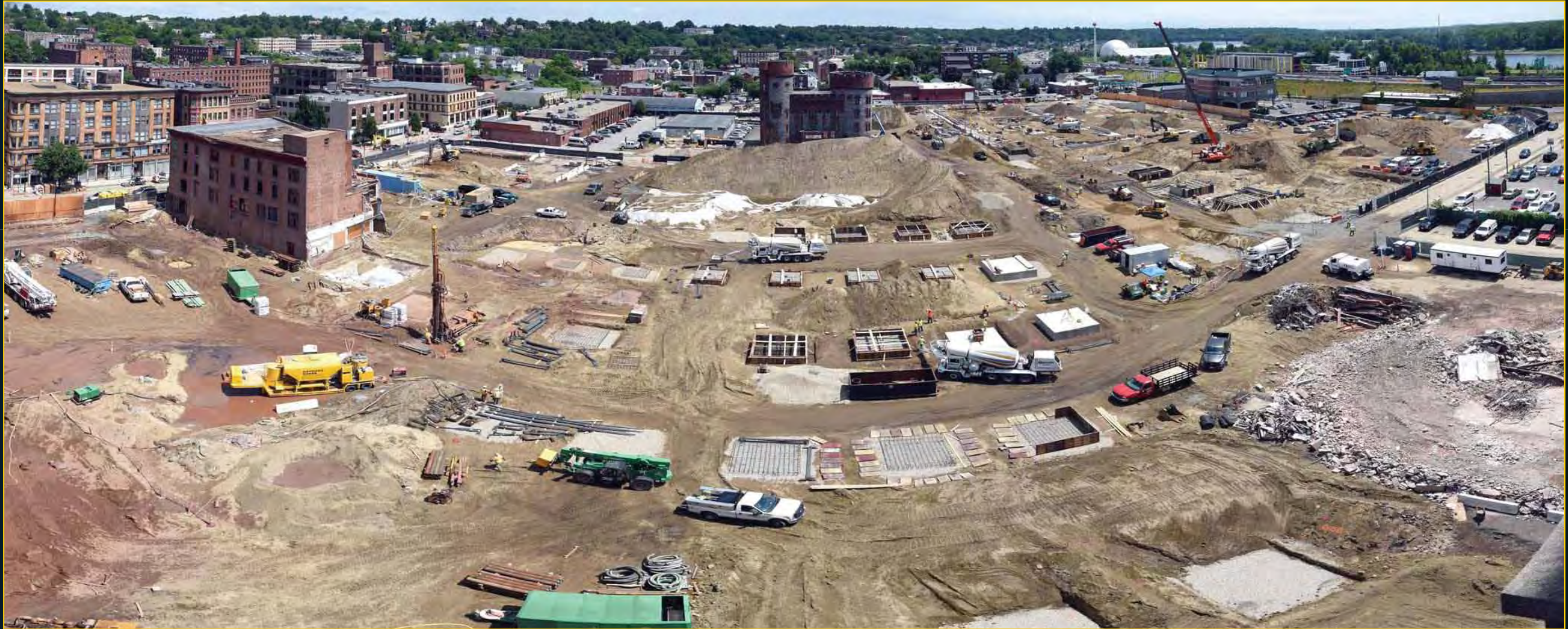
Overall Site Activity - June 28, 2016
