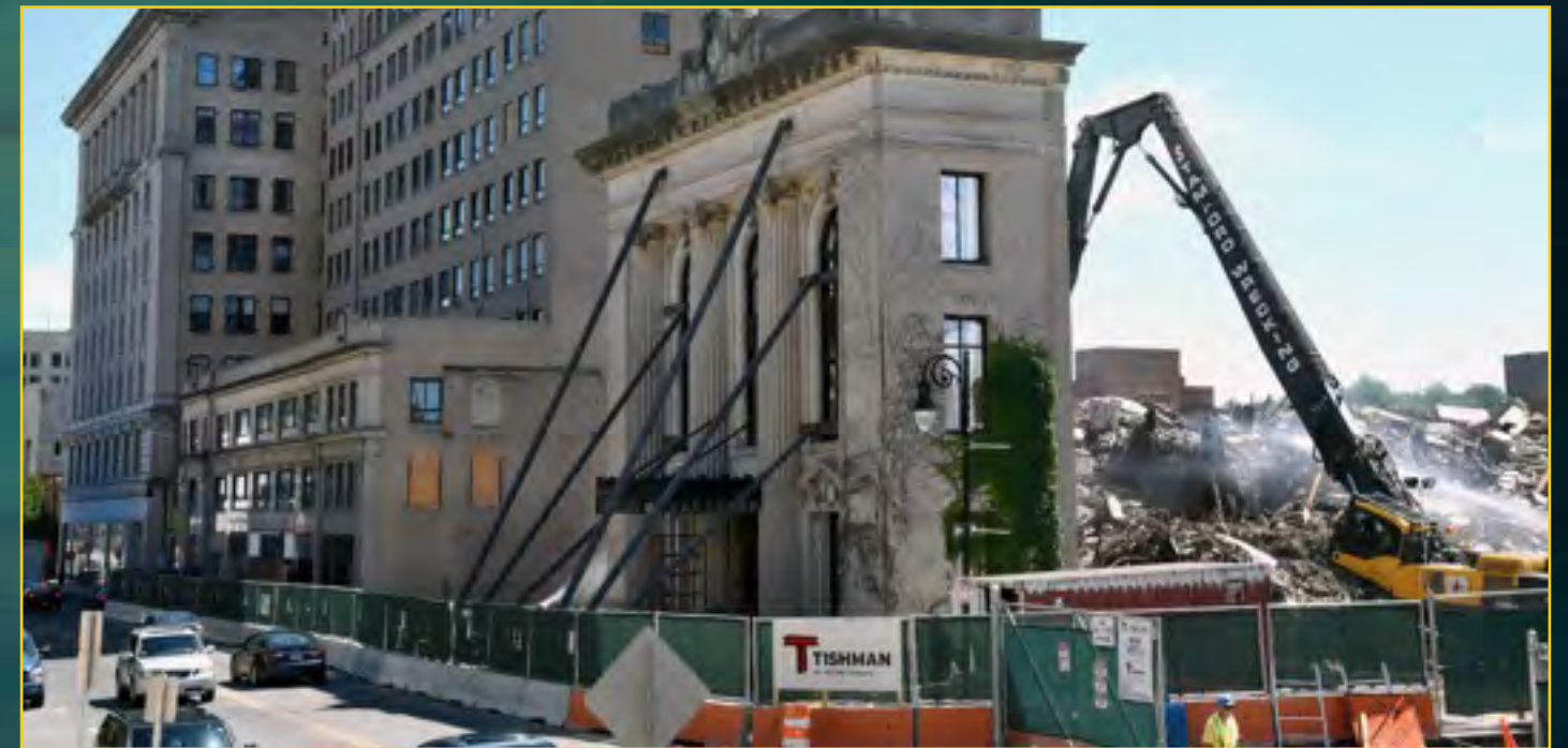
73 State Demolition - June 21, 2016
