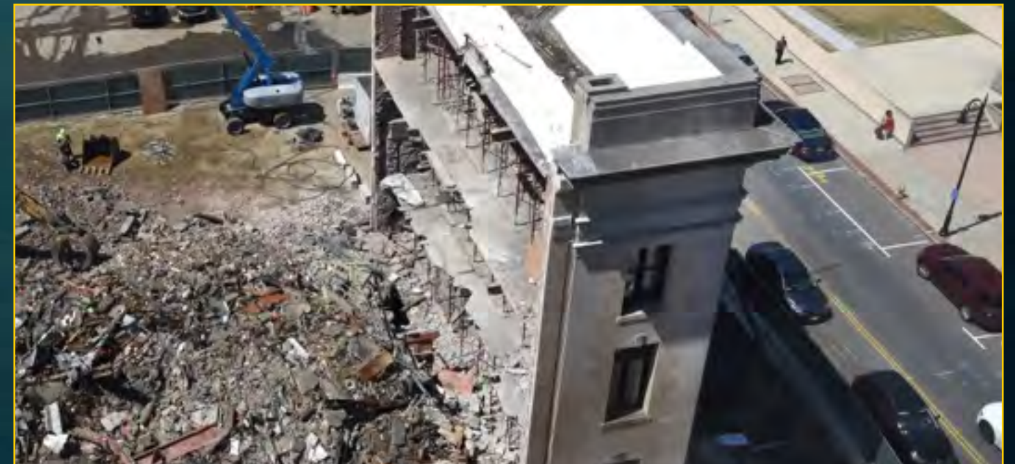
73 State Demolition - June 24, 2016
