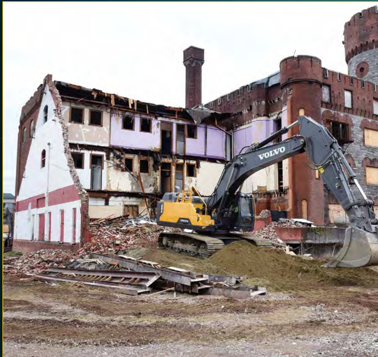
Armory Demolition - May 5, 2016
