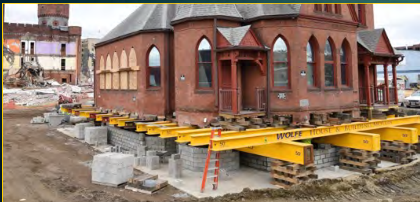
New Church Foundation - May 6, 2016
