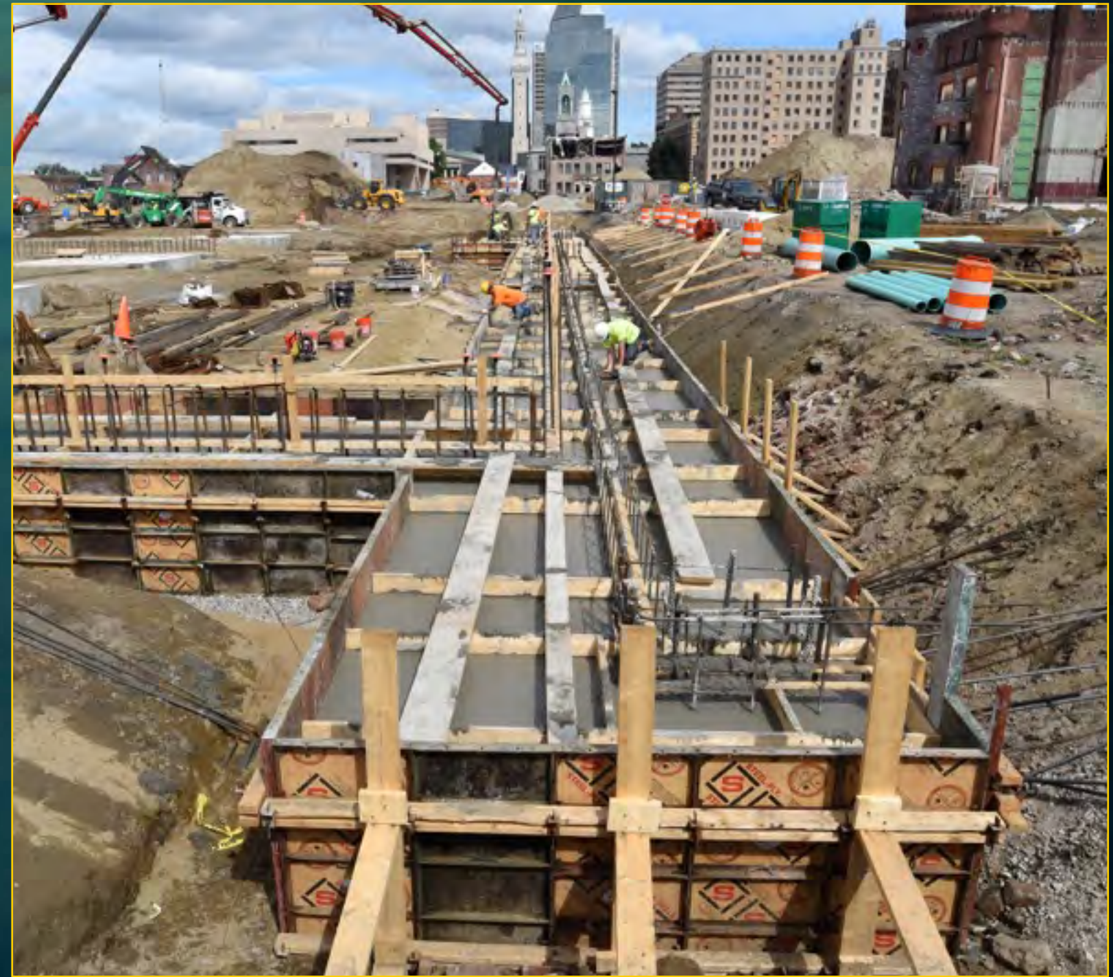
Garage Construction - June 8, 2016
