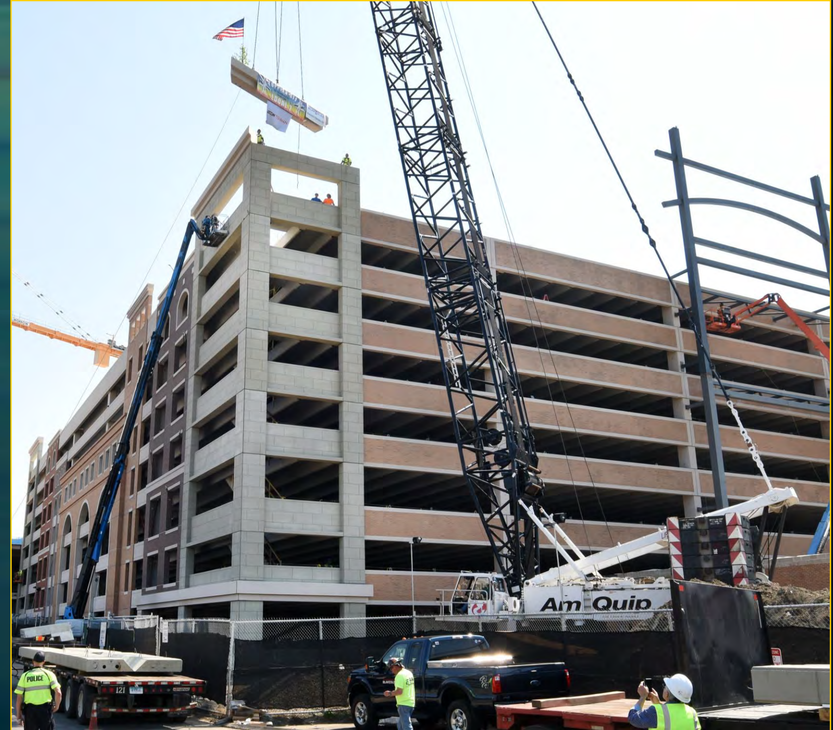
Garage Topping Off - May 17, 2017
