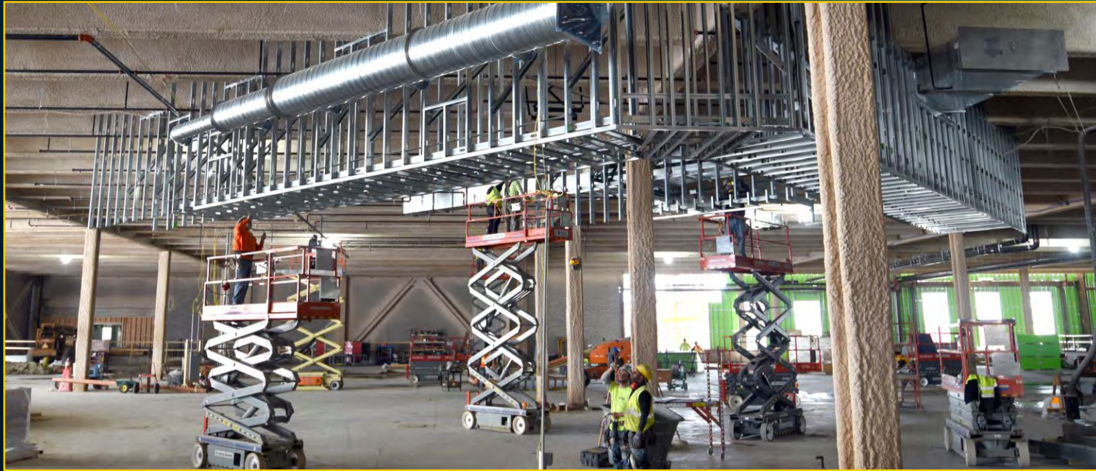
Podium Framing - May 23, 2017
