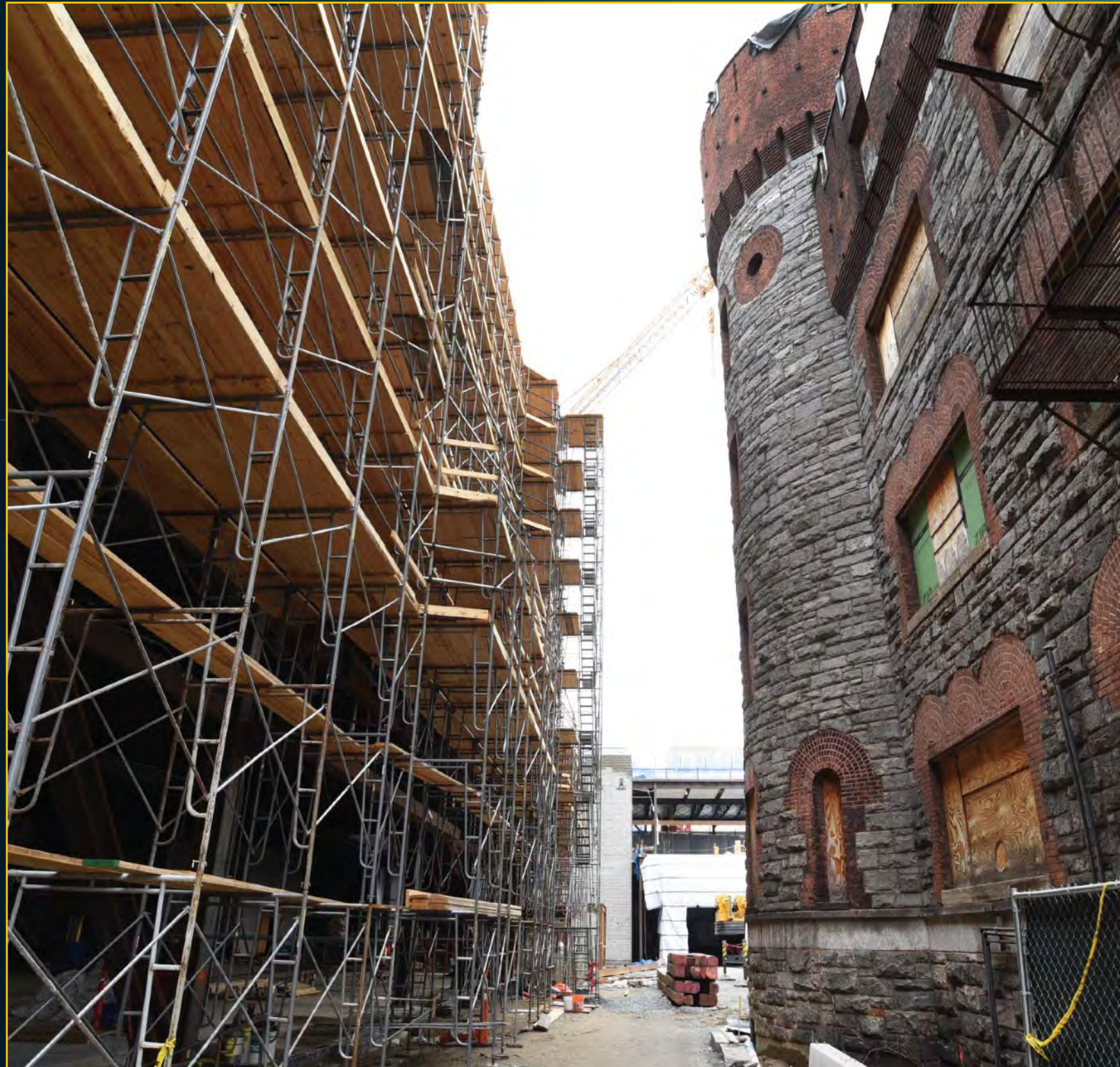
Entertainment Block Construction - April 5, 2017
