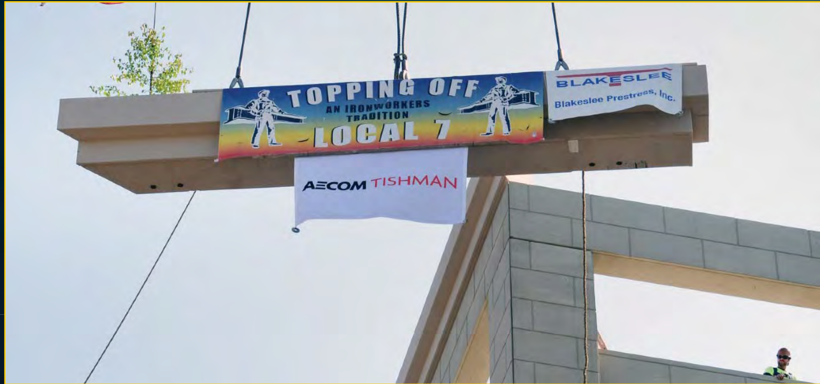
Garage Topping Off - May 17, 2017
