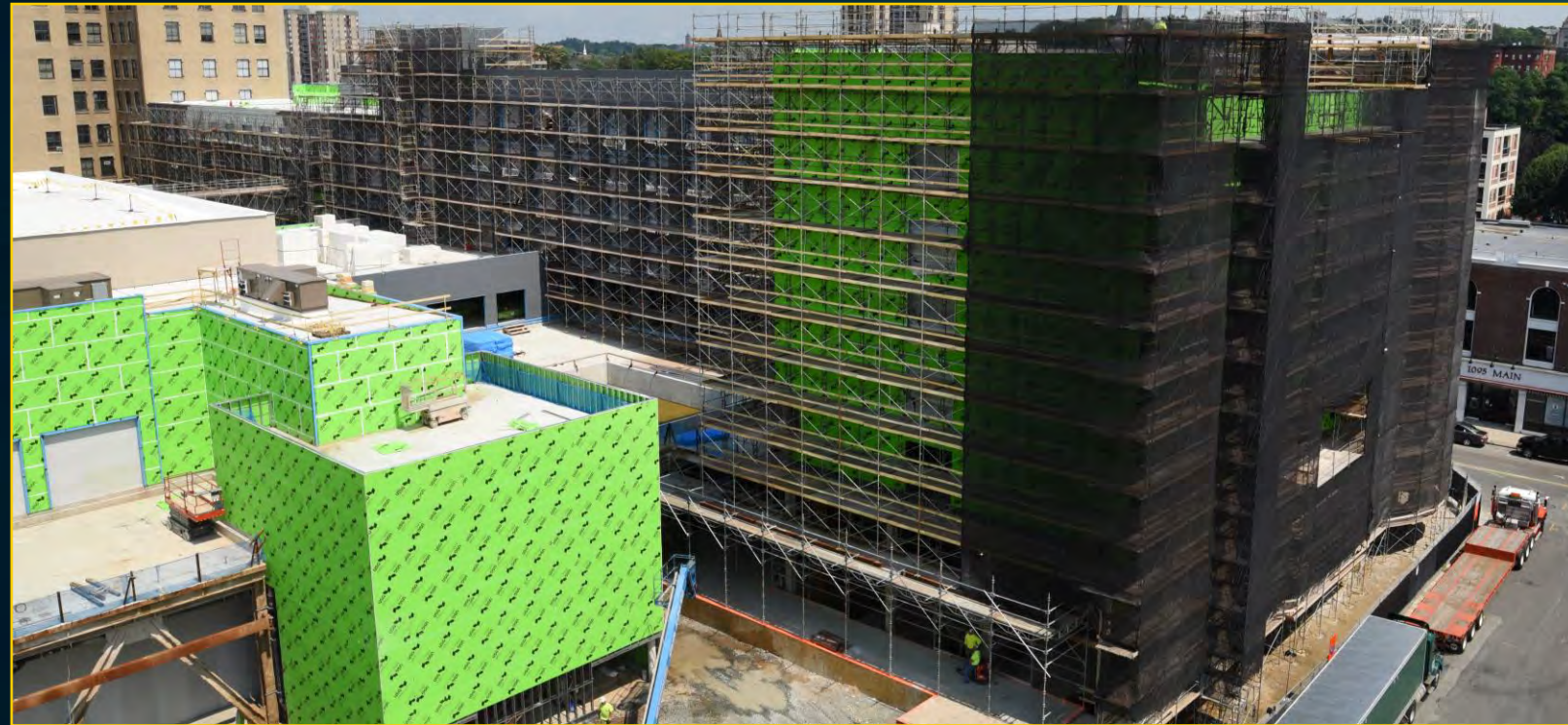
Hotel Construction - July 18, 2017
