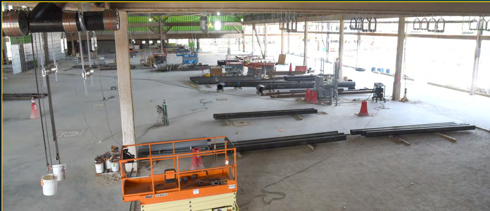
Podium MEP - May 23, 2017
