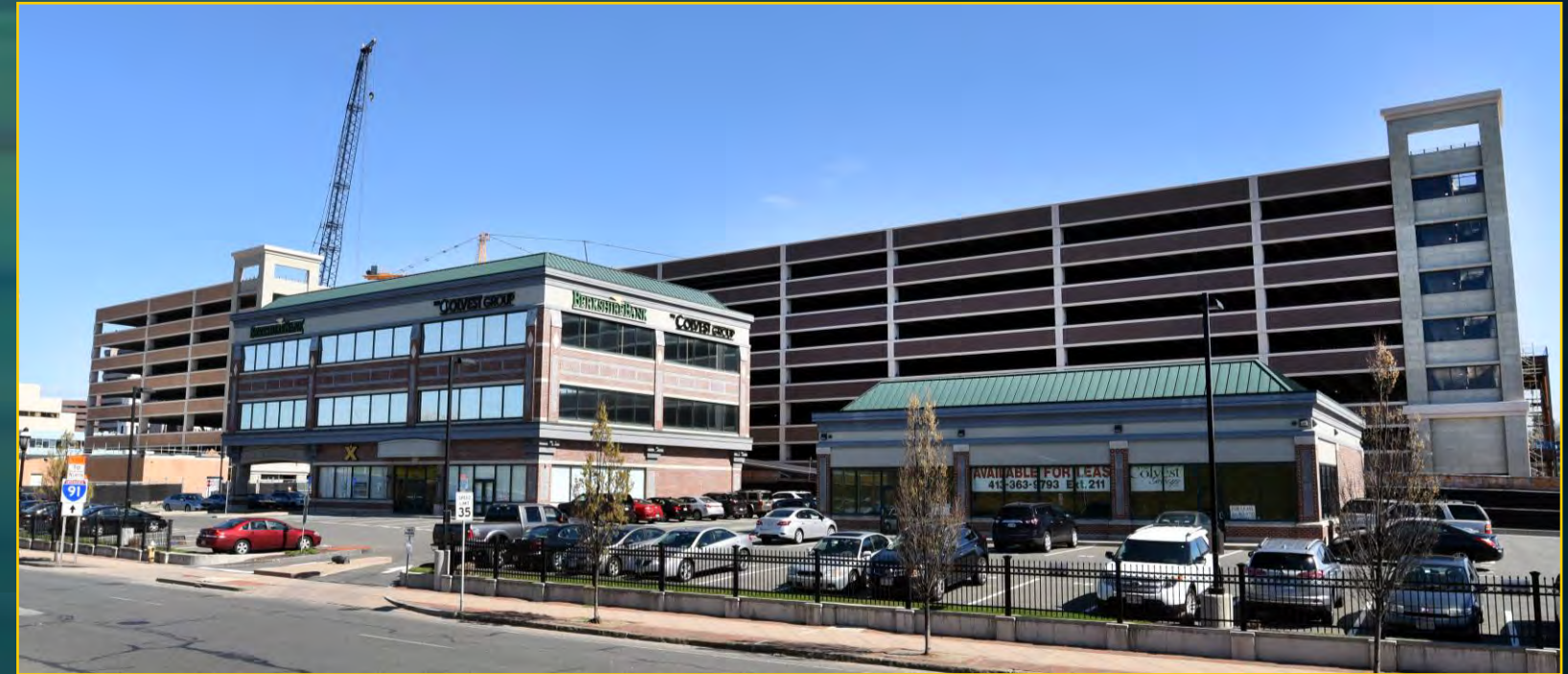
Garage Construction - April 18, 2017
