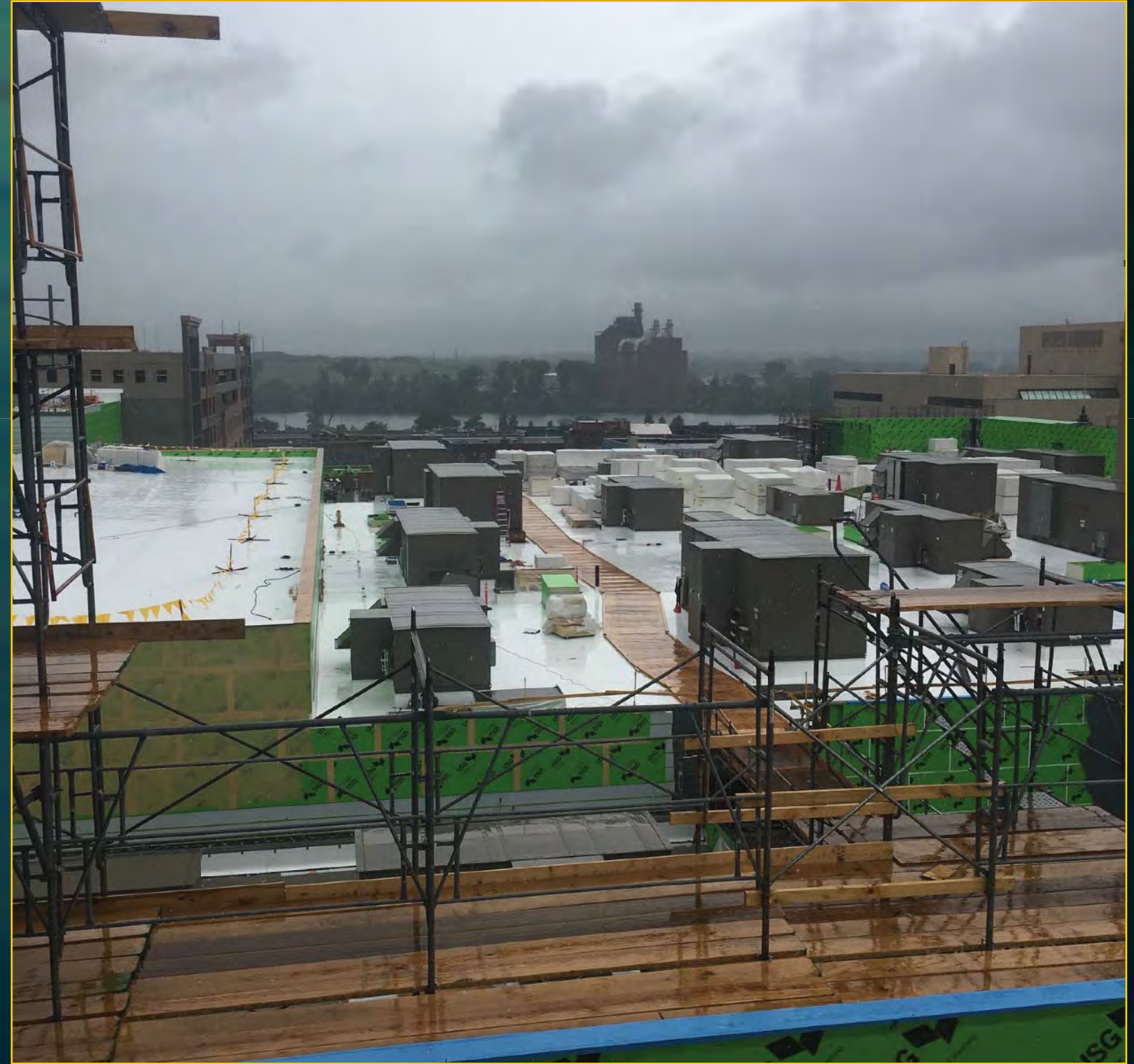
Podium Air Handlers Lifted in Place - June 6, 2017
