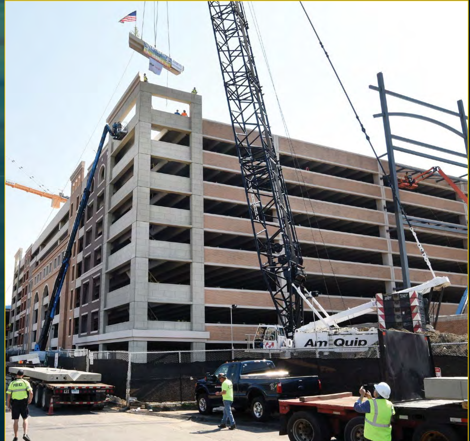
Garage Topping Off - May 17, 2017
