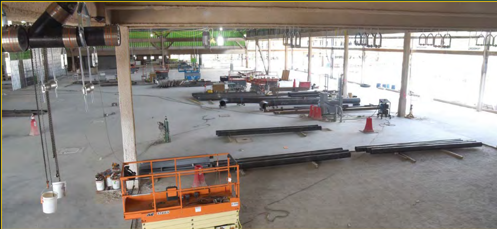
Podium MEP - May 23, 2017
