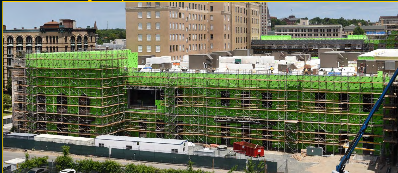
Podium Construction - June 15, 2017
