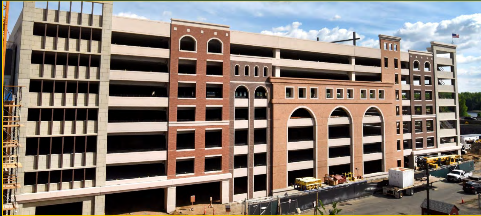
Parking Garage Facade - May 24, 2017
