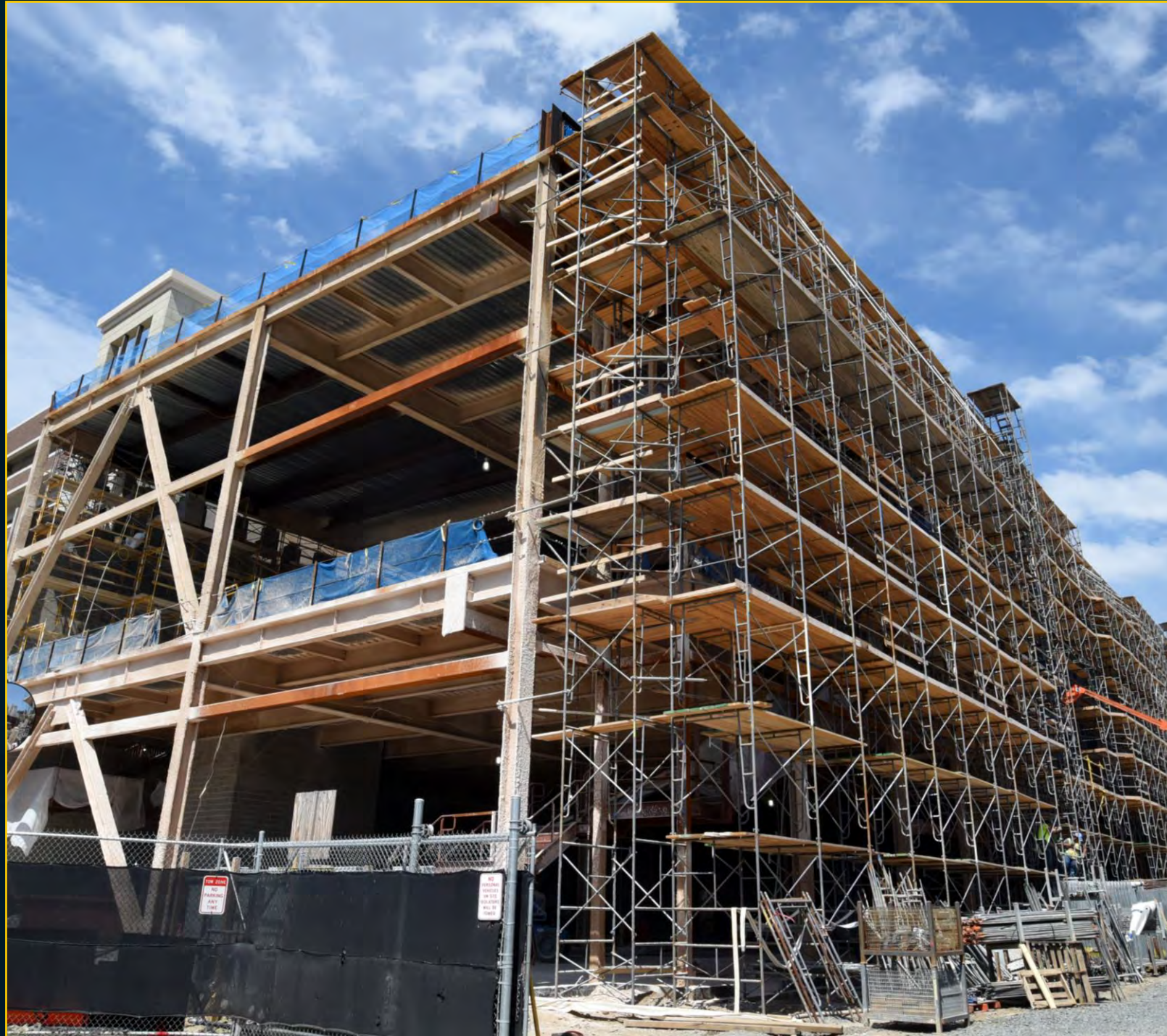
Entertainment Block Construction - June 15, 2017
