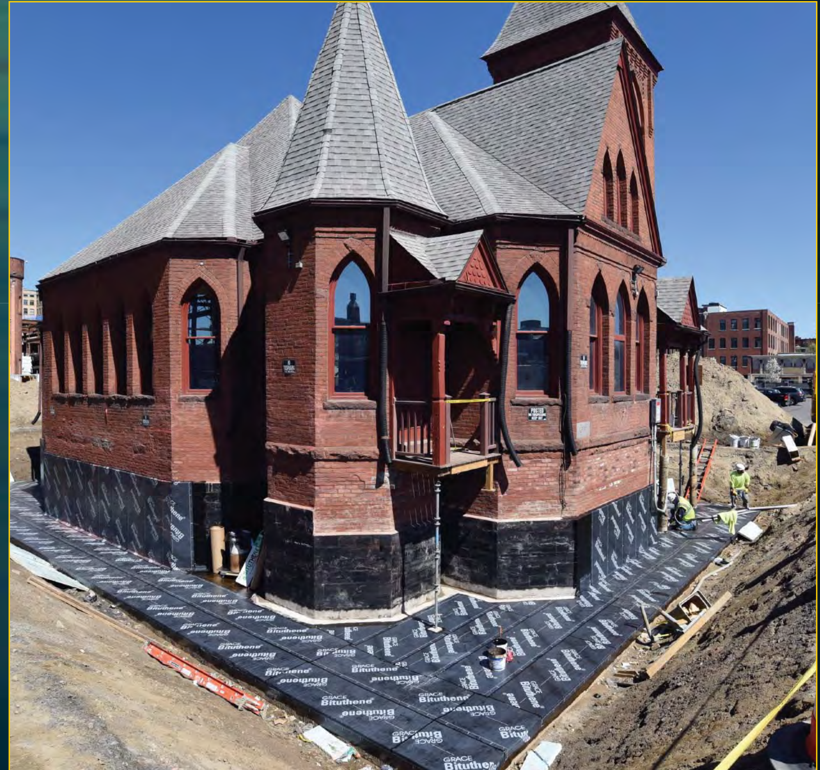
Church Construction - April 18, 2017
