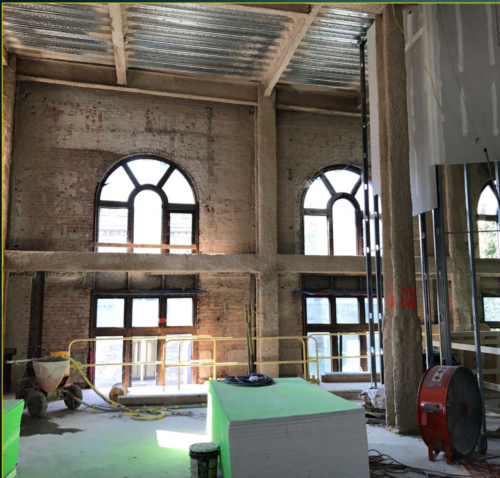
Uniform Control Construction - August 1, 2017
