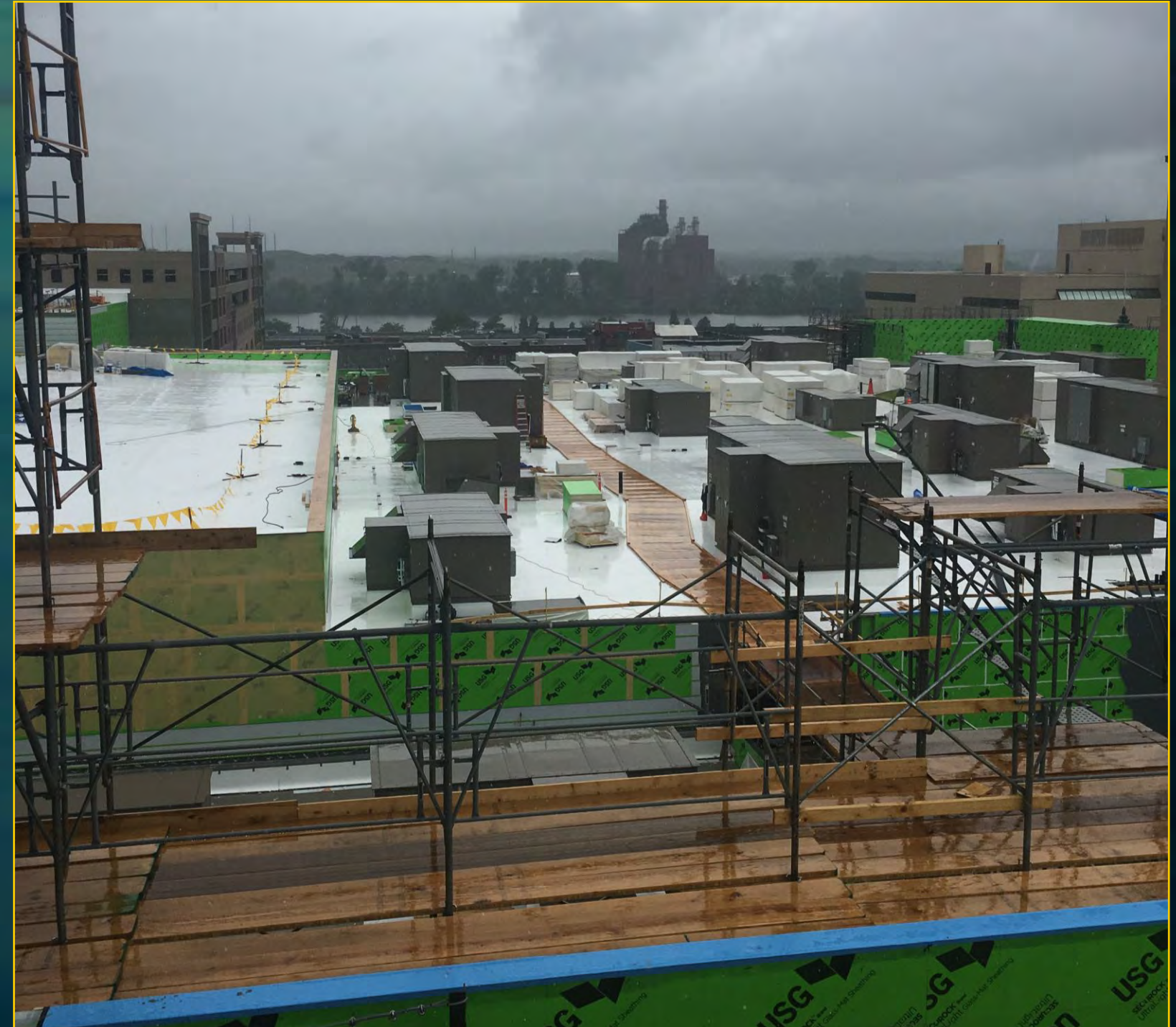
Podium Air Handlers Lifted in Place - June 6, 2017
