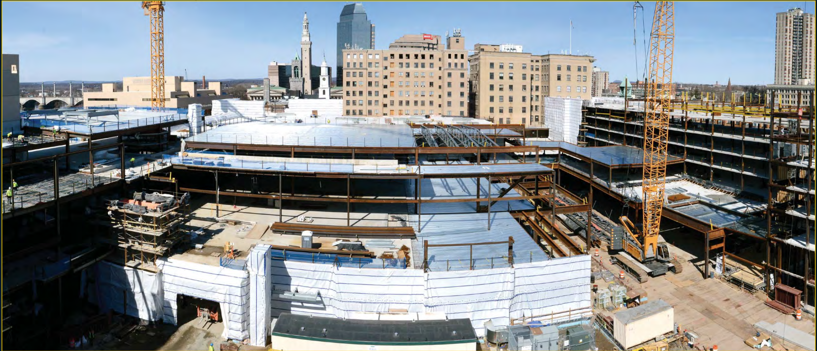
Overall Site Activity from Armory - March 13, 2017
