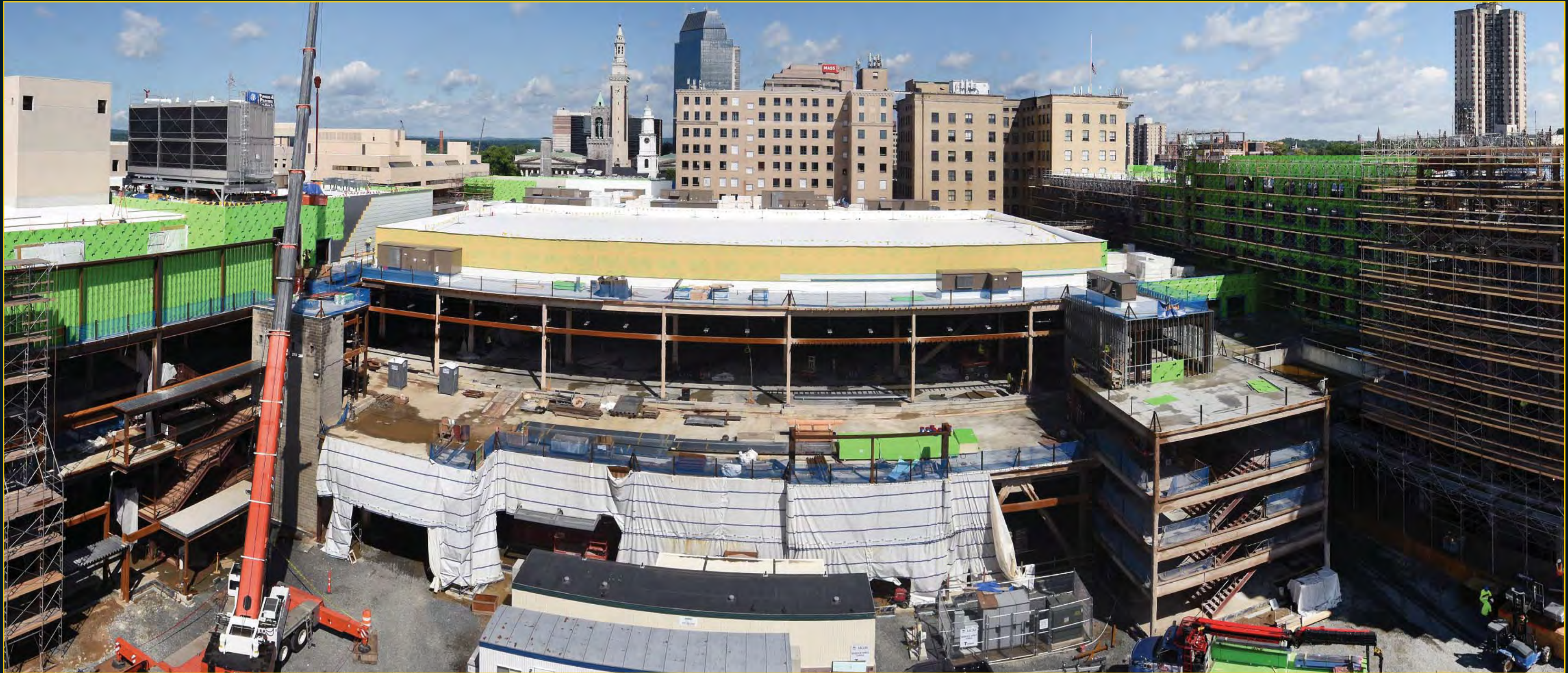
Overall Site Activity from Armory - June 20, 2017
