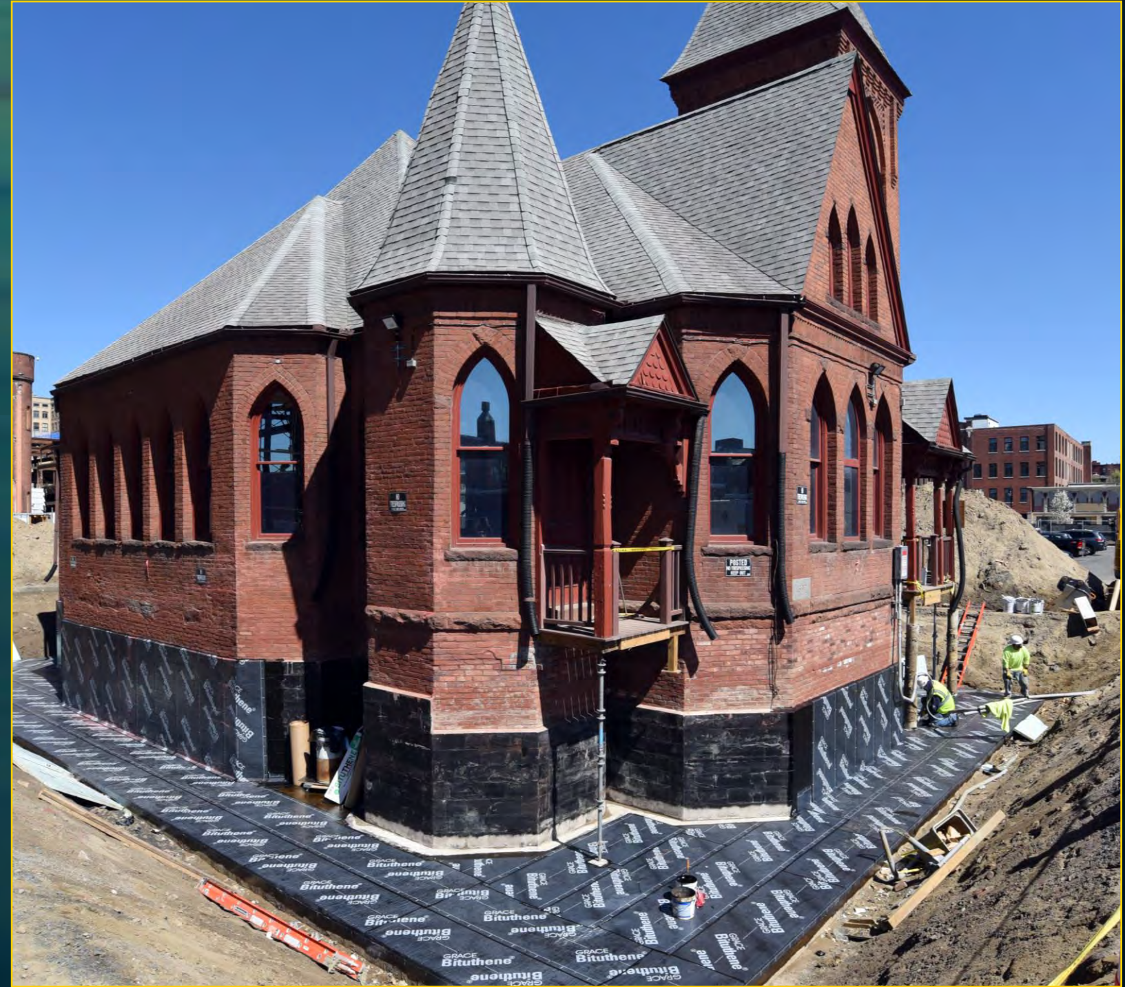
Church Construction - April 18, 2017
