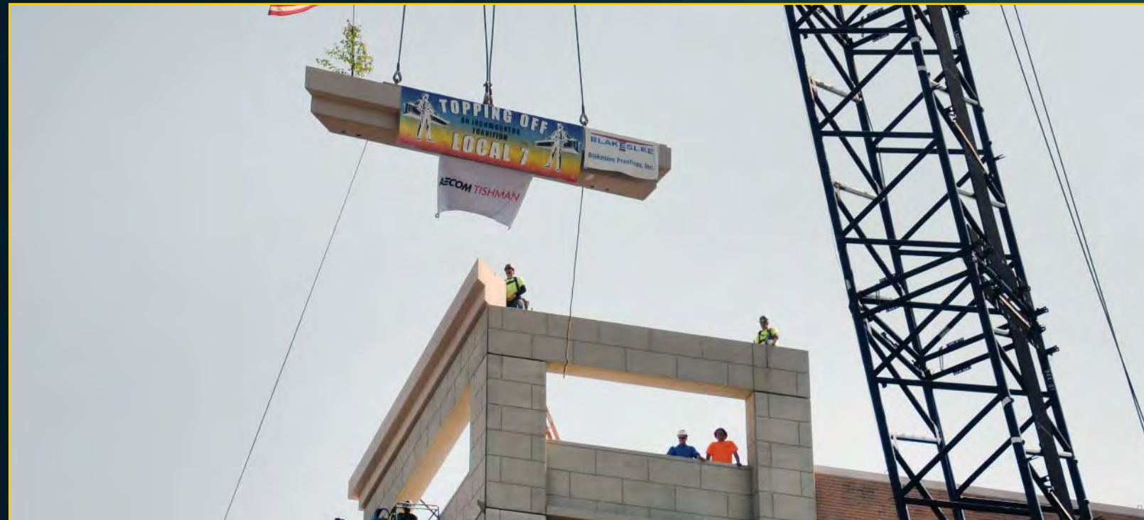
Garage Topping Off - May 17, 2017
