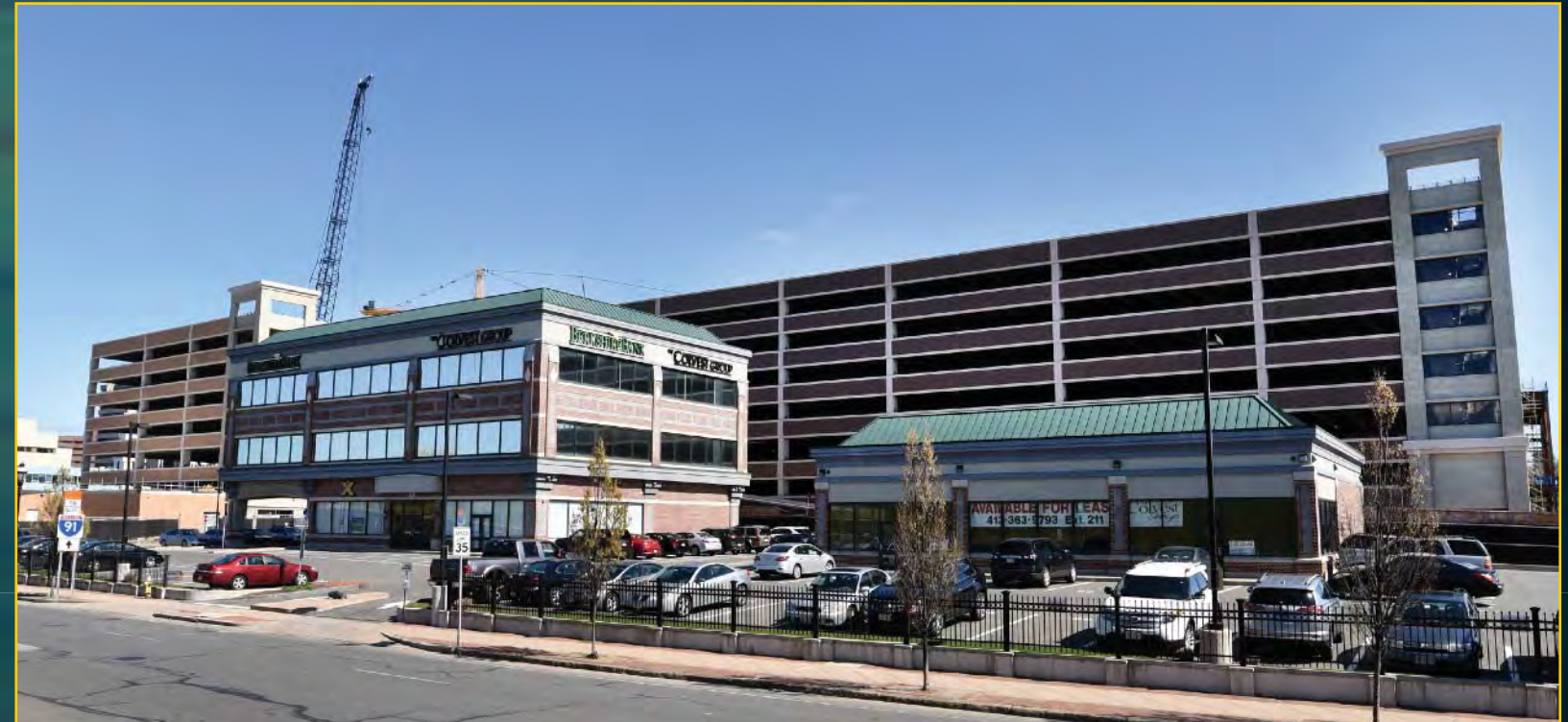
Garage Construction - April 18, 2017
