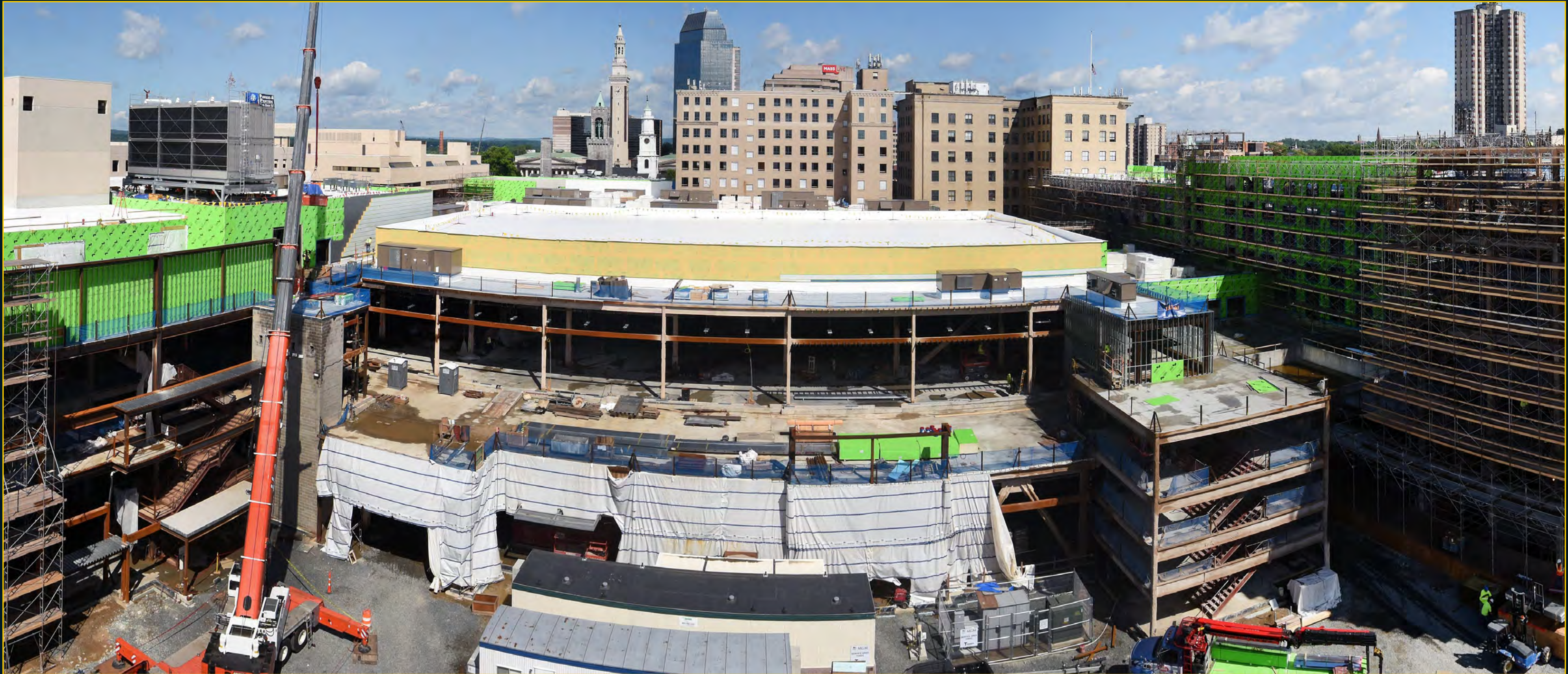
Overall Site Activity from Armory - June 20, 2017
