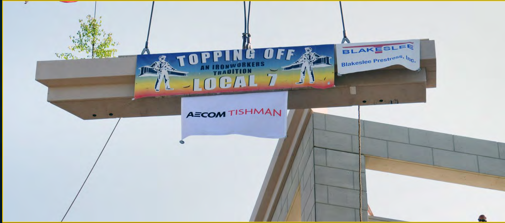
Garage Topping Off - May 17, 2017
