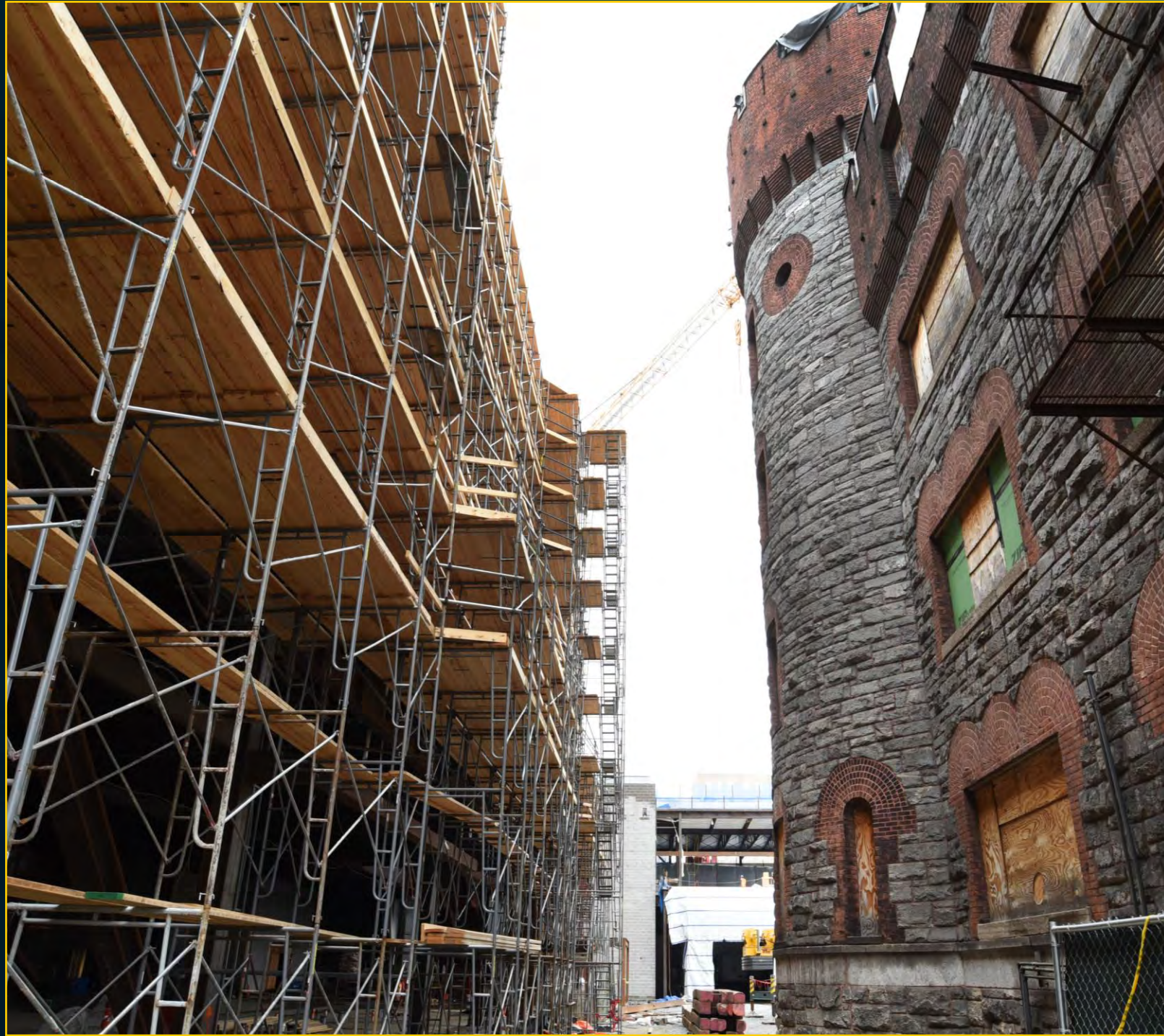
Entertainment Block Construction - April 5, 2017
