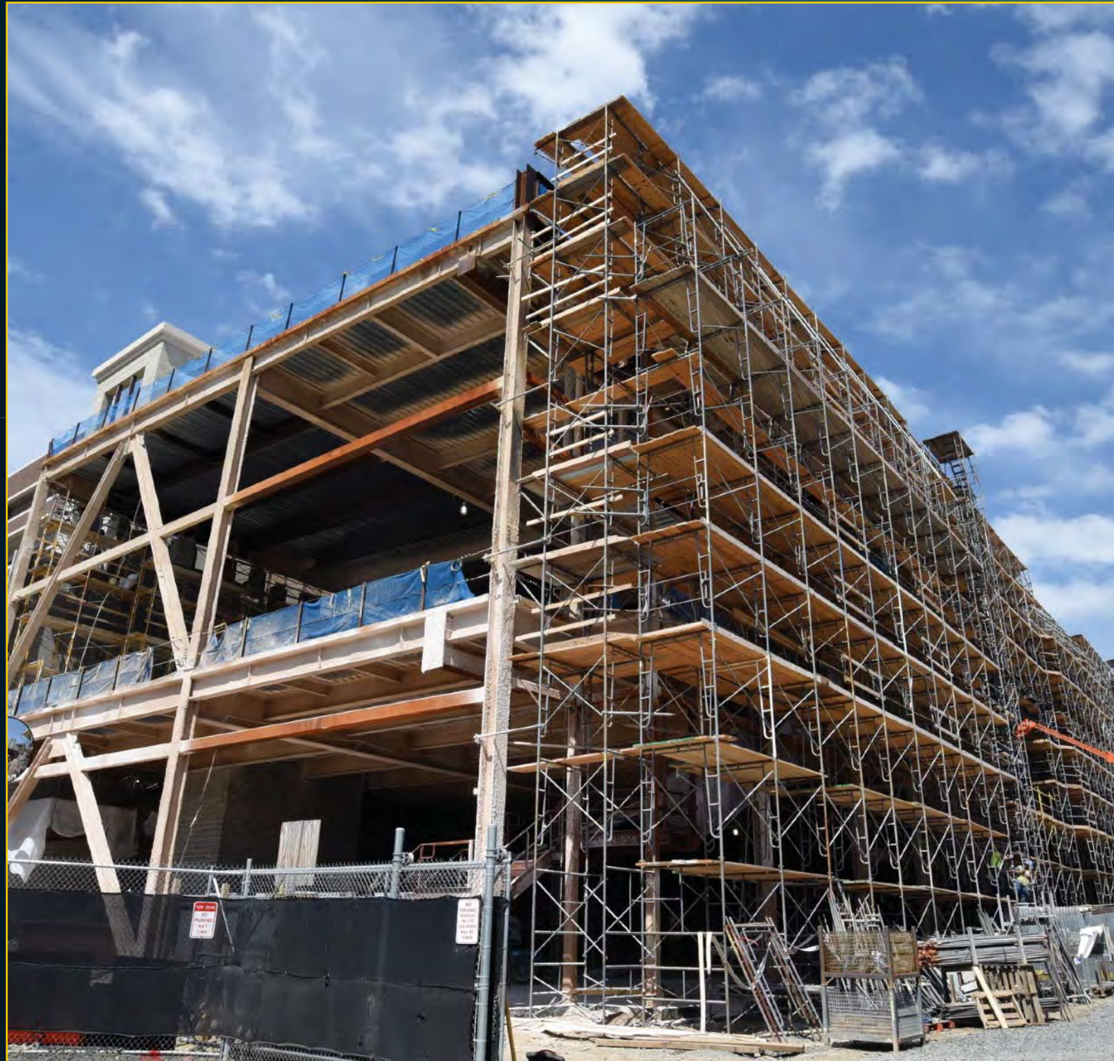
Entertainment Block Construction - June 15, 2017
