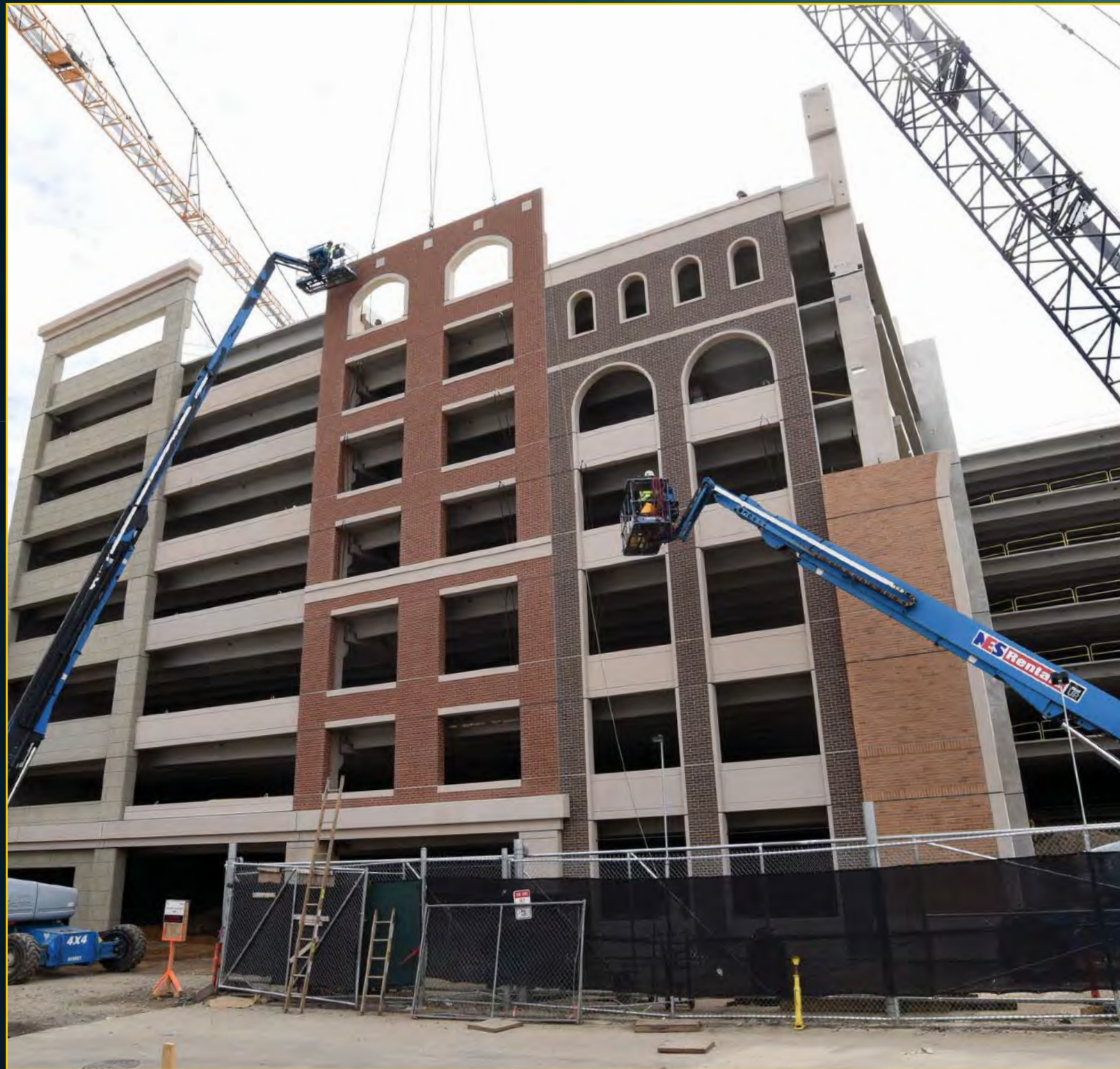
Garage Facade - April 19, 2017
