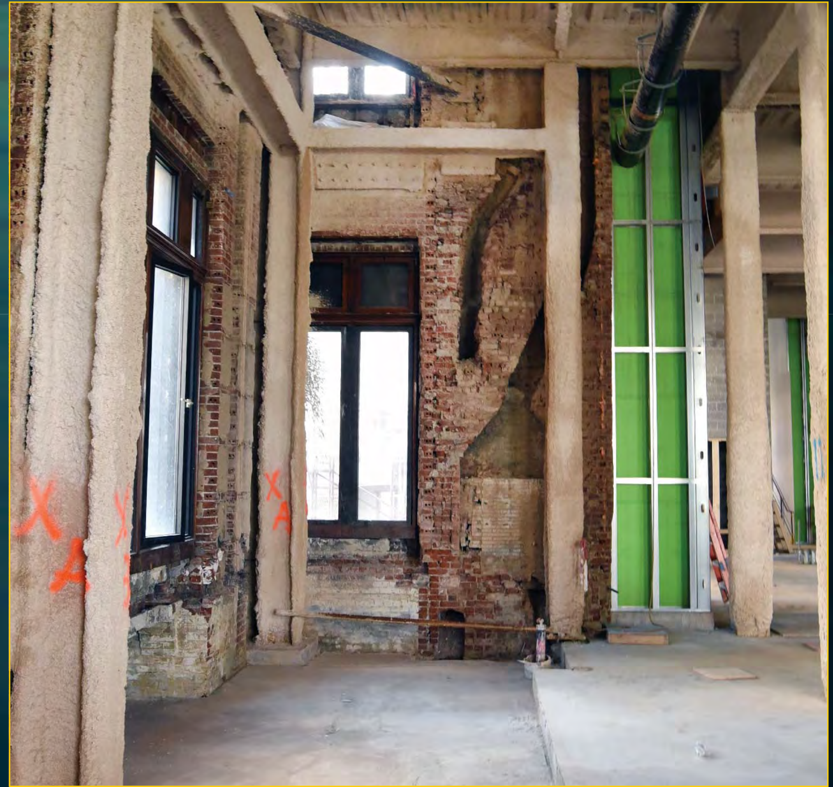
73 State Chimney - June 26, 2017
