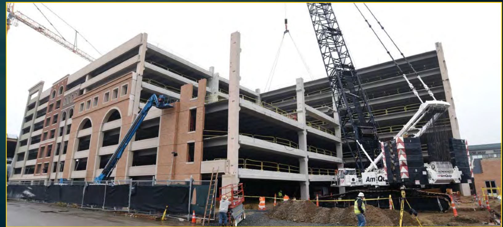
Garage Facade - April 28, 2017
