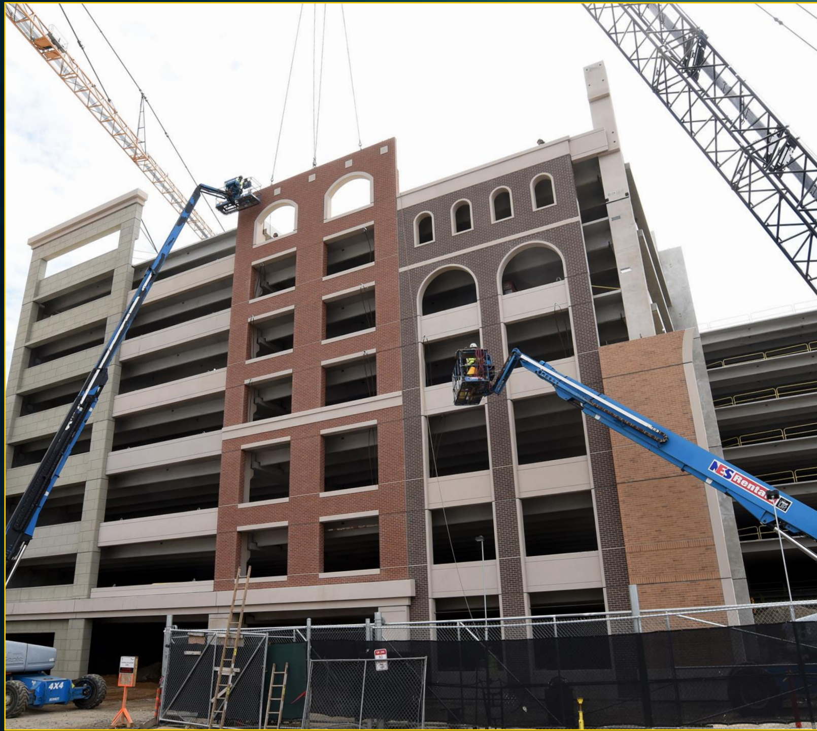
Garage Facade - April 19, 2017
