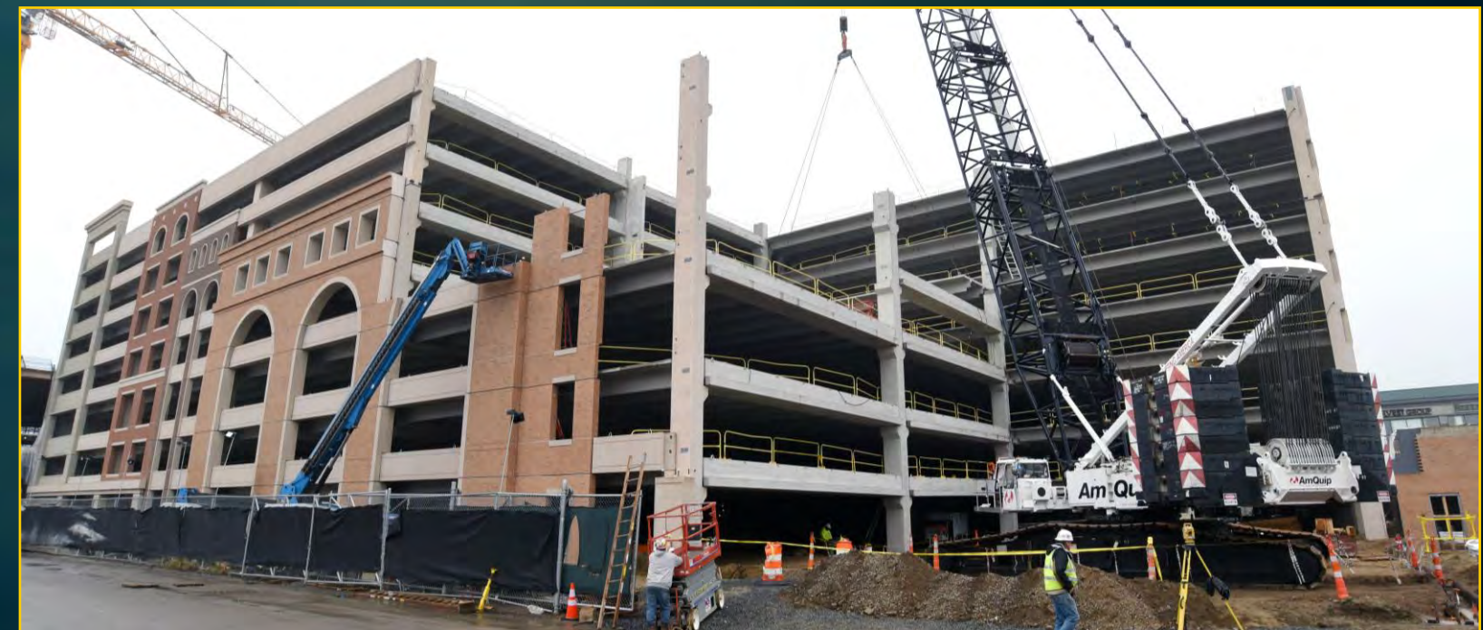
Garage Facade - April 28, 2017
