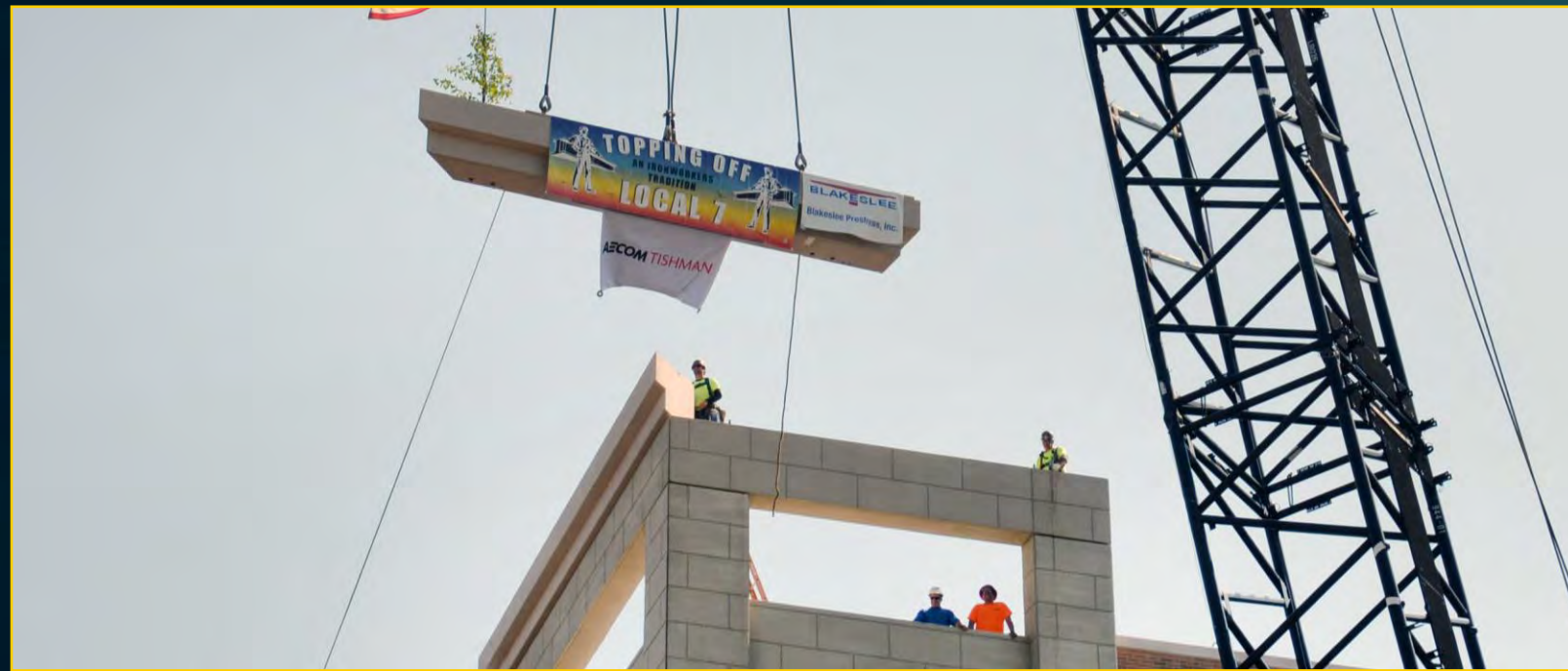
Garage Topping Off - May 17, 2017
