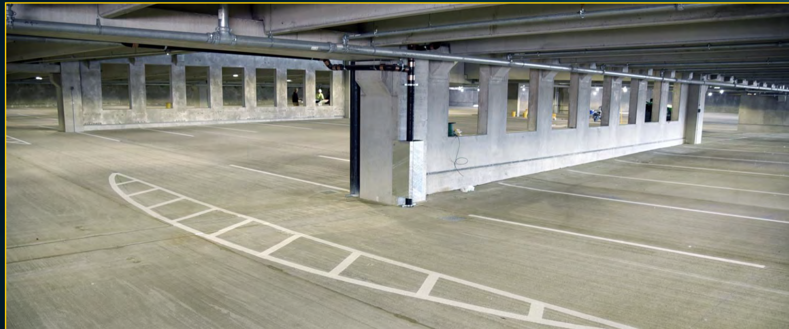
Parking Garage Striping - June 7, 2017
