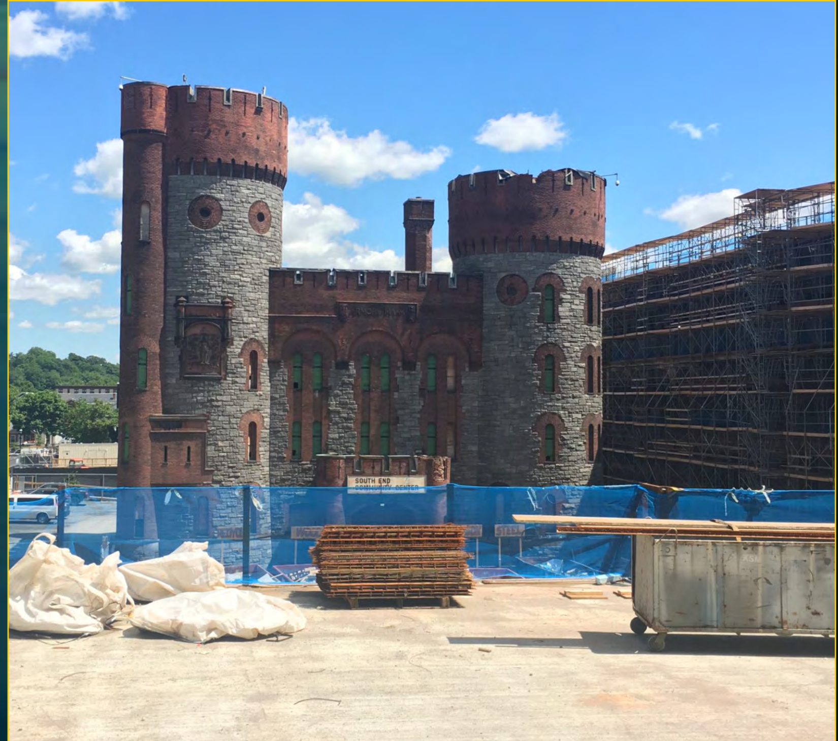
Convention Center Green Roof - June 8, 2017
