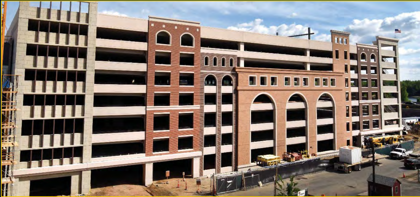
Parking Garage Facade - May 24, 2017
