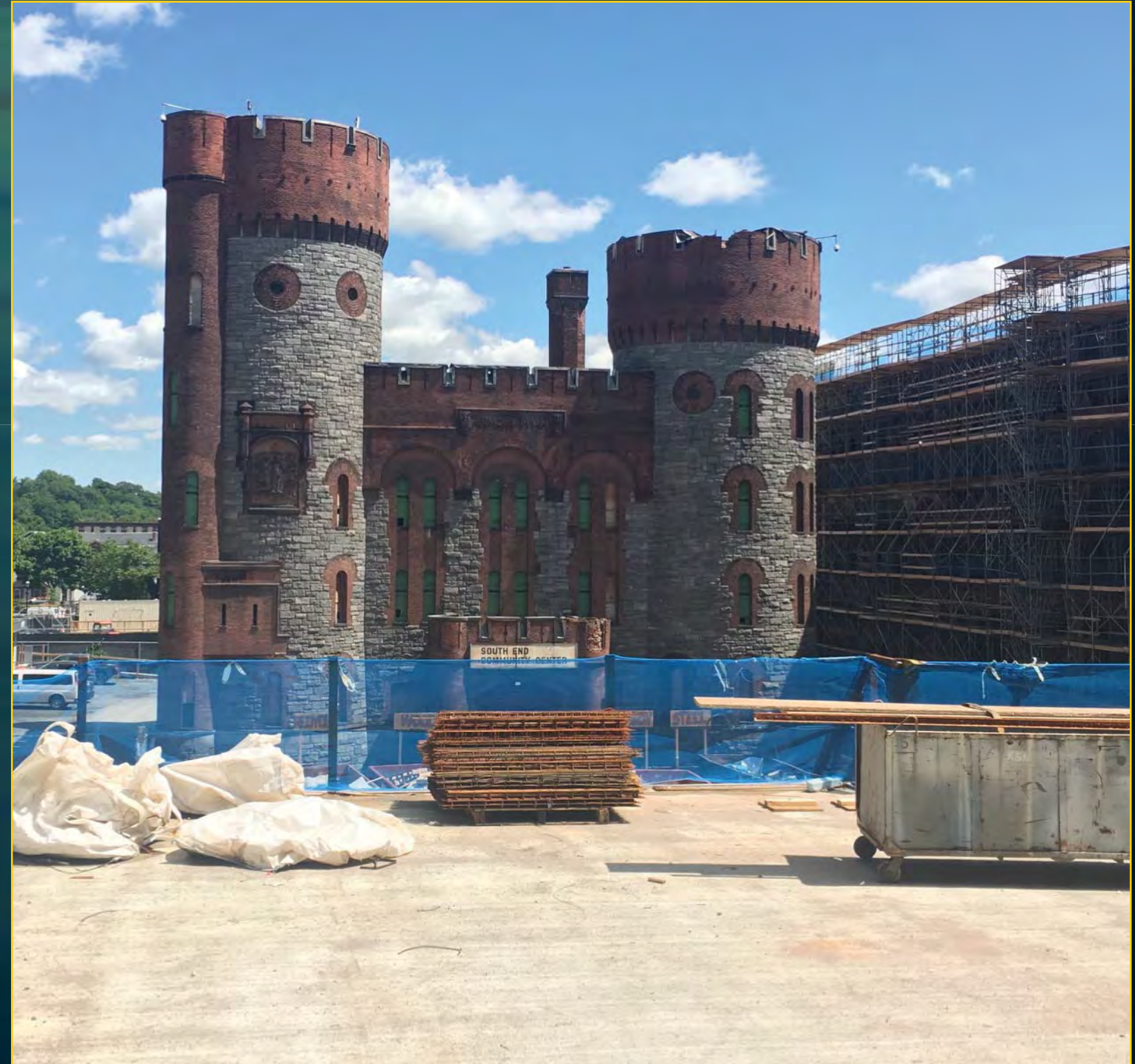
Convention Center Green Roof - June 8, 2017
