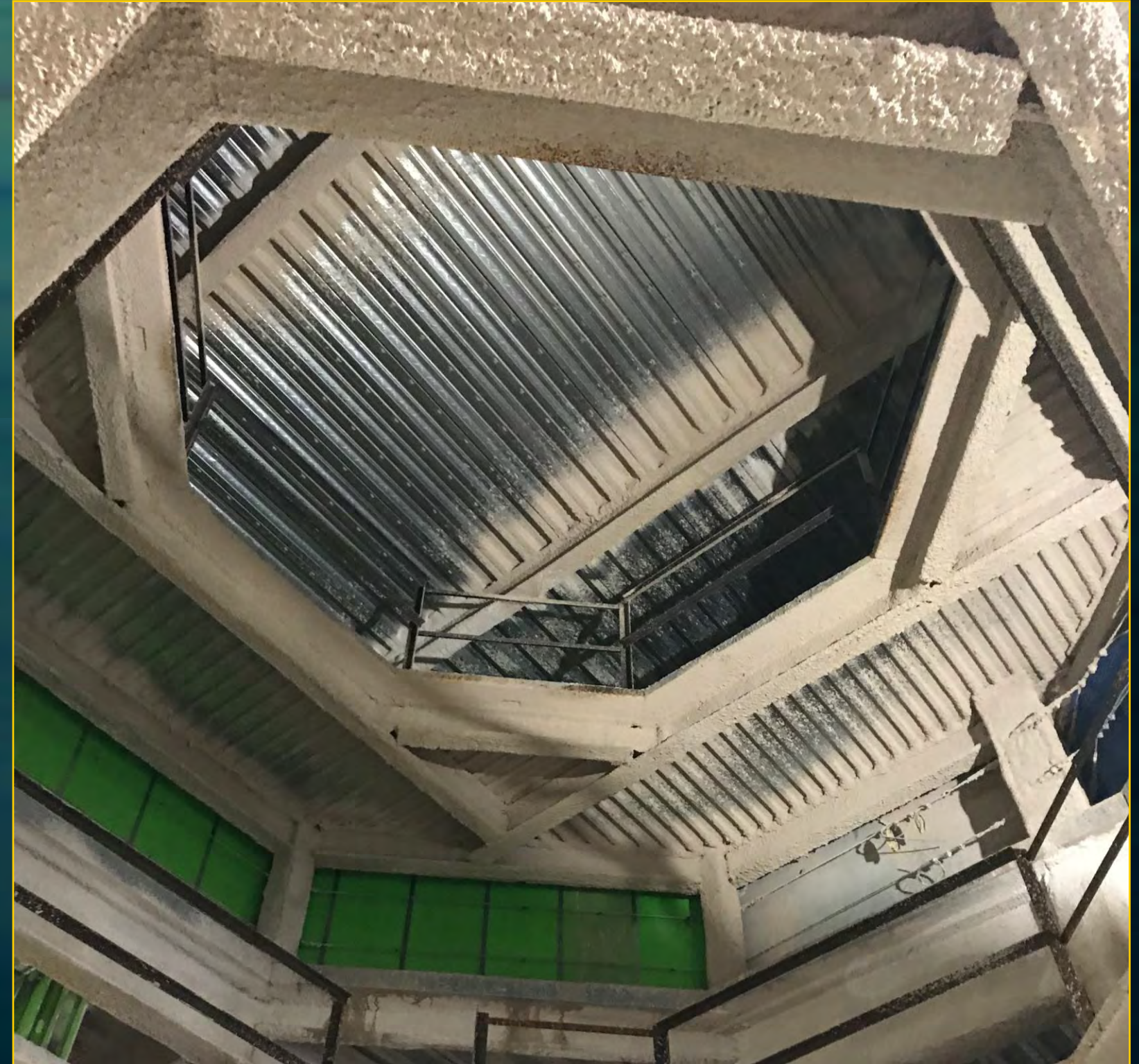
Dome Construction - August 1, 2017
