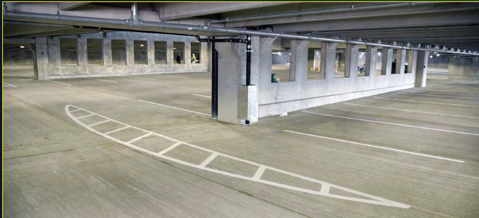
Parking Garage Striping - June 7, 2017
