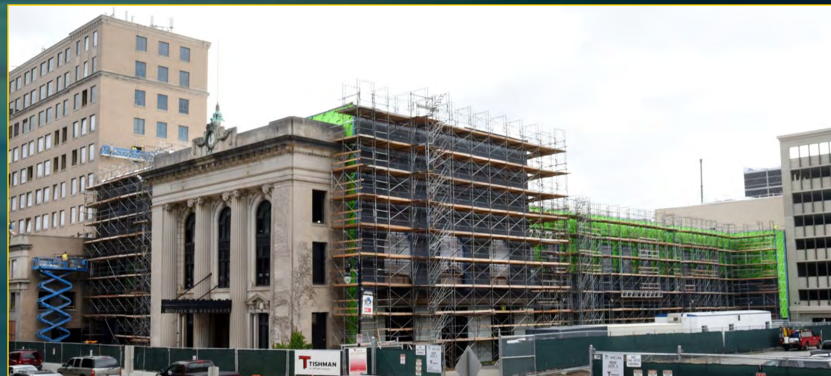
Podium Construction - July 18, 2017
