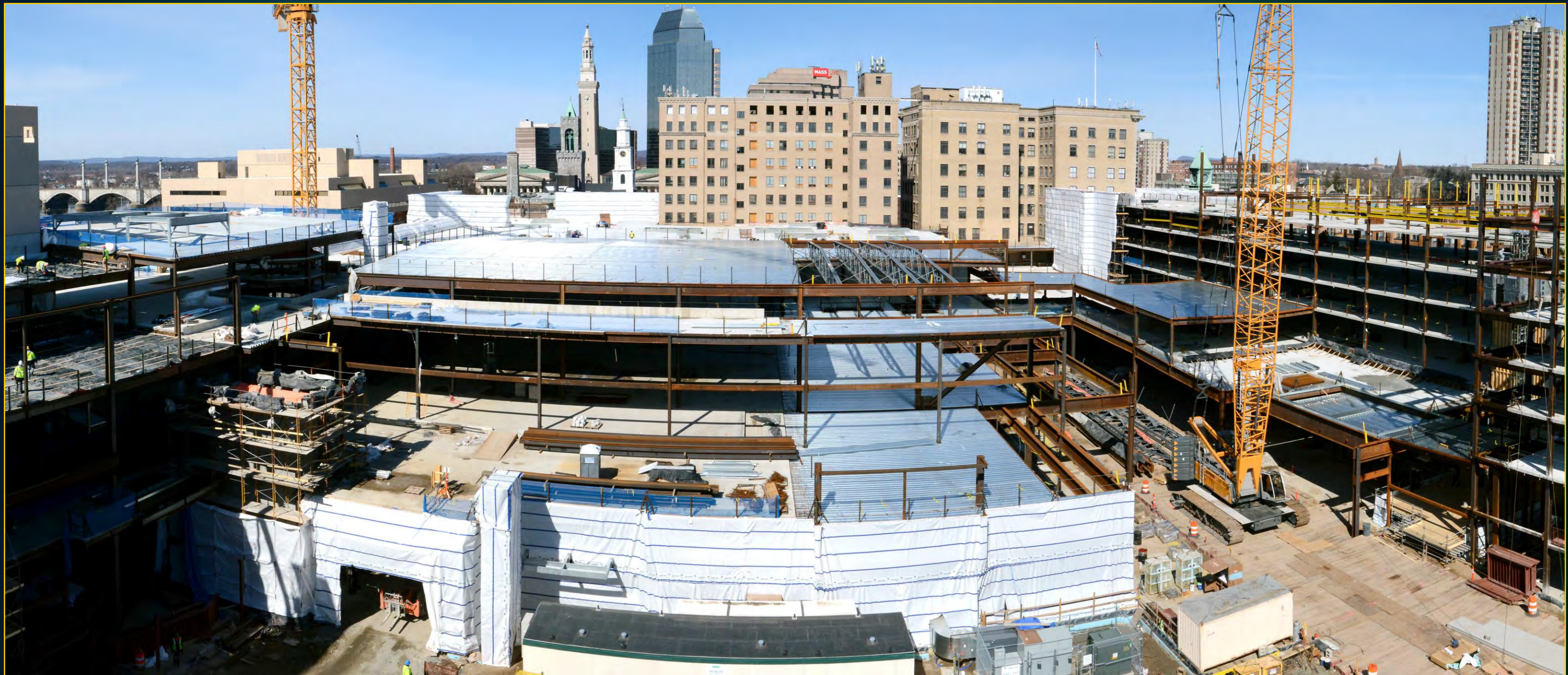
Overall Site Activity from Armory - March 13, 2017
