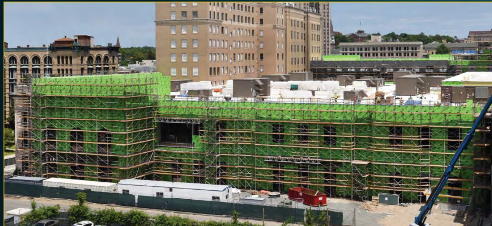
Podium Construction - June 15, 2017
