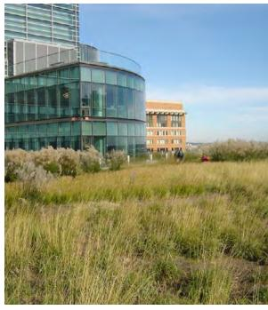
A GREEN ROOF, REDUCES STORM WATER RUNOFF AND THE HEAT ISLAND EFFECT
