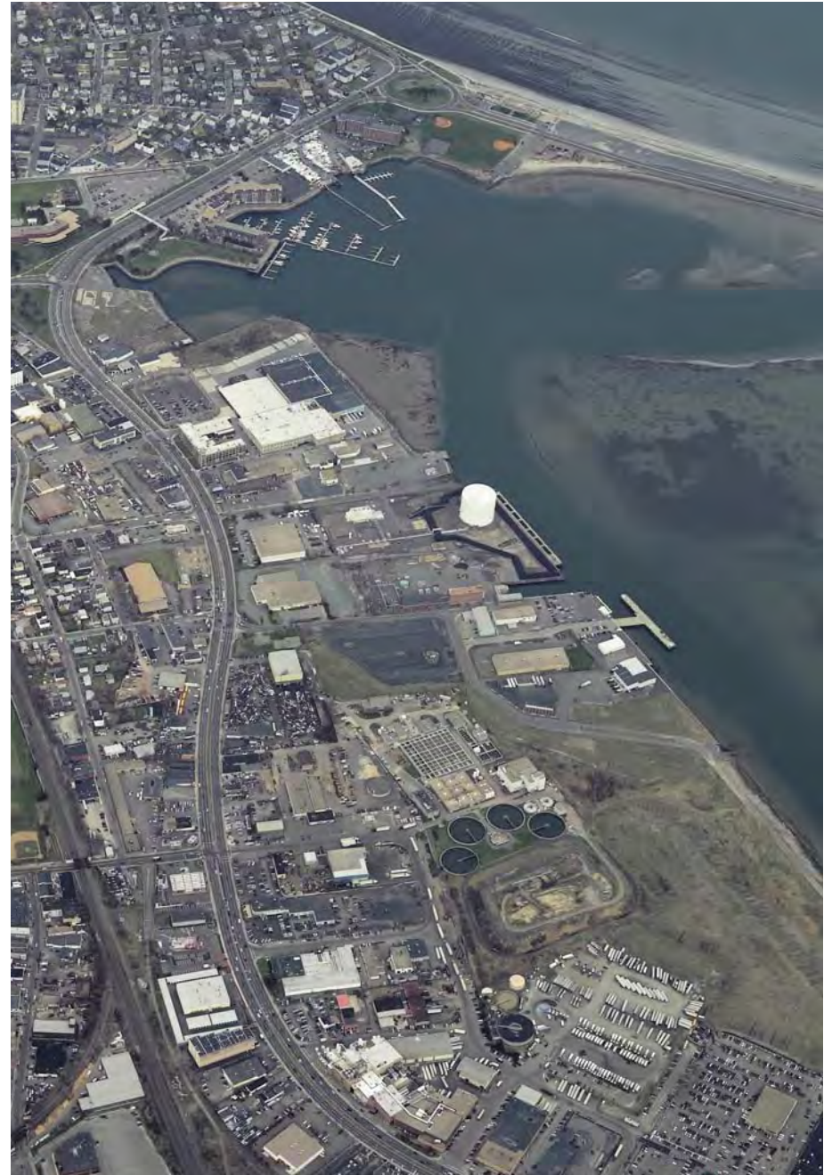
AN AERIAL VIEW OF THE 250+ ACRE WATERFRONT SITE
