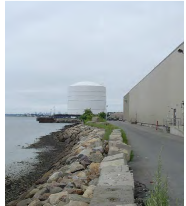
THE LNG TANK AND A DISTRIBUTION FACILITY ARE WINDOWLESS STRUCTURES FEET FROM THE WATER
