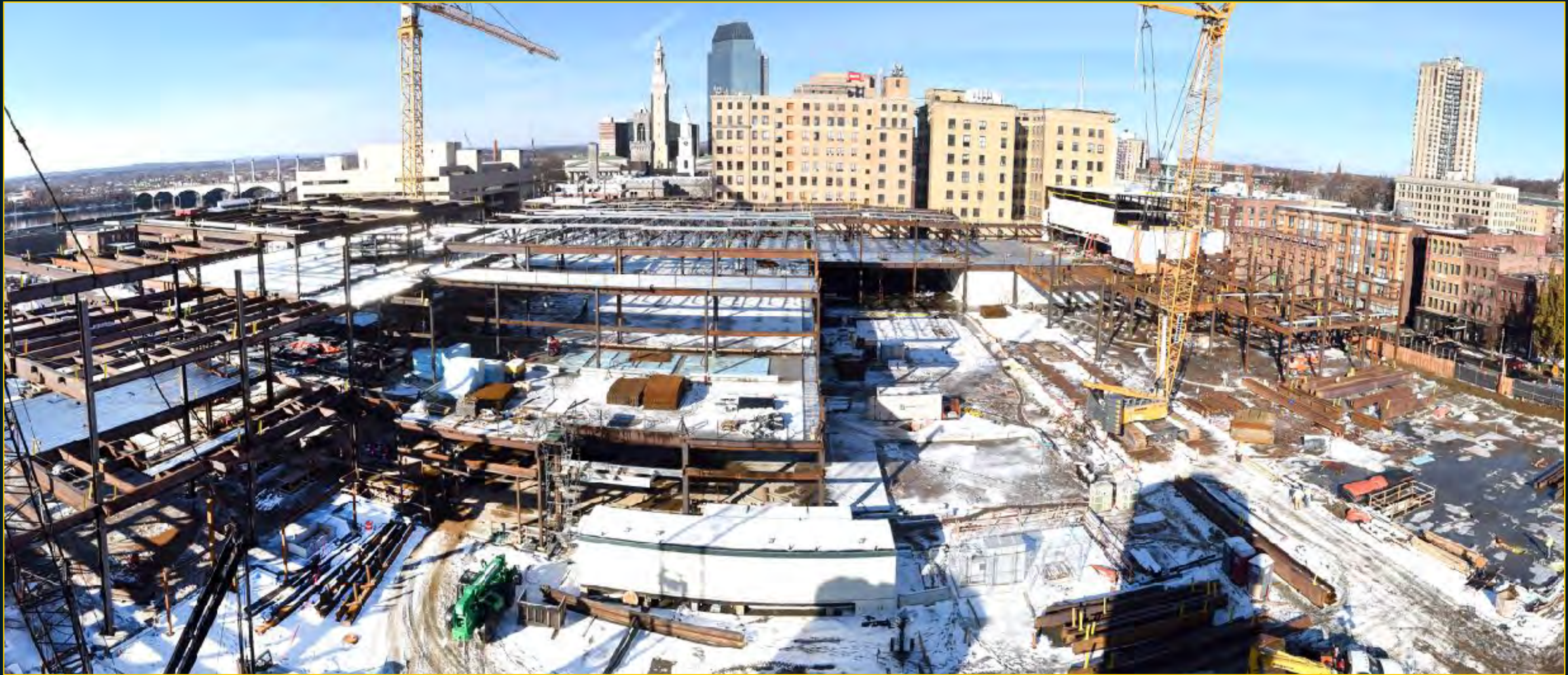
Overall Site Activity from Armory - December 13, 2016
