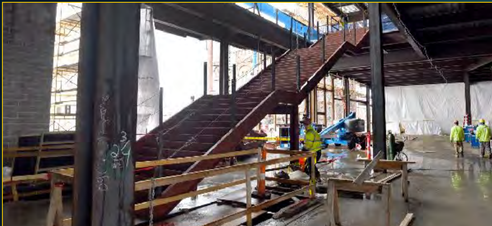
Podium Construction - March 8, 2017
