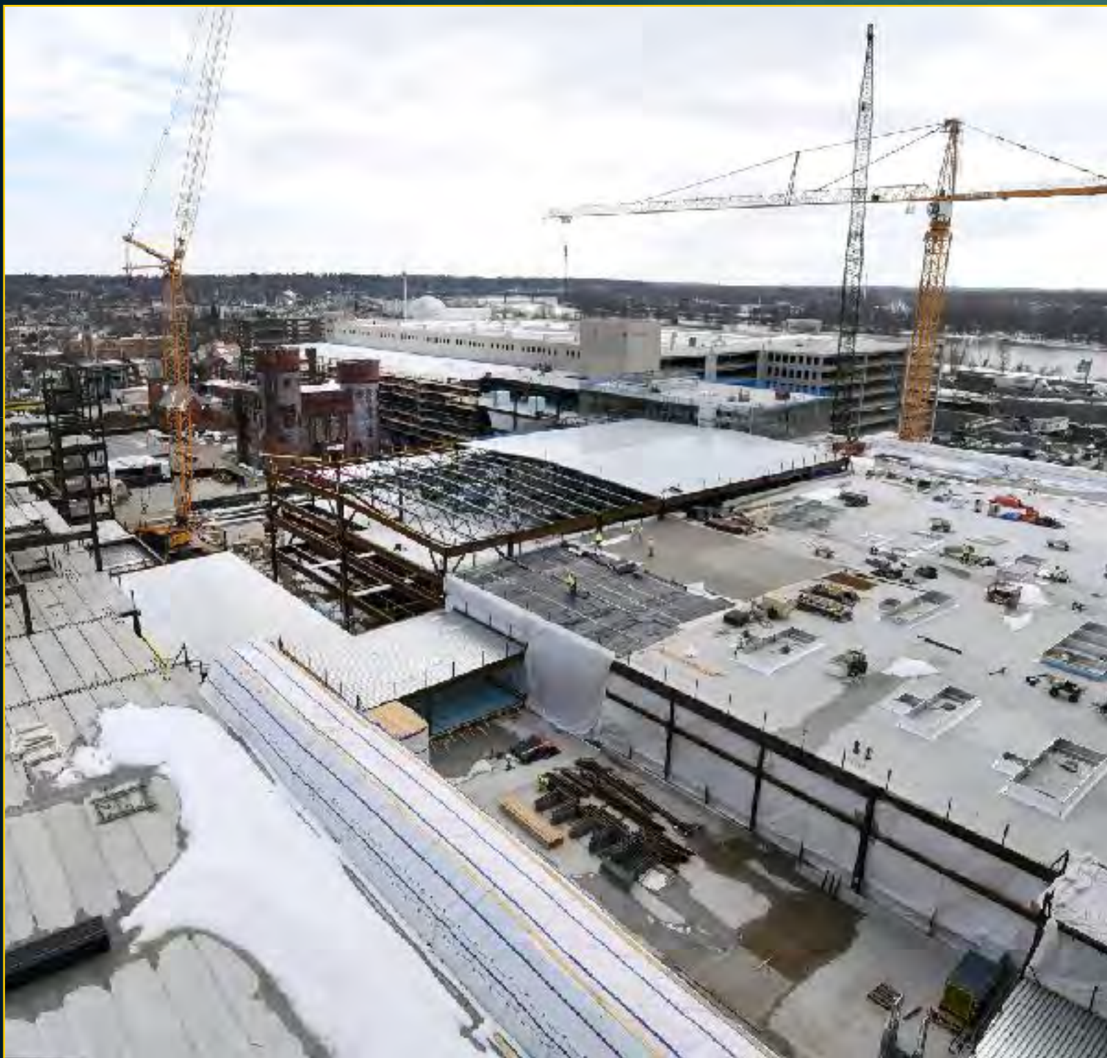
Podium Enclosure - March 21, 2017
