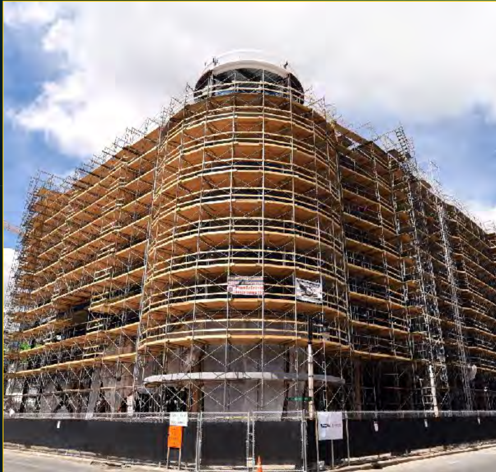
Hotel Construction - May 11, 2017
