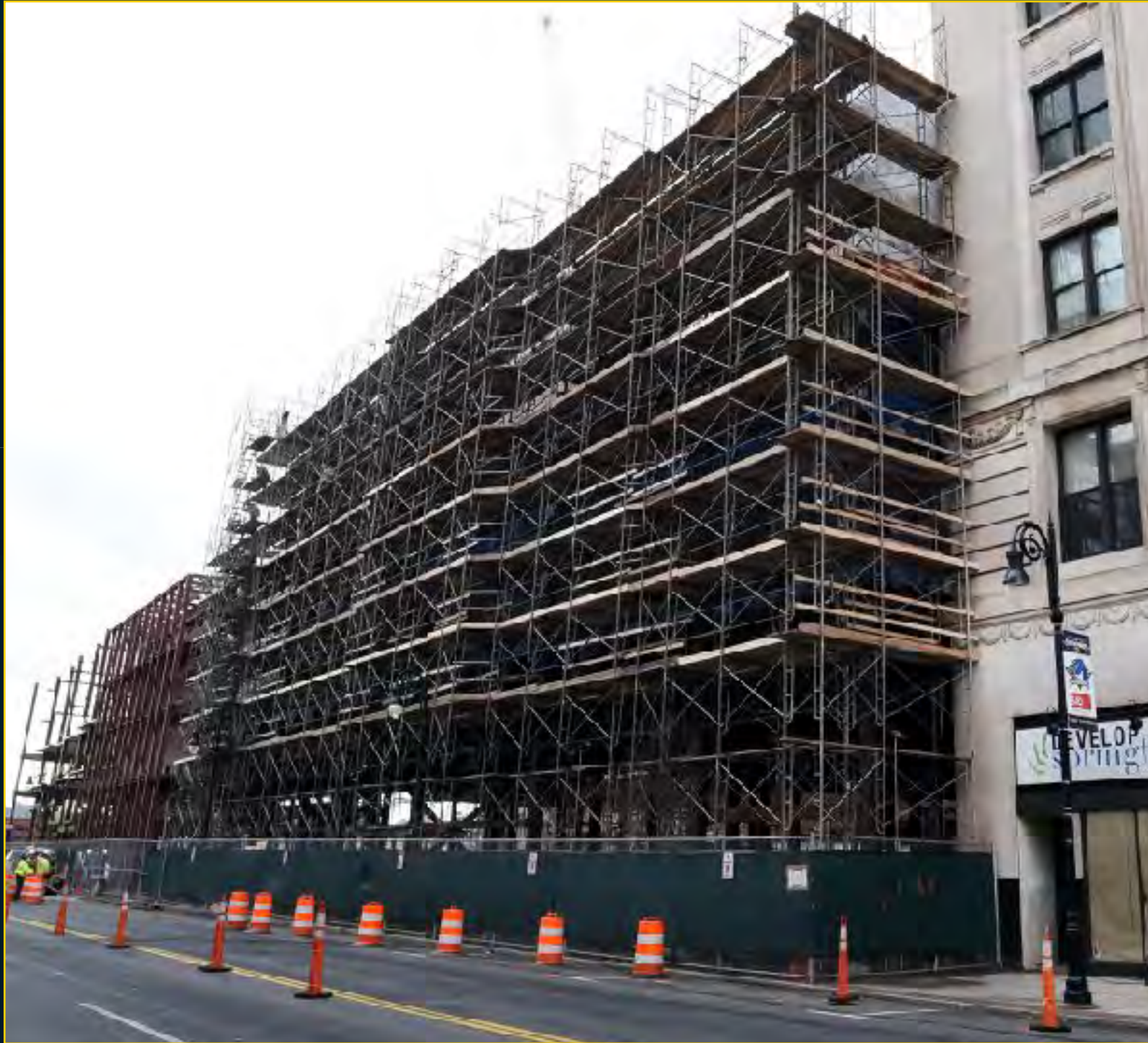
Main Street Scaffolding - January 19, 2017
