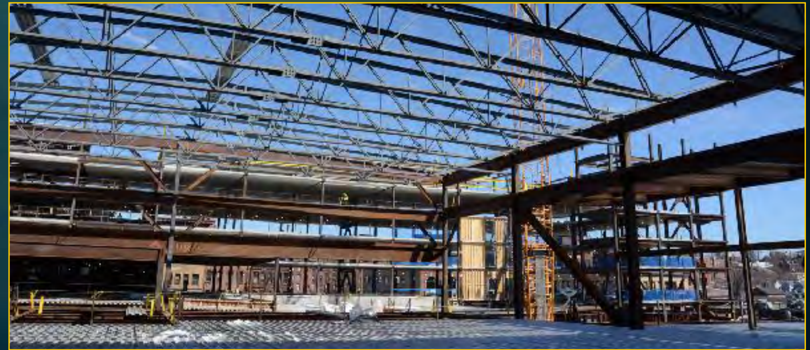
Podium Steel - March 28, 2017
