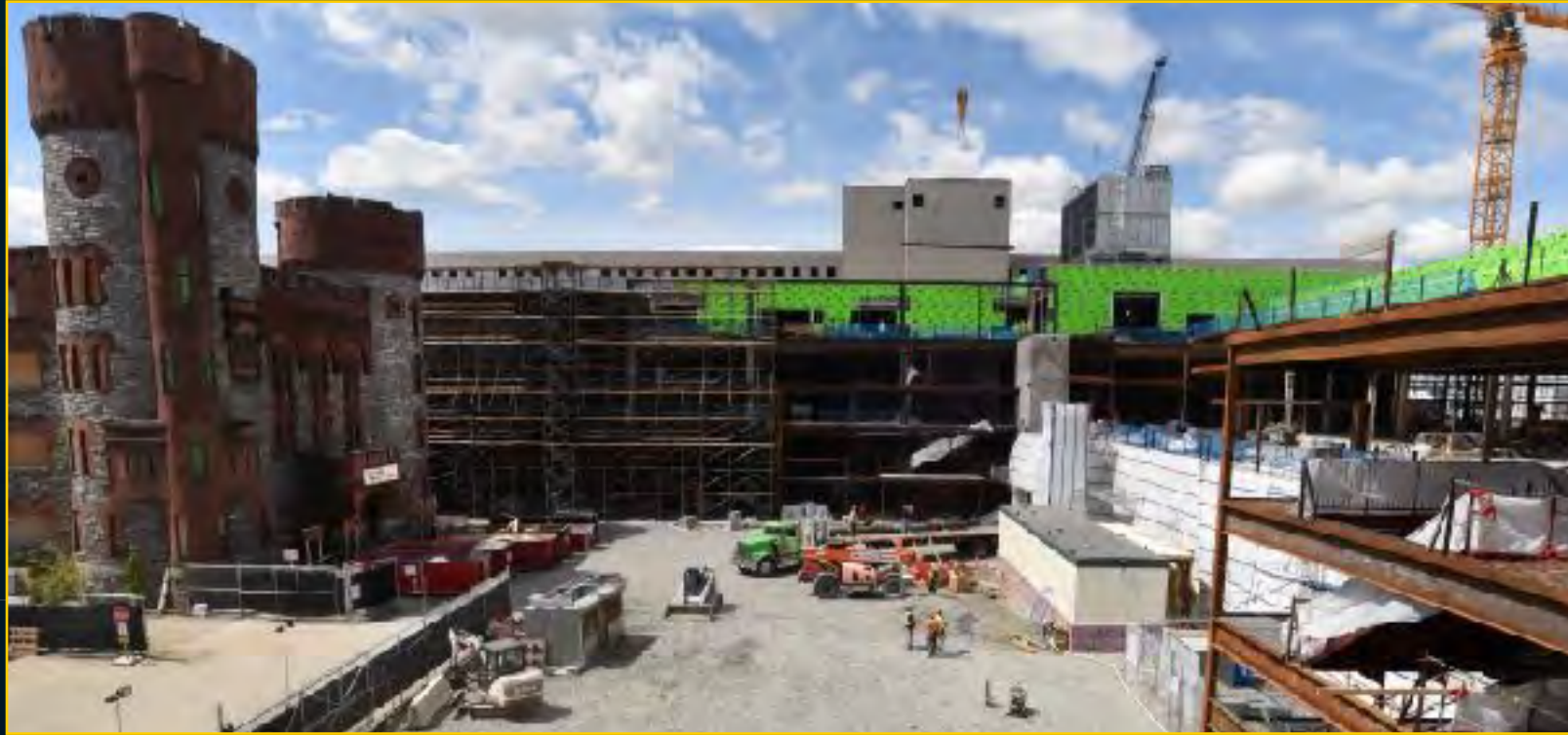
Podium Construction - May 12, 2017
