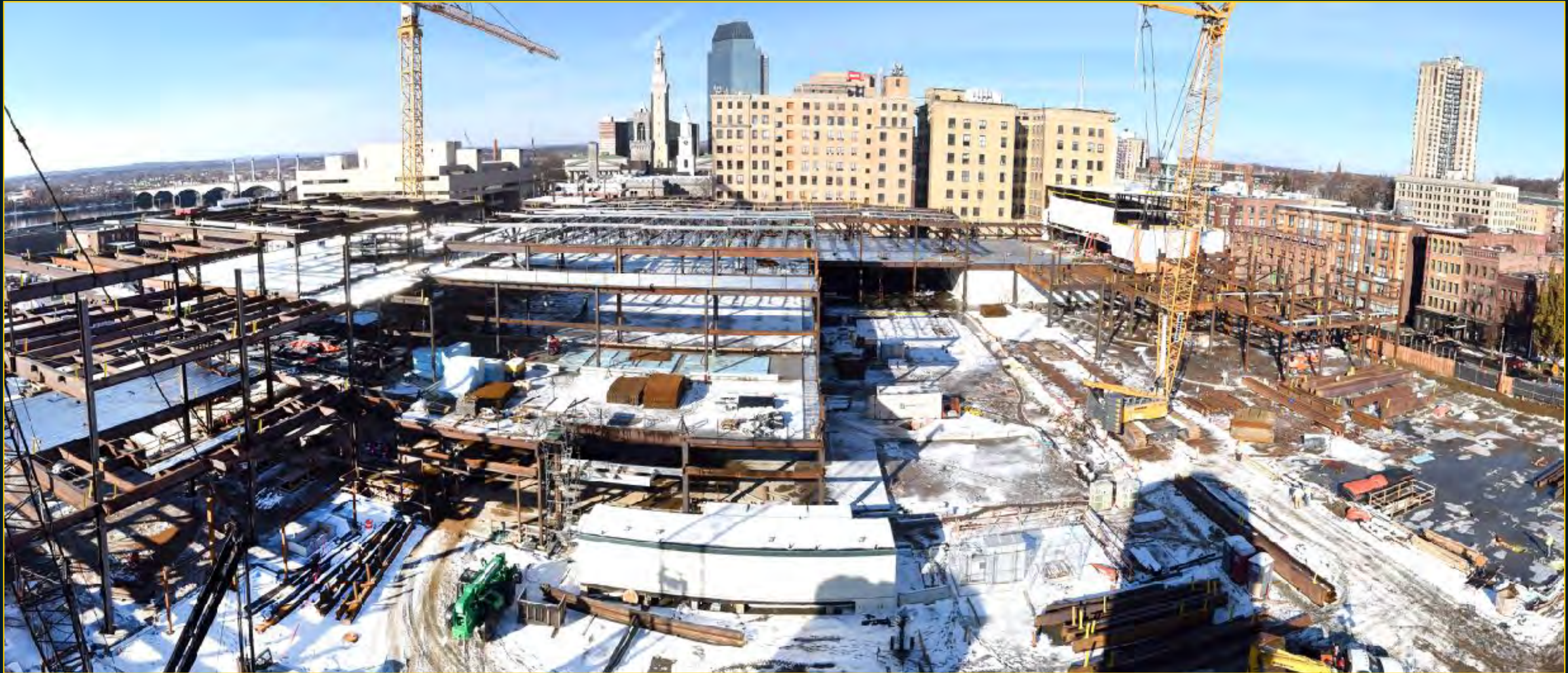
Overall Site Activity from Armory - December 13, 2016
