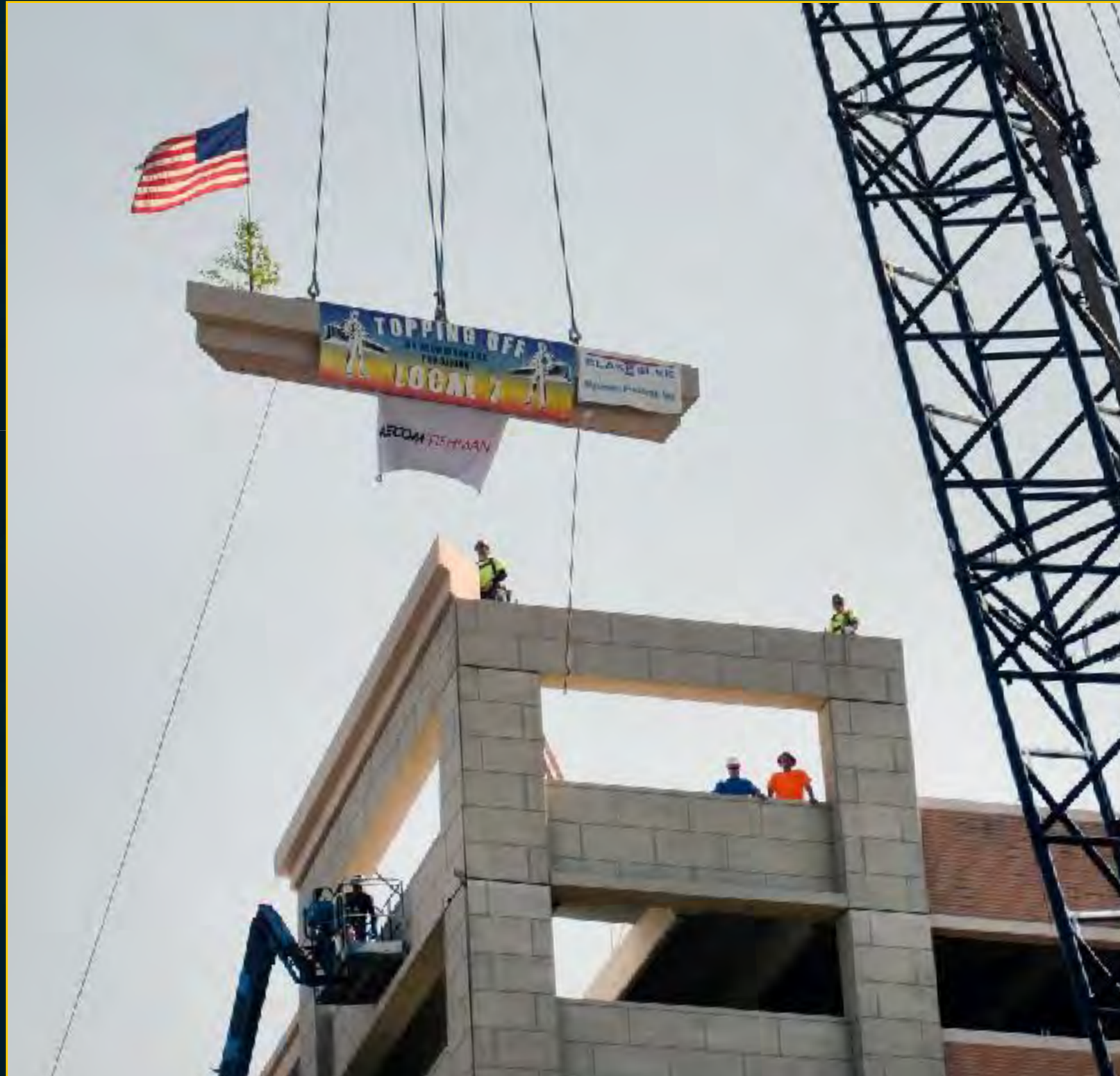
Garage Topping Off - May 17, 2017
