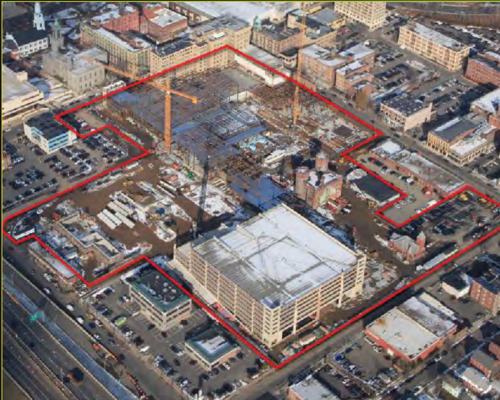
Aerial View - December 14, 2016
