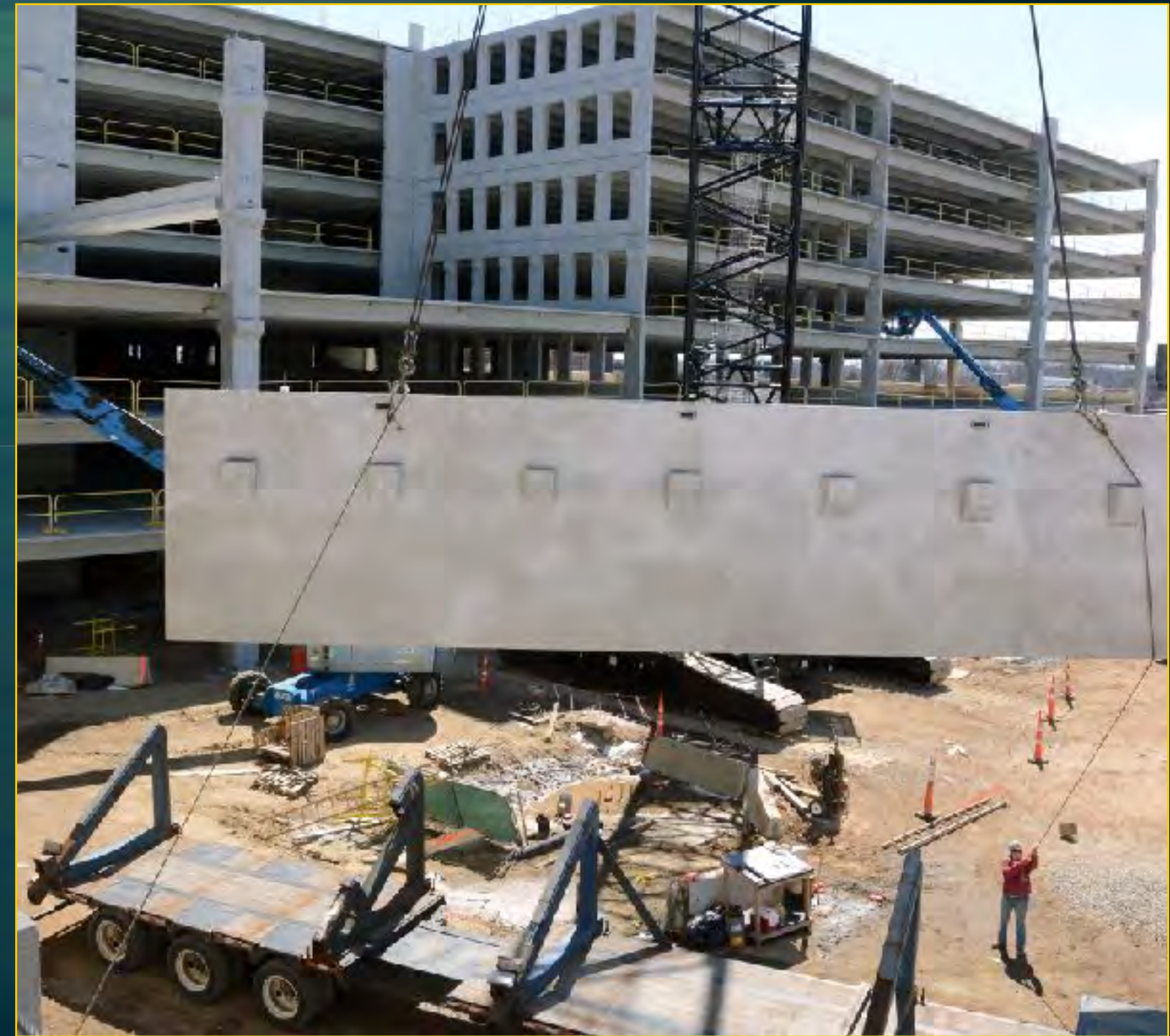
Garage Construction - March 28, 2017
