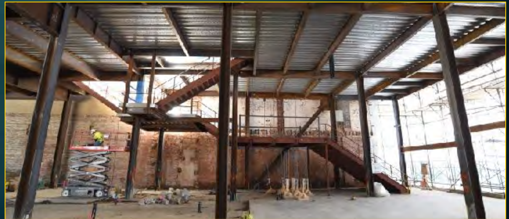
Hotel Construction - February 7, 2017
