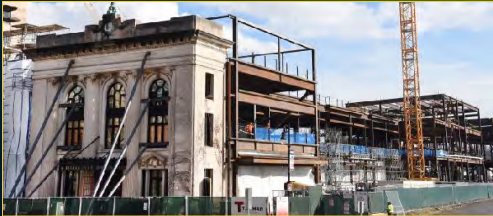
73 State Construction - January 26, 2017
