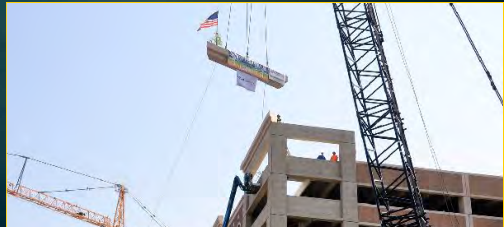
Garage Topping Off - May 17, 2017
