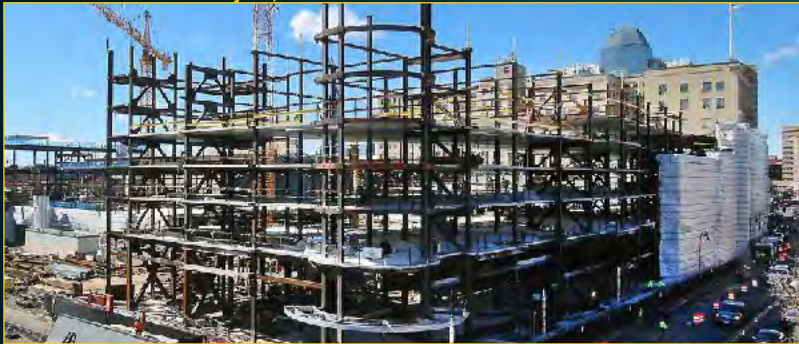
Hotel Entrance - March 8, 2017
