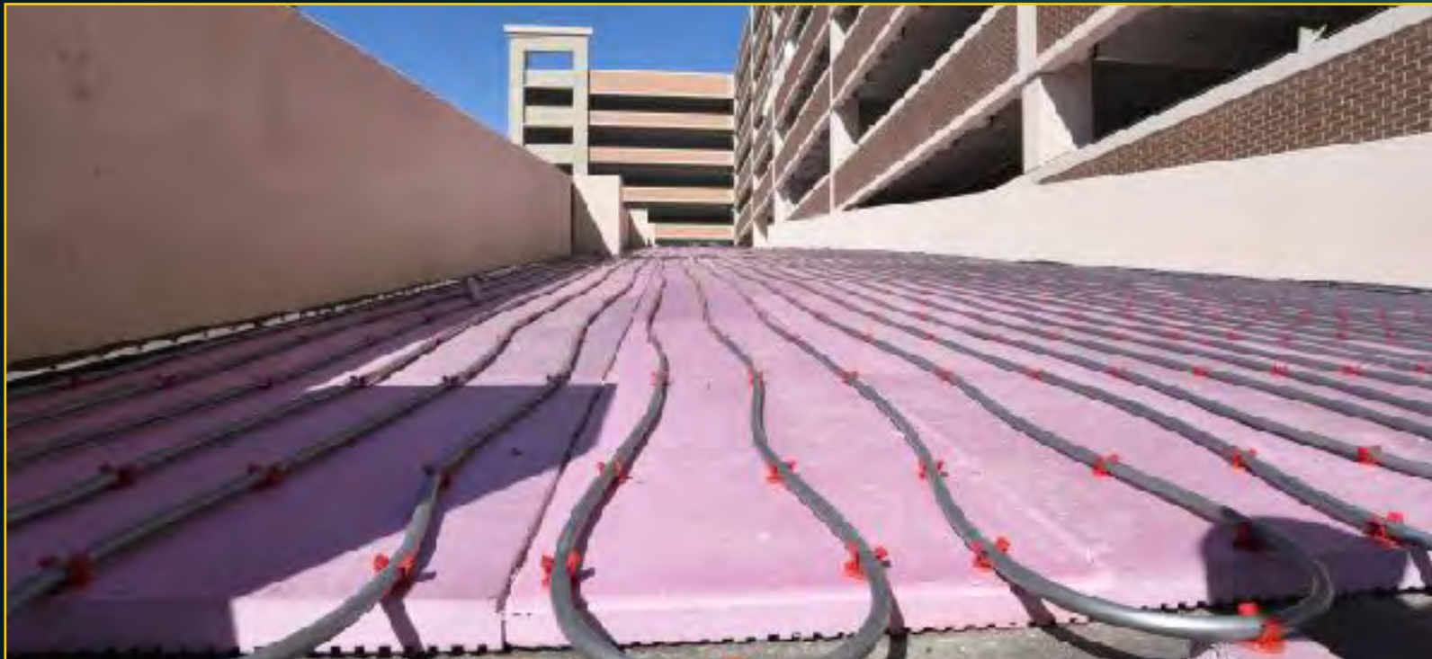
Garage Construction - March 3, 2017
