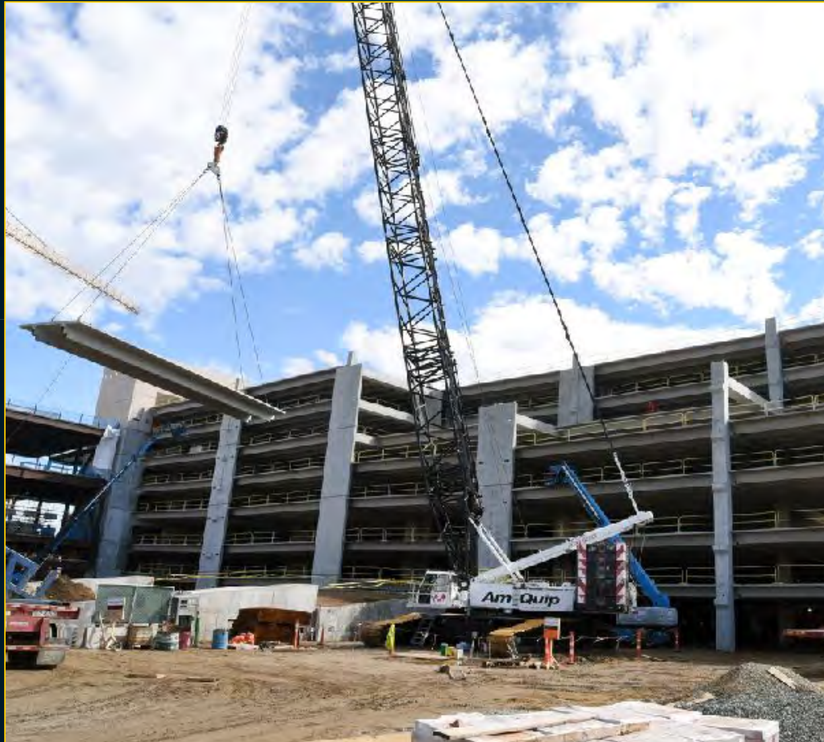
Garage Construction - March 8, 2017
