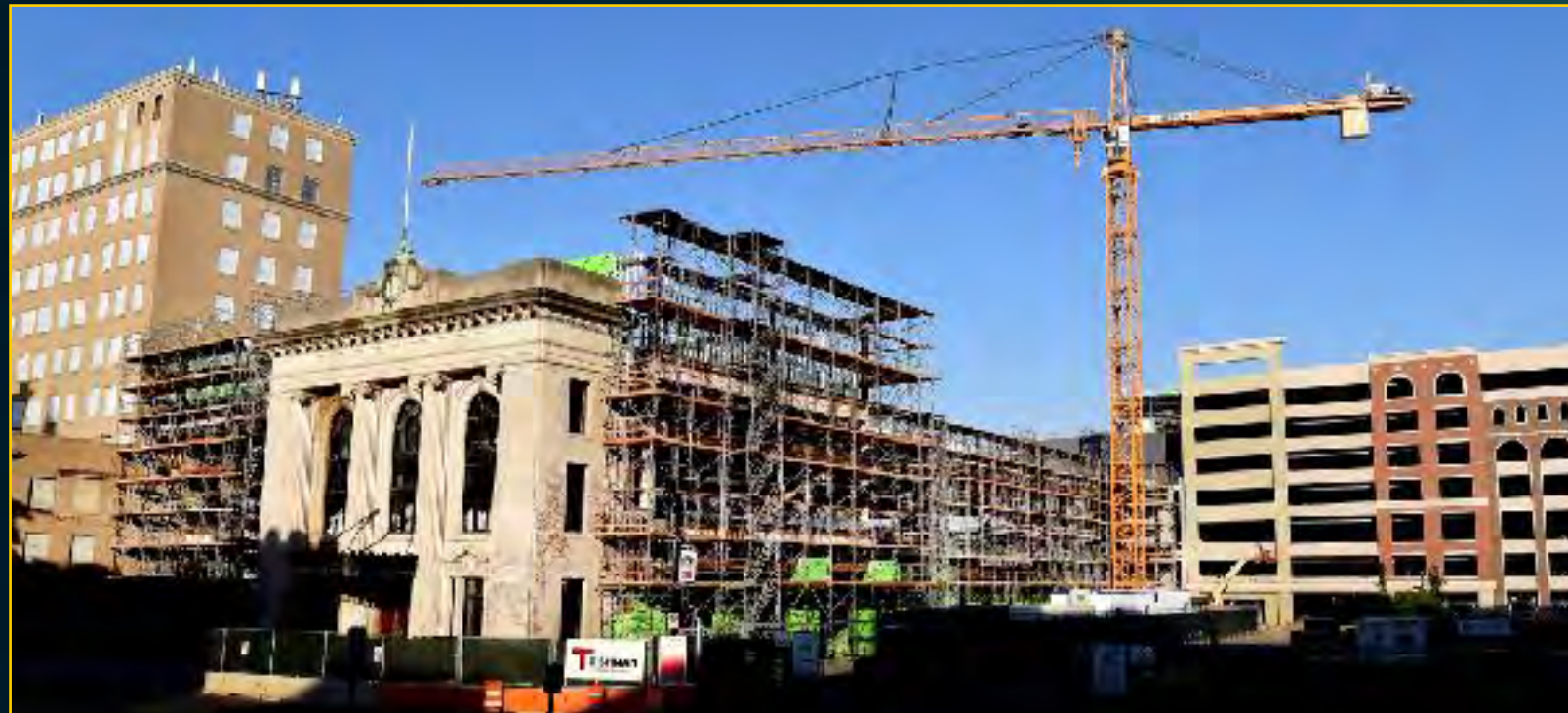
Podium Construction - May 19, 2017
