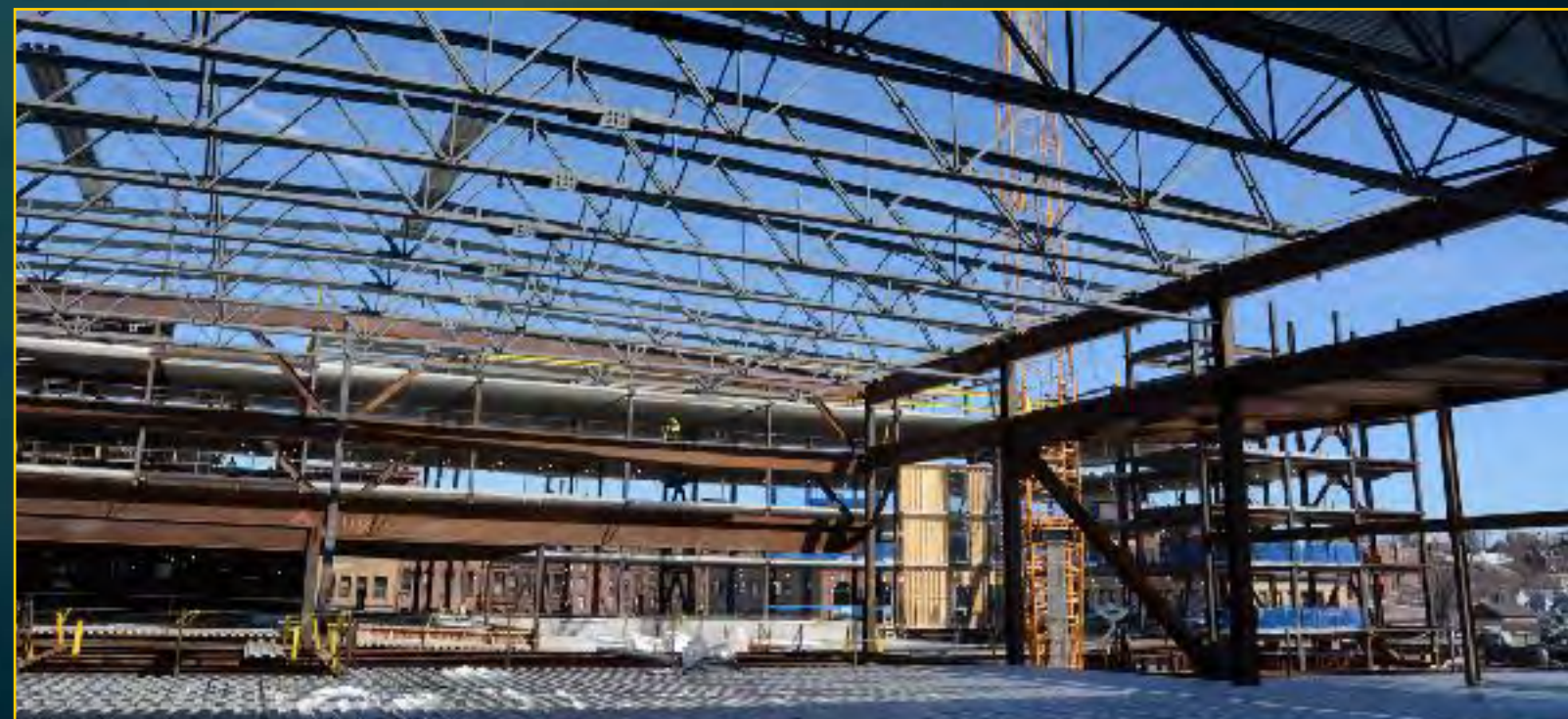
Podium Steel - March 28, 2017
