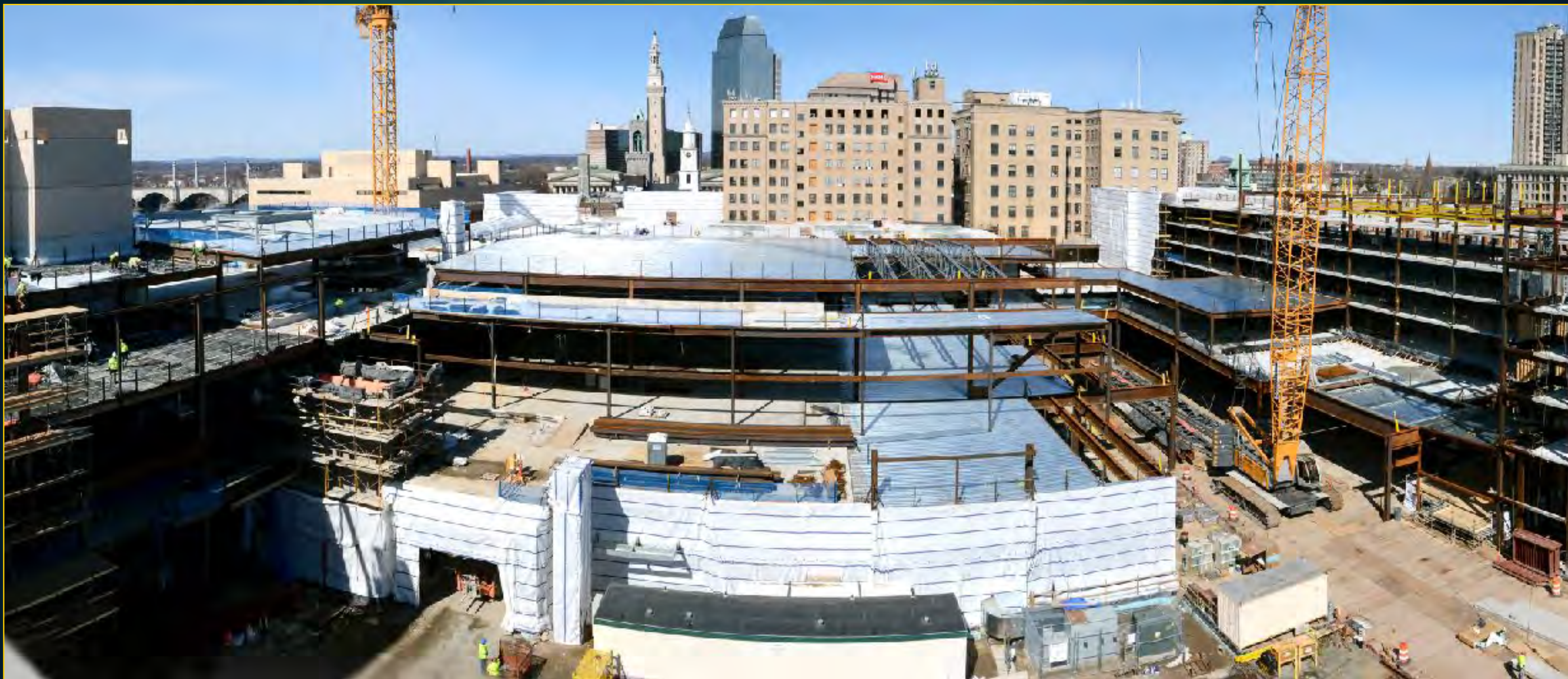
Overall Site Activity from Armory - March 13, 2017
