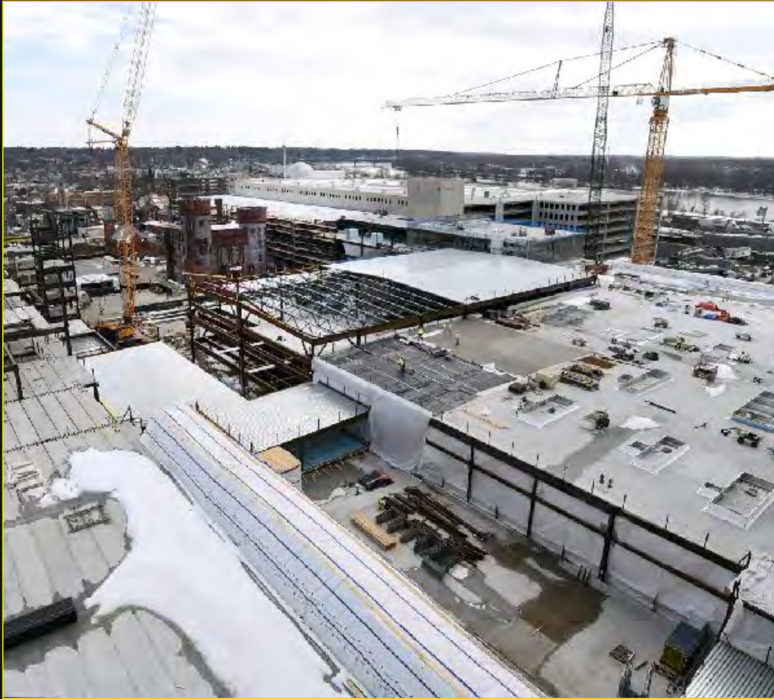
Podium Enclosure - March 21, 2017
