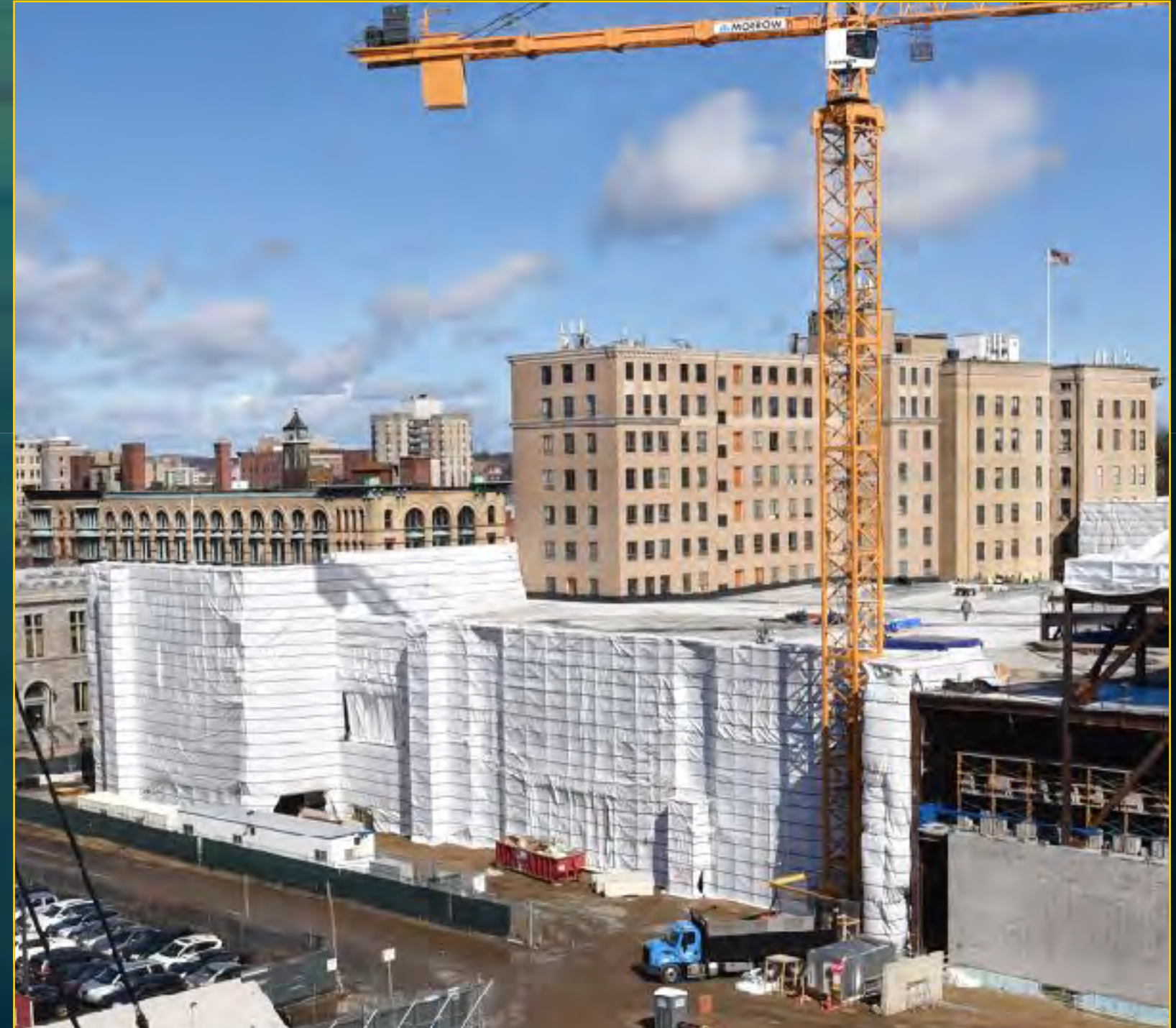
Podium Enclosure - March 8, 2017
