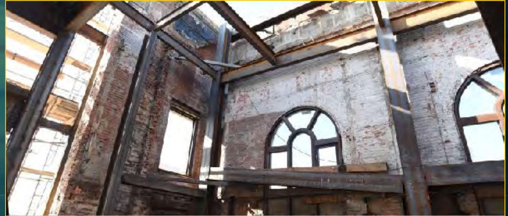
Hotel Construction - February 8, 2017
