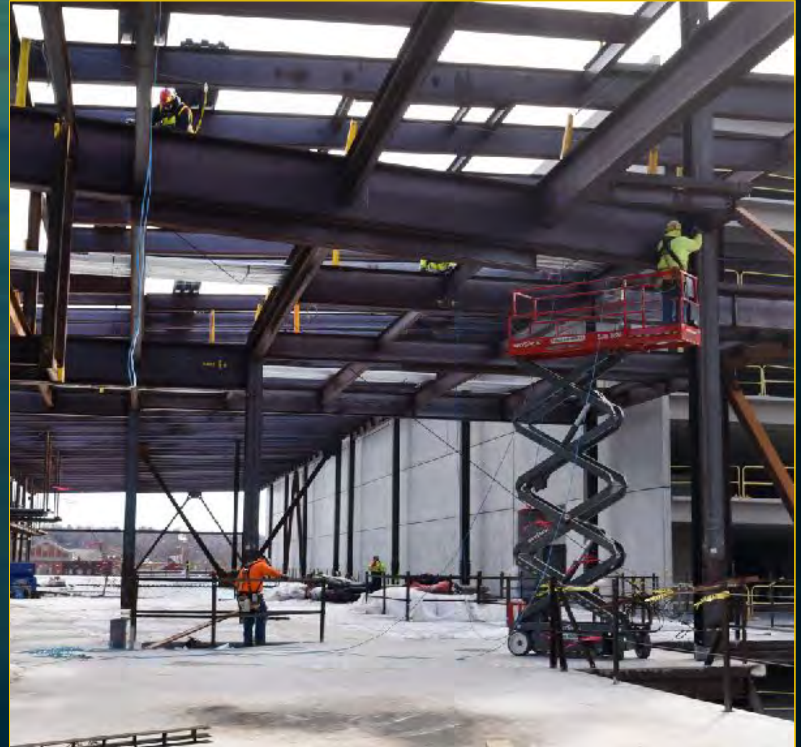
Entertainment Steel Erection - February 6, 2017
