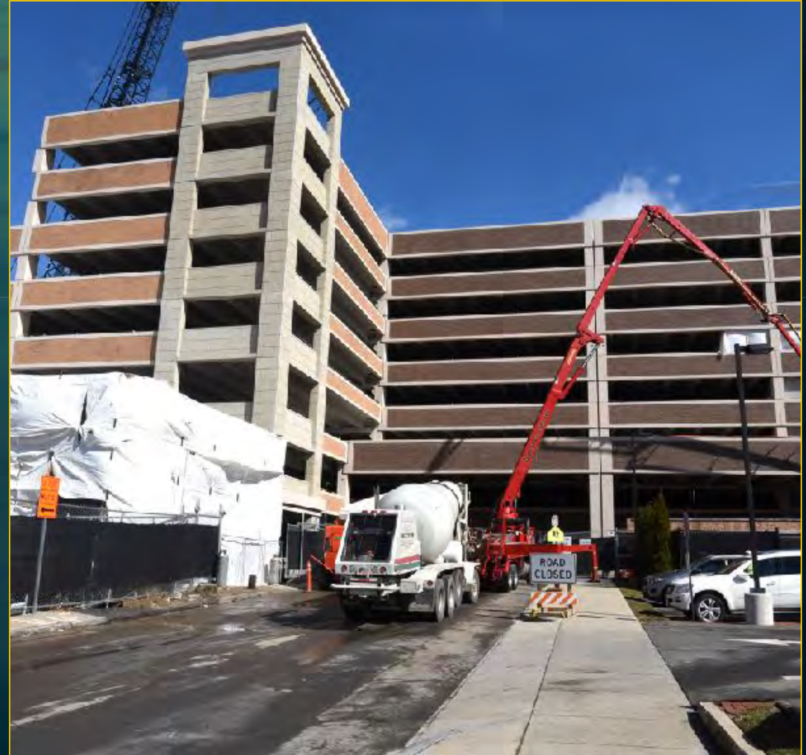
Garage Construction - March 8, 2017
