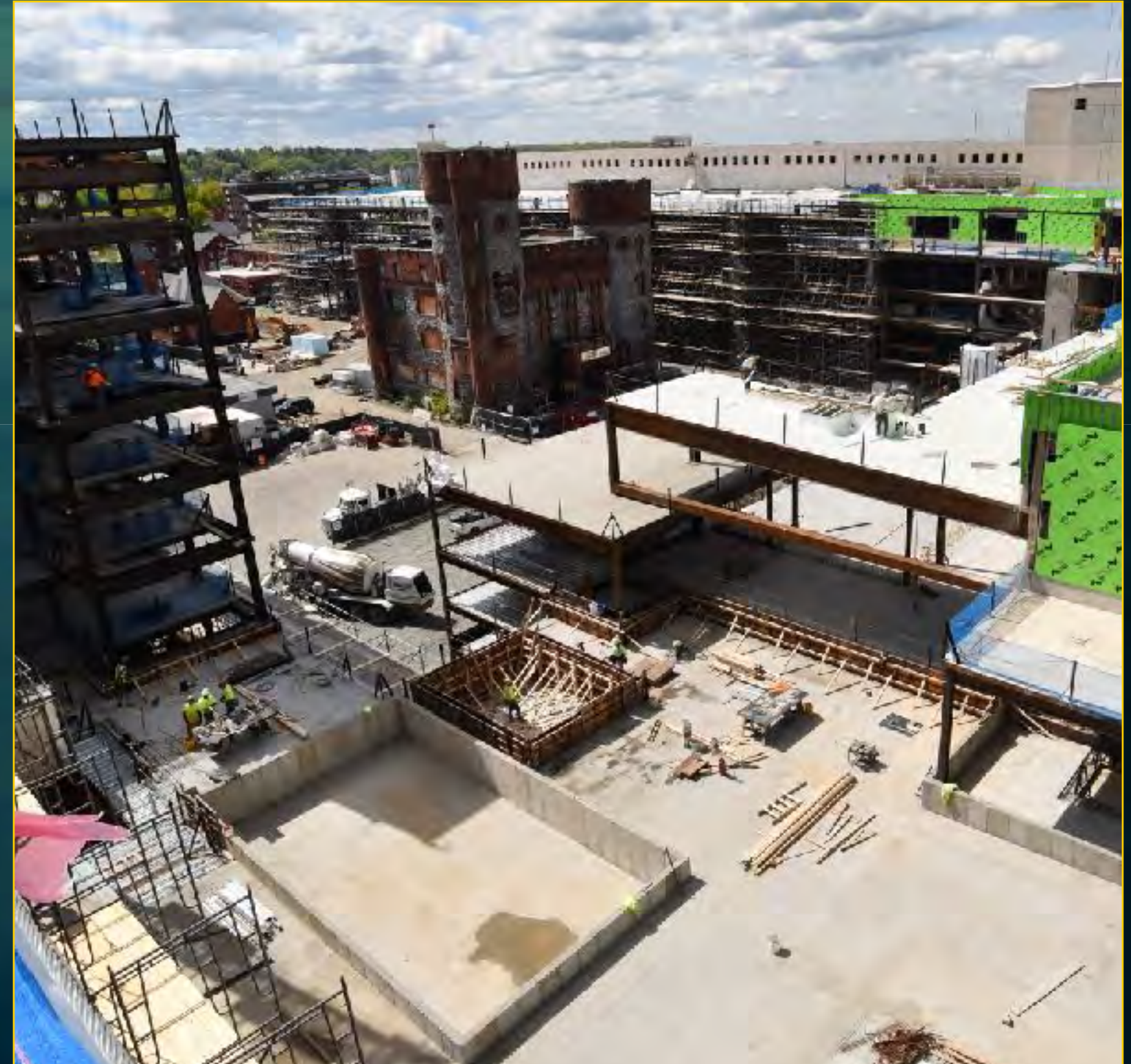
Hotel Construction - May 12, 2017
