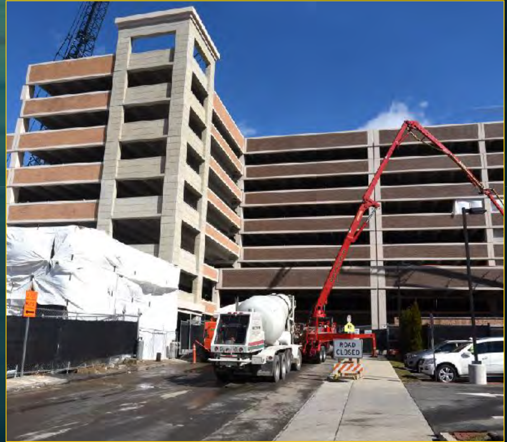
Garage Construction - March 8, 2017
