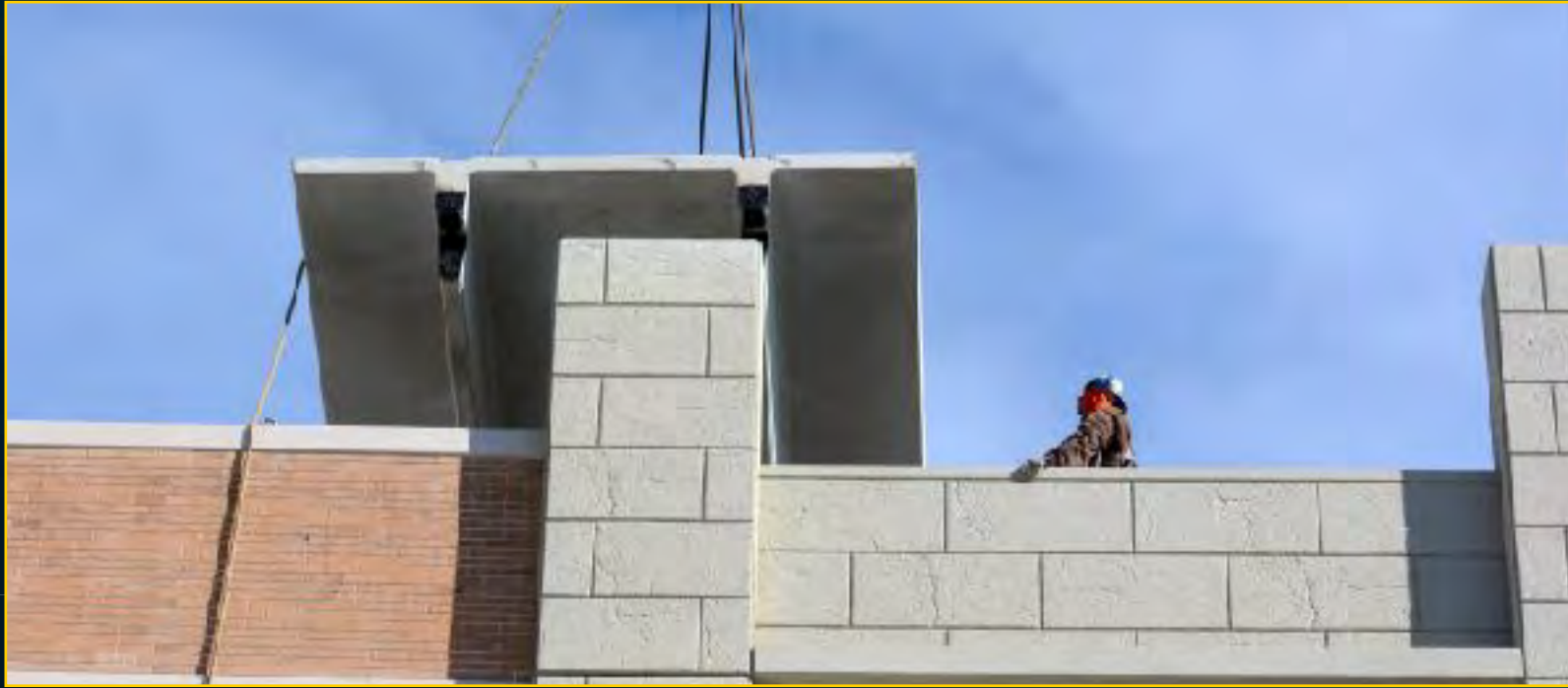
Garage Construction - February 6, 2017
