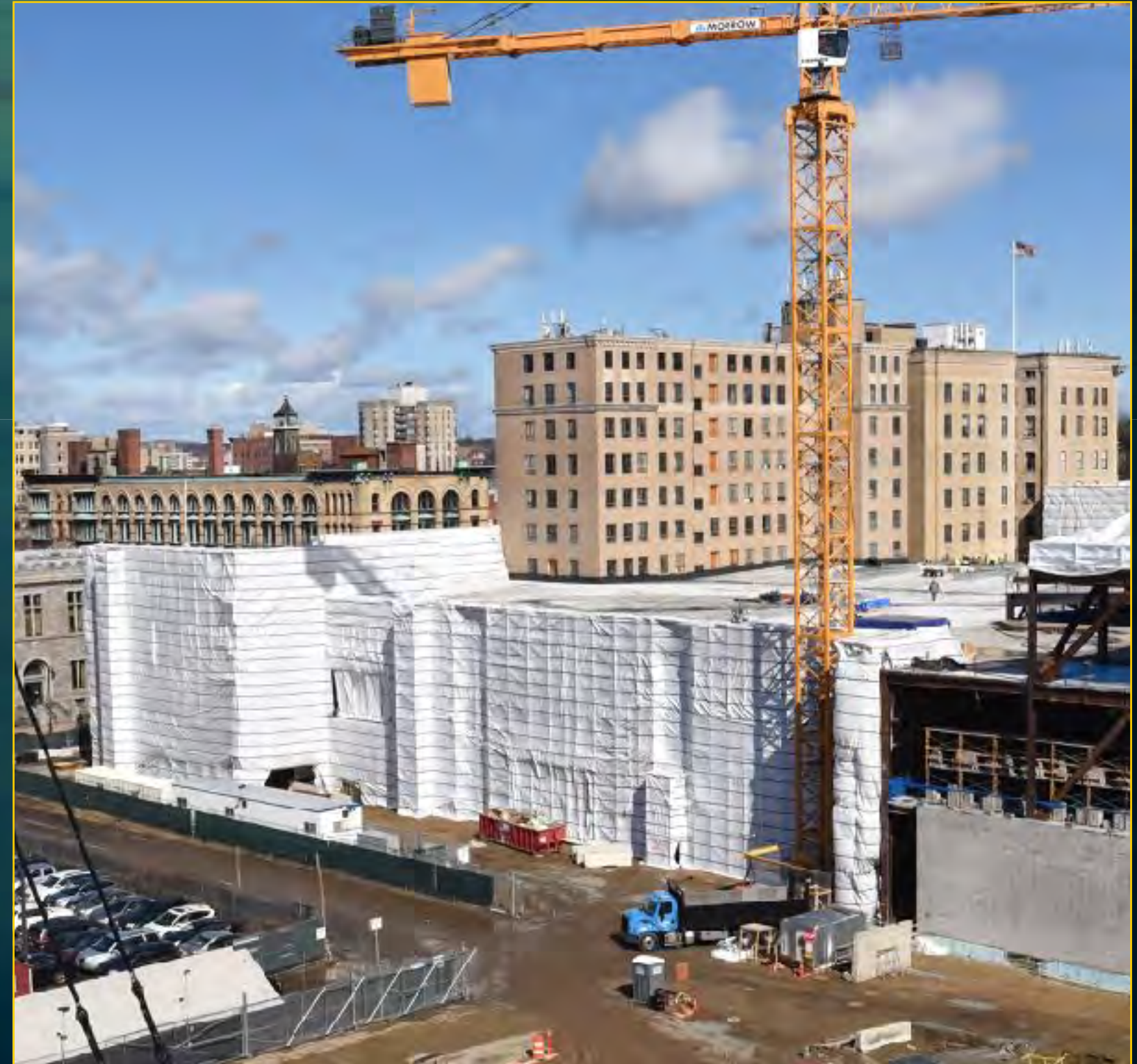
Podium Enclosure - March 8, 2017
