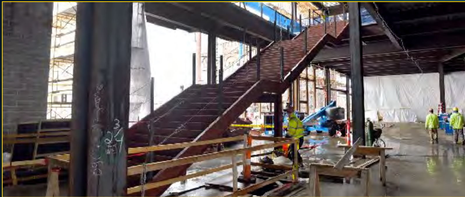
Podium Construction - March 8, 2017
