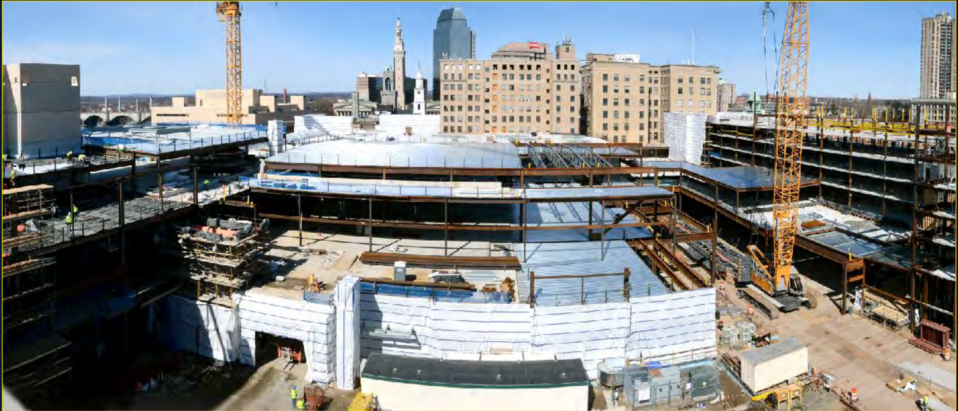
Overall Site Activity from Armory - March 13, 2017
