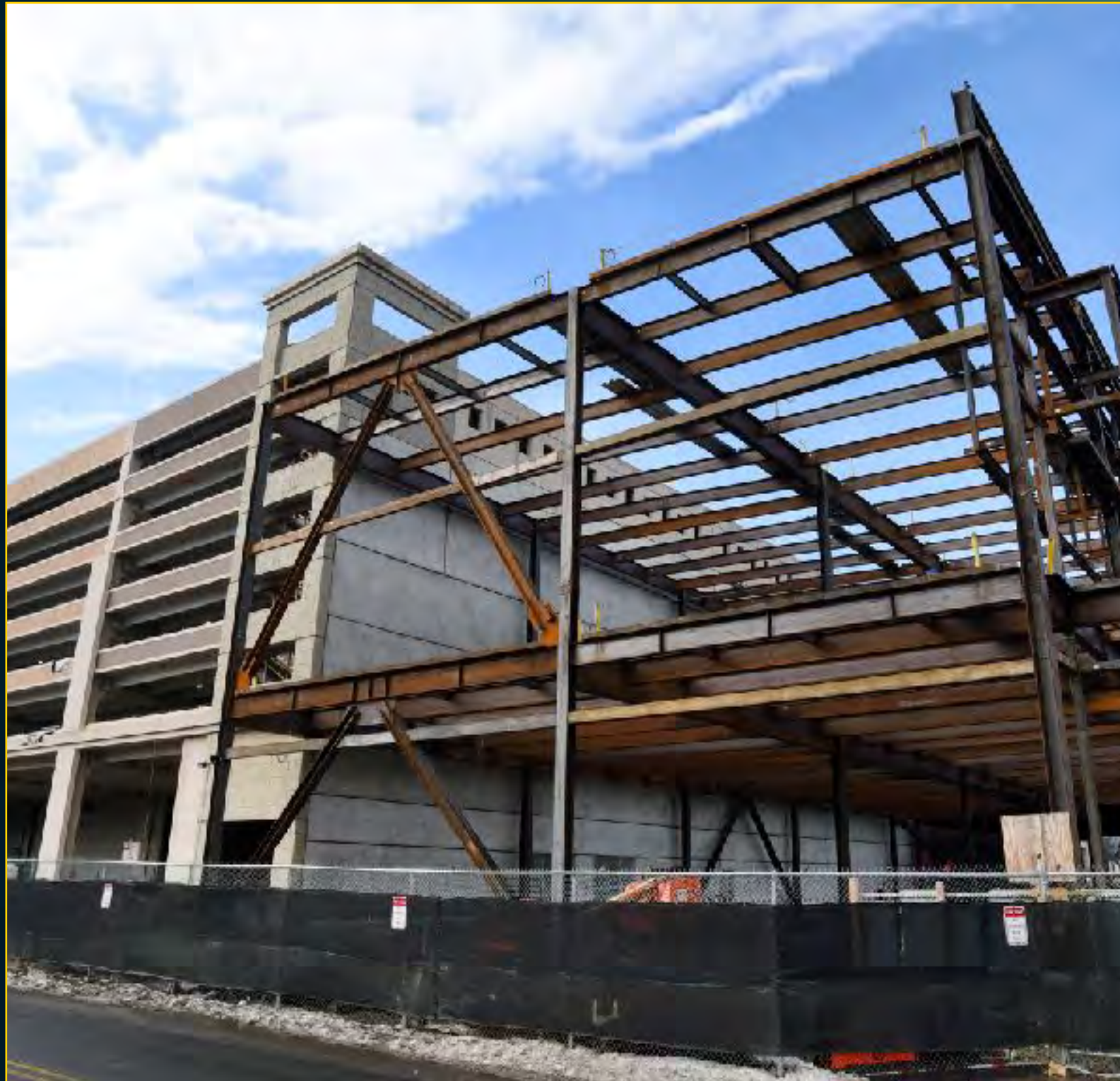
Entertainment Steel Erection - January 26, 2017
