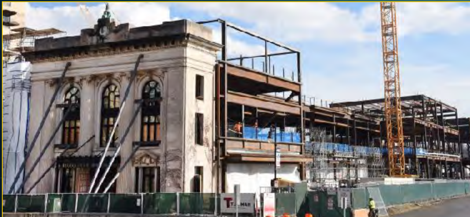
73 State Construction - January 26, 2017
