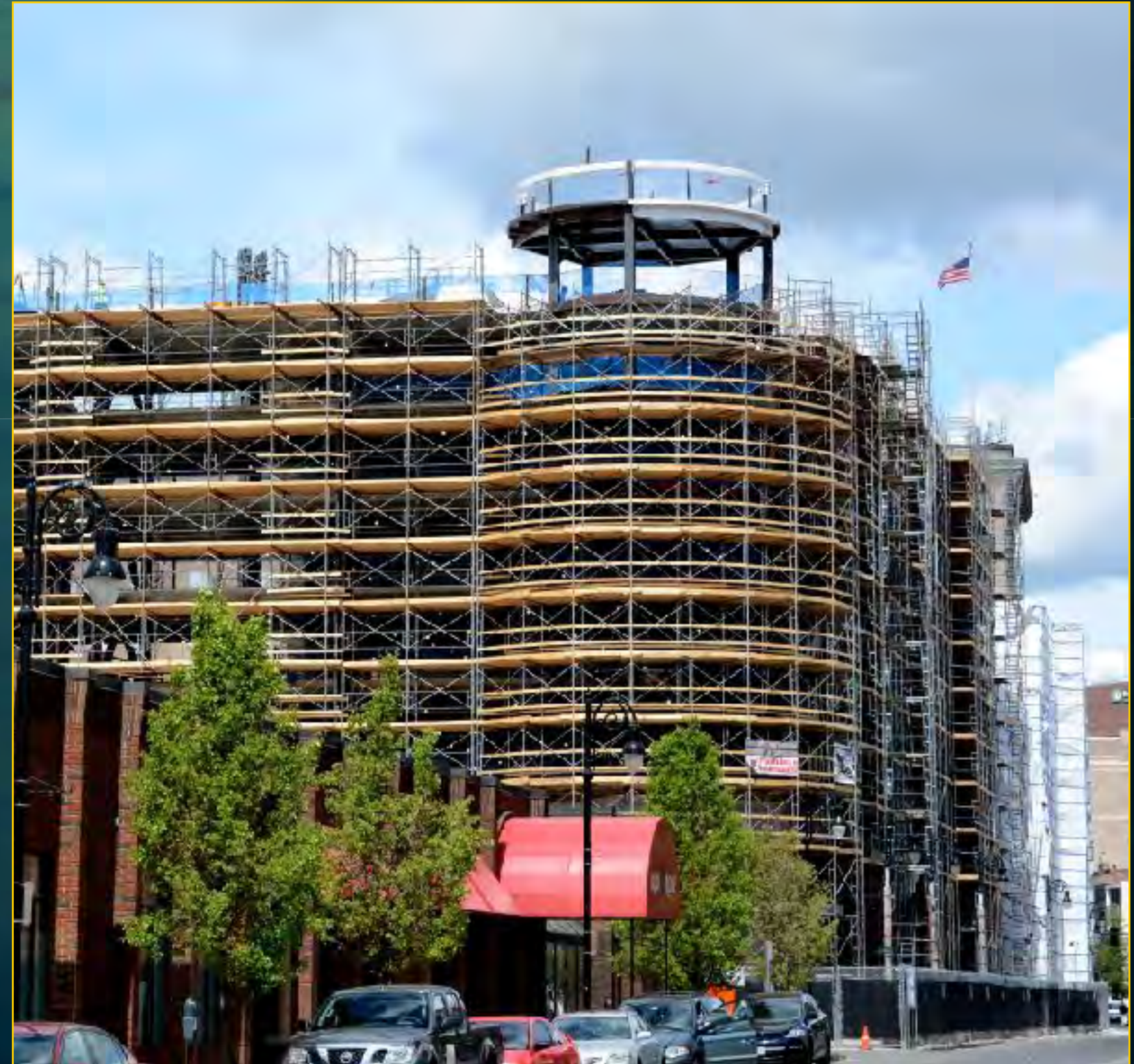
Hotel Construction - May 12, 2017
