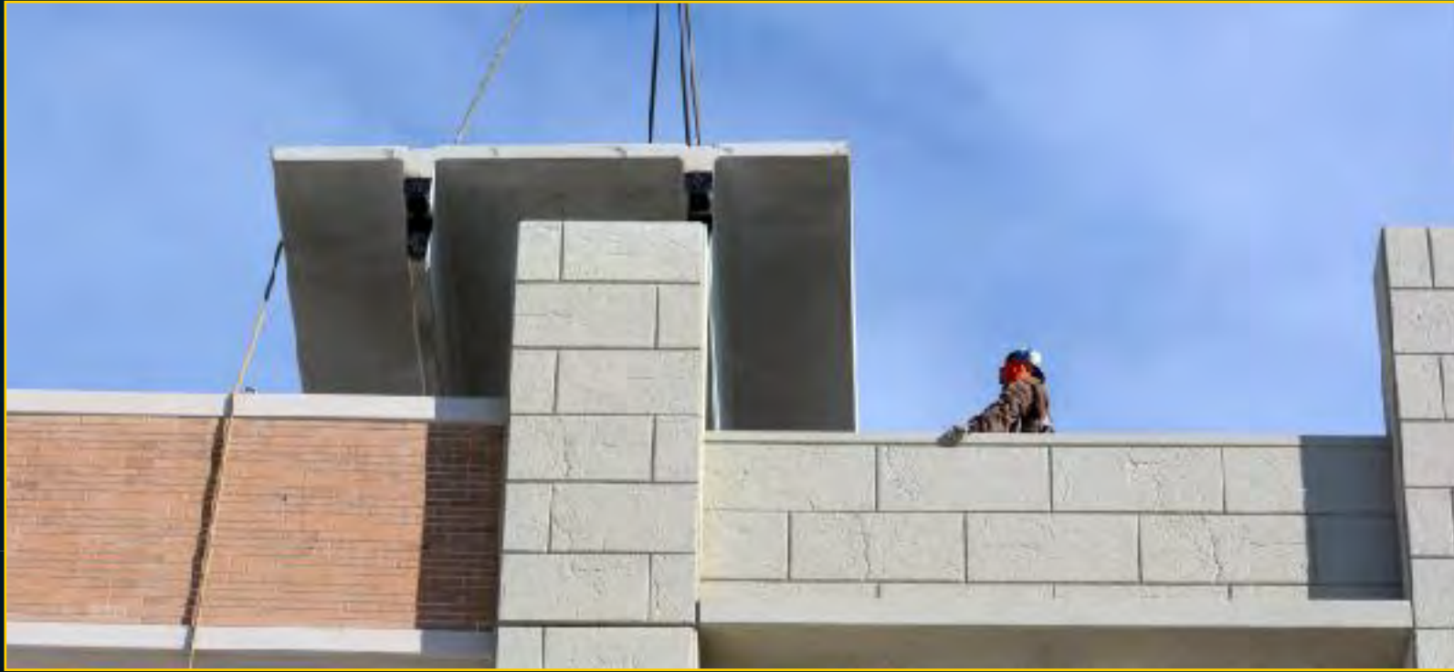
Garage Construction - February 6, 2017
