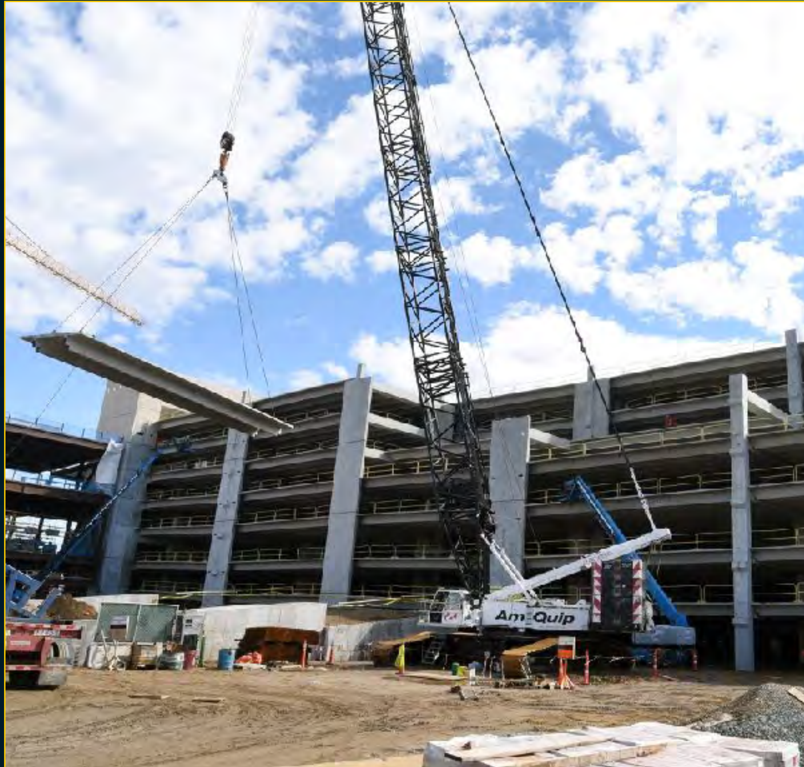
Garage Construction - March 8, 2017
