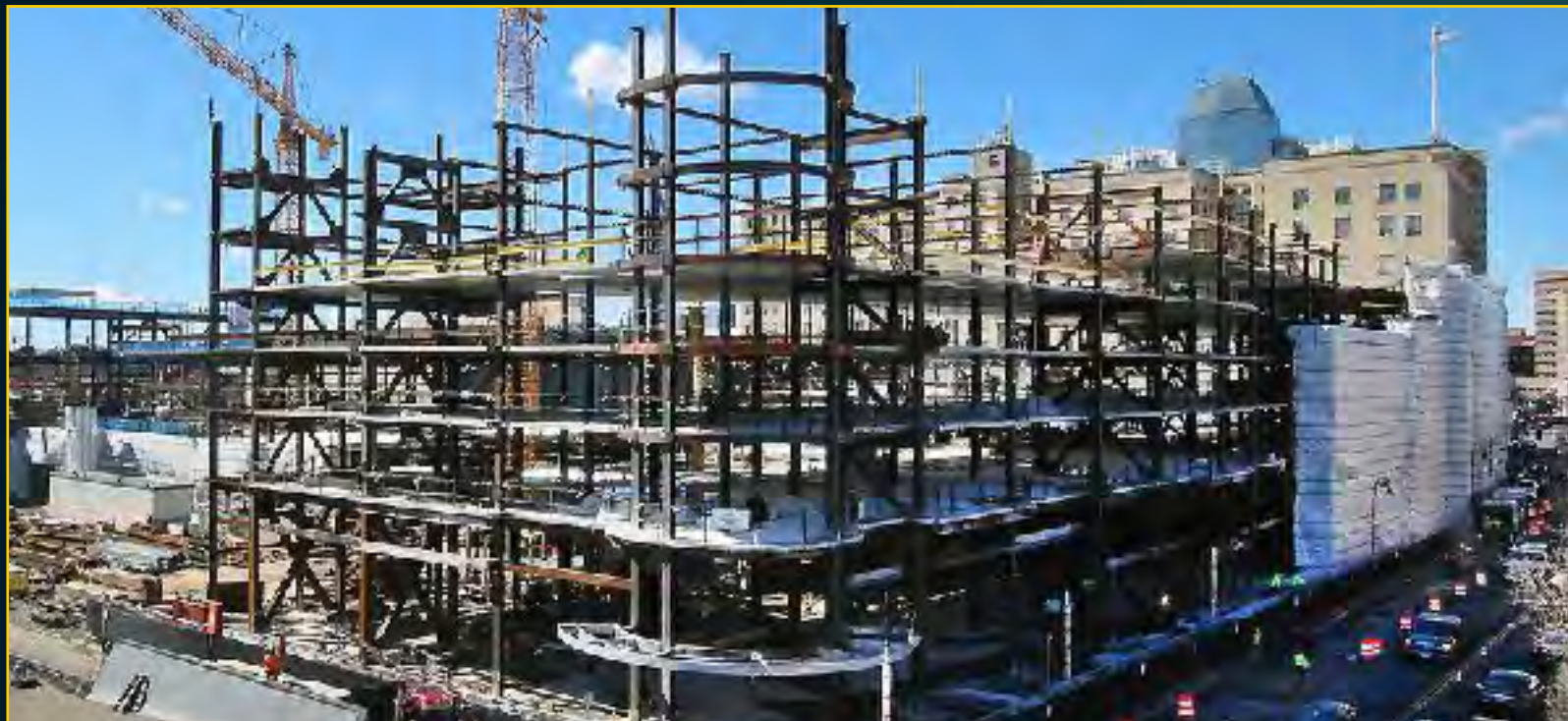
Hotel Entrance - March 8, 2017
