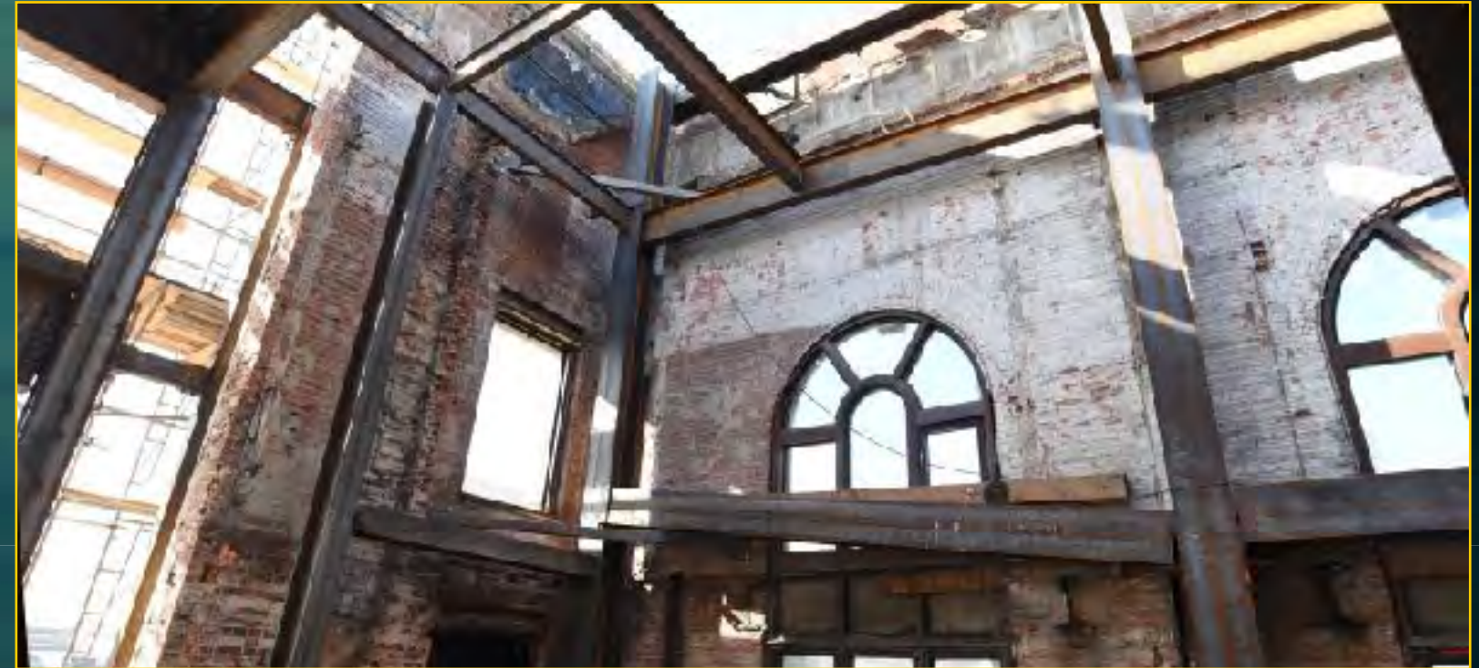
Hotel Construction - February 8, 2017
