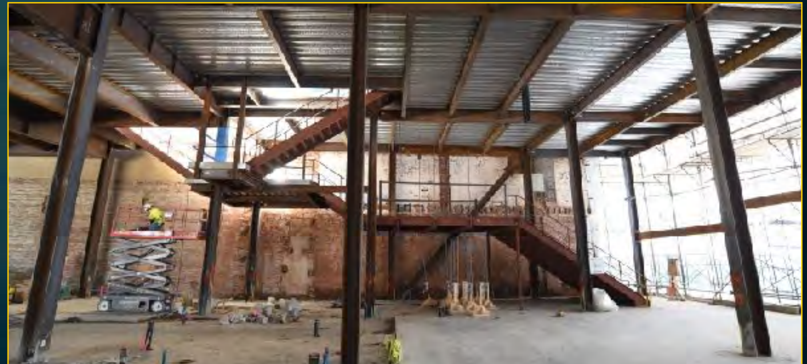
Hotel Construction - February 7, 2017
