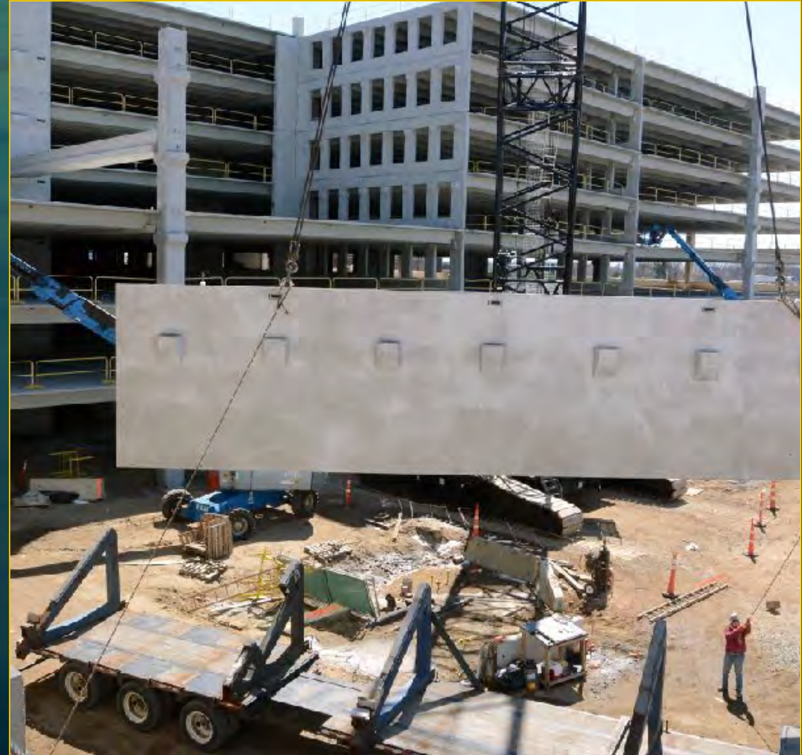
Garage Construction - March 28, 2017
