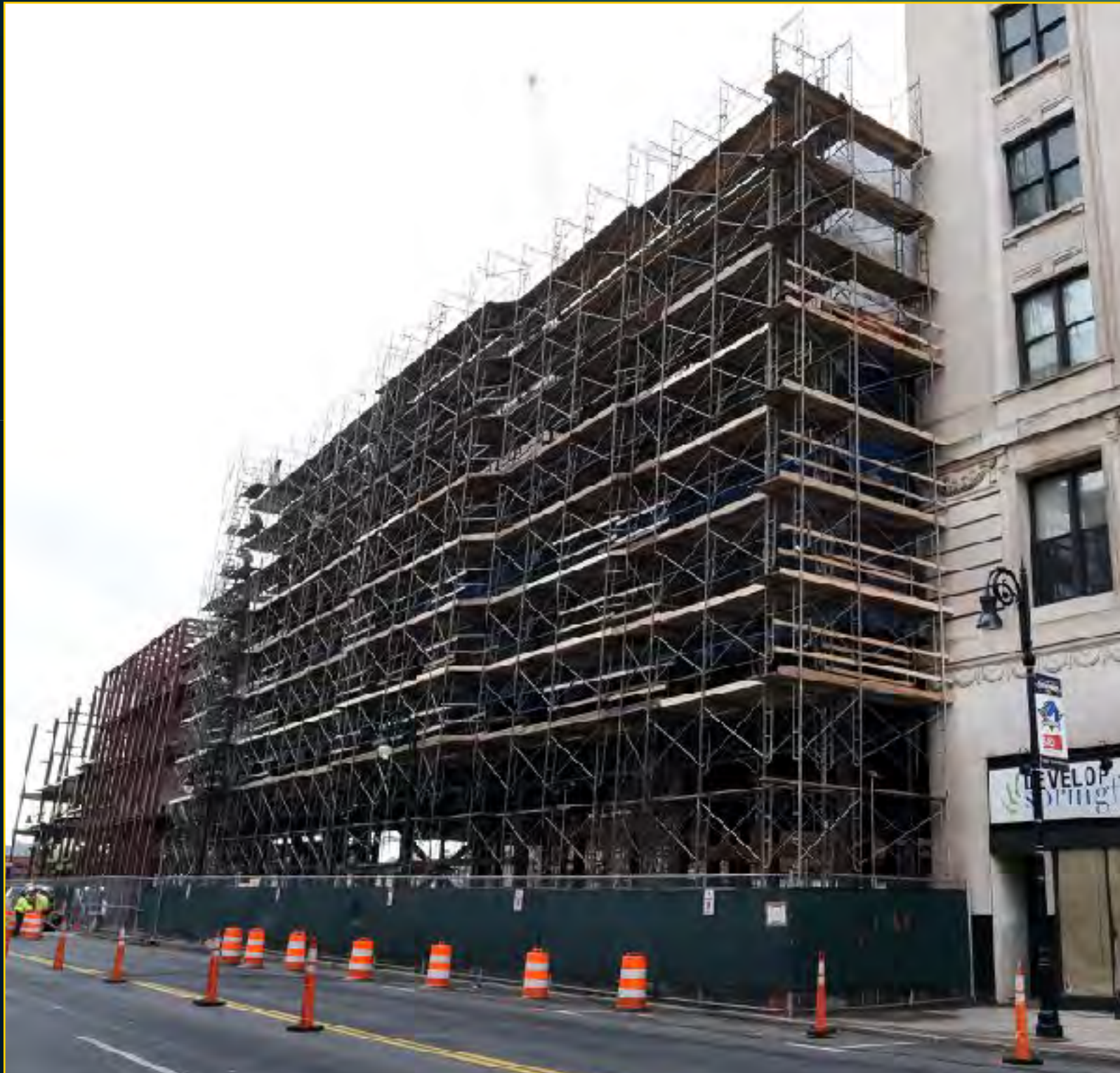
Main Street Scaffolding - January 19, 2017
