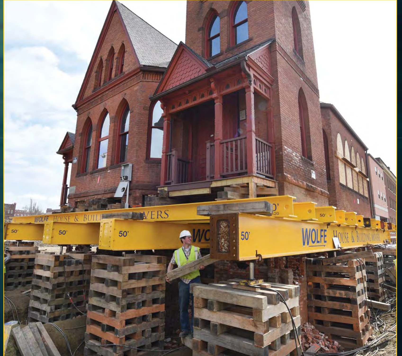
Lifting Church for relocation - March 31, 2016
