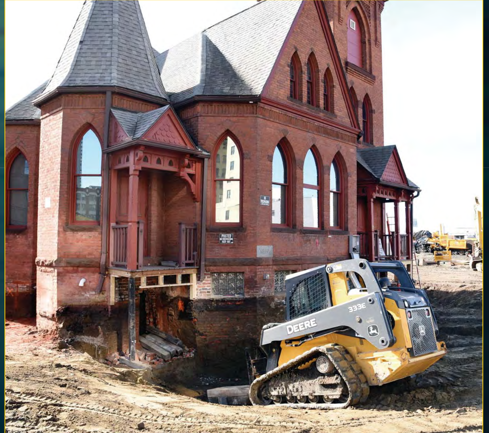
Clearing soil from Church foundations - March 16, 2016
