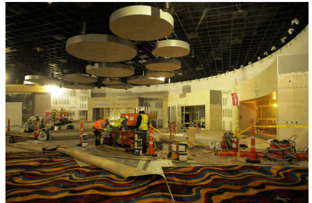
Laying Carpet at Food Court
