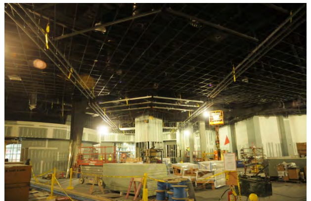
Framing for ceiling Chevrons Toward Casino
