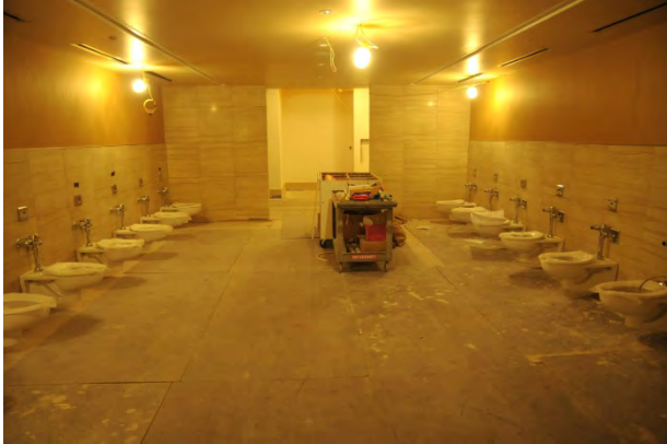
Women's Restroom Adjacent to Stage Area
