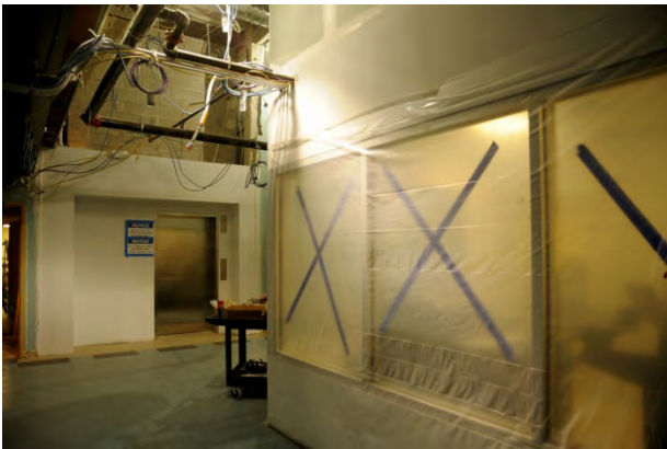
New Elevator Lobby at Track GM Office
