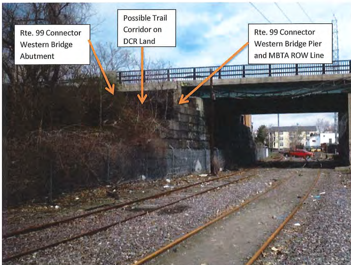
Figure 3 - Route 99 Connector Overpass
