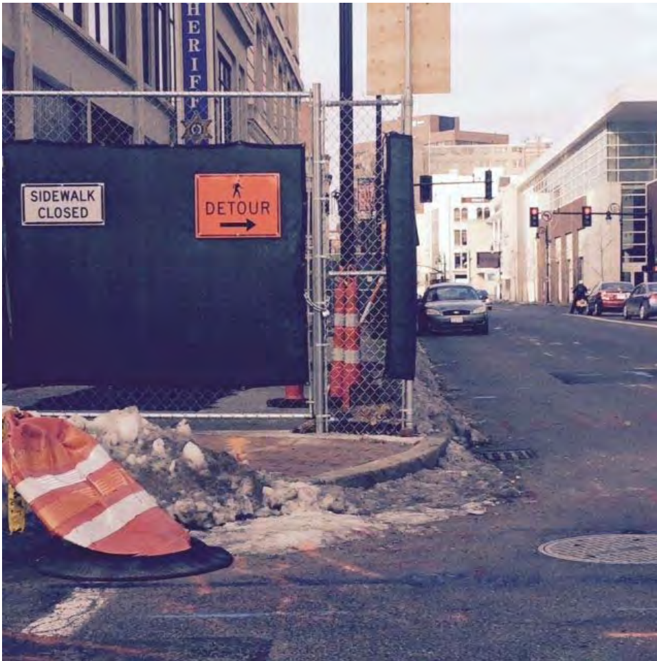
Figure 3. Main Street sidewalk is closed. The pedestrian detour sign directs people to walk in the street. This illustrates a street corner blocked by construction, snow and ice, with no handicap access.
