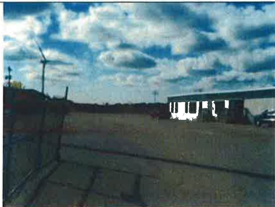
Modular office building shown at the right.
