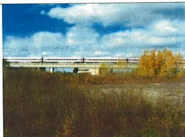
View looking the MBTA rail line along the subject's northern bound
