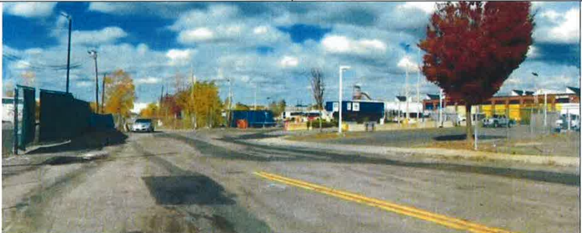
View looking at site at the end of Chemical Lane from Route 99. The MBTA facility is to the right foreground
