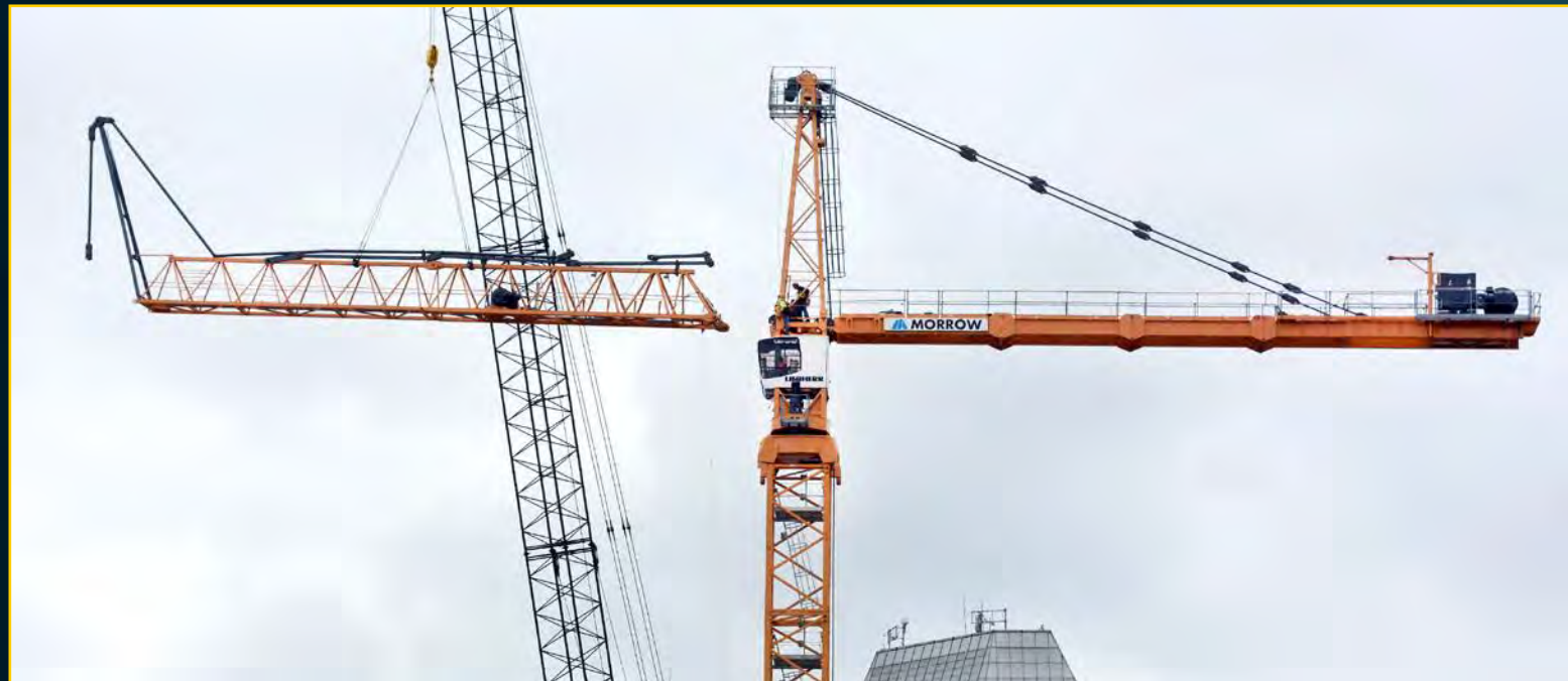
Crane Erection - September 28, 2016
