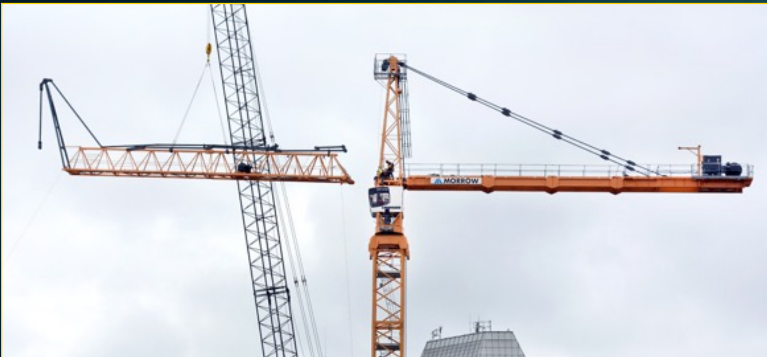
Crane Erection - September 28, 2016
