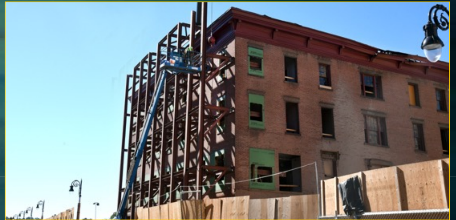
Union Chandler Facade Stabilization - August 22, 2016
