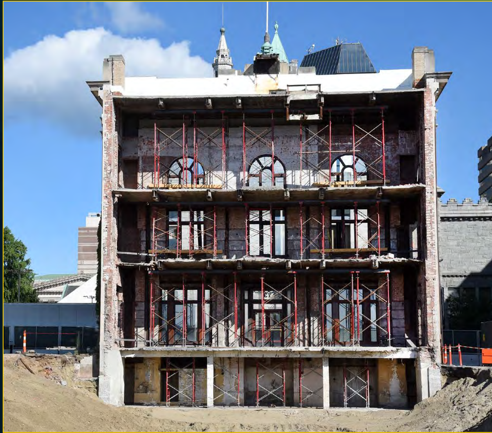
73 State Street Completed Facade Demo - July 19, 2016
