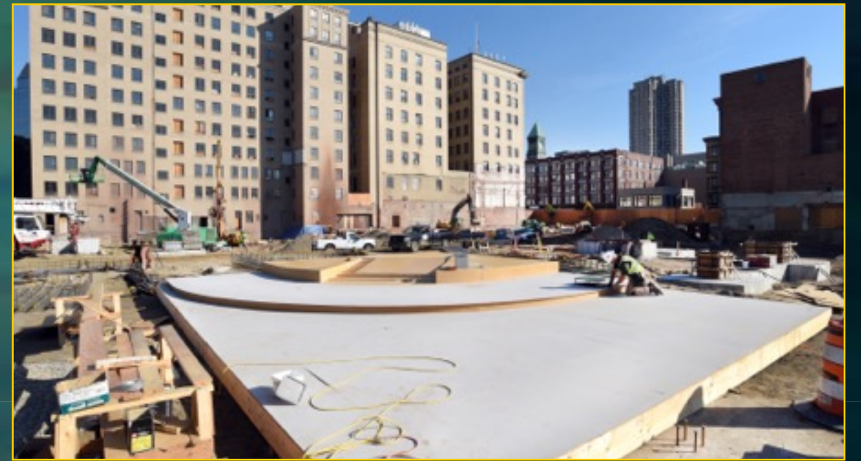
Podium Construction - July 28, 2016
