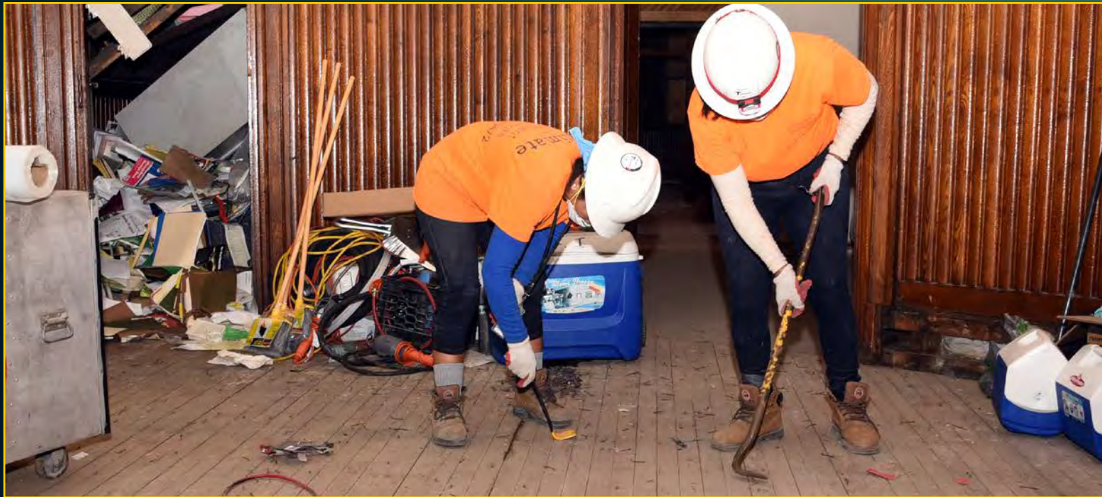
Armory Abatement - September 12, 2016
