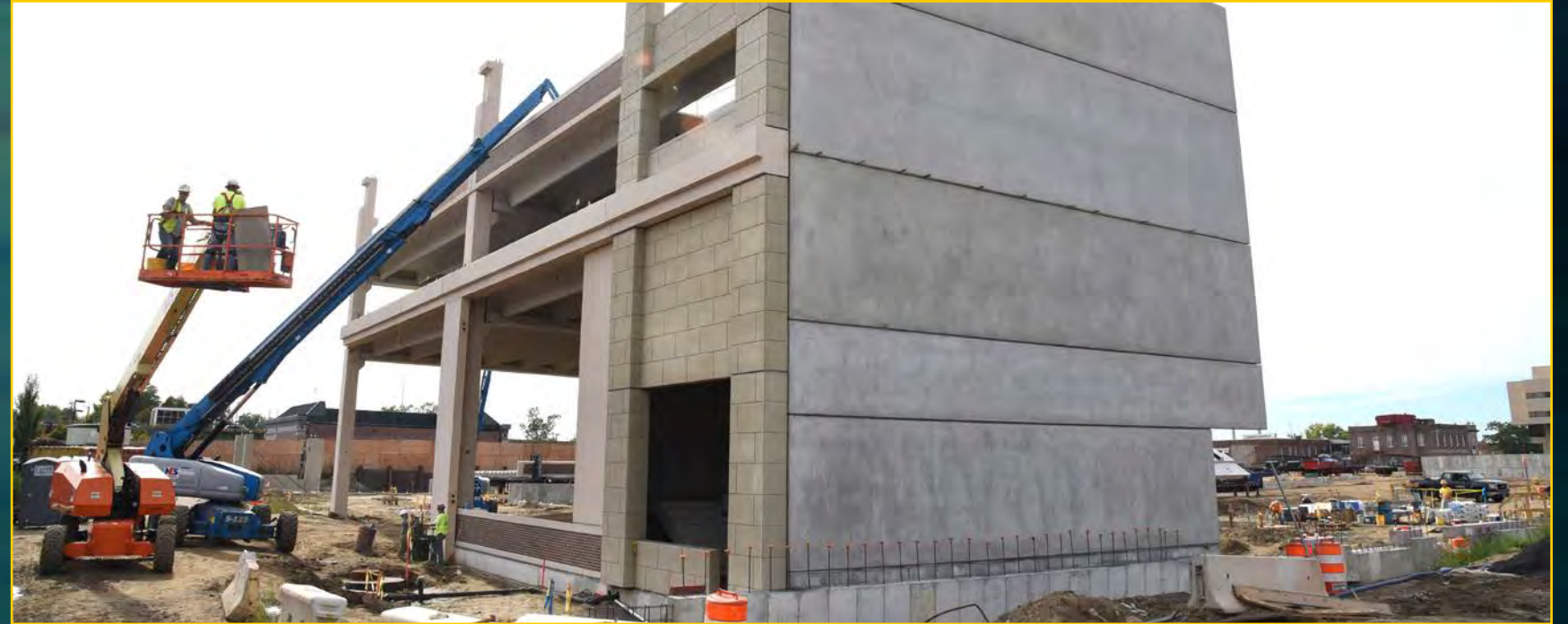
Garage Construction - September 22, 2016
