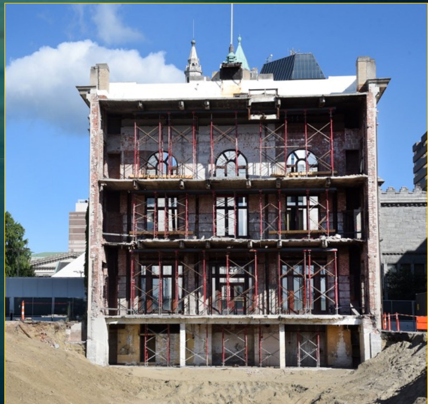
73 State Street Completed Facade Demo - July 19, 2016
