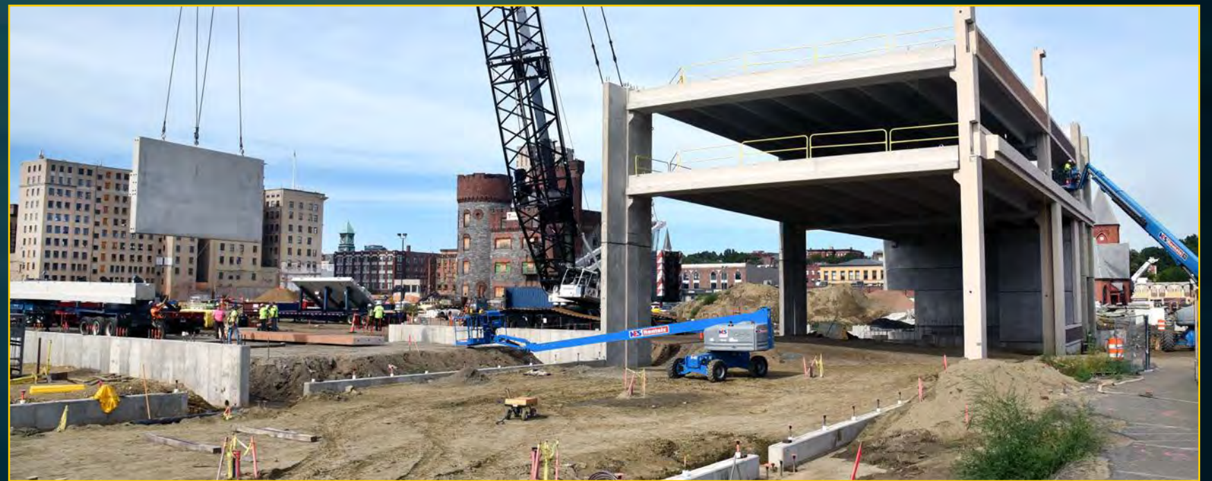
Garage Construction - September 22, 2016
