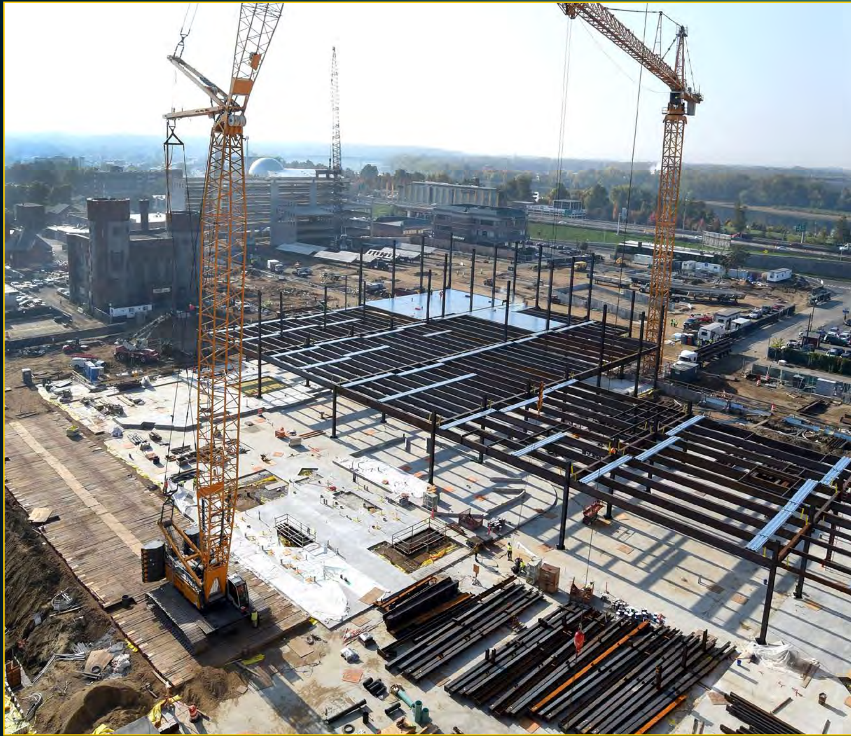
Podium Steel - October 18, 2016
