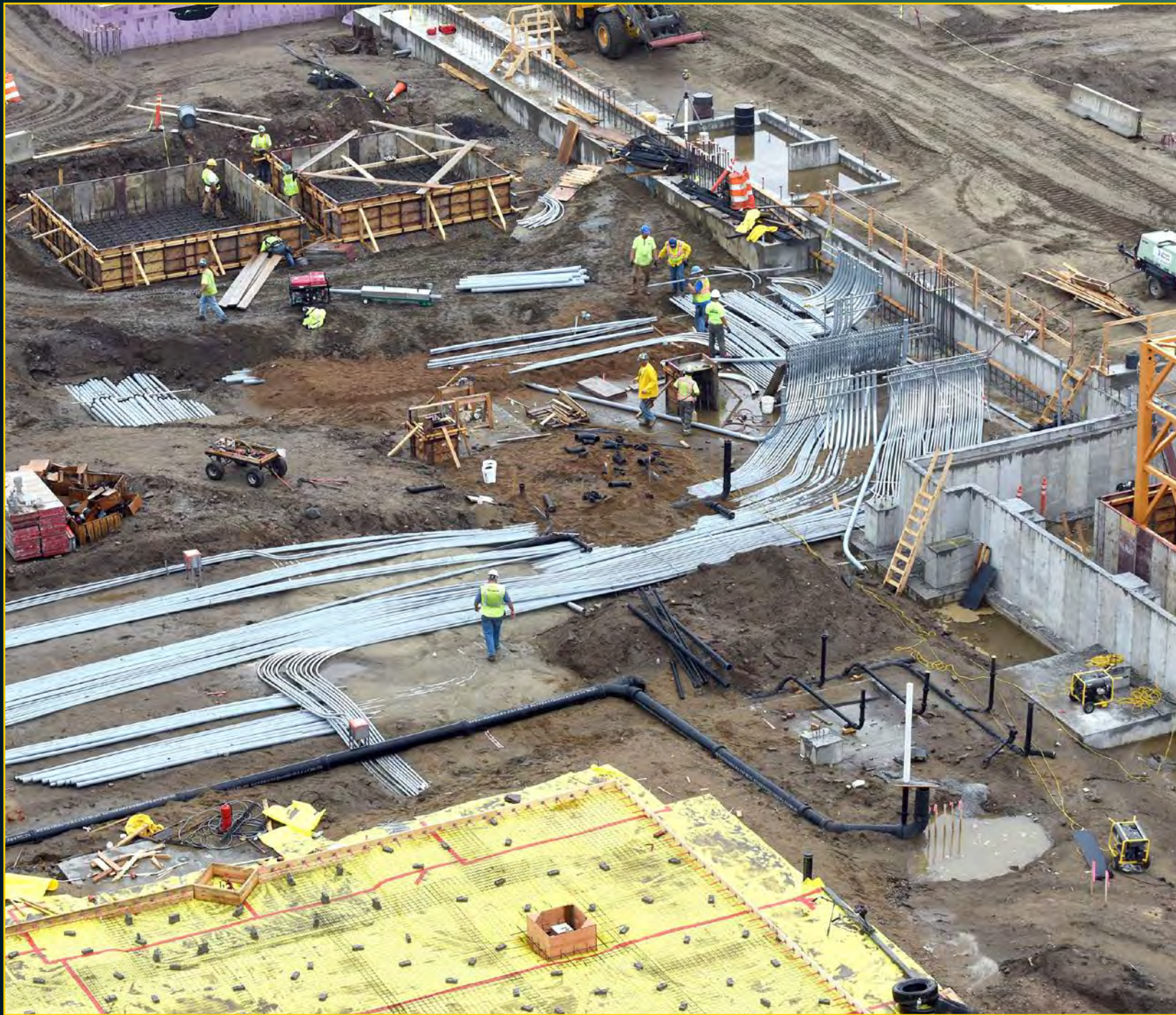
Podium Construction - September 1, 2016
