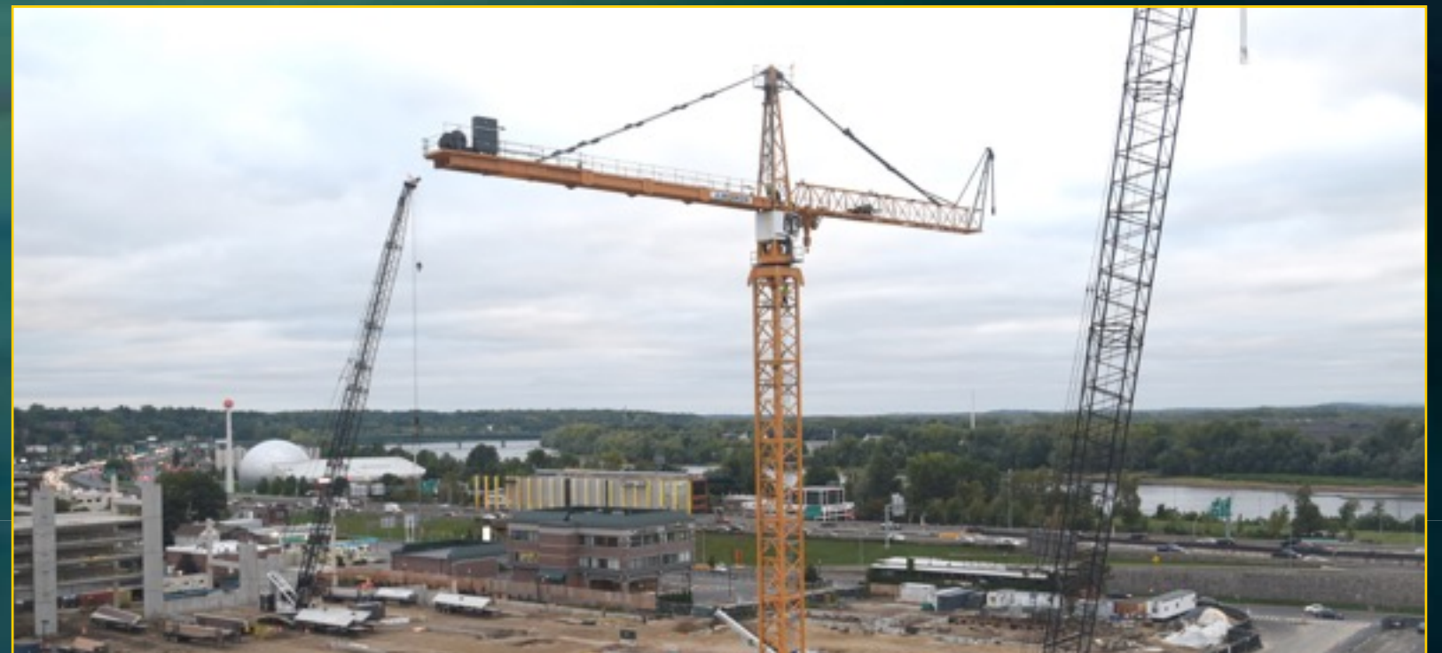
Crane Erection - September 29, 2016
