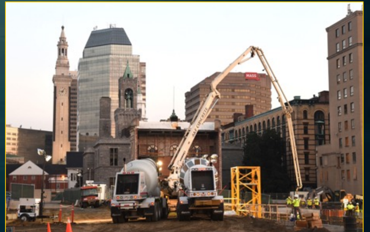
Foundation Construction - August 13, 2016
