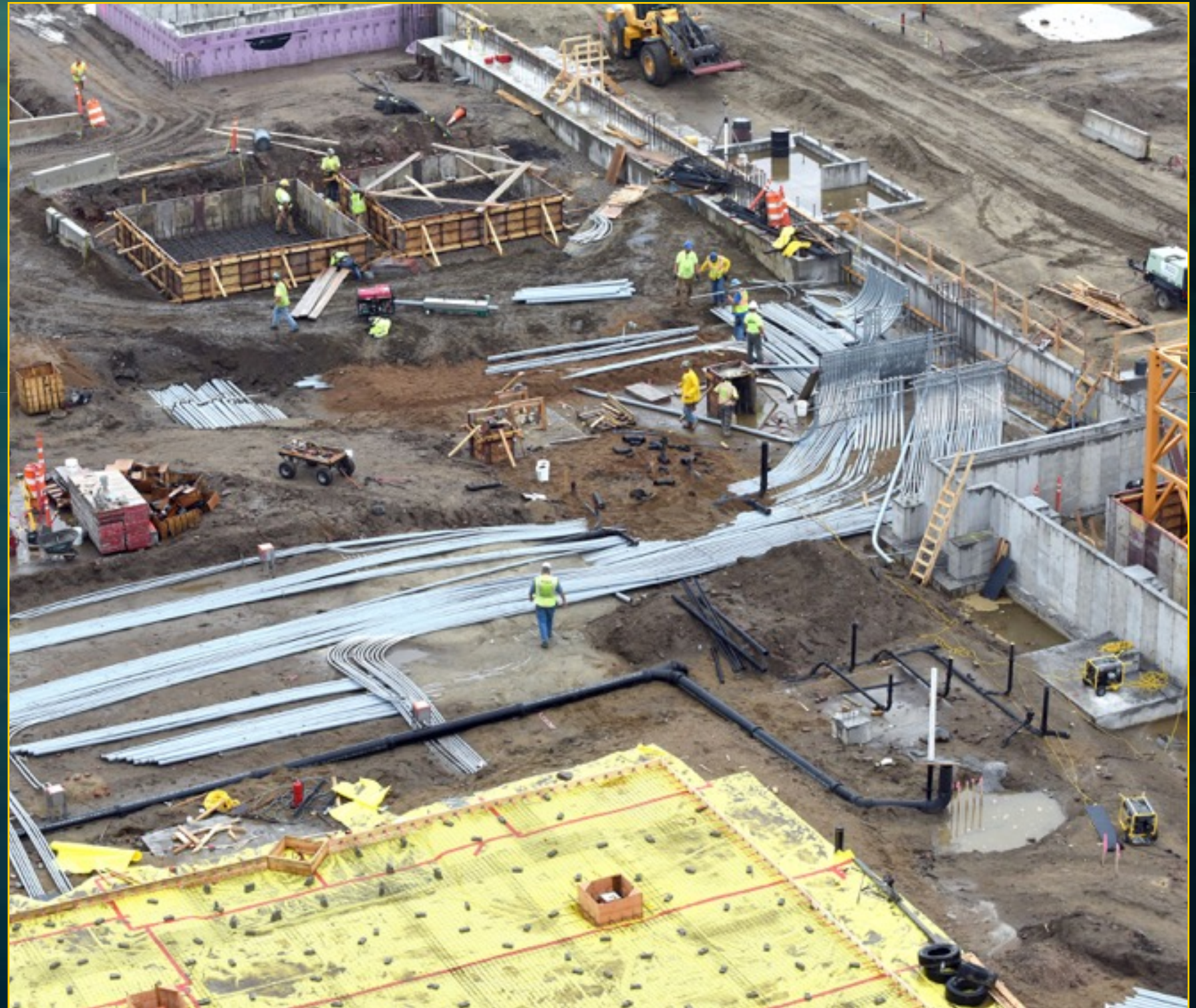
Podium Construction - September 1, 2016
