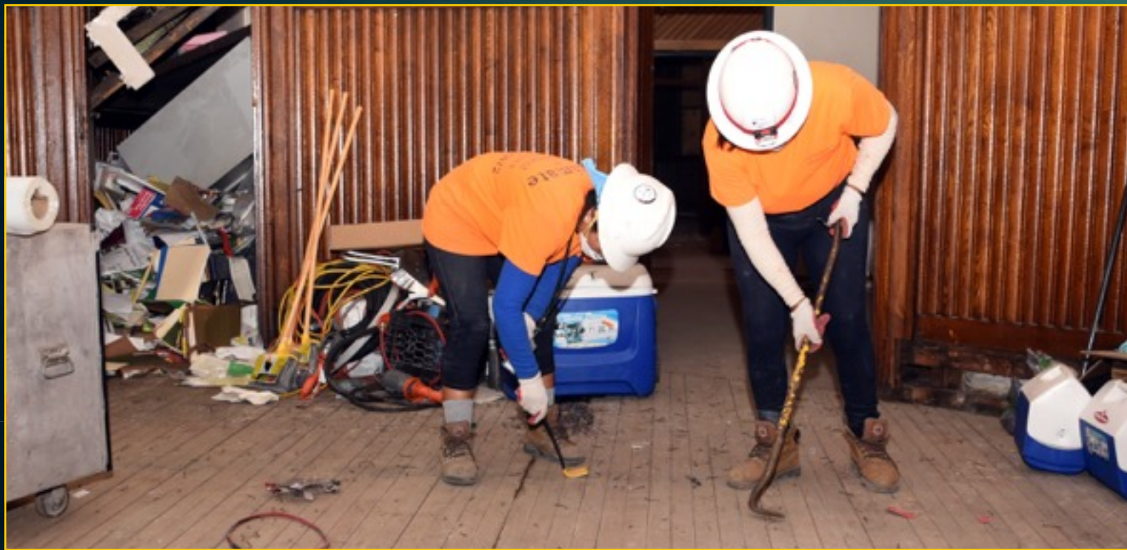
Armory Abatement - September 12, 2016
