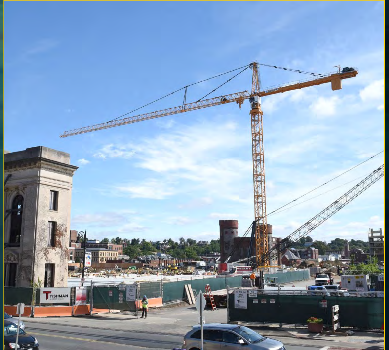
Crane Erection - September 29, 2016
