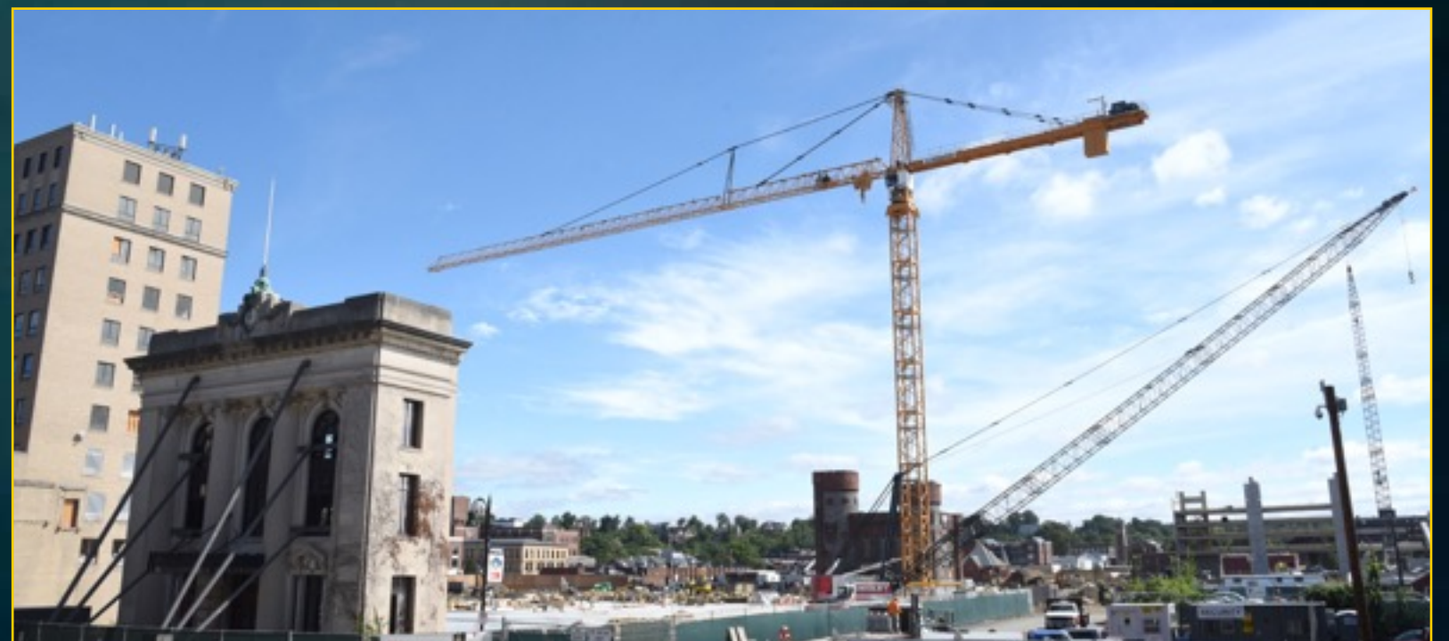
Crane Erection - September 29, 2016
