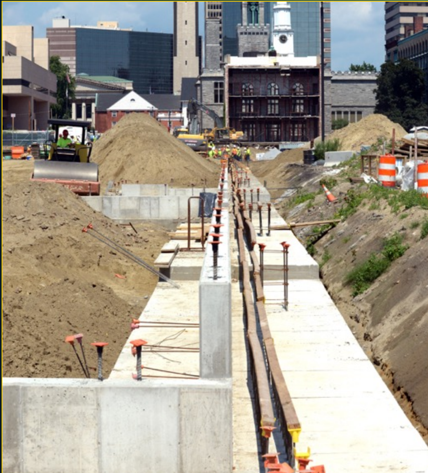
Garage Construction - July 13, 2016
