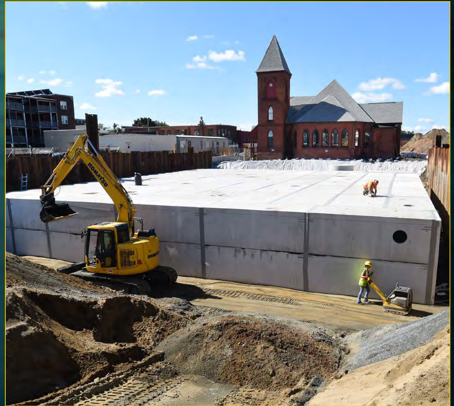
Stormwater Retention - September 2, 2016
