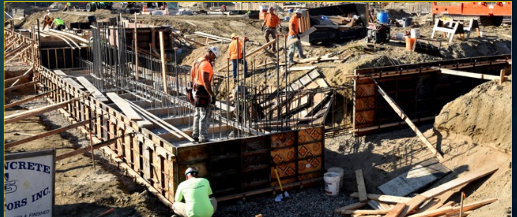
Garage Construction - July 18, 2016
