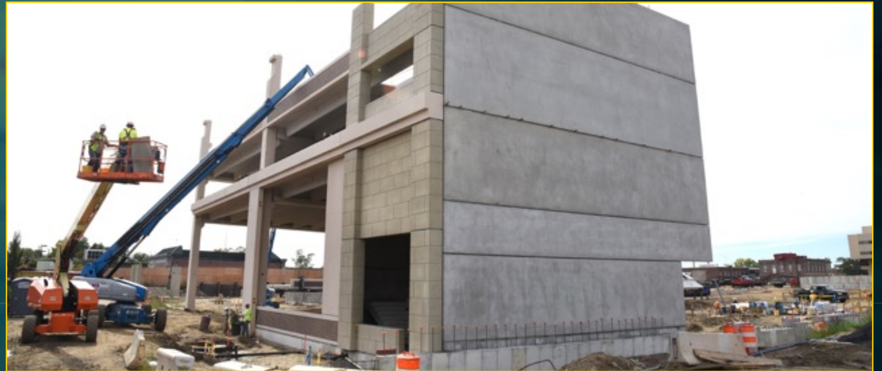
Garage Construction - September 22, 2016
