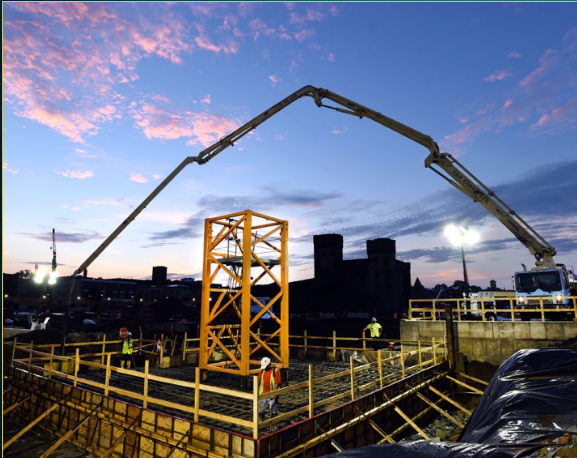
Foundation Construction - August 13, 2016
