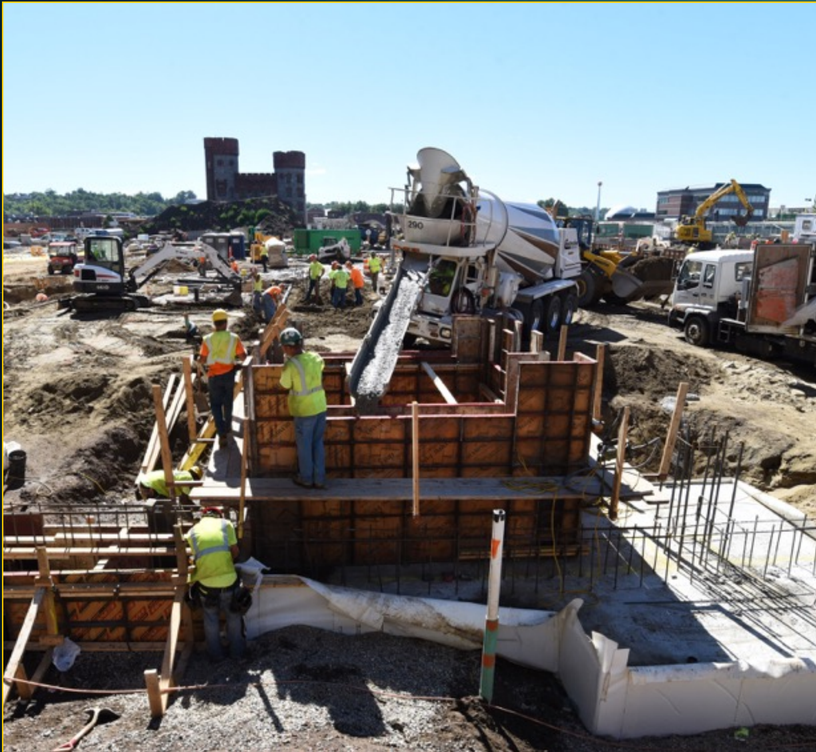
Podium Construction - August 22, 2016
