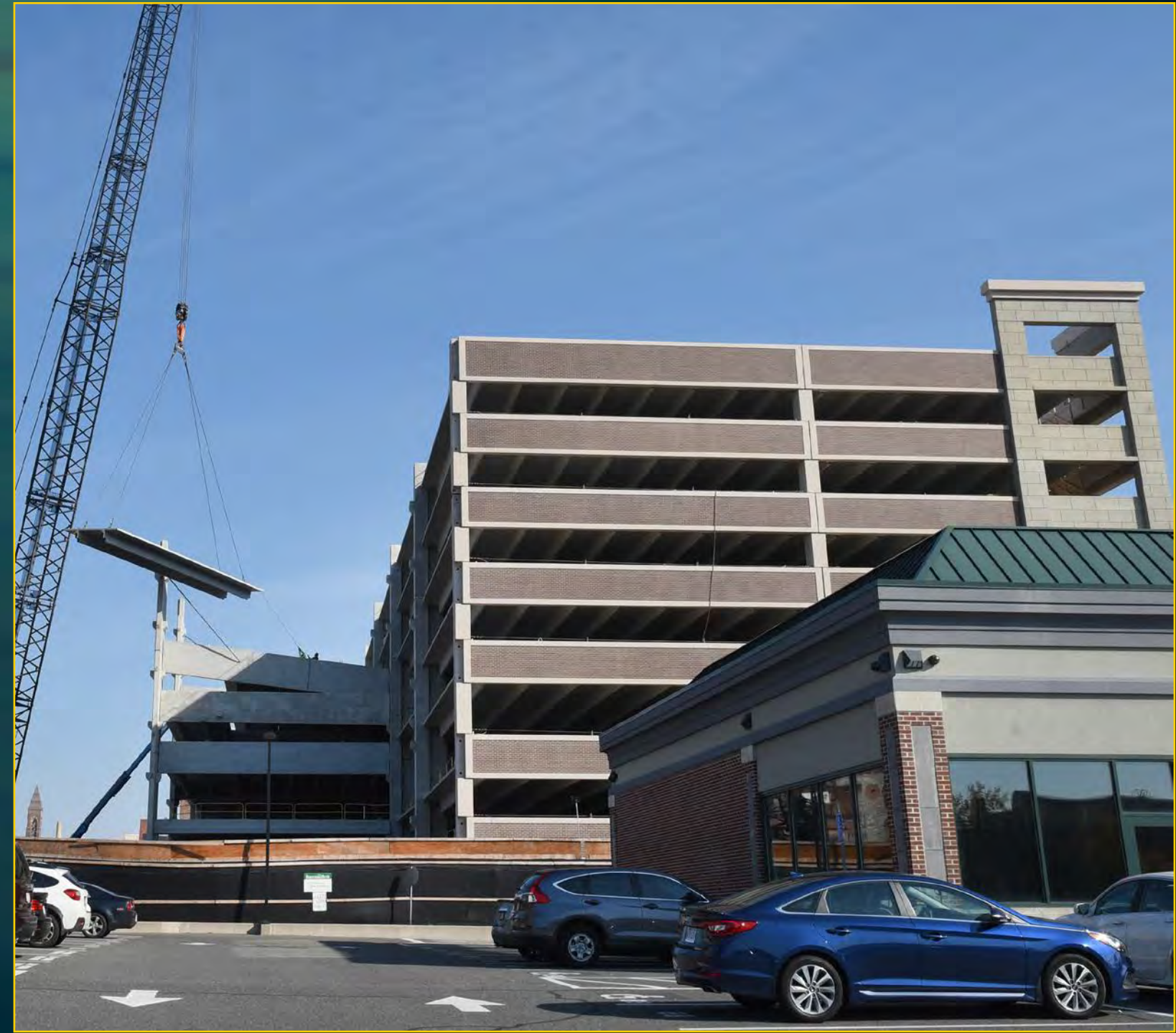
Garage Progress - November 2, 2016
