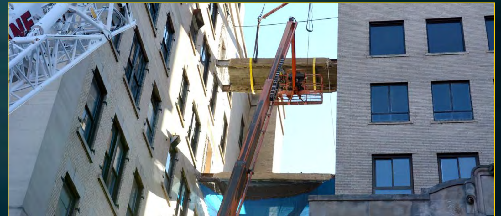
Pedestrian Bridges Demolition - November 19, 2016
