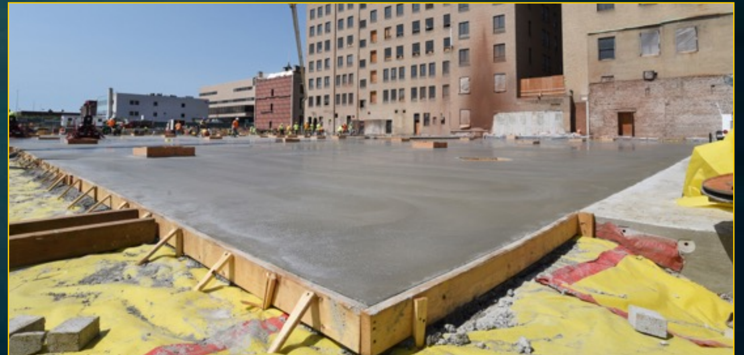
Podium Construction - August 24, 2016
