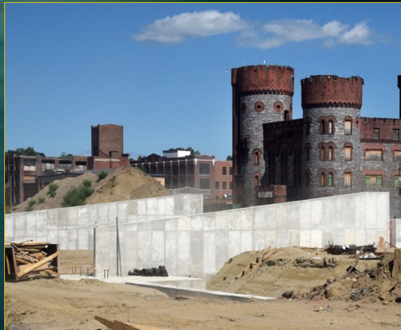
Garage Construction - August 29, 2016
