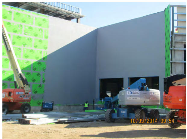
INSTALLATION OF AVB ON EXTERIOR WALLS
