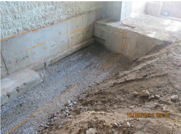
EXCAVATION FOR FOOTINGS AT STAIR 9
