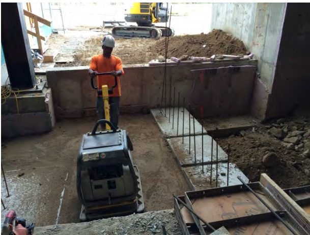
BACKFILLING AT STAIR 9 FOOTINGS
