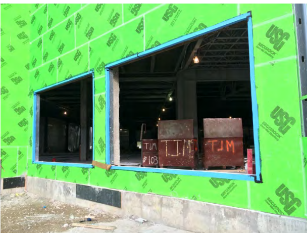
DETAILING OF AVB AT EXTERIOR WINDOWS
