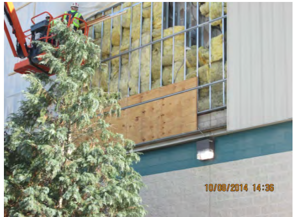
INSTALLATION WALL BLOCKING FOR SIGNAGE
