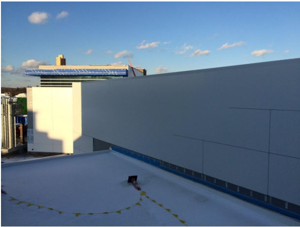
West Side of Casino Exterior Wall in Progress of Being Caulked
