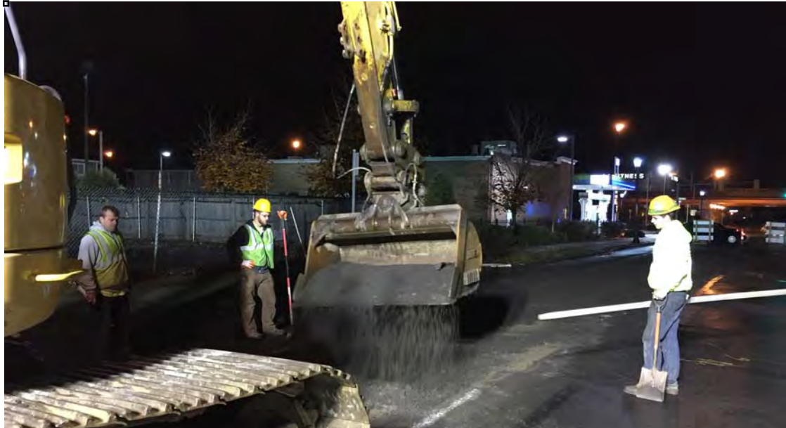
11/13/15 Offsite Utilities - Patching Union Street
