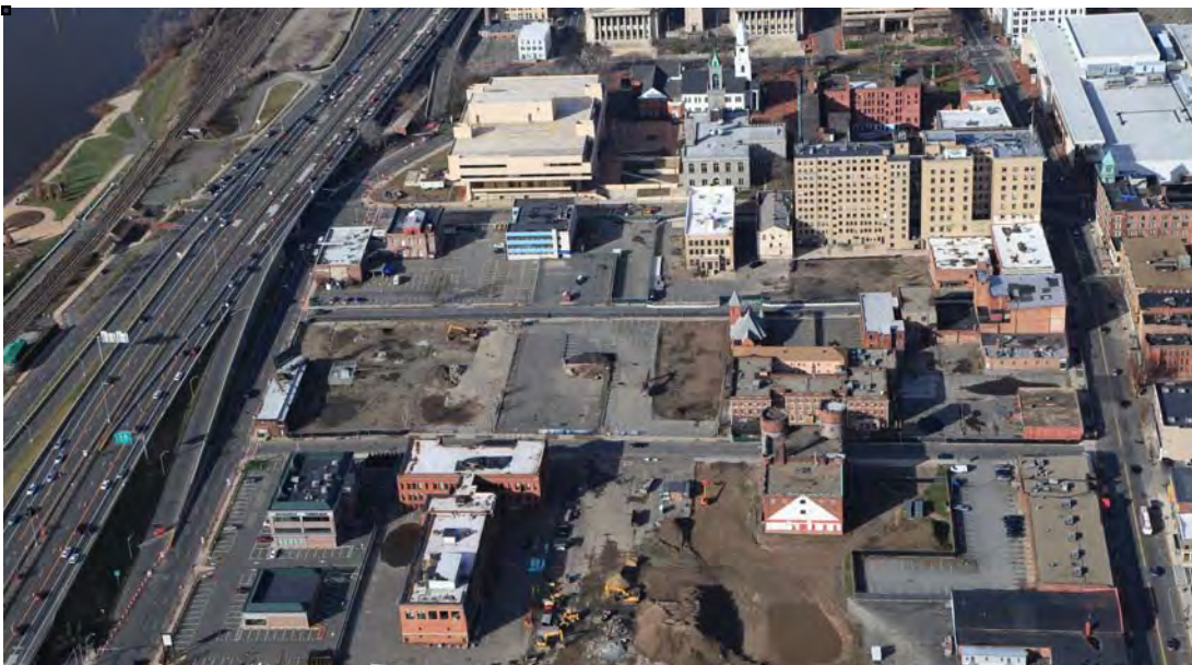
12/26/15 Site Aerial Showing Church Haul Road Progress.
