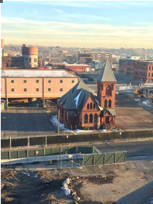
French Church Ready for Relocation
