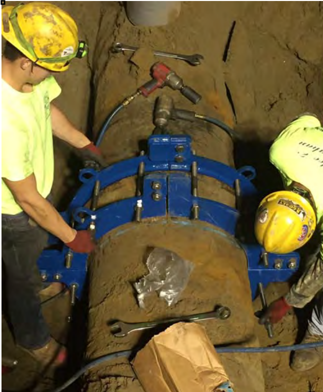
11/10/15 Offsite Utilities - Union Street
