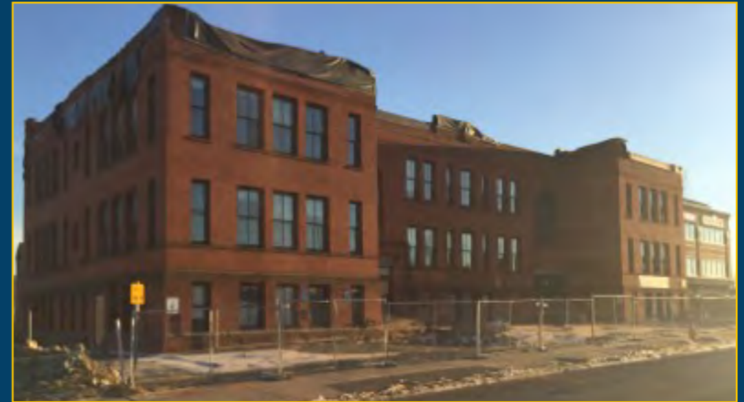
Zanetti School ready for demolition
