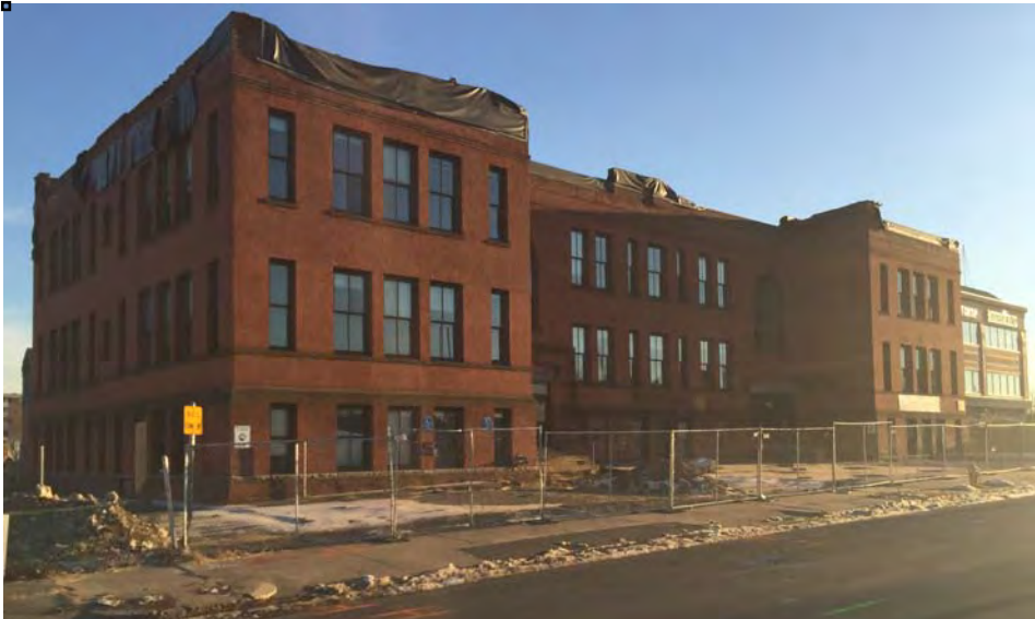
Zanetti School Ready for Demolition Planned for 1/11/16
