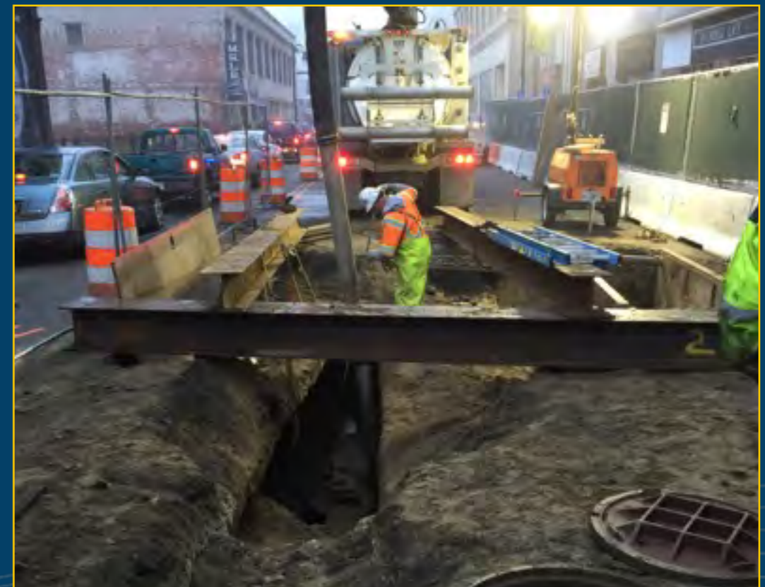
Roadway utility work
