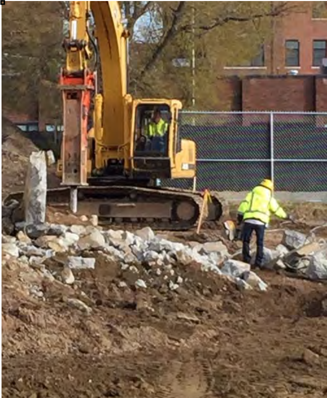
12/1/15 French Church Haul Road Construction
